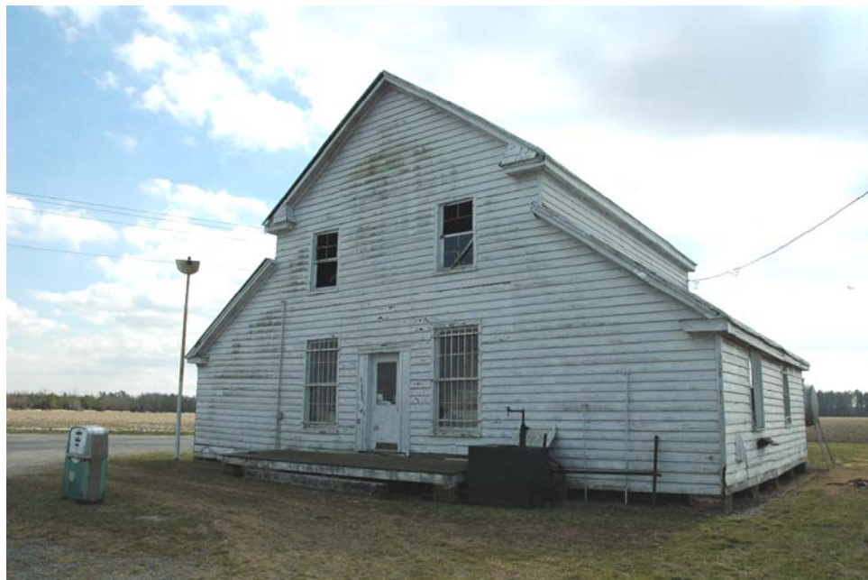
Figure 62: Store, Intersection Mill Swamp Road and Sycamore Cross Drive (046-5149).
