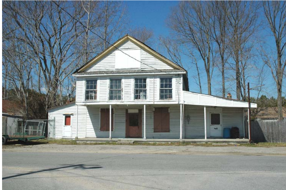
Figure 61: Store, 21155 Reynolds Drive (046-5172).
