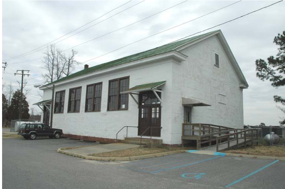
Figure 73: Carrsville Elementary School Gymnasium (046-5200).
