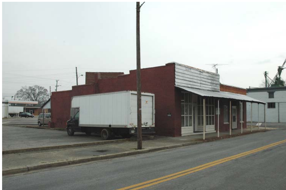
Figure 65: Store, West N&W Street (328-5002).
