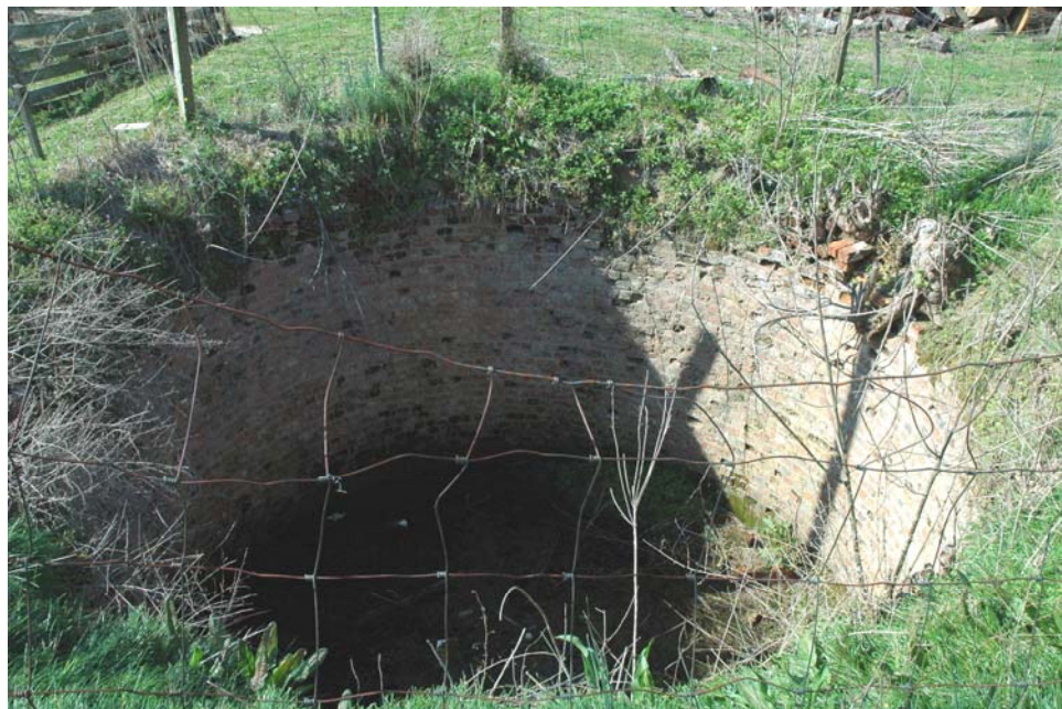
Figure 14: Ice House foundation at Strawberry Plains (046-5233).
