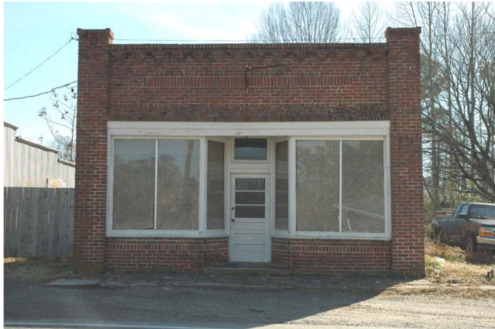
Figure 81: Store, Walters Highway in Walters (046-5123).
