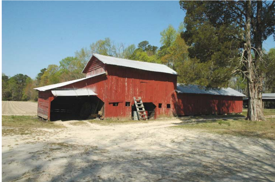
Figure 47: Barn at Farmhouse, 14200 Raynor Road (046-5235).
