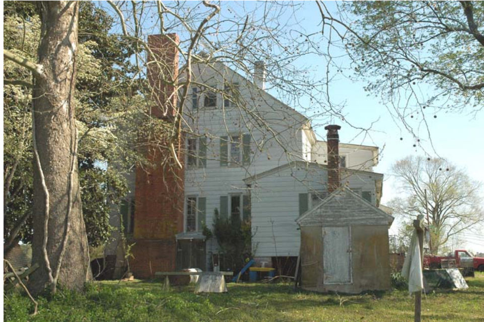
Figure 8: Marshall-Edwards House (046-5236), view of side elevation with chimney.
