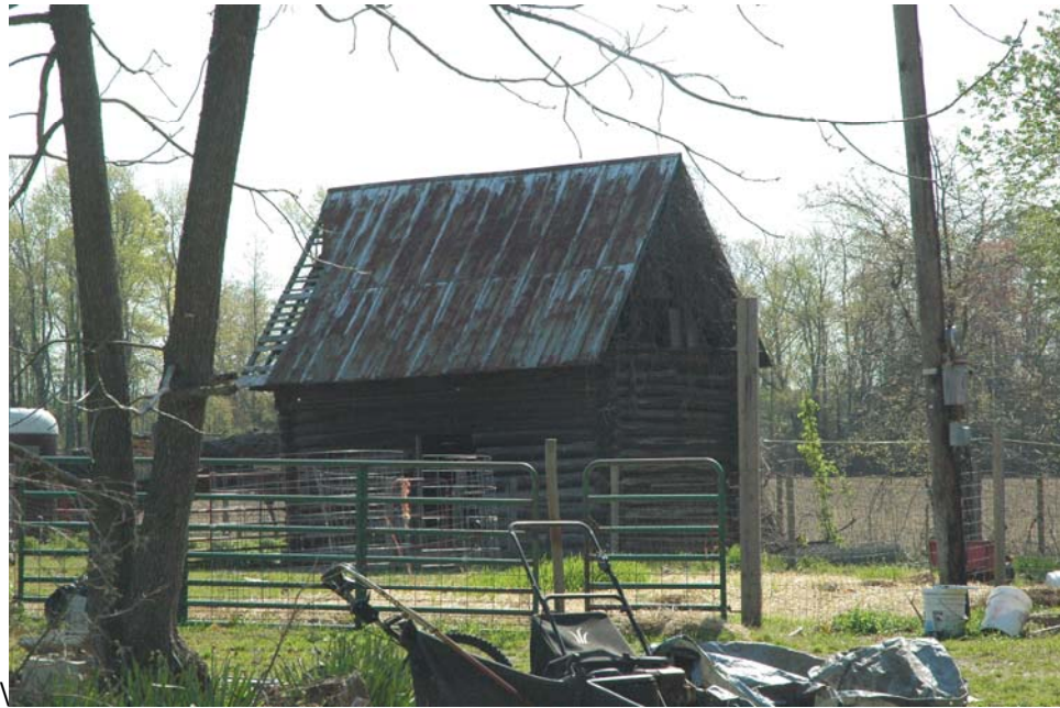
Figure 31: Barn at Marshall-Edwards House (046-5236).
