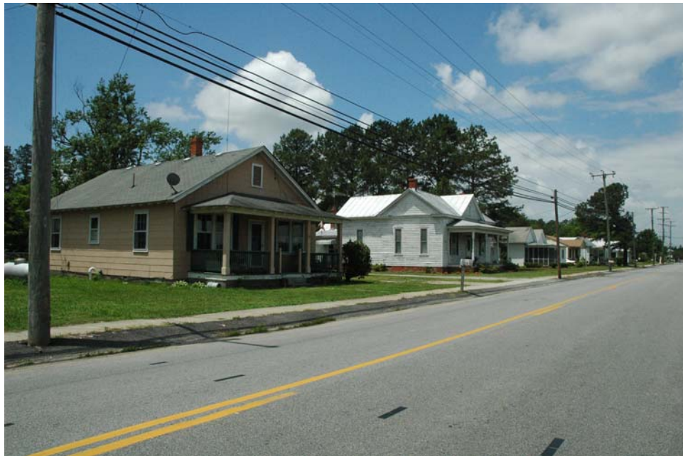
Figure 112: View west on Bank Street in the Windsor Historic District (328-5010).
