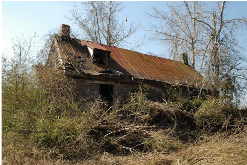
Figure 11: House, Foursquare Road (046-5207)
