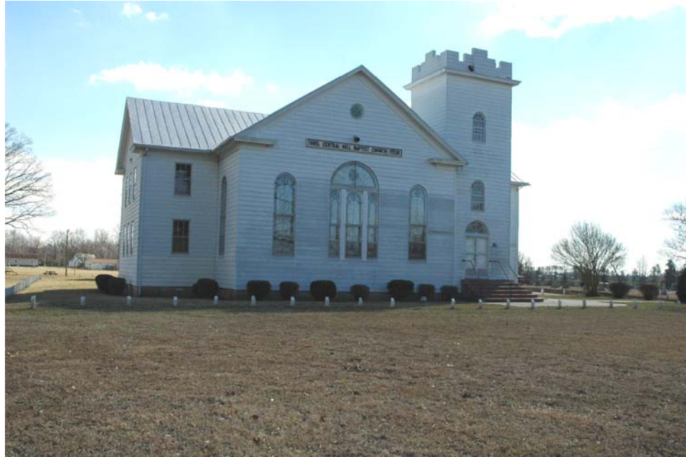
Figure 56: Central Hill Baptist Church (046-5153).
