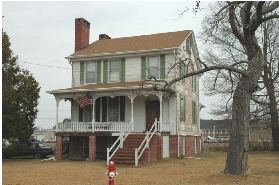
Figure 21: Ashburn, Alexander H. House (328-5004).
