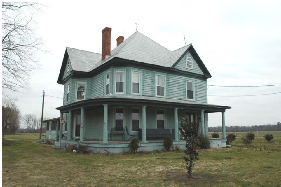
Figure 39: Farmhouse, 27202 Spivey Town Road (046-5194).
