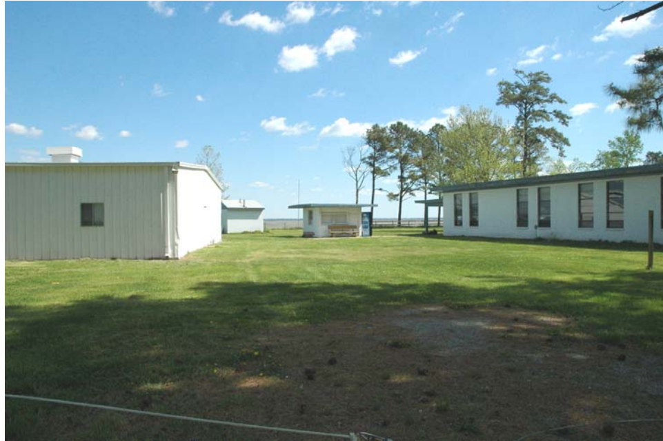
Figure 79: Morgart's Beach Hotel Site (046-5241).
