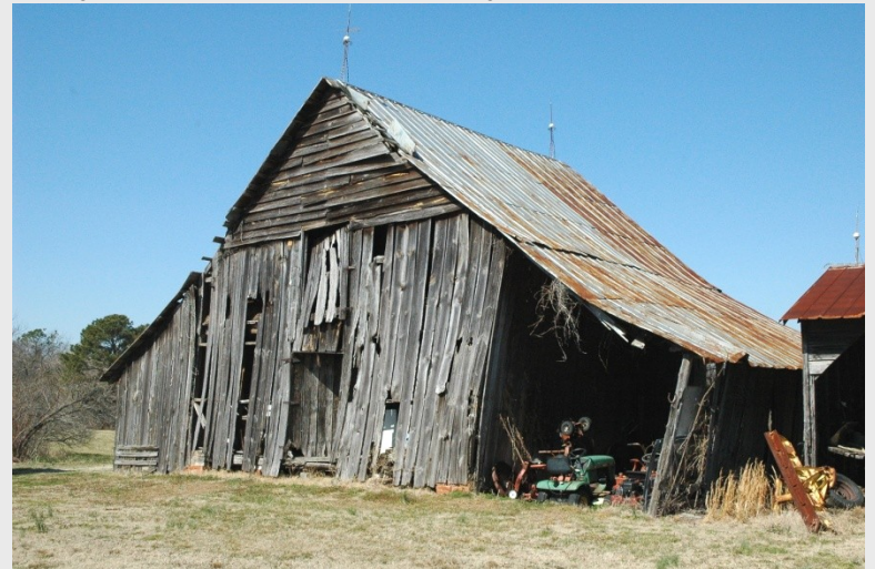
Barn at Edwards House (046-5209)
