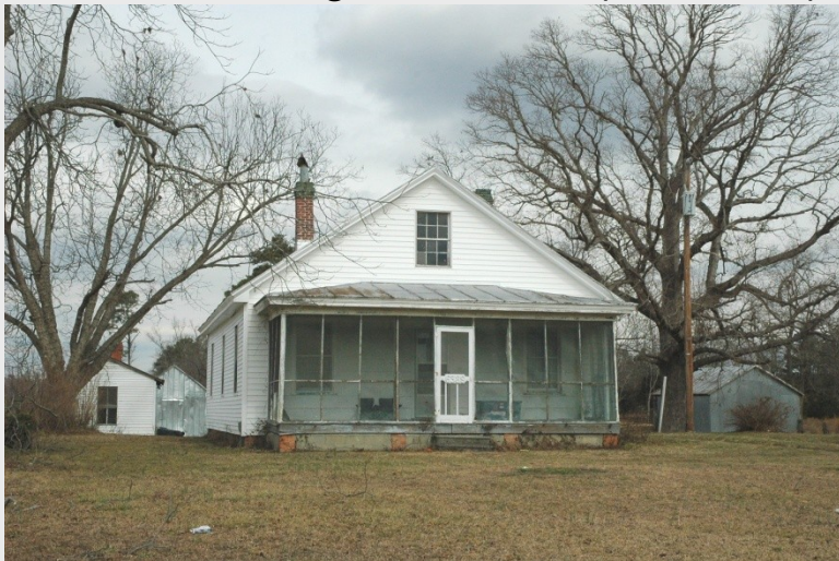
Farmhouse, Barlow Lane (046-5141)
