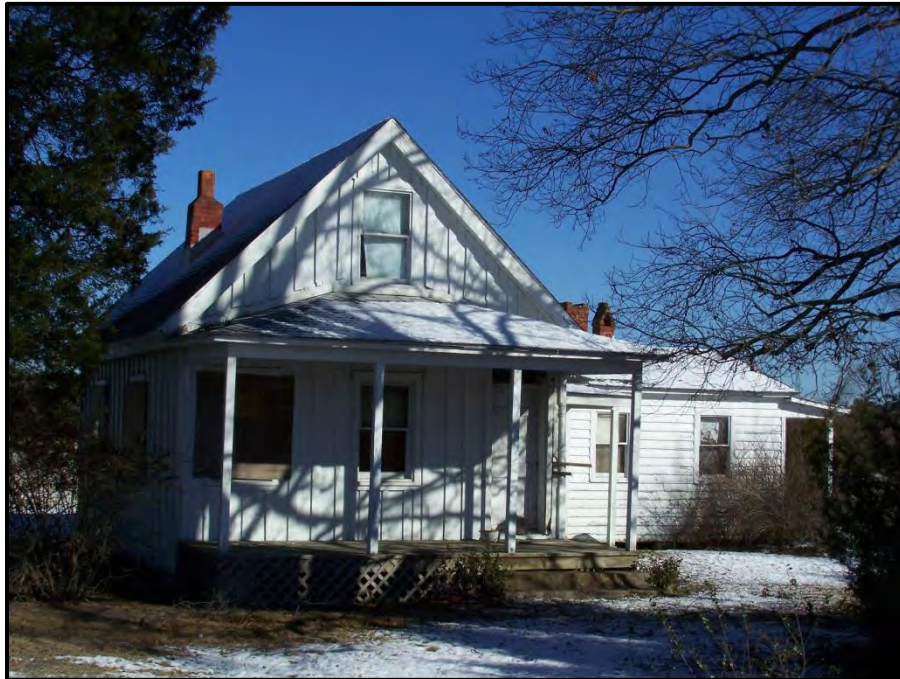
Figure 40. Store (VDHR #050-5034), West River Road, View Looking Northeast.
