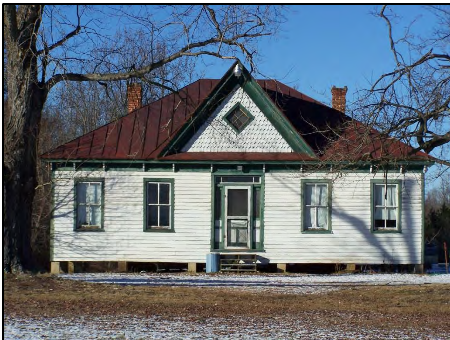
Figure 29. House (c. 1880; VDHR #050-5038), 501 Locust Hill Road, View Looking North.
