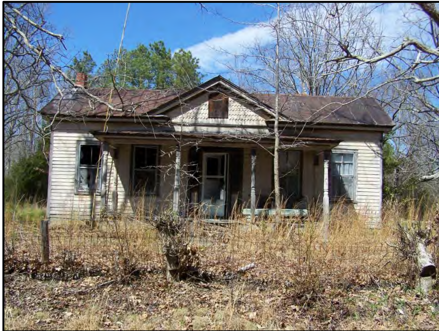
Figure 28. House (c. 1870; VDHR #050-0179), 2 Route 624, View Looking North.
