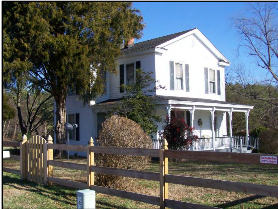
Figure 61. House (c. 1900; VHDR #050-5060), 1342 Etna Mills Road, View Looking Northeast.
