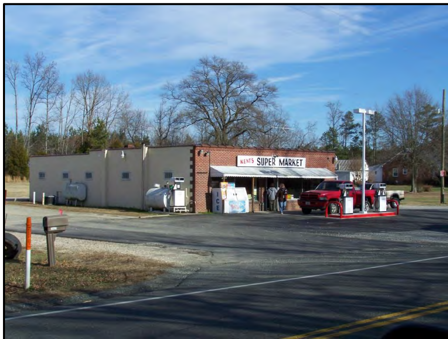
Figure 71. Kent's Super Market (c. 1950; VDHR #050-5065), 20623 King William Road, View Looking East.
