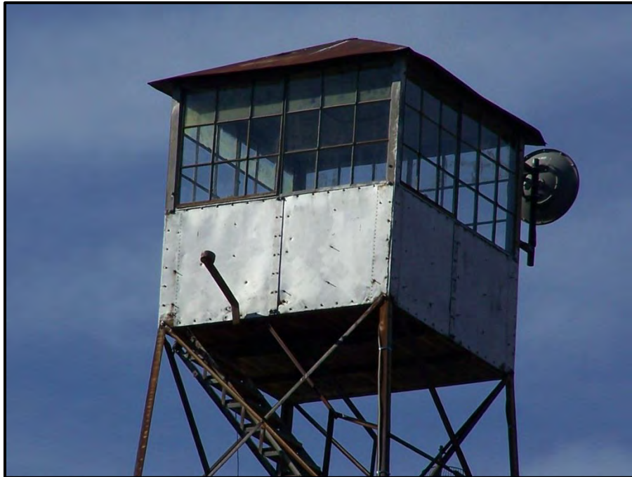
Figure 85. Fire Tower (c. 1935; VDHR #050-5062), King William Road, View Looking West.
