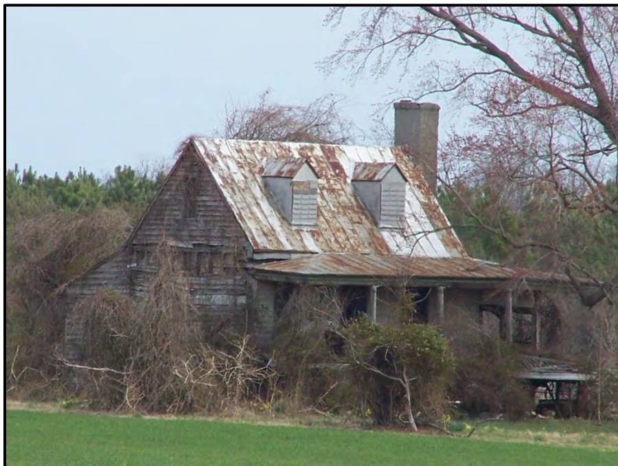
Figure 31. Cottage at Seatons Place (c. 1800; VDHR #050-0099), 125 Seaton's Lane, View Looking Northeast.
