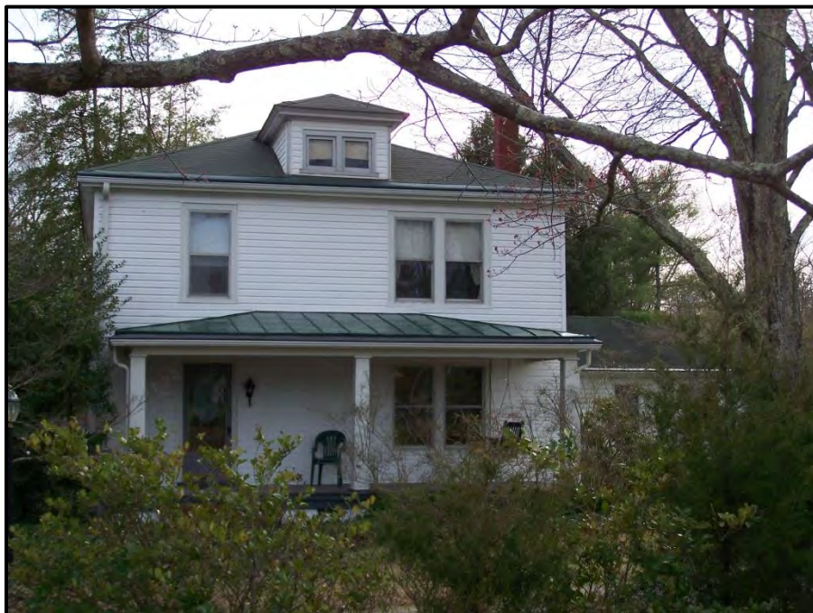
Figure 62. American Foursquare Dwelling (VDHR #050-0162), 20516 King William Road, View Looking Southwest.
