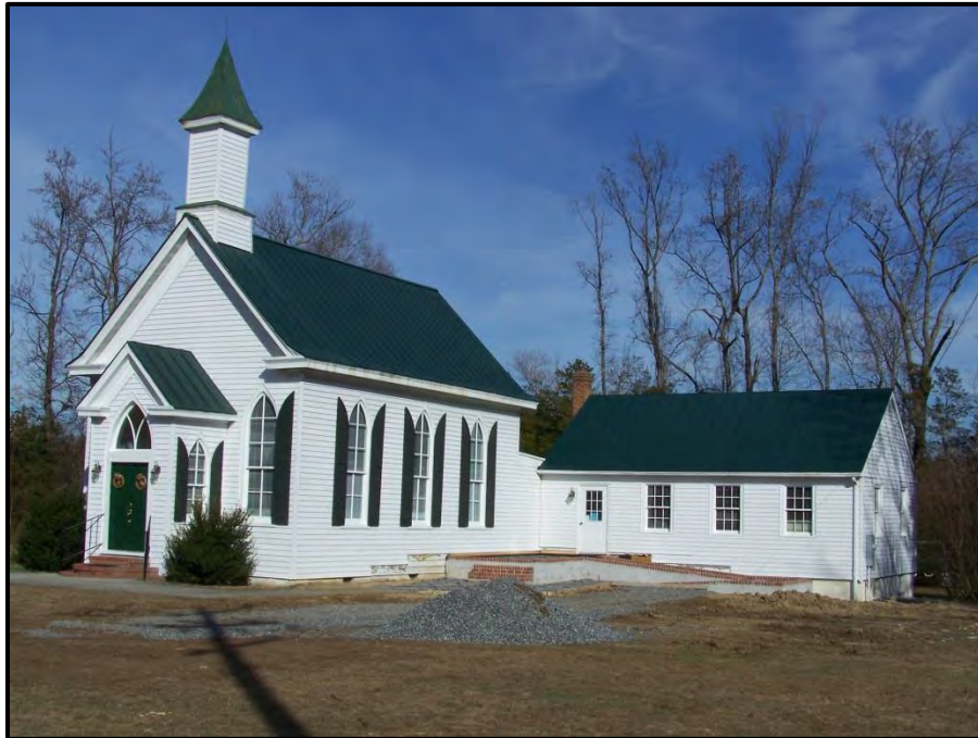
Figure 47. St. James Presbyterian Church (VDHR #050-5064), 411 Courthouse Lane, View Looking North.
