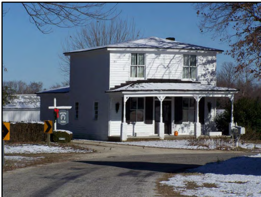
Figure 41. Duane Store (VDHR #050-5033), 4929 Herring Creek Road, View Looking Northeast.
