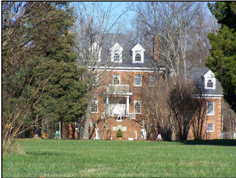
Figure 63. Fontainebleau (c. 1845; Rebuilt 1930; VDHR #050-0025), 1377 Acqinton Church Road, View Looking Northeast.
