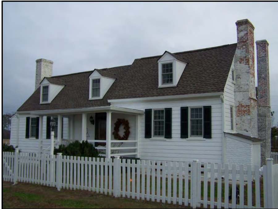
Figure 21. Brighton (c. 1765; VDHR #050-0007), 1600 Upshaw Road, View Looking Southeast.
