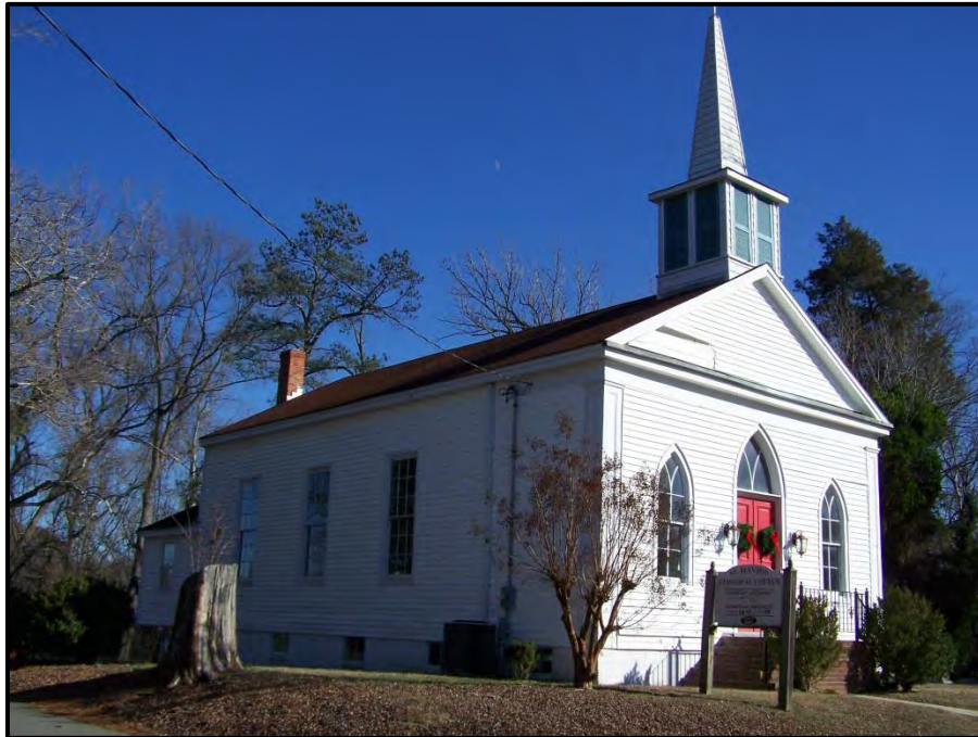
Figure 45. St. David's Church (VDHR #050-5050), 11291 W. River Road, View Looking East.
