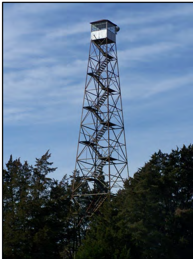
Figure 84. Fire Tower (c. 1935; VDHR #050-5062), King William Road, View Looking West.
