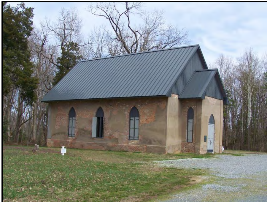
Figure 25. Acquinton Church (VDHR #050-0002), 5703 Acquinton Church Road, View Looking Northeast.
