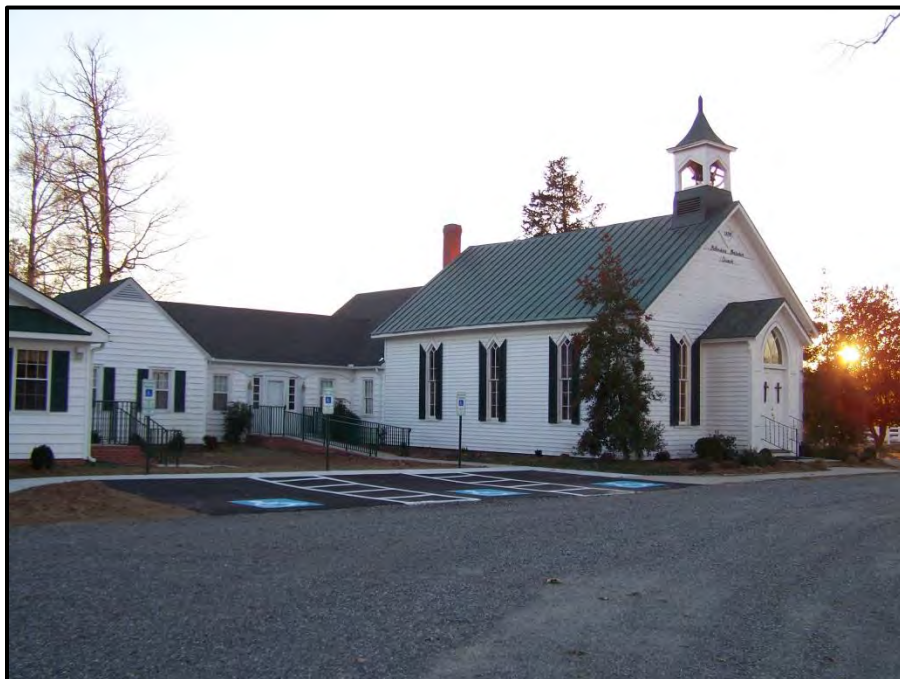
Figure 46. McKendree Methodist Church (VDHR #050-5055), 4347 Manfield Road, View Looking Southwest.
