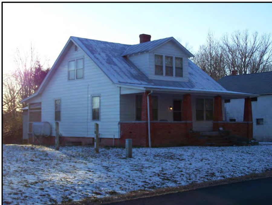
Figure 56. House Associated with Store (VDHR #050-5040), 5698 West River Road, View Looking West.
