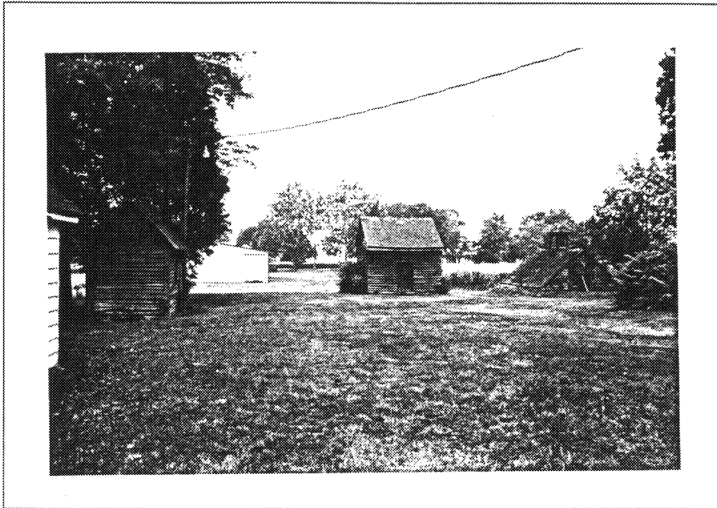
Figure 70: Outbuildings at Epping Forest (051-0008)
