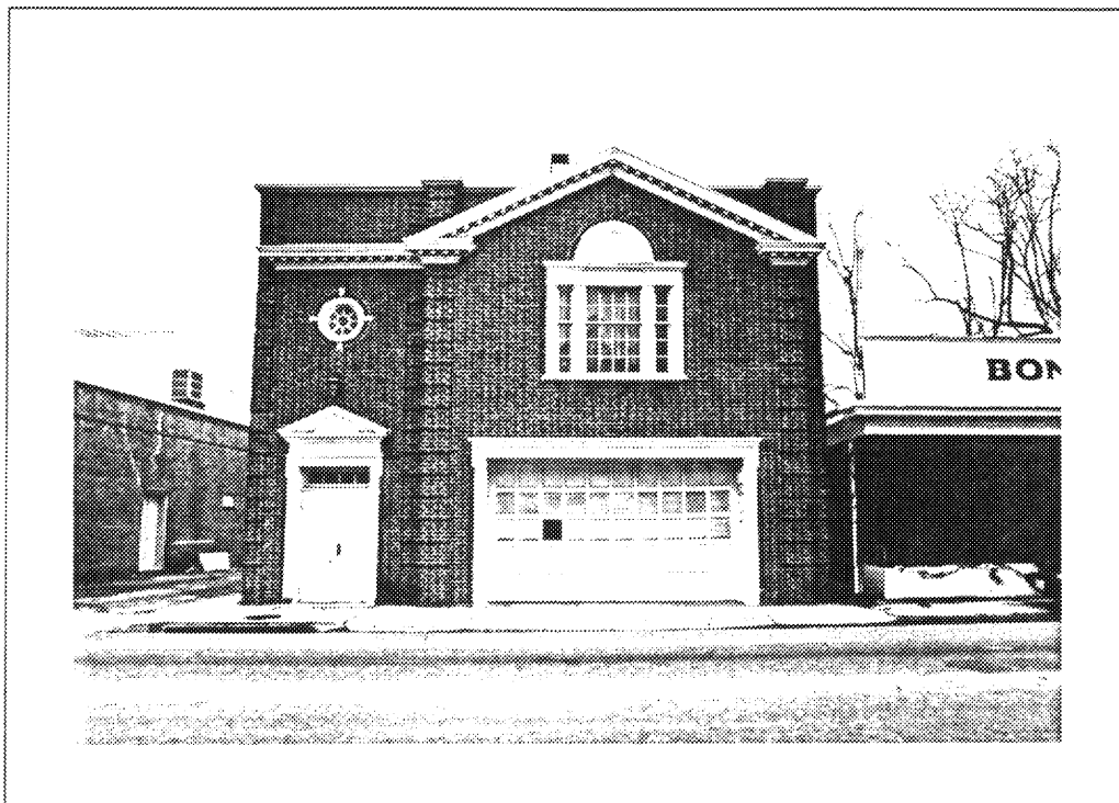
Figure 107: Kilmarnock Fire Station (249-5005)
