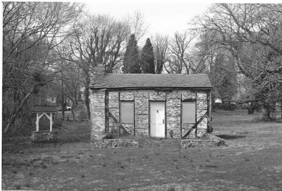
Figure 11: Workshop and Well, 302 North King Street (253-5122)
