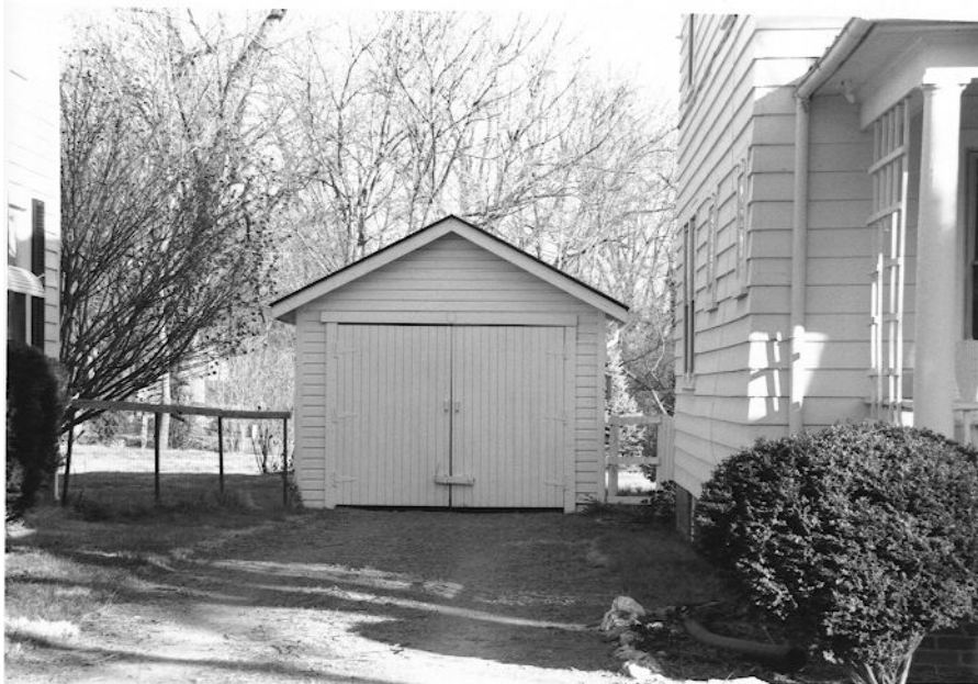
Figure 8: Garage, 10 Wilson Avenue (253-5129)
