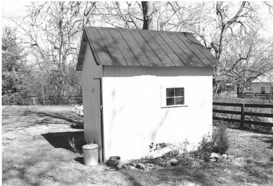
Figure 9: Shed, 310 Edwards Ferry Road (253-5080)
