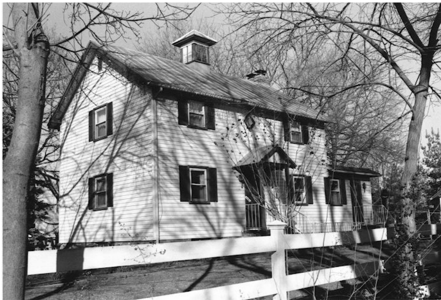
Figure 16: Former Barn, 18 Wilson Avenue (253-5132)
