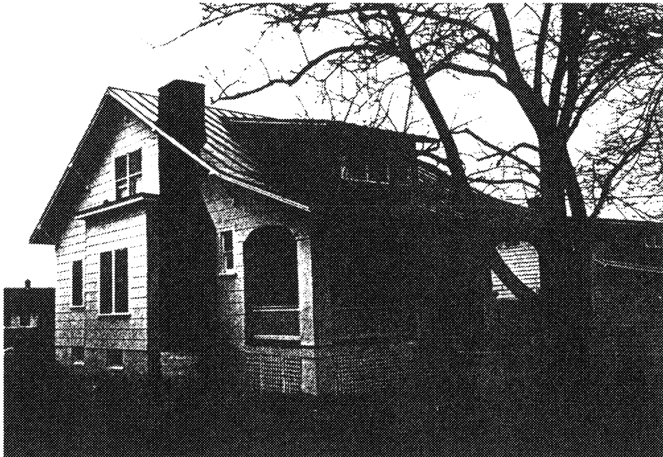
Photo 18 House at 225 Loudoun Street (253-35-552)
