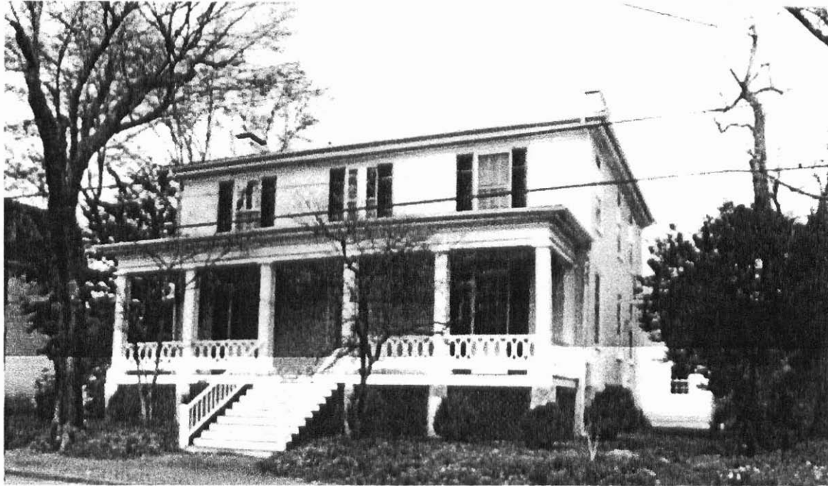
Figure 37 253-0030 St. James Episcopal Church Rectory (South elevation)
