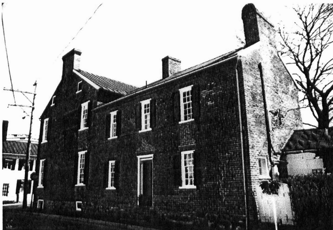
Figure 2 253-0035-0179 Birkby/Bengston House (West Elevation)
