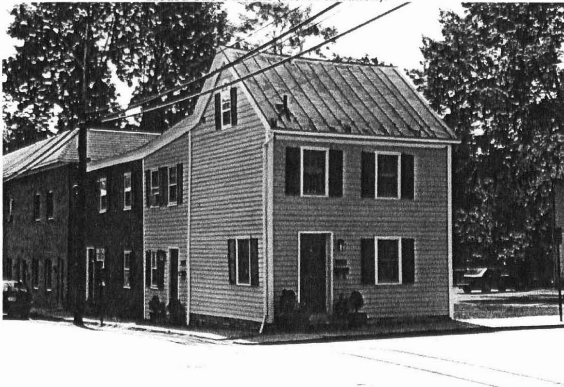
Figure 25 253-0035-0346 Nixon/Carrera House (West elevation).
