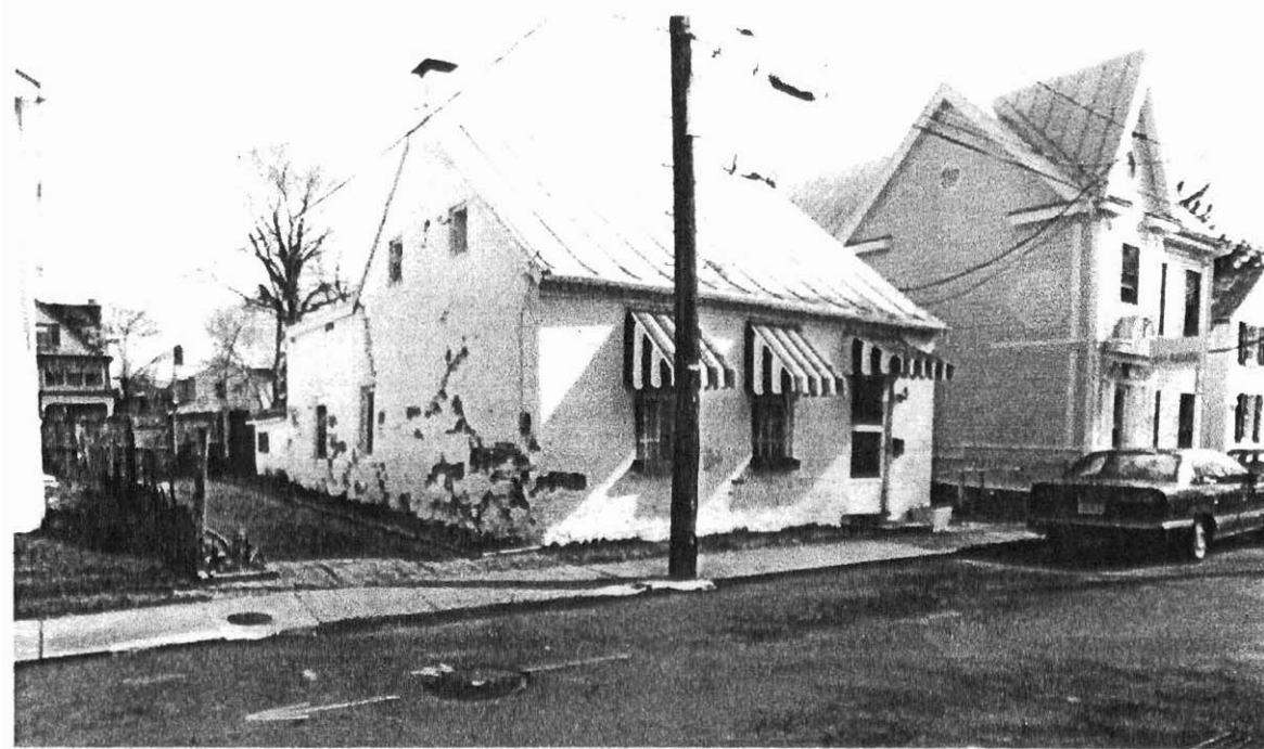
Figure 30 253-0035-0164 Parsel (West elevation)
