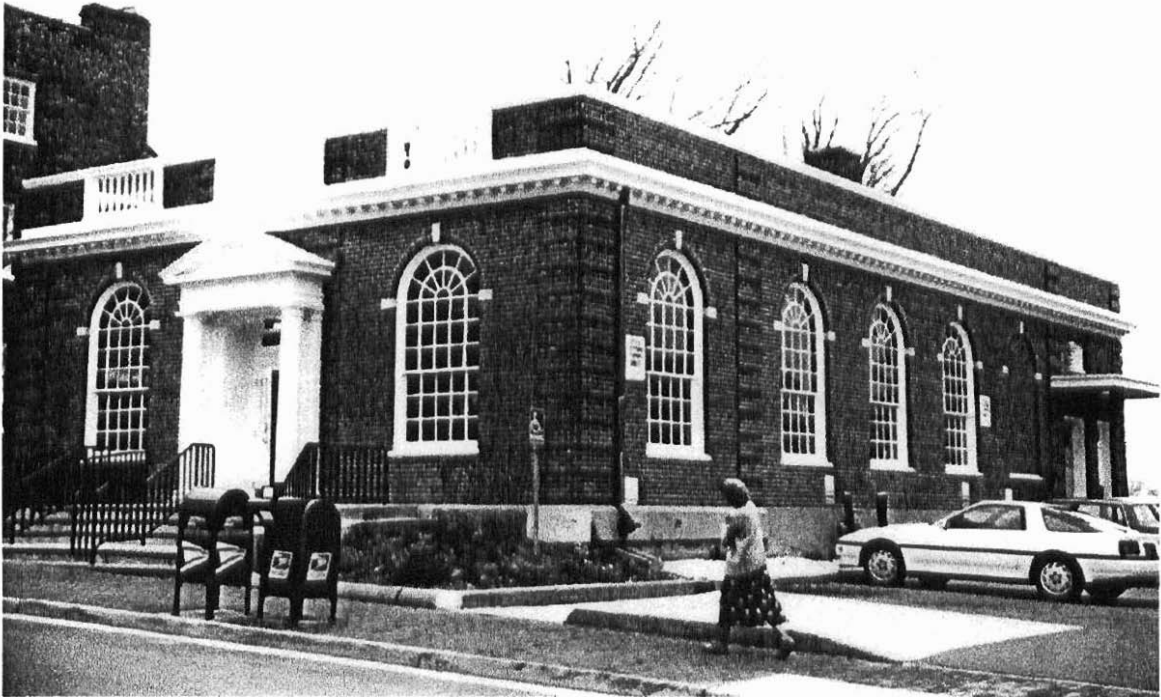
Figure 65 253-0008 U.S. Post Office (North West elevation).
