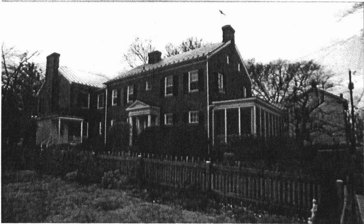
Figure 69 253-0035-0362 Engles House (East elevation).
