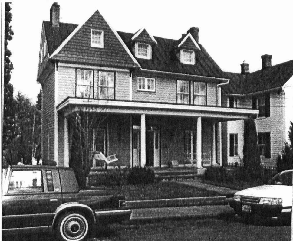
Figure 47 253-0035-0352 Reimer House (South elevation).
