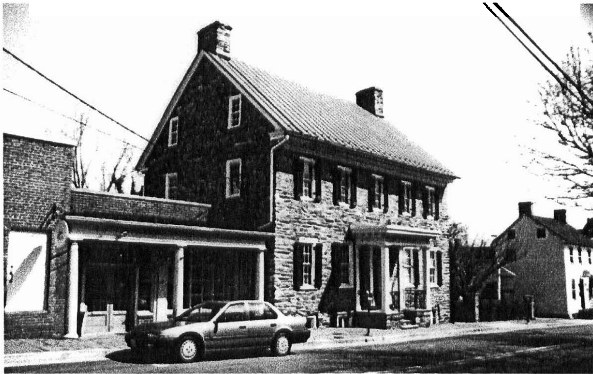
Figure 8 253-0004 Patterson House/McCabe Tavern (South elevation)
