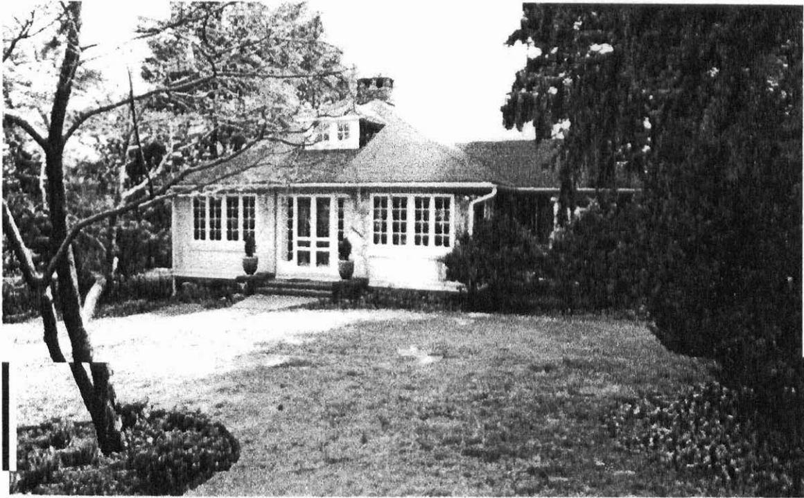
Figure 52 253-0035-0273 Hincerick-Pittman House (North elevation)
