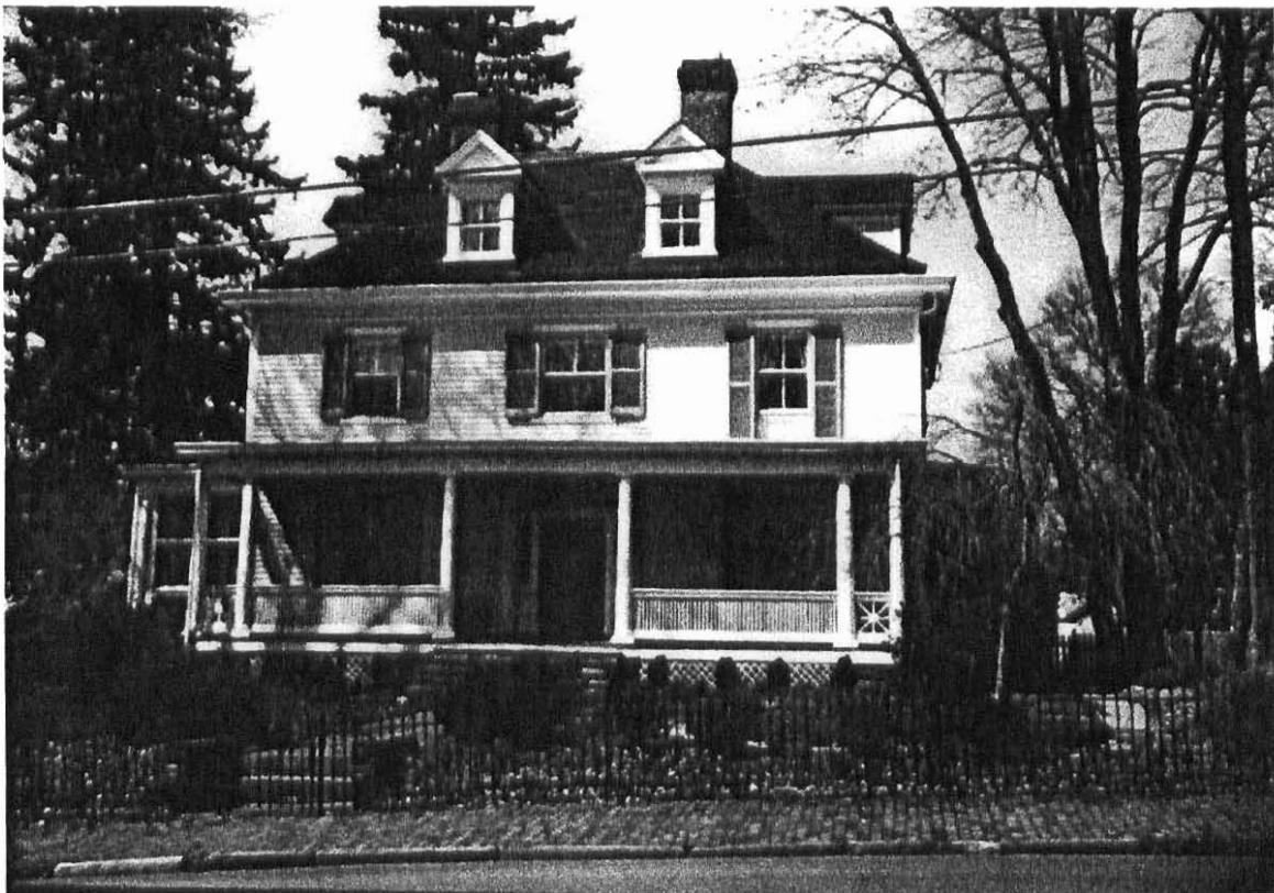
Figure 49 253-0035-0151 McCabe/Grimshaw House (East elevation)
