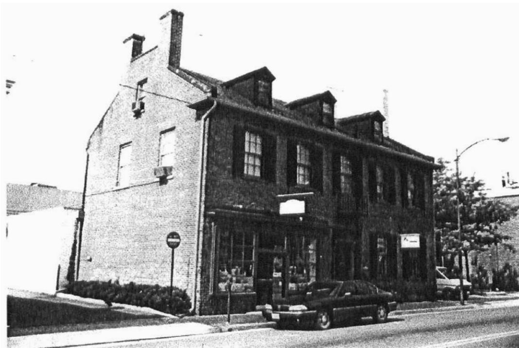
Figure 40 253-0035-0247 Leesburg Hospital/Crafters Gallery (North elevation).
