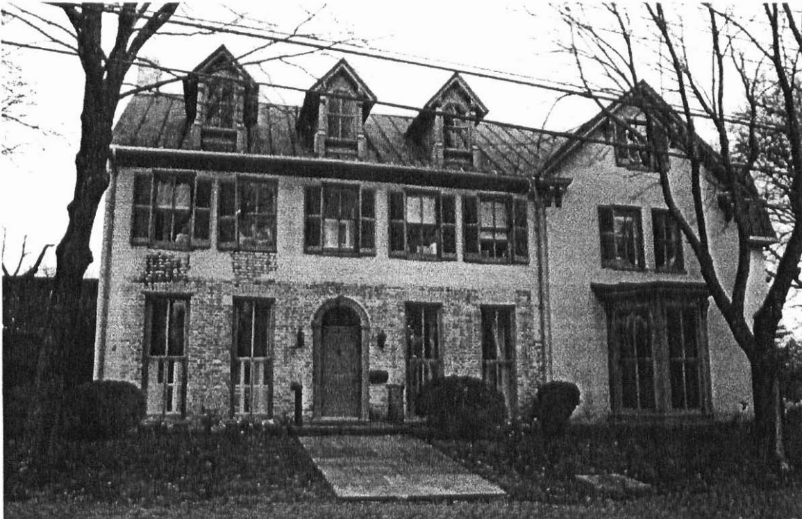
Figure 44 253-0030AA Chas. Janney House (South elevation).
