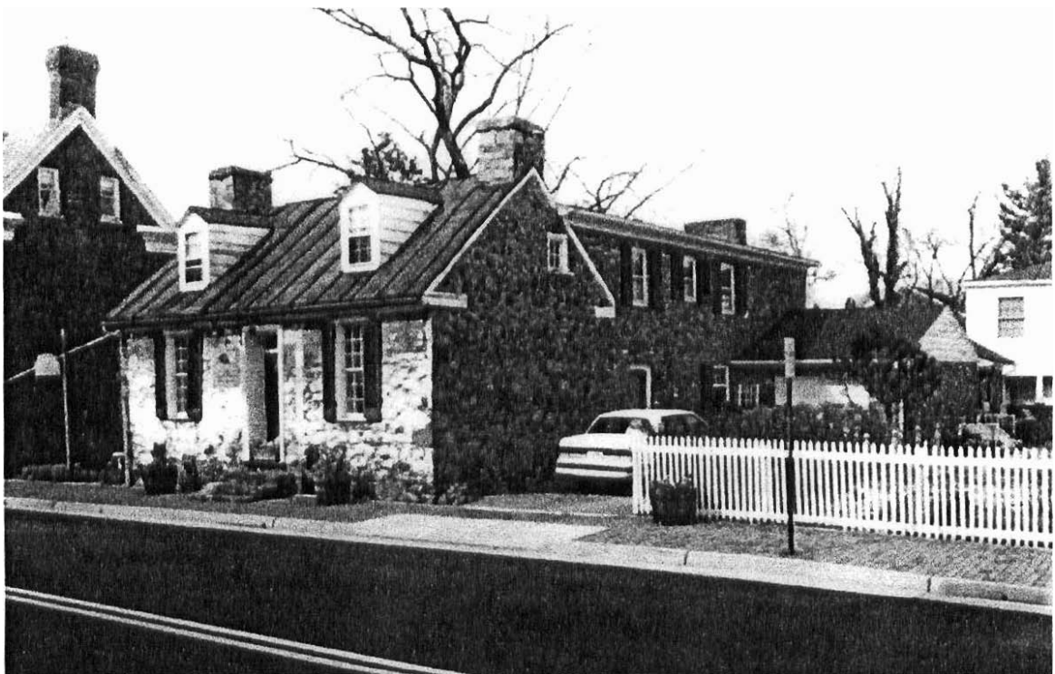
Figure 16 253-0003 (253-0035-0159) Stone House Tea Room (South Elevation)
