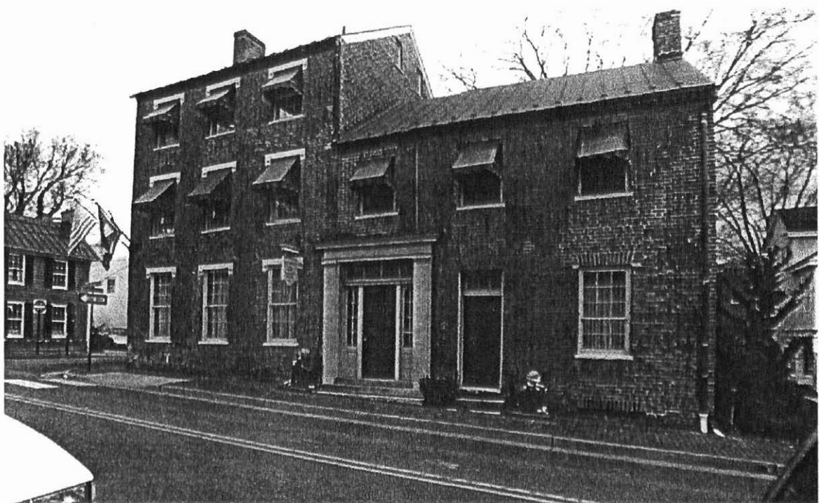
Figure 21 253-0035-0365 Philip-Hall Building (West elevation)
