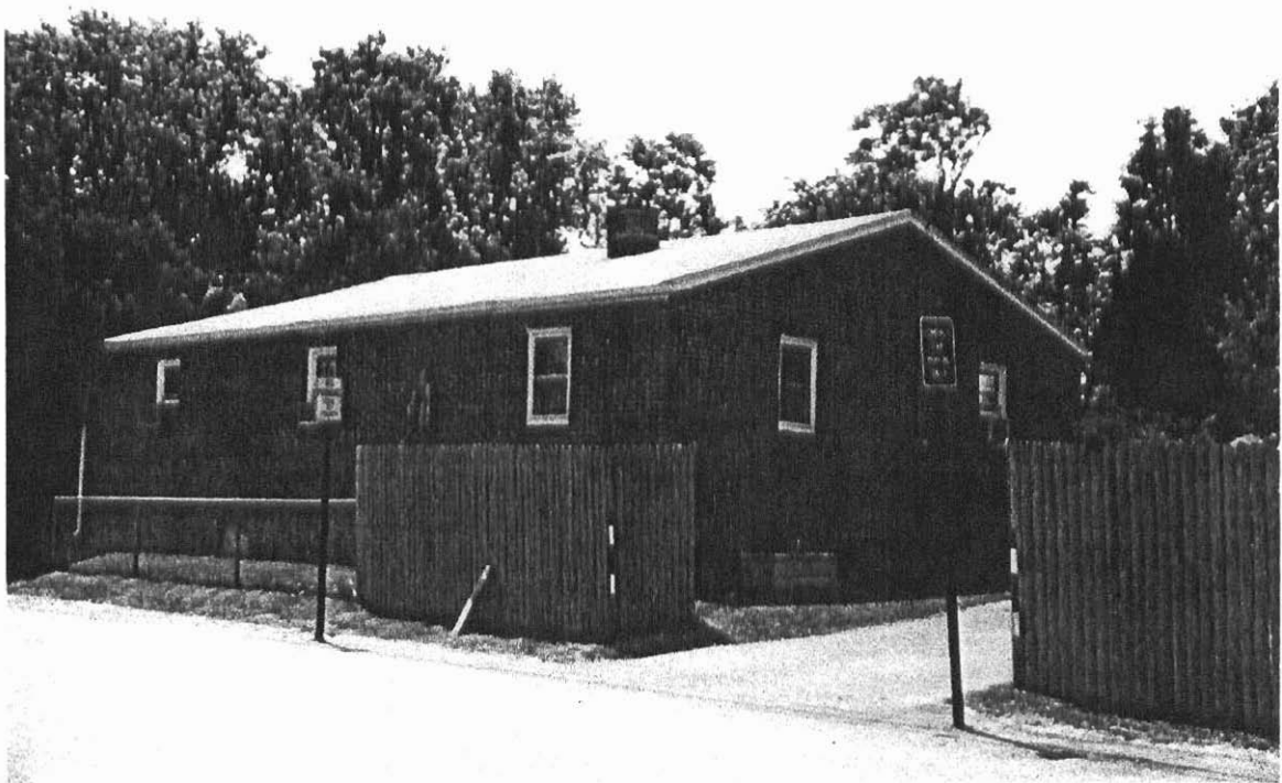
Figure 72 253-0035-0357 Bell House (North elevation).
