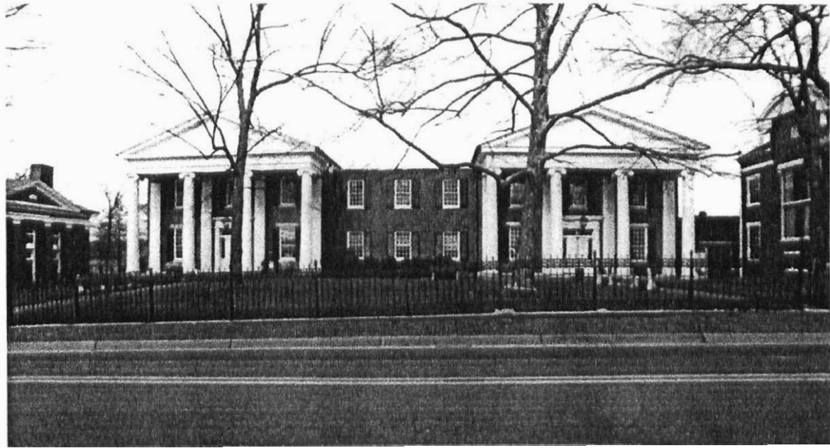
Figure 35 253-0005 Leesburg Boys academy/Loudoun County Clerks Office (South elevation).
