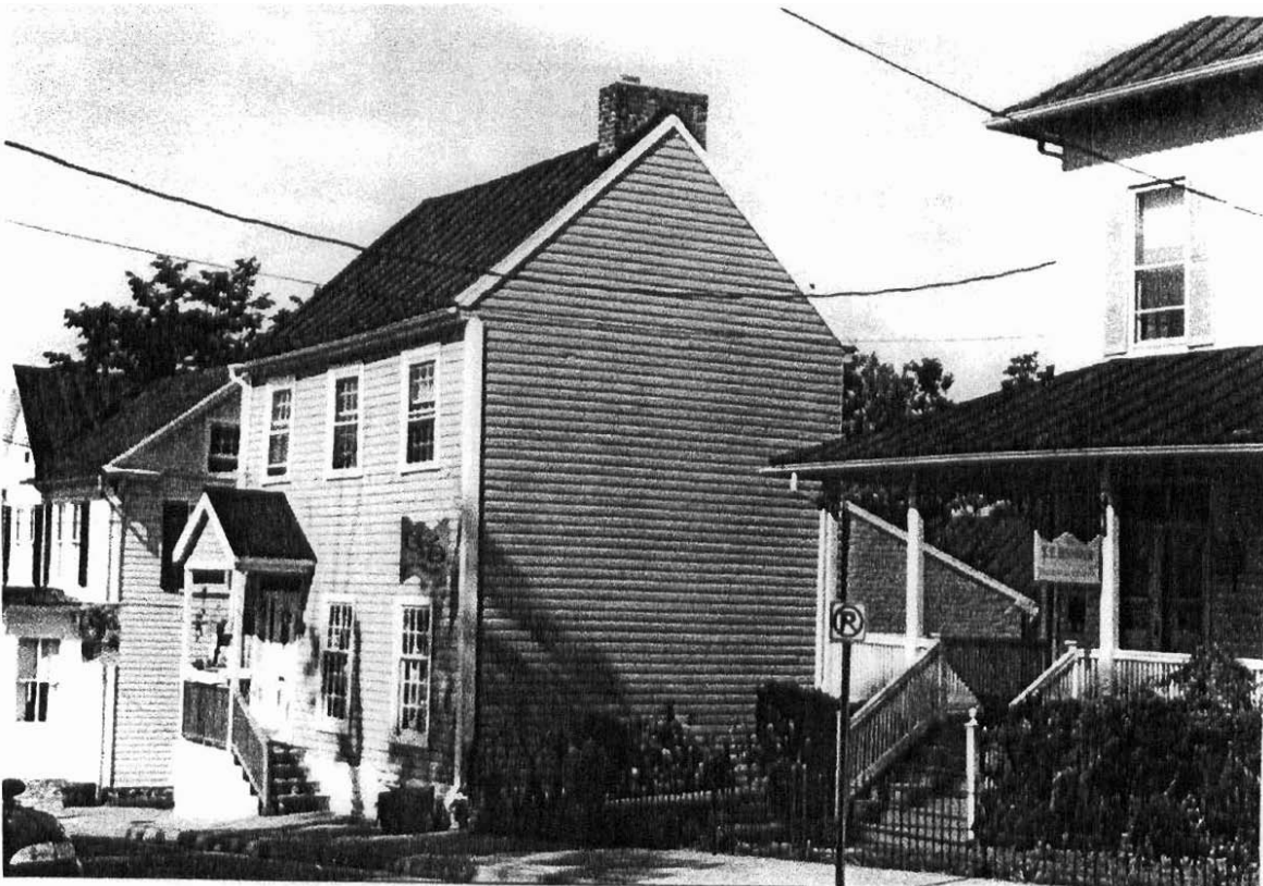
Figure 12 253-0042 (253-0035-0219) Janney/Bredimus House (East elevation).
