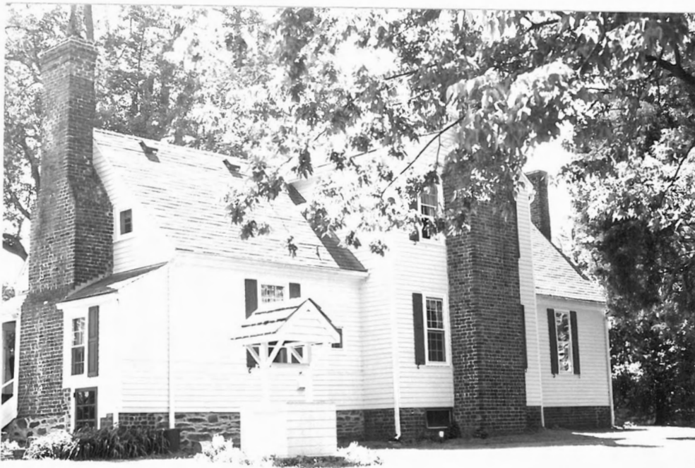
Figure 6 Dunlore (DHR 54-18) Land and Community Associates
