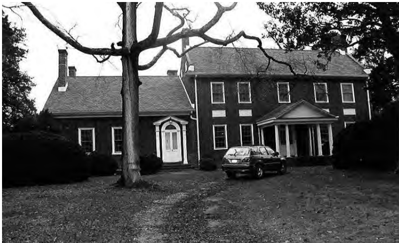
Figure 19: Brickland was constructed in two phases, the left side in 1818 and the right side in 1822 (055-0002)
