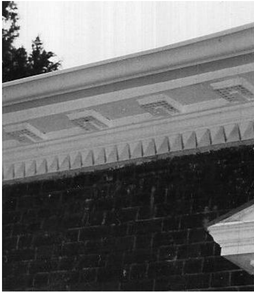
Figure 20: Cornice at Brickland, ca. 1818
