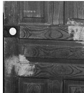
Figure 56: Interior door graining detail at the Jeter House (055-5036)
