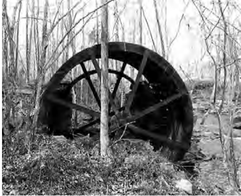
Figure 88: Stones Mill Ruins, ca. 1870 (055-5067)
