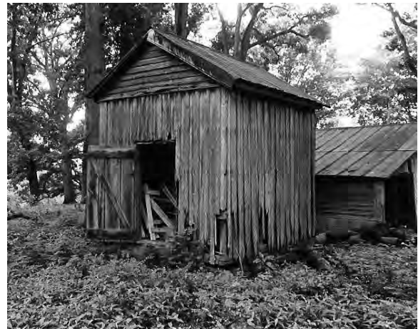
Figure 66: Smokehouse, ca. 1860, House in the Grove (055-5072-0003)
