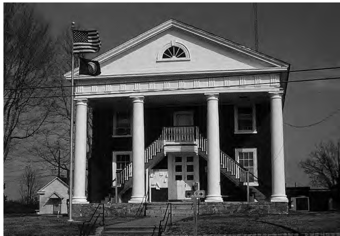
Figure 18: Lunenburg County Courthouse, 1827 (055-0105-0025/055-0014)
