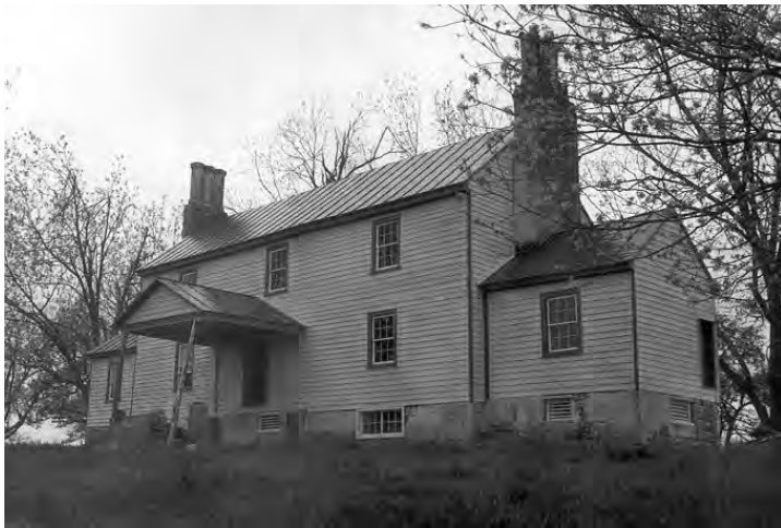
Figure 47: Flat Rock, ca. 1780, chimneys added ca. 1856 (055-0003)
