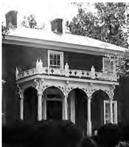
Figure 40: Elmwood, Holt inspired porch added ca. 1870 (055-0042)
