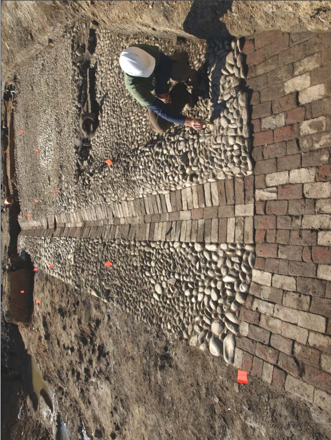
Figure 31. Detail of cobble paving, brick drain, and berm feature, view to south.
