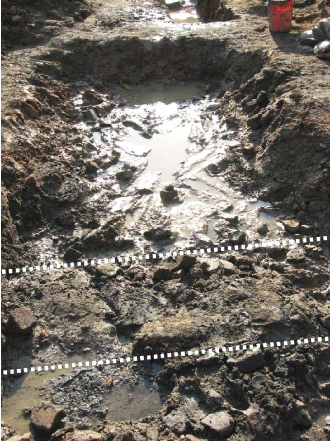
Figure 78. North foundation wall of the jail building.
