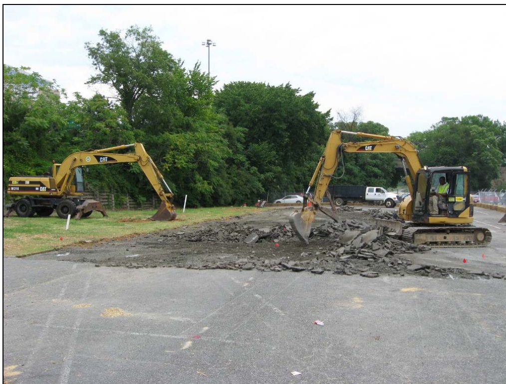
Figure 20. Removing asphalt paving within excavation area, August 2008.
