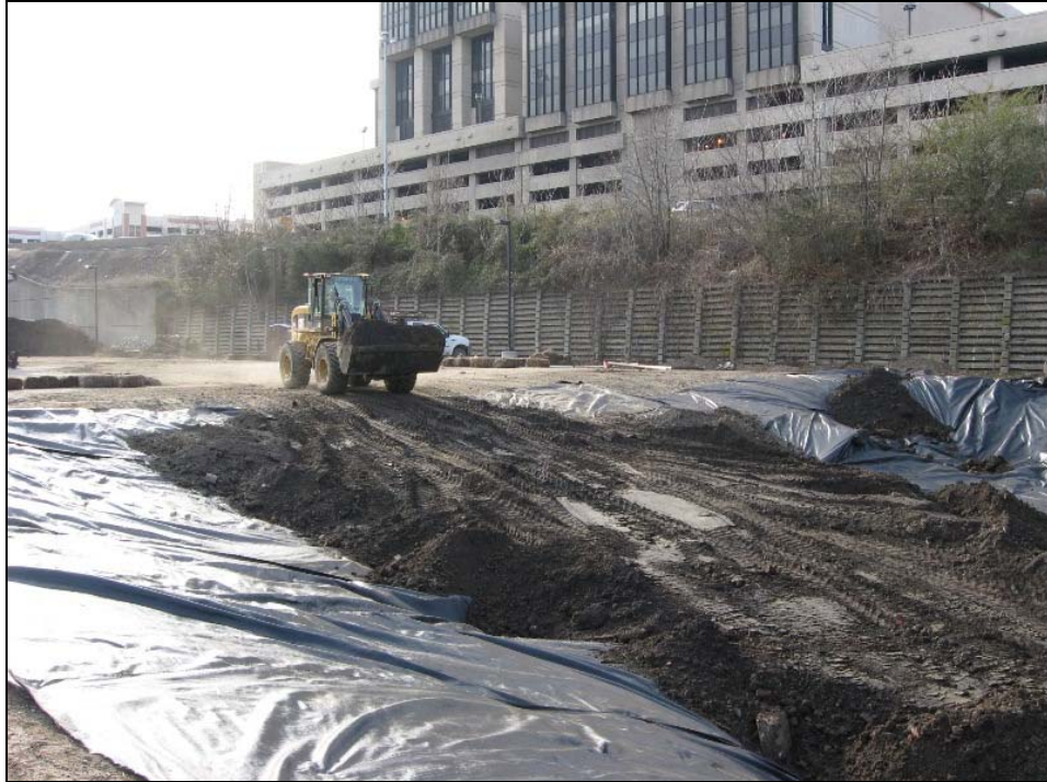
Figure 81. Completing the initial lift of backfill soils.
