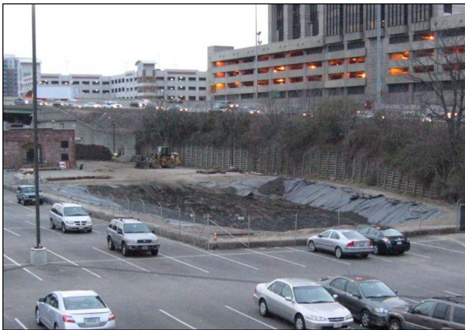
Figure 82. Excavation area after the initial lift of backfill material was completed.
