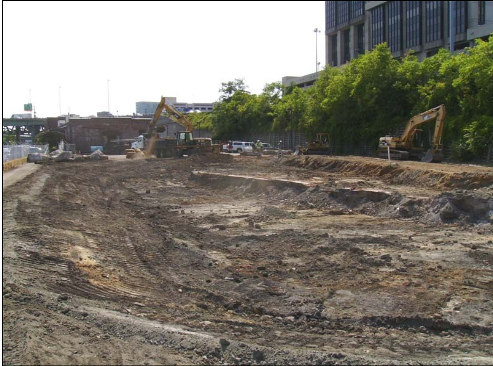
Figure 24. Mechanical excavation reveals the Richmond Iron Works foundation.
