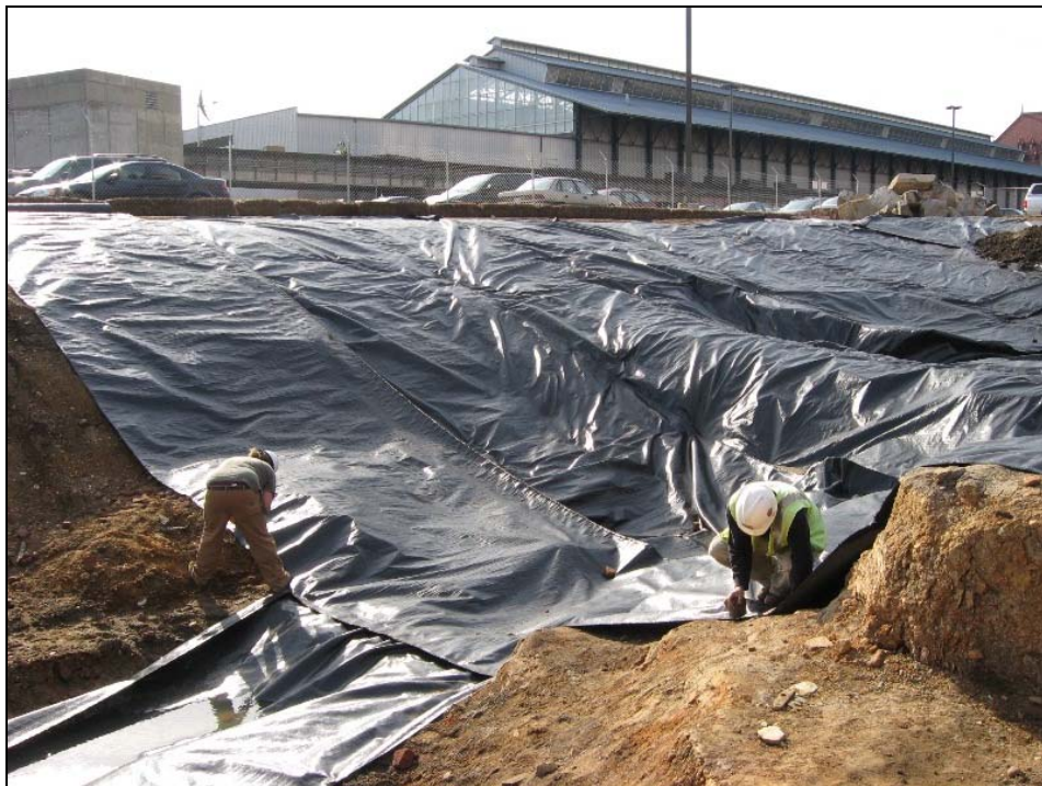
Figure 80. Covering the excavation area with woven geotextile fabric.
