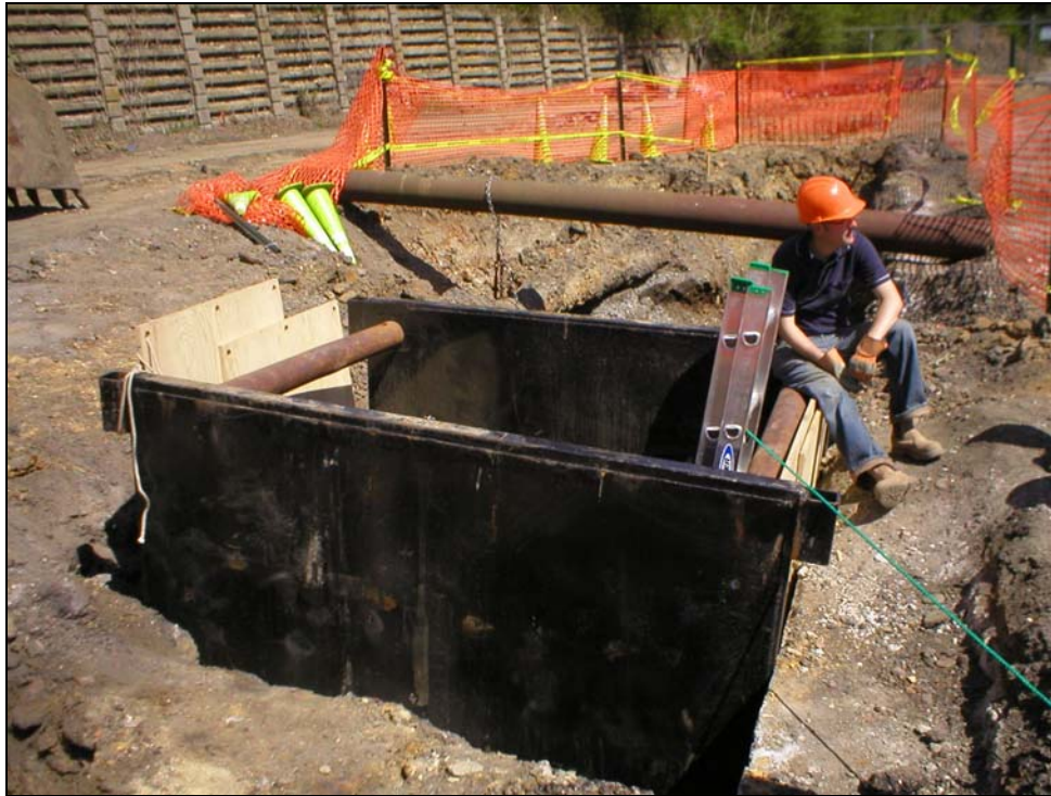
Figure 17. Trench 2 with steel trench box in place.
