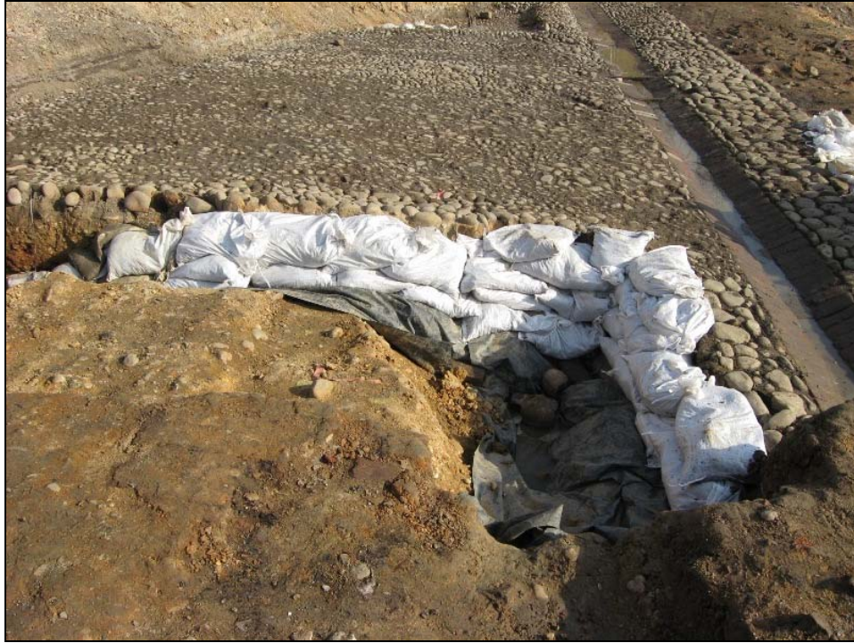
Figure 79. Securing the Lumpkin period kitchen foundation prior to reburial.
