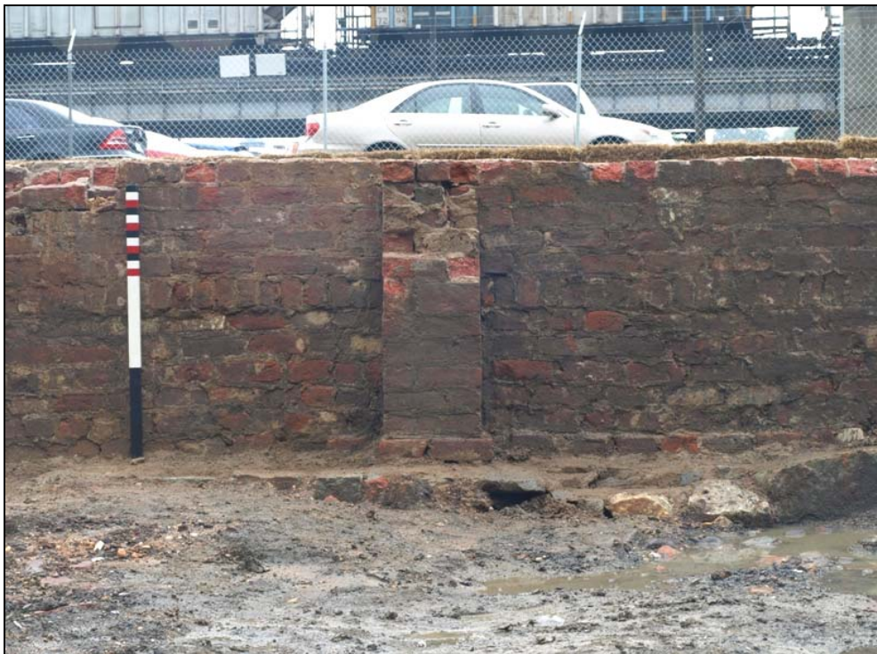
Figure 25. Detail of Richmond Iron Works foundations.
