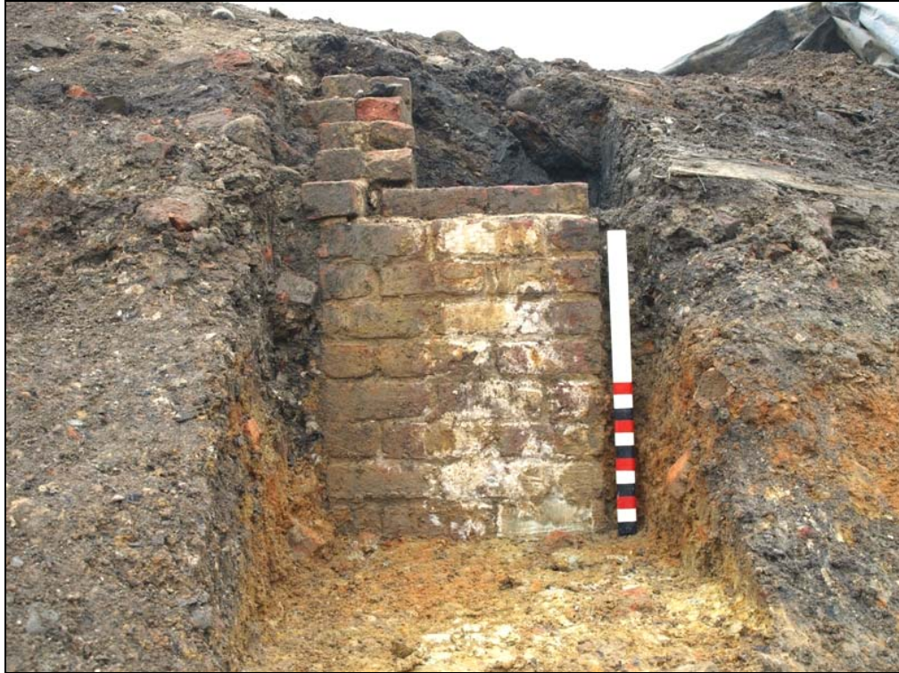
Figure 74. Brick pier at northeast corner of Structure 44, view to south.
