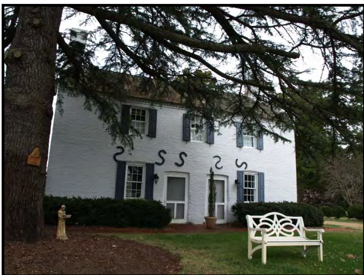
Figure 6. The kitchen at Auburn (057-0001) dates to the early 19th century and likely served as a slave quarter.
