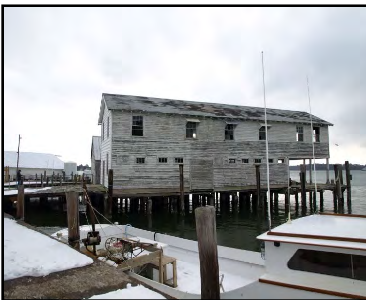
Figure 13. Callis Wharf (057-5234), warehouse west elevation.
