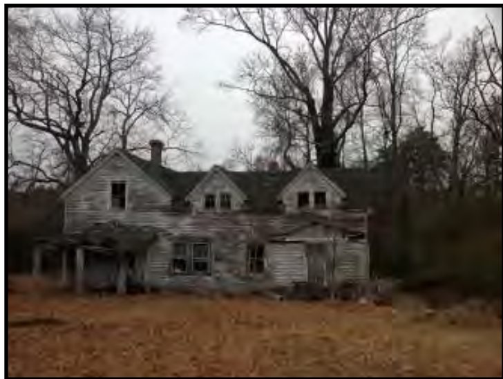
Figure 10. House on Sandberg Lane (057-5152), south elevation.
