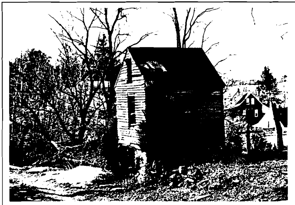
Fig. 64. Stevens' House Shed (DHR 62-042)
