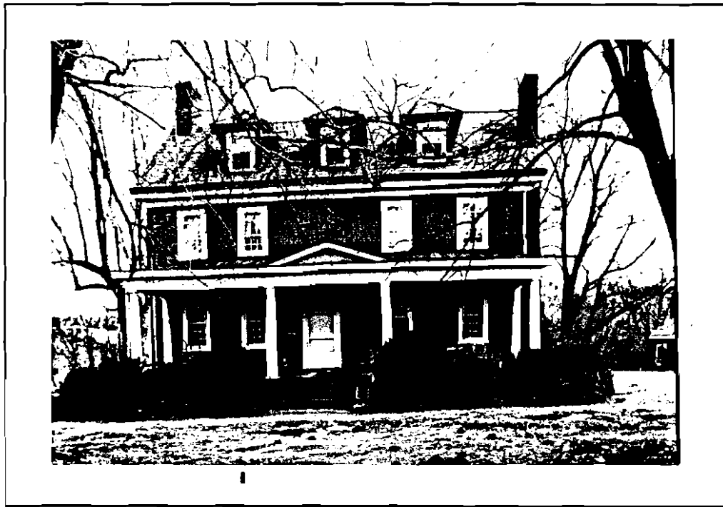
Fig. 22. Three Chimneys (DHR 62-433)
