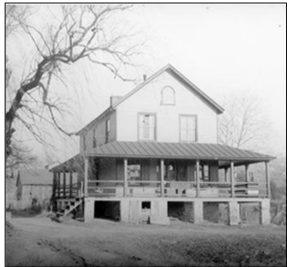
Figure 22- Following the 1870 flood, Norwood merchant Charles Andrew Stratton constructed a new store (062-0238) along the canal about one mile downriver from Norwood. (Image: WPA VA Historical Inventory, Library of Virginia)
