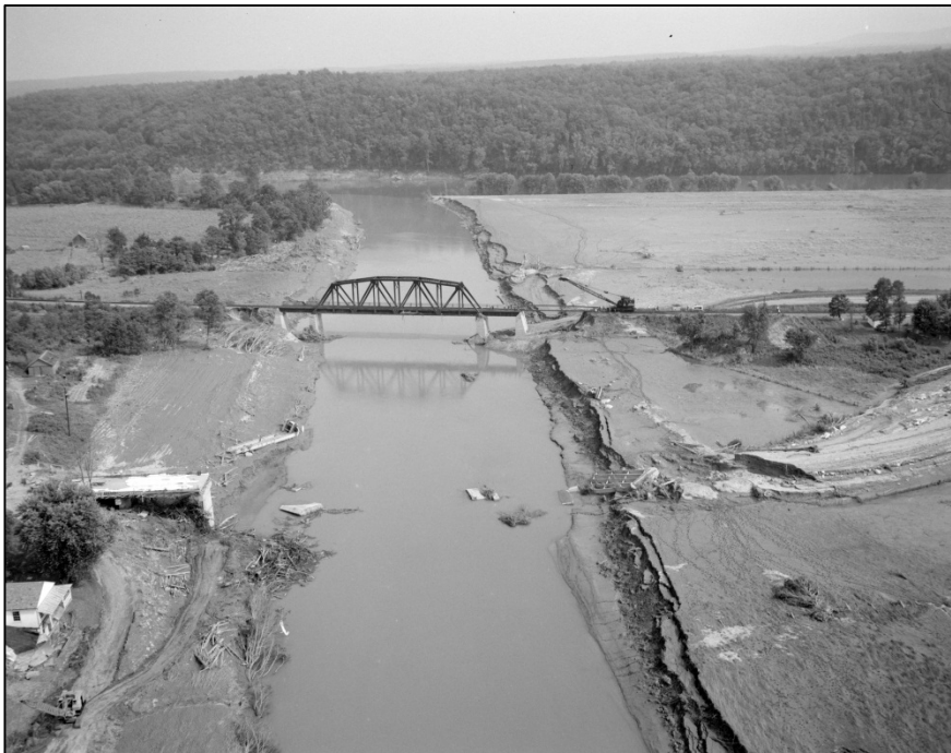
Figure 36- Hurricane Camille destroyed the Tye River road bridge at Norwood. The damaged porches of Peters Store (062-0216) can be seen in the lower left corner
