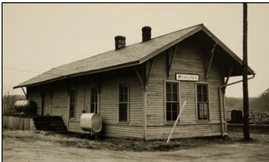
Figure 29- Wingina's Depot on the C&O Railroad (062-0034) (demolished)
