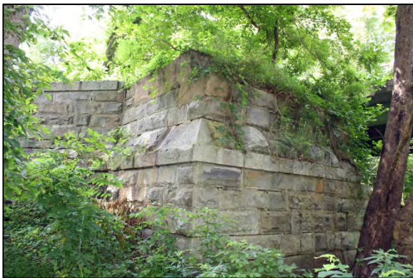
Figure 15- Finely crafted stone bridge abutment (ca. 1849) (062-0035) on the south end of the Route 56 bridge over the James River in Buckingham County.
