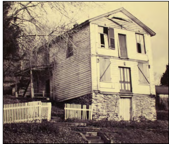
Figure 40- The Nelson Store (062-0218) burned in the early 1990s. Only its foundation remains.
