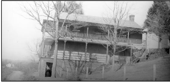
Figure 18- An early image of Peters Store showing the later porches. Peters' large frame house (no longer extant) can be seen to the right across Variety Mills Road. (WPA VA Historical Inventory)
