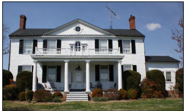
Figure 7- Soldier's Joy (062-0015) is one of the earliest extant buildings in the Norwood-Wingina study area
