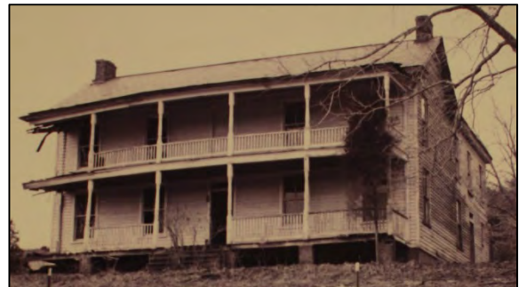
Figure 42- This dwelling (062-0232) on the west side of the Tye River is one of several that have been demolished since the last survey was conducted in the 1990s
