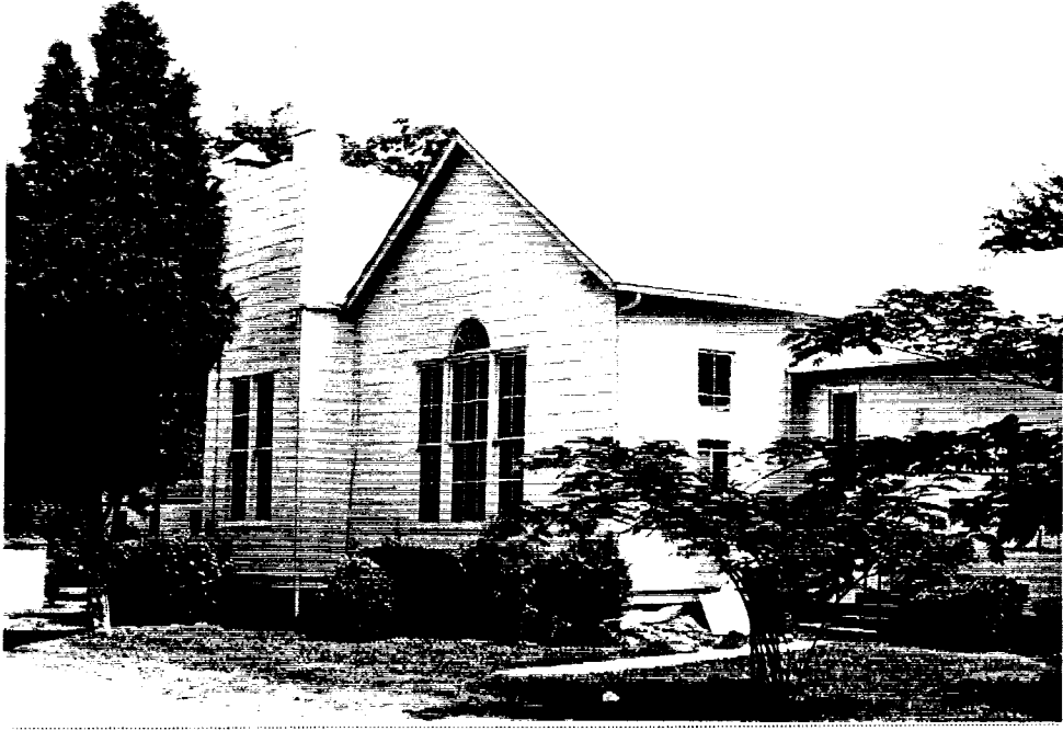
Figure 196: Church at 1801 Princeton Avenue
