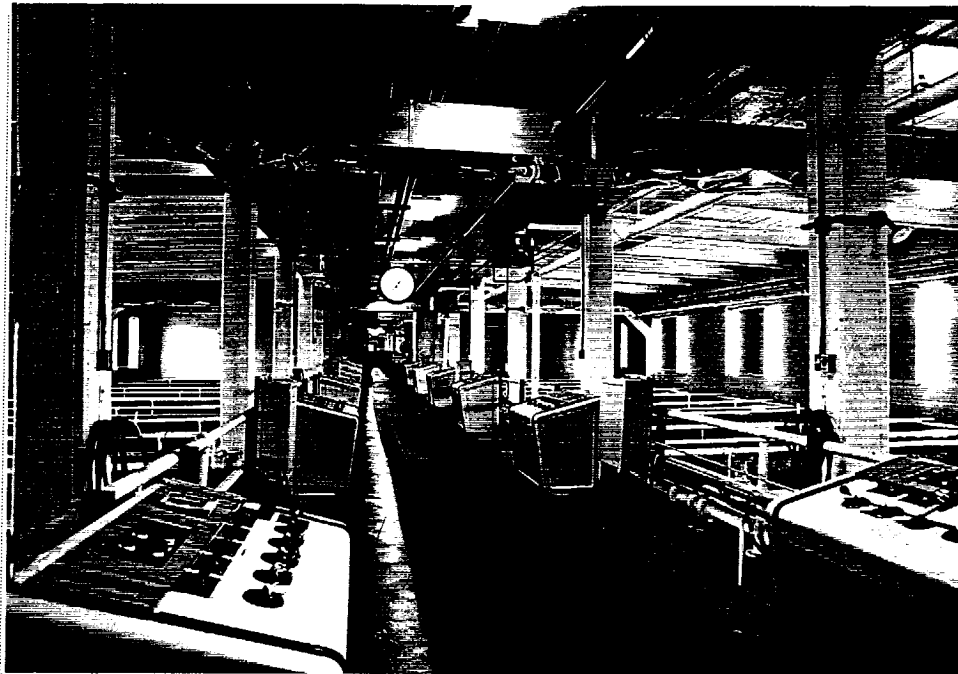
Figure 173: Lake Prince Water Treatment Plant, Filtration Building Interior
