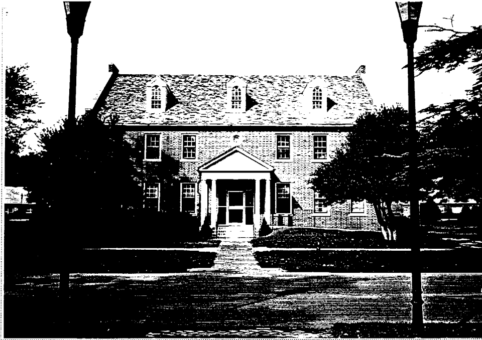
Figure 58: Barry Robinson Center, Administration Building
