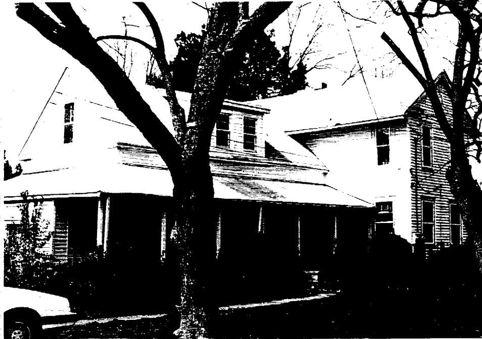
Figure 4: House at 716 Dudley Avenue
