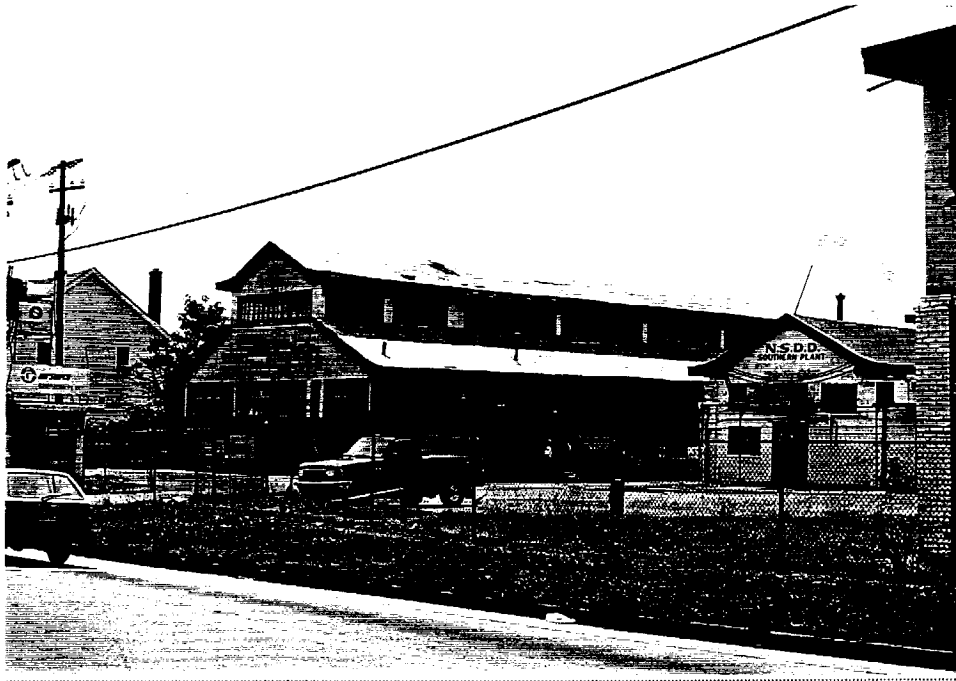
Figure 157: Norshipco Southern Plant
