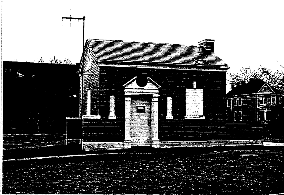
Figure 178: Pump Station in Park Place
