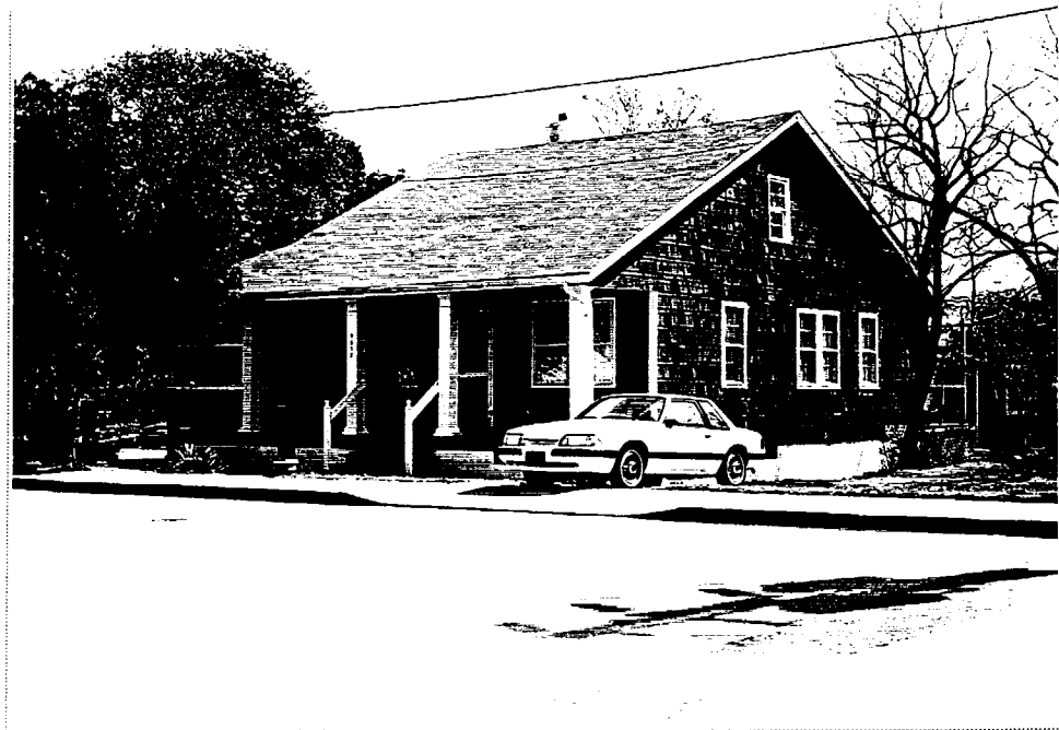
Figure 22: House at 9638 Thirteenth View Street
