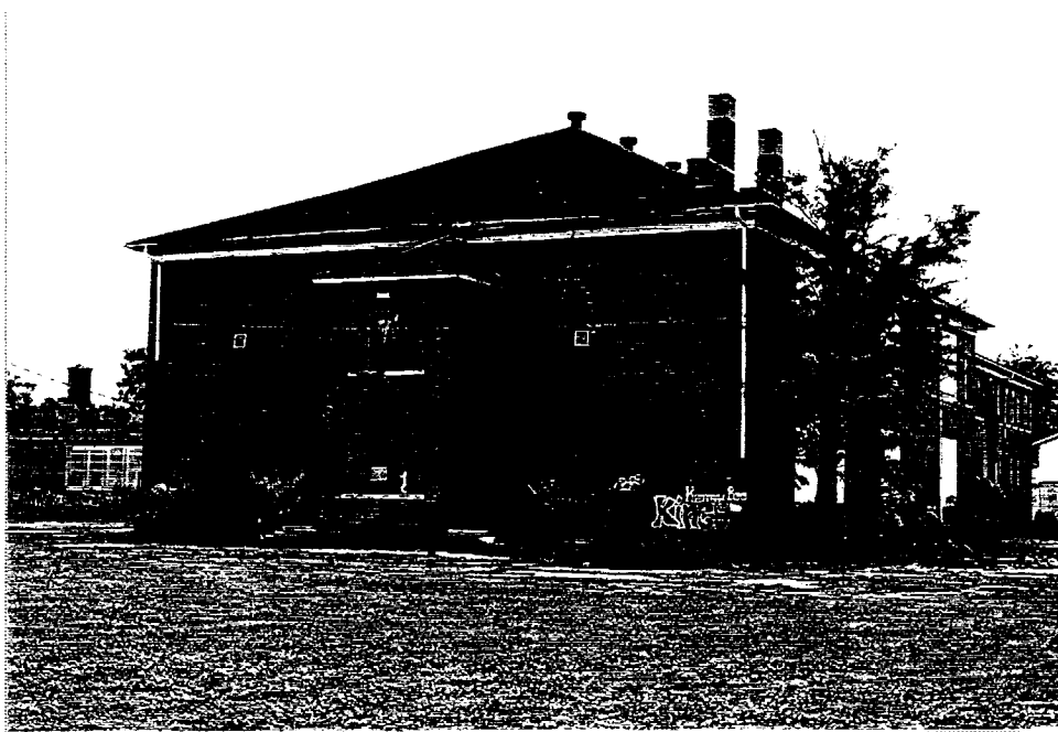
Figure 61: John T. West School, South Building
