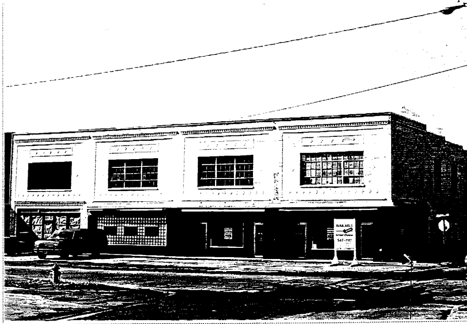
Figure 111: Building at 2111-2123 Colonial Avenue
