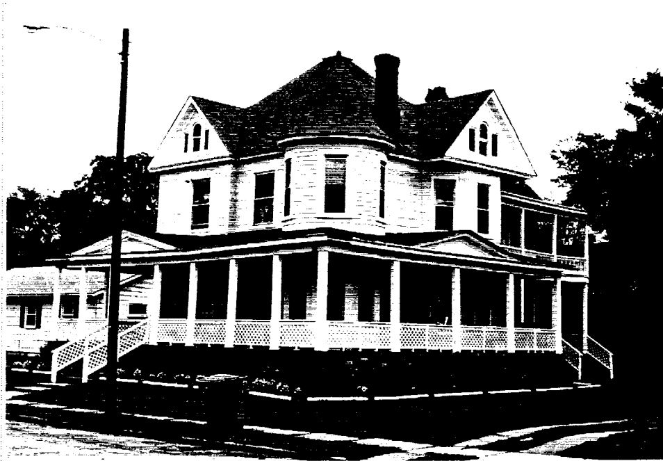
Figure 190: House at 1721 Arlington Avenue
