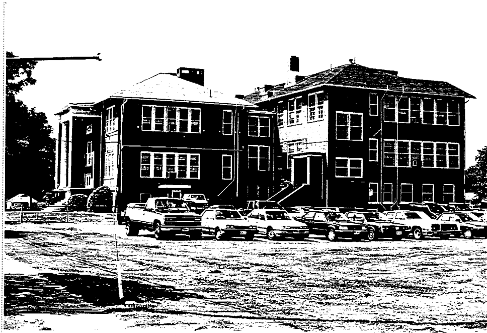
Figure 65: Ballentine School, Showing West Addition
