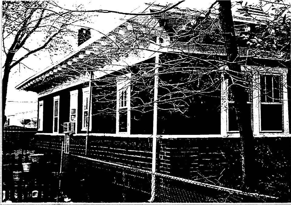
Figure 23: House at 9274 Rippard Avenue
