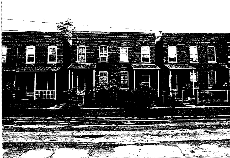
Figure 29: Duplex at 1527-1531 Dungee Street
