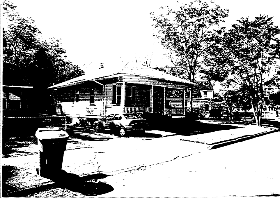
Figure 183: House at 2853 Keller Avenue
