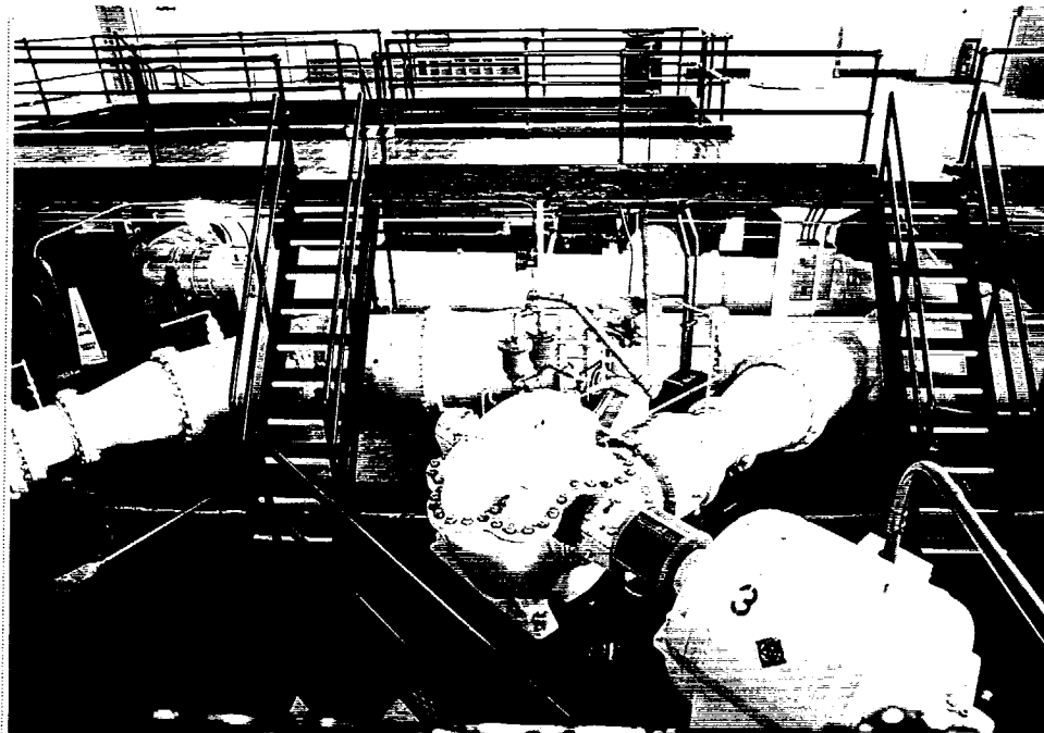
Figure 175: Lake Prince Water Treatment Plant, Pumping Station Interior
