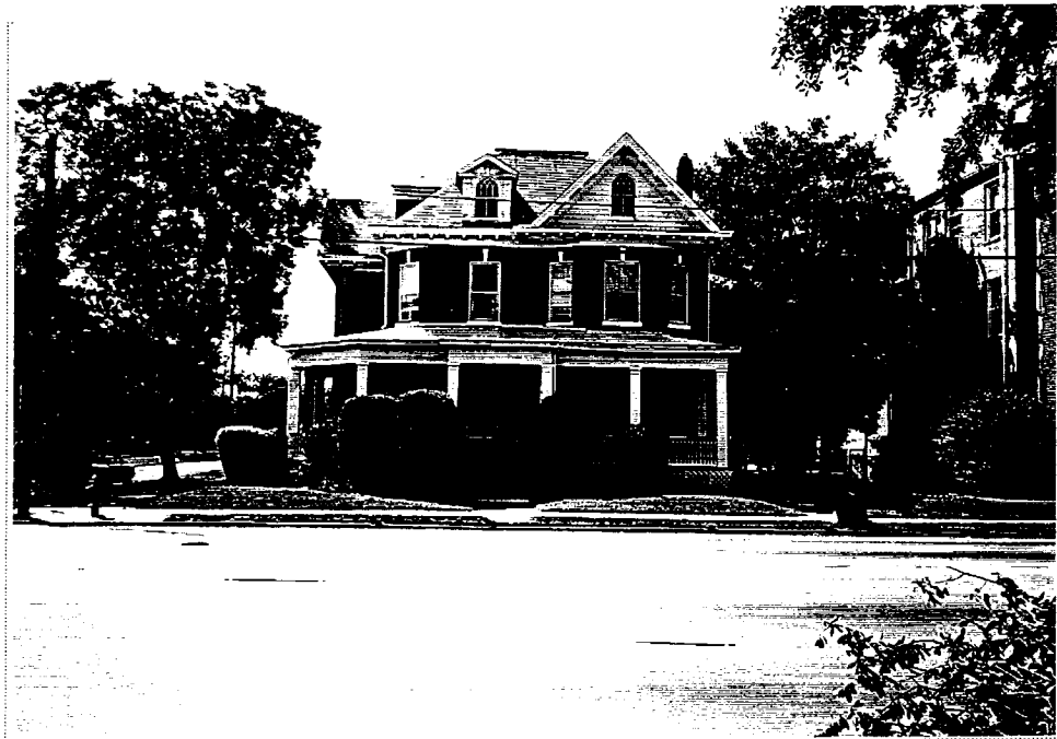
Figure 14: House at 3701 Granby Street
