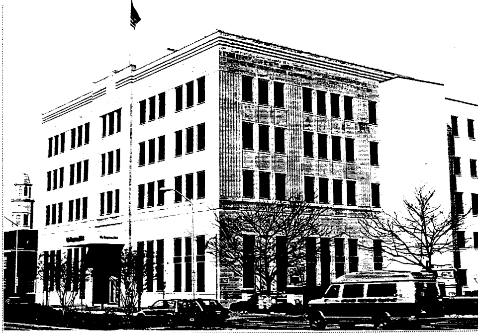
Figure 122: Virginian Pilot Building
