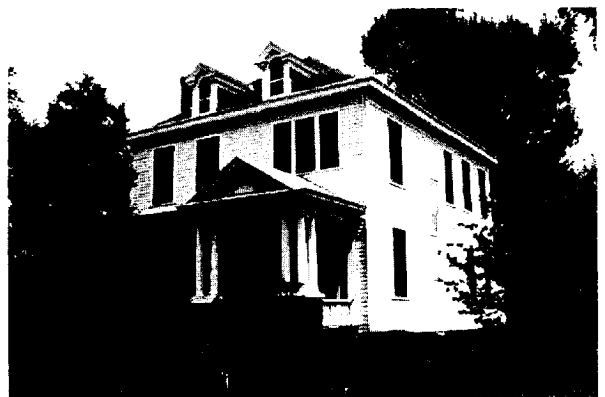
Figure 35. House, 1316 W. Virginia Ave. (203-0039).
