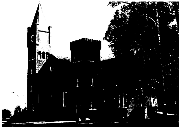
Figure 48. Crenshaw United Methodist Church
