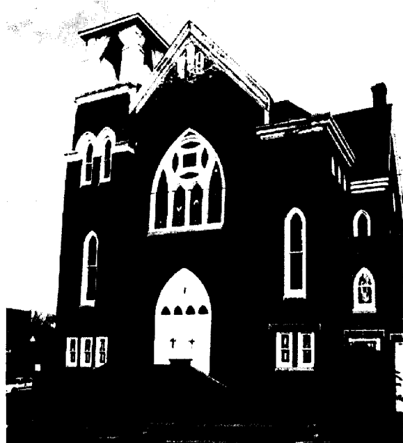
Figure 49 Crewe Methodist Church (203-0001)
