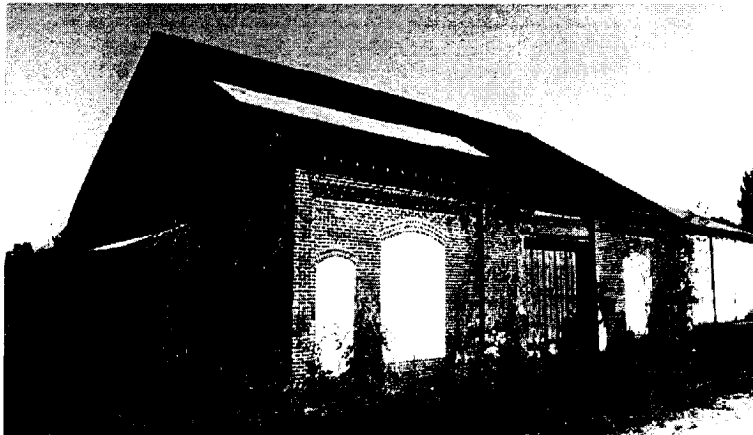
Figure 56. Crewe Power Plant (203-46)
