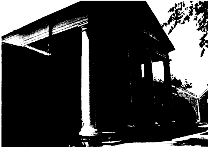
Figure 39. Nottoway Court House (67-4)
