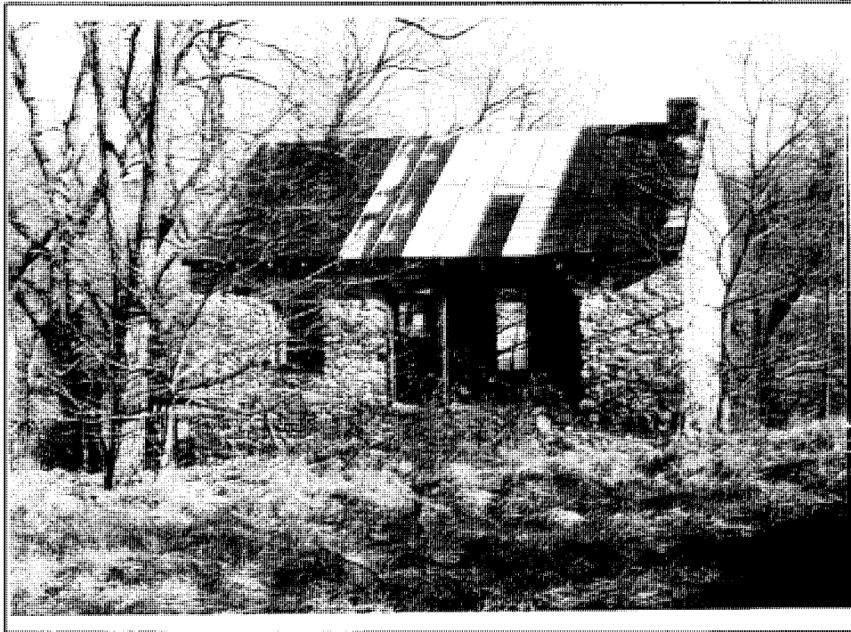
Fig. 17. A stone building near the site of Isabella Furnace that is believed to have functioned as the ironworks office (069-0193). The ruinous building is built into a bank and has Federal interior detail that suggests a date of construction in the early nineteenth century.
