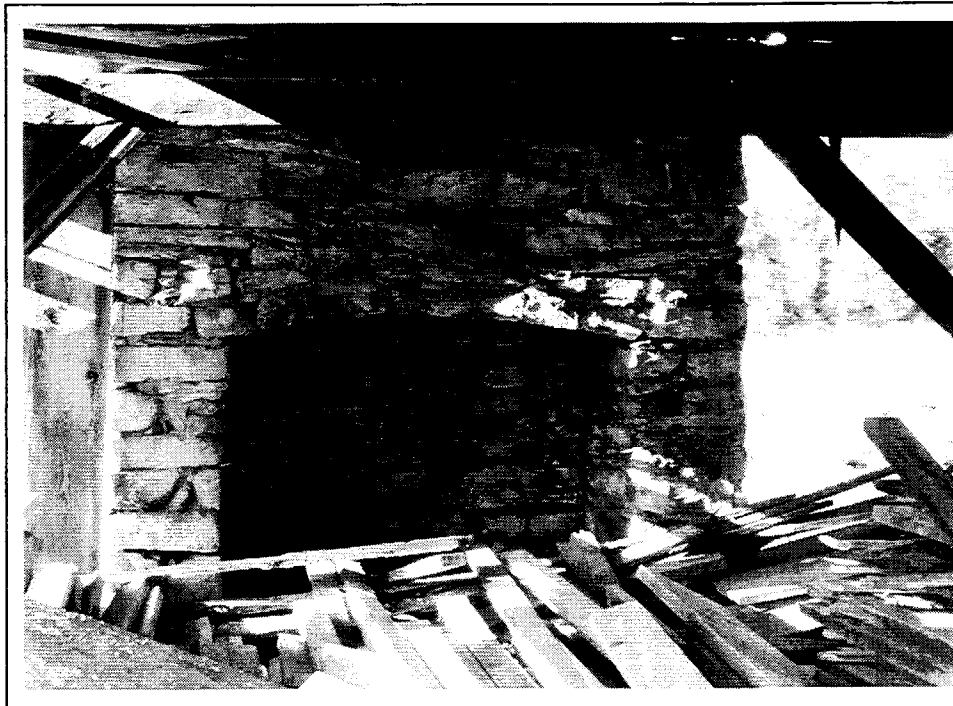
Fig. 23. The wide fireplace in this outbuilding on the Coffman-Hite Farm (069-5009) near Leaksville identifies it as a washhouse or possibly a detached kitchen. The date "1816" is pecked into a stone on the left fireplace jamb.
