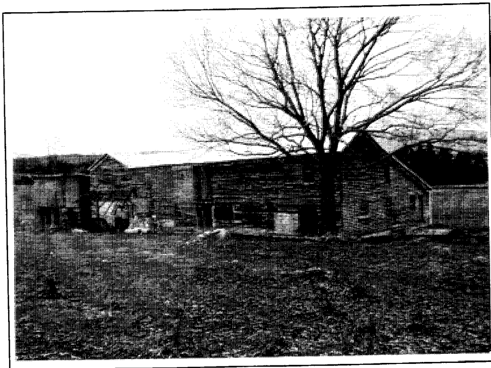
Fig. 41. C. V. Shaffer Cannery (069-5069) near Leaksville.
