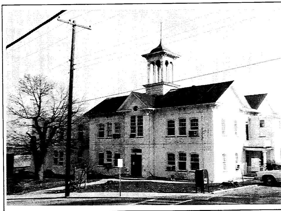
Fig. 46. The 1881 Luray Graded and High School (159-5032) on Court Street in Luray is a remarkably intact large-scale educational building from the era of the town's railroad boom.
