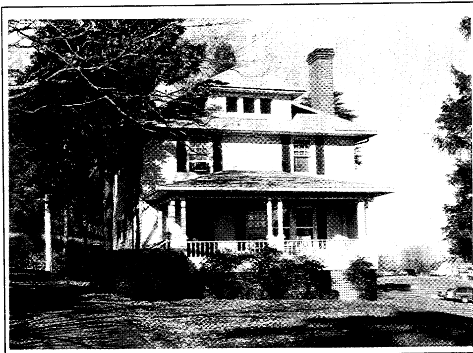
Fig. 53. The Clarence and Mamie Logan House (159-5019), a kit house erected in 1923 at Luray Caverns, epitomizes the new architectural order of the railroad era. The Logan house and its kin were assembled from prefabricated components shipped over the rails from a distant supplier, in this case the mail-order firm Alladin Company.
