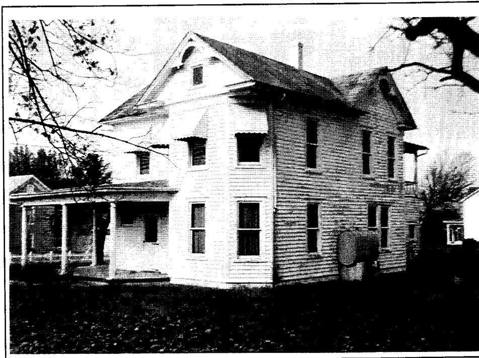
Fig. 56. This house of ca. 1910 on Center Avenue in Shenandoah (069-5107) illustrates several characteristics of Victorian/Queen Anne massing and styling such as the complex roofline, gable ornament, two-story bay window, and wraparound porch.
