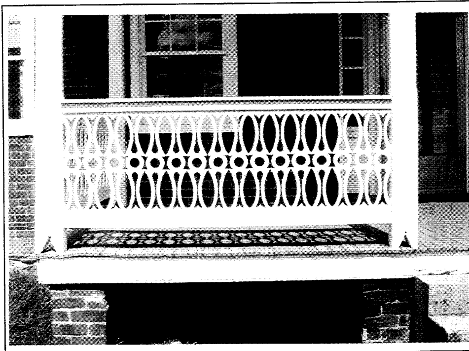
Fig. 55. A delicate porch balustrade on the ca. 1875 James W. Kibler House (069-5092) near Kimball illustrates the advanced woodworking capabilities of the Victorian era.
