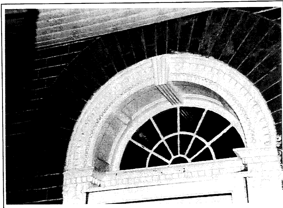
Fig. 28. The intricately detailed fanlight above the entrance to the Peter Ruffner Jr. House (159-5025) in Luray is indicative of the Federal style.
