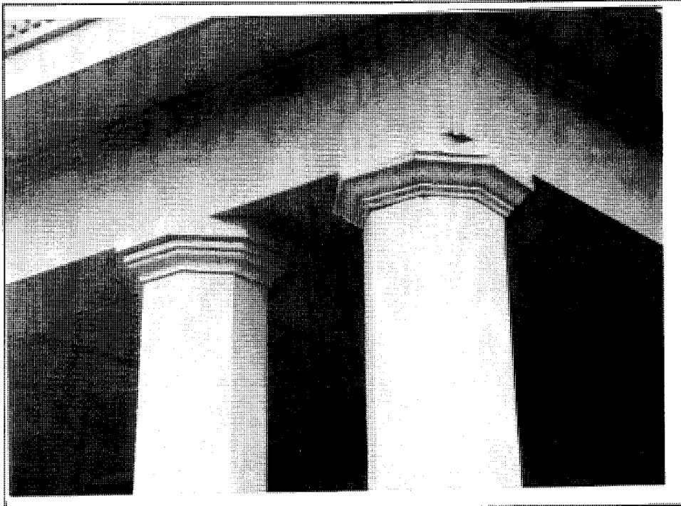
Fig. 33. Porch columns of the farmhouse at Meadow Mills Farm (069-0054).
