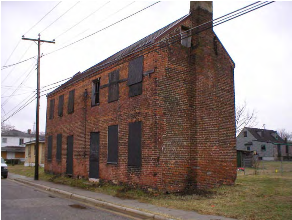
Figure 4. Jarratt House, front (east) façade.
