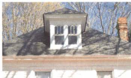
Hipped roof dormer with multi-pane paired windows.
