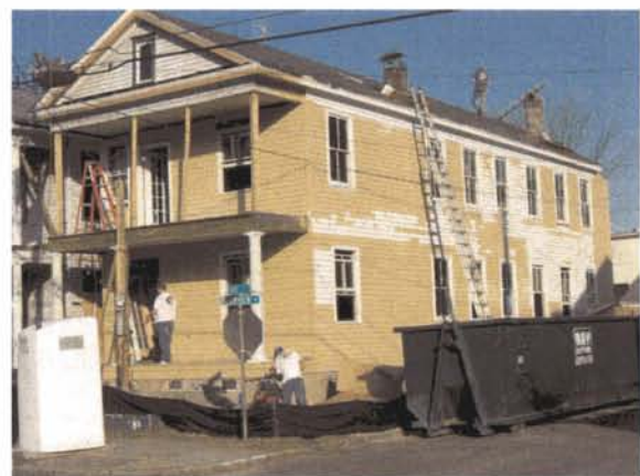
Rehabilitation of this structure in Park View is well underway.
