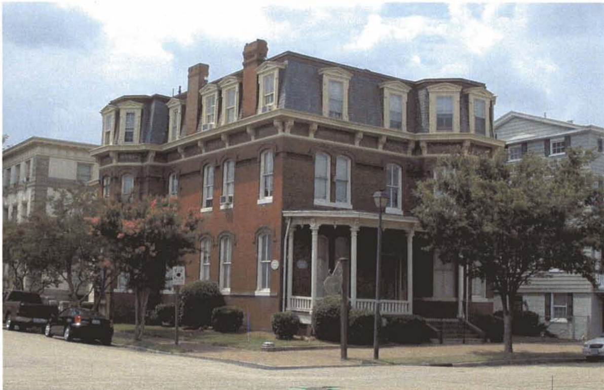
A Second Empire style is characterized by the shingle-clad, third story Mansard roof.
