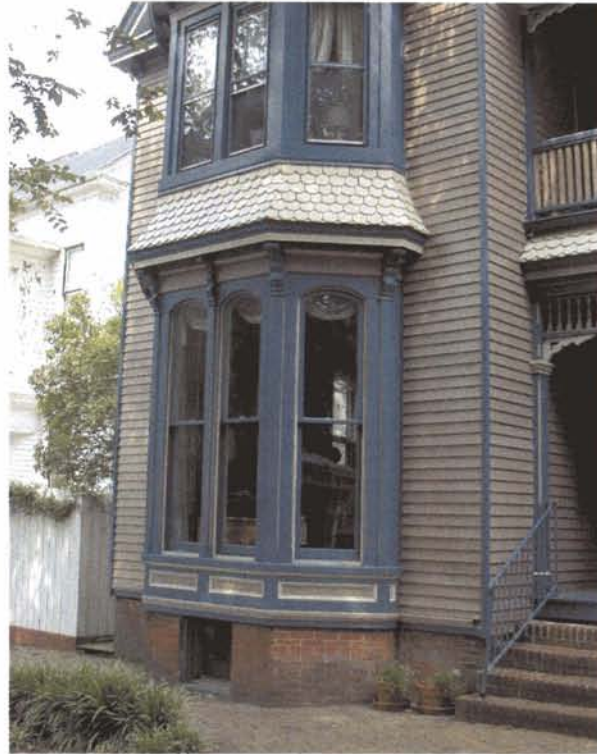
A tall, narrow window bay provides a strong vertical orientation for this Italianate dwelling.
