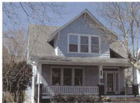
Cross-gable dormer with bracketed eaves.
