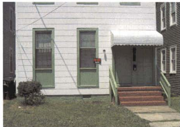
Many modifications lead to a loss of historical integrity.
