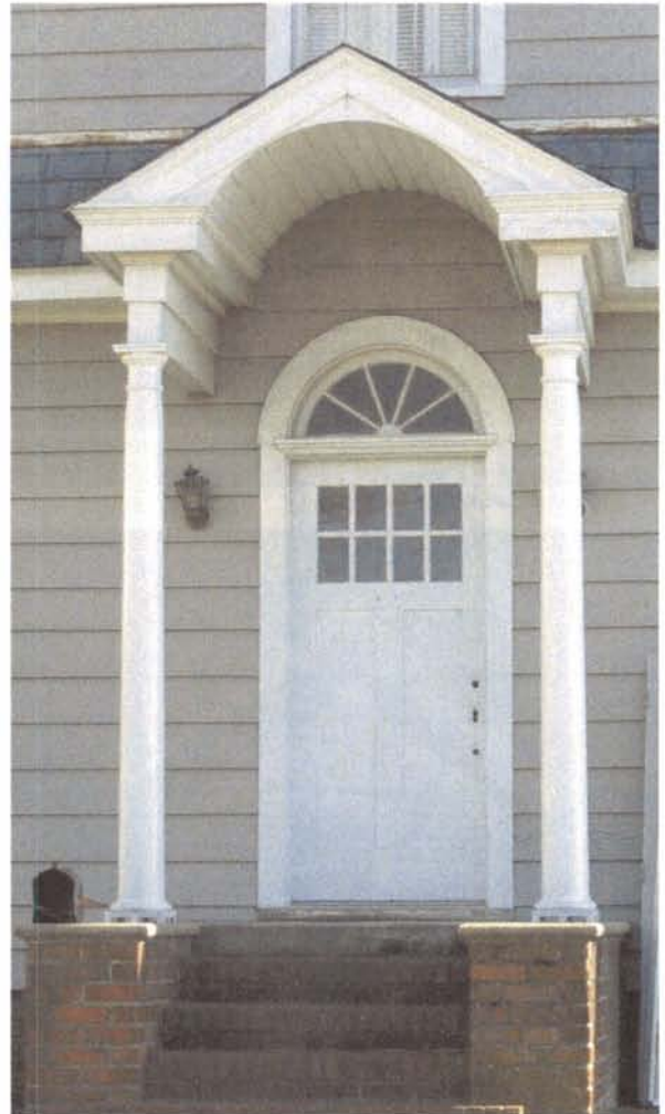
This partially glazed door is capped by a fanlight and sheltered by a classically inspired portico.
