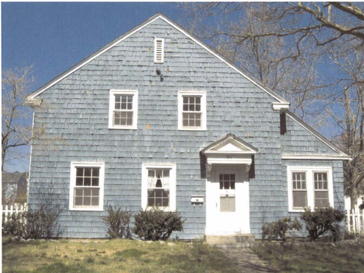
A shingle-clad front-gable house in Cradock retains a high level of historic integrity.
