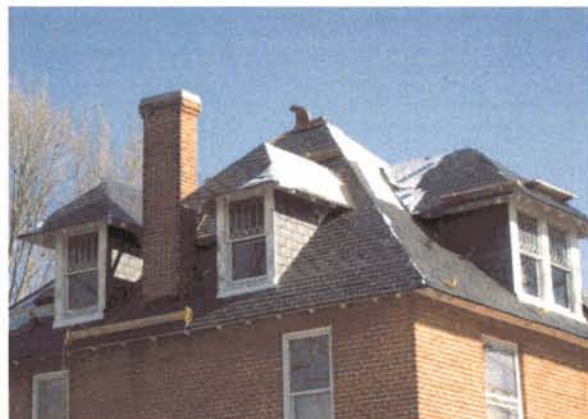
Artificial slate was installed on this roof in the district.
