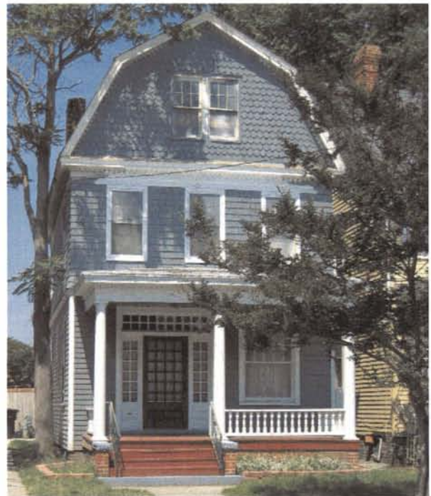
The gambrel roof or Dutch sub-type of the Colonial Revival style shown here is partially clad in shingles more closely associated with the Victorian era.
