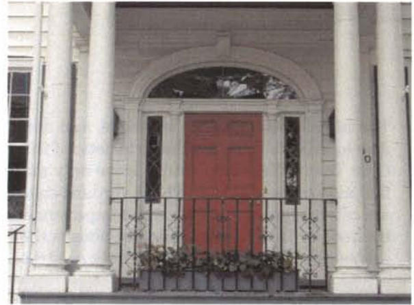
A six-panel door with fanlight and sidelights.
