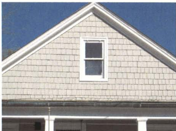
An end-gable clad in wood shingles.
