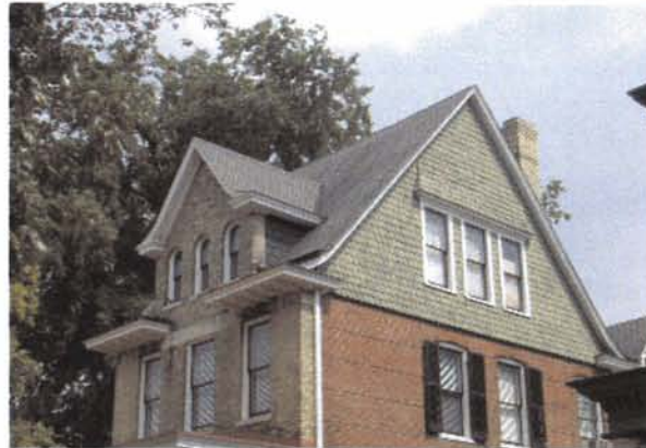
Brick wood and stone provide a symphony of textures on this unique example.
