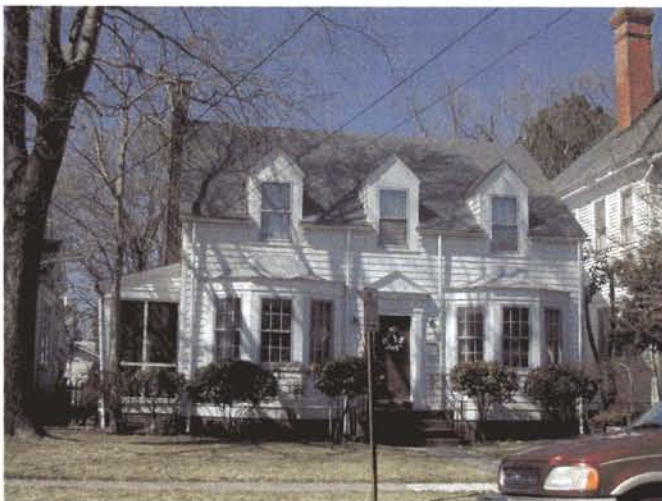
Small-pane bay windows and through-the-wall dormers are typical of the Cape Code variant of the Colonial Revival style.
