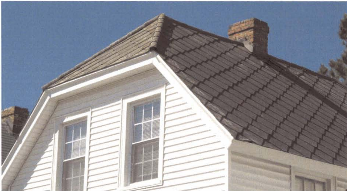
The clipped-gable or Jerkinhead roof is synonymous with Truxtun's architectural identity.
