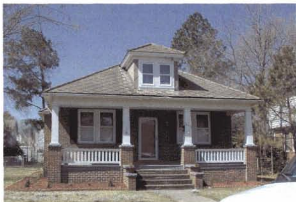
A brick bungalow in Port Norfolk retains a high-degree of historic integrity.
