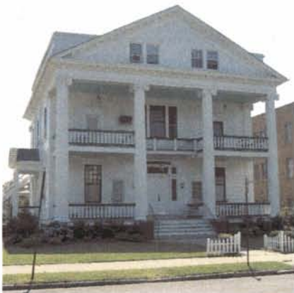
A classically inspired early twentieth-century apartment building.
