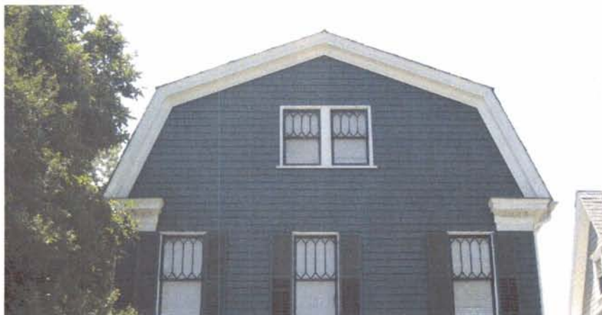
A multi-paned window glazing pattern is an important feature of this Colonial Revival facade.
