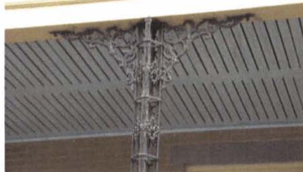
Decorative ironwork should be retained.
