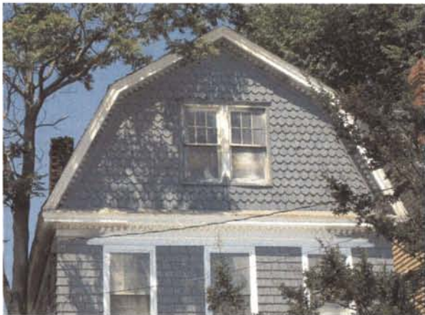
This shingle-clad gambrel end faces onto the street.
