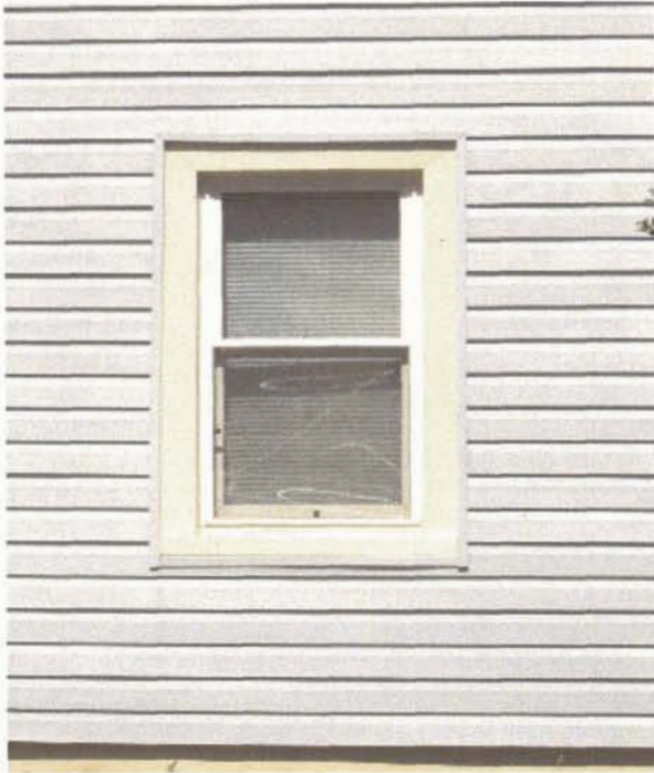
Replacement siding and windows detract from the historic appearance of this house and the district.
