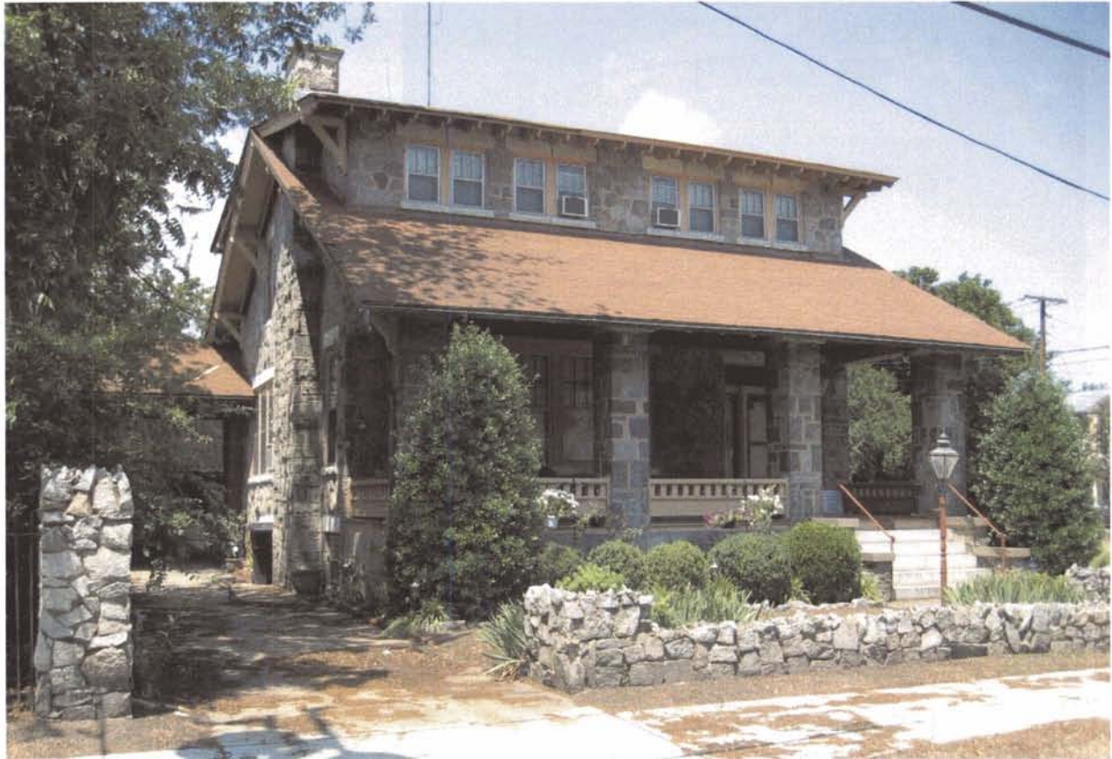
A continuous shed roof dormer is a character-defining element of the only stone bungalow in the district.
