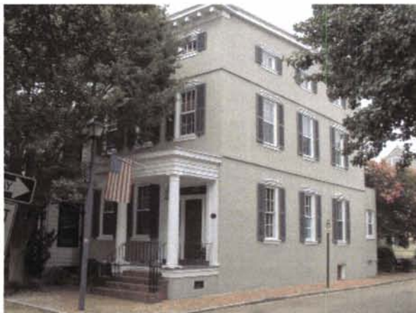
A Greek Revival dwelling clad in stucco and accentuated by horizontal banding.
