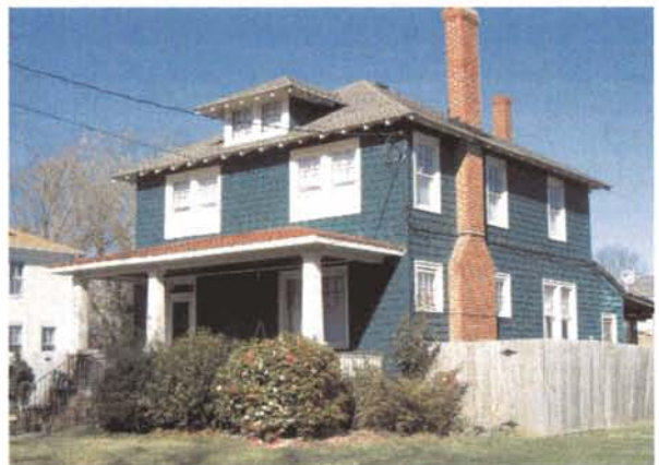
This shingle-clad Foursquare has bracketed eaves and a red tile porch roof.
