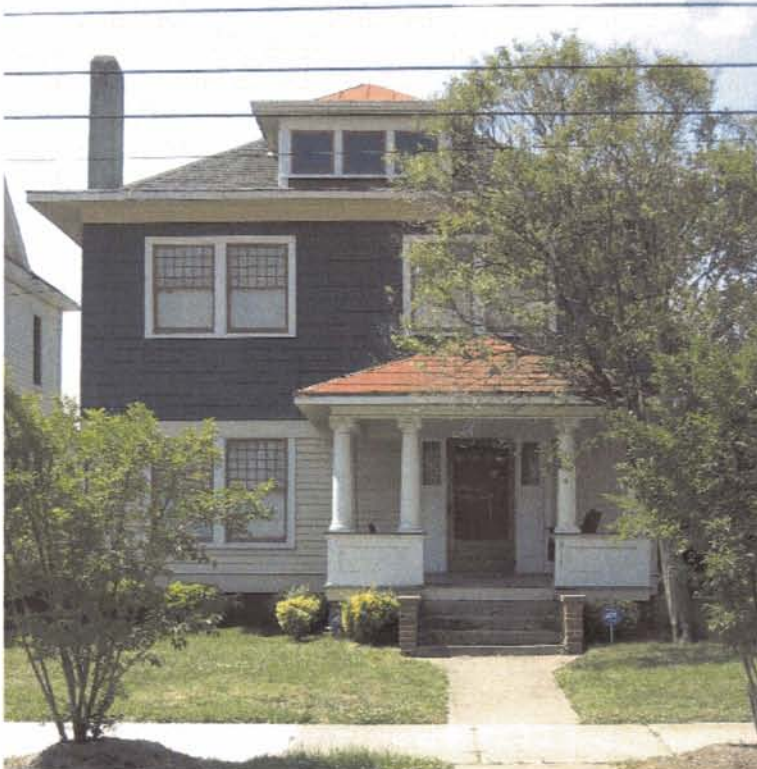
A more high-style example, this Foursquare is defined by its shingled second level and twenty-four over one window glazing.
