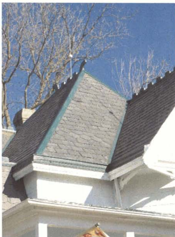
Metal roof cresting and patterned slate roof.
