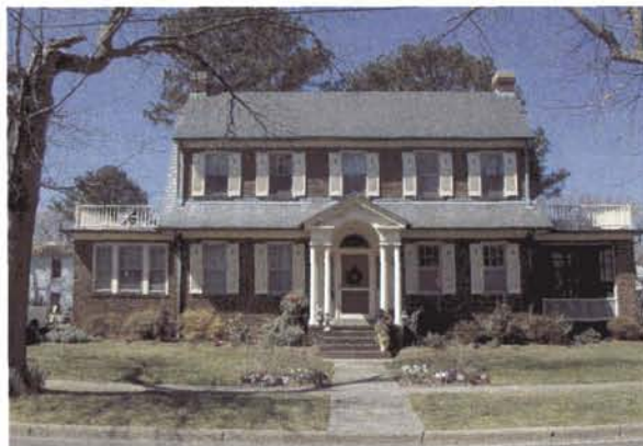
This Colonial Revival house appears to retain many of its original character-defining features.
