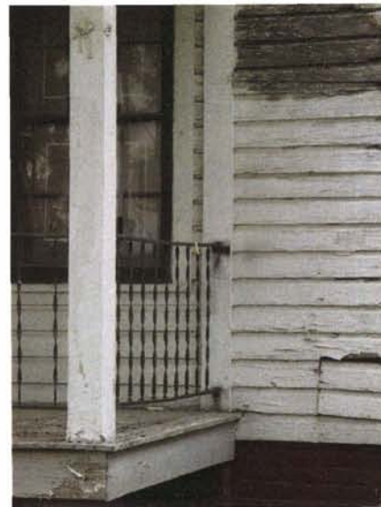
Wood needs constant maintenance. By keeping siding and trim repaired and painted, you can protect these features from moisture penetration.
