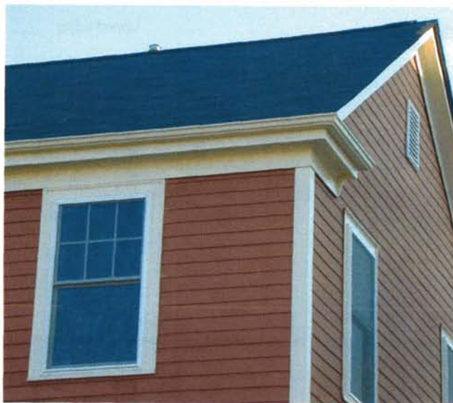
New construction outside of the historic district has successfully used substitute materials, such as cementitious siding and trim details, to achieve a traditional appearance.
