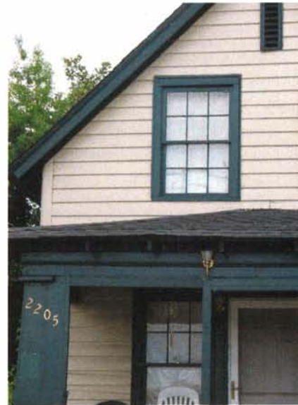
This house retains many original wood elements including windows, window and porch trim, siding and exposed rafter ends.
