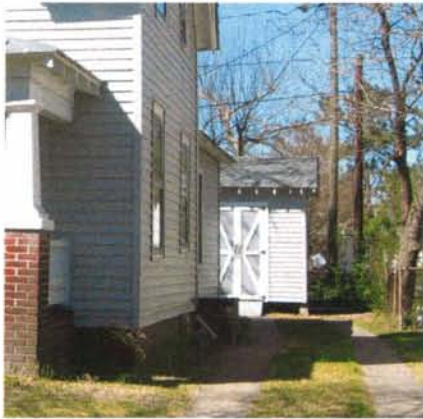
A shed repeats the colors and materials of the main structure and even the exposed rafter detail.
