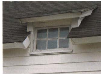
Original dormer windows in Truxtun were six-light casement windows.
