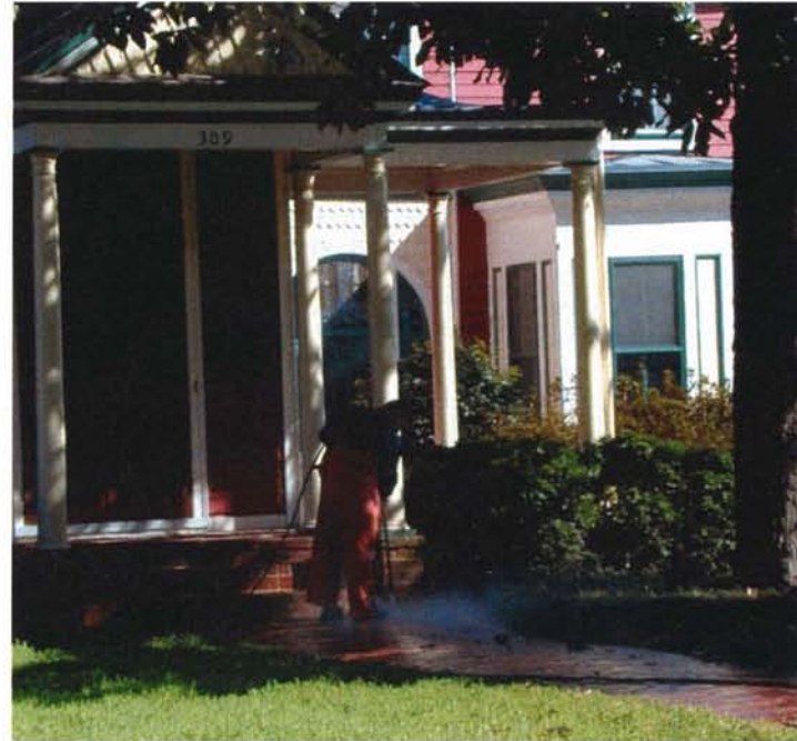
Low-pressure power-washing can be an environmentally sensitive approach to cleaning historic masonry.
