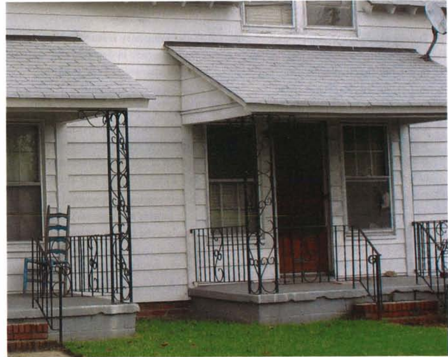
Many of the Truxtun house porch posts and railings have been replaced with decorative metal work that detracts from the historic character of the district.
