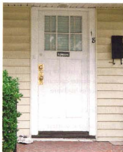
Wooden doors with six glass panes over two vertical wooden recessed panels were the standard original front and back doors in Truxtun.
