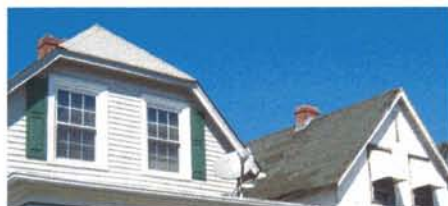
Roof shapes in Truxtun are either Jerkinhead (left) or gable (right).
