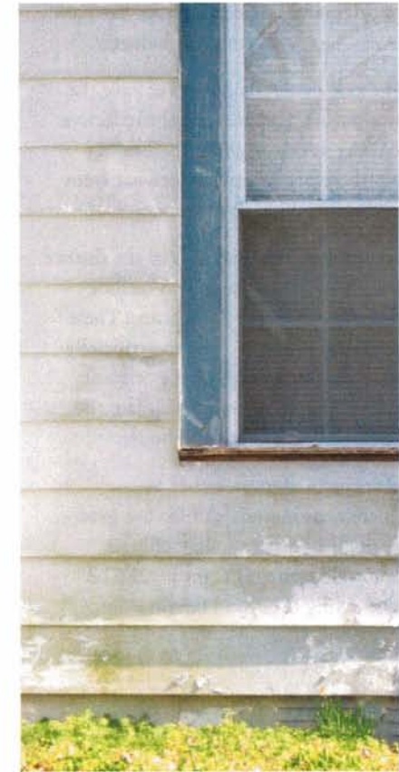
Often, the effects of cleaning or painting vinyl siding can leave the siding with an uneven appearance.
