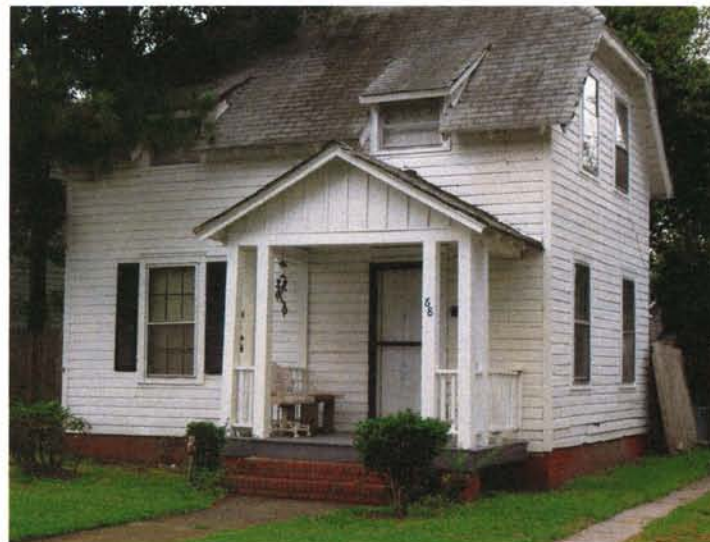
This Truxtun house retains its original wood siding, porch materials and configuration and six-over-six wooden windows. The roof materials and fixed shutters are not original.
