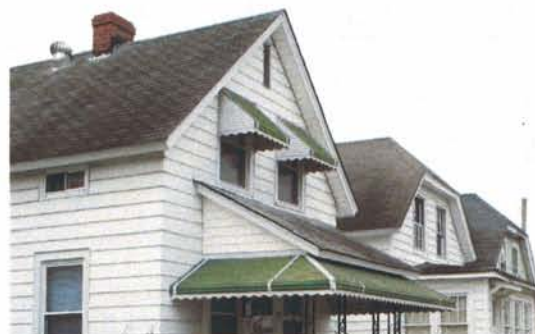
Low-contrast, darkly colored asphalt shingles provide an appearance similar to the original asbestos roofs found in Truxtun.
