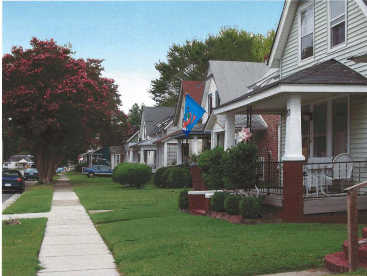
This block view shows many elements typical of the site character in the Truxtun Historic District including small front yards with mature plantings.
