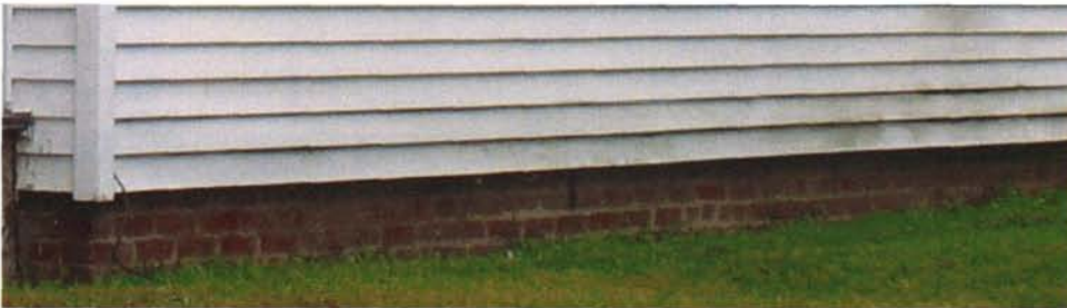
A low, unpainted brick foundation is an original characteristic of Truxtun houses.
