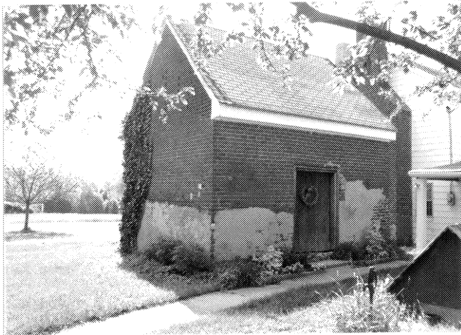
Figure 43: Smokehouse at Liberty Hill Farm (72-108), East Elevation Source: Tracerics, 1991
