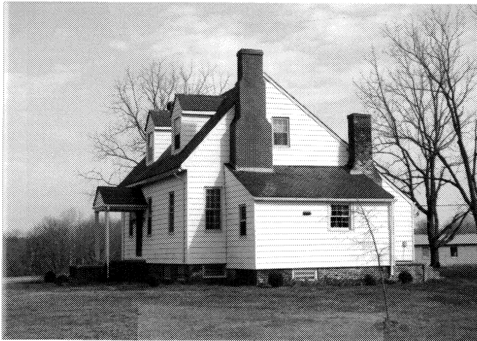
Figure 13: Somerset (72-40), East Elevation Source: Tracerics, 1991
