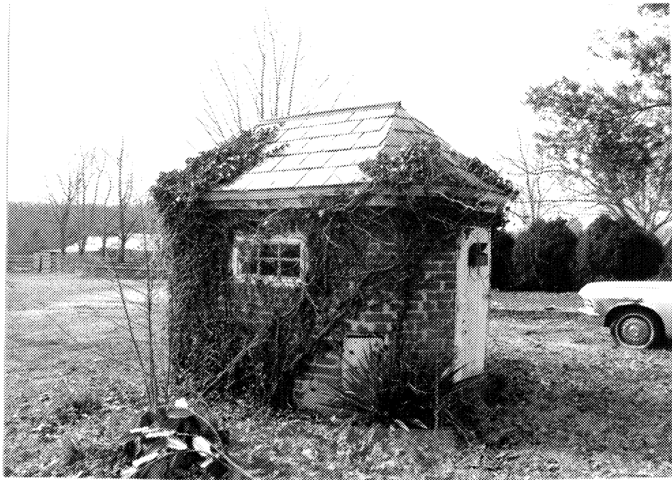
Figure 46: Spring House at Hughes Creek (72-71), West Elevation Source: Traceries, 1991
