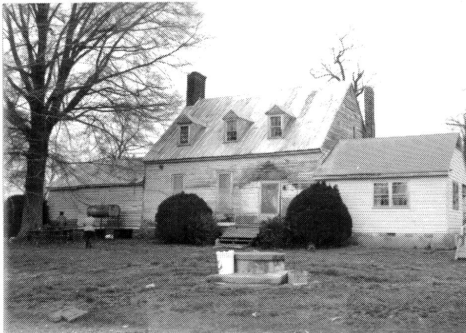
Figure 53: Dispatch (72-10), East Elevation Source: Tracerics, 1991
