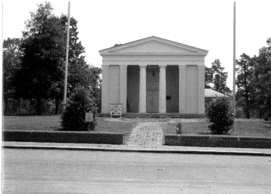
Figure 52: Powhatan Courthouse (72-68), West Elevation Source: Tracerics, 1991
