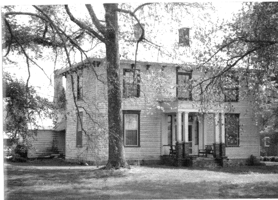
Figure 75: New Castle Farm (72-115), North and West Elevations Source: Tracerics, 1991
