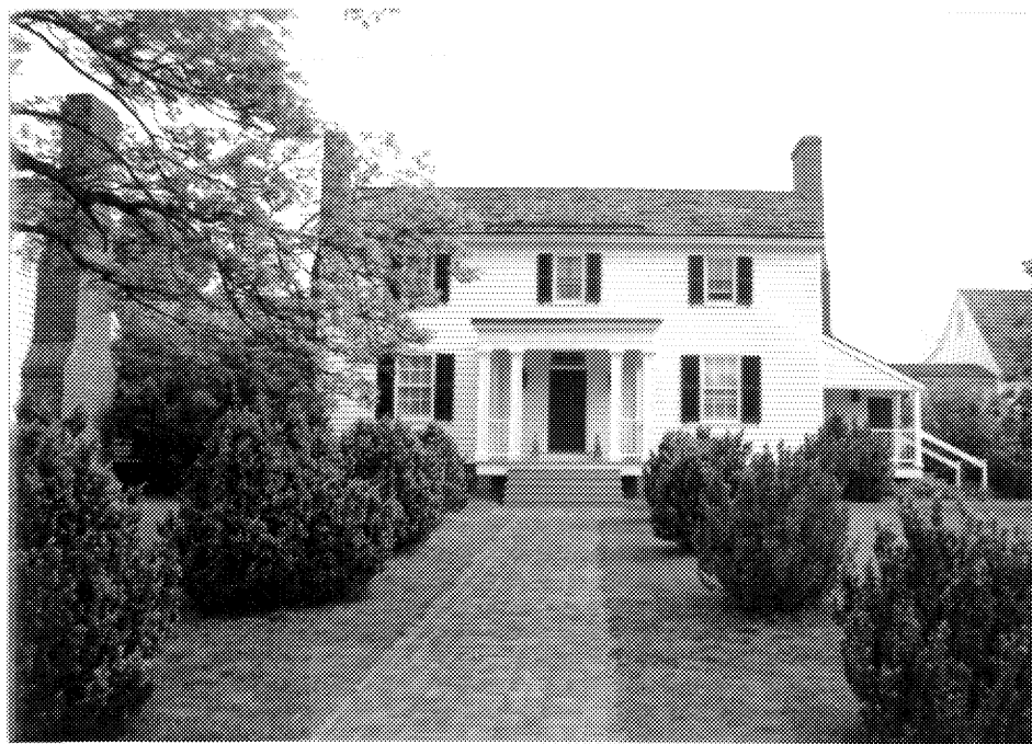
Figure 15: Derwent (72-9), South Elevation Source: Tracerics, 1991
