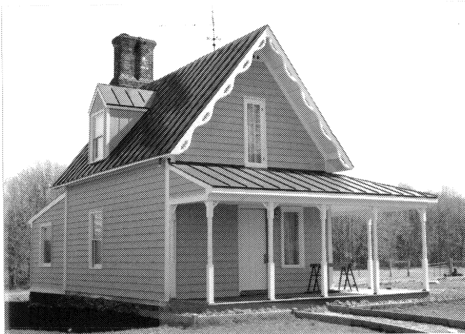
Figure 33: Cottage at Brooklyn (72-67), North and West Elevations Source: Tracerics, 1991
