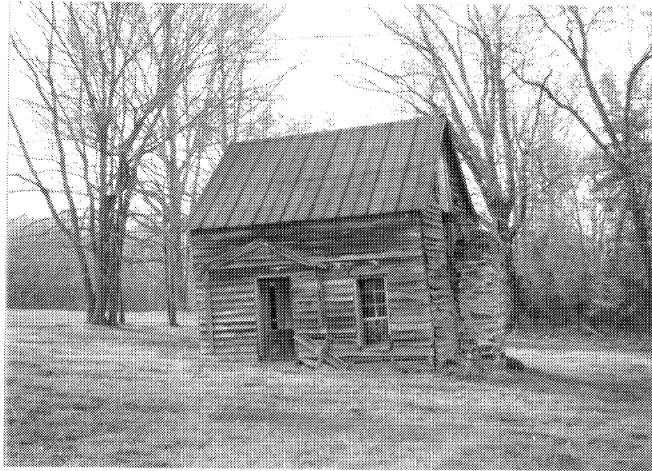
Figure 41: Slave Quarters at Whitewood (72-88), West Elevation Source: Tracerries, 1991
