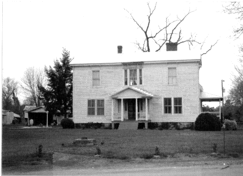
Figure 62: Macon Tavern (72-227), East Elevation Source: Traceries, 1991
