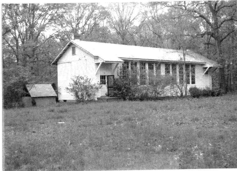
Figure 54: School near Subletts (72-313), North and East Elevations Source: Tracerics, 1991
