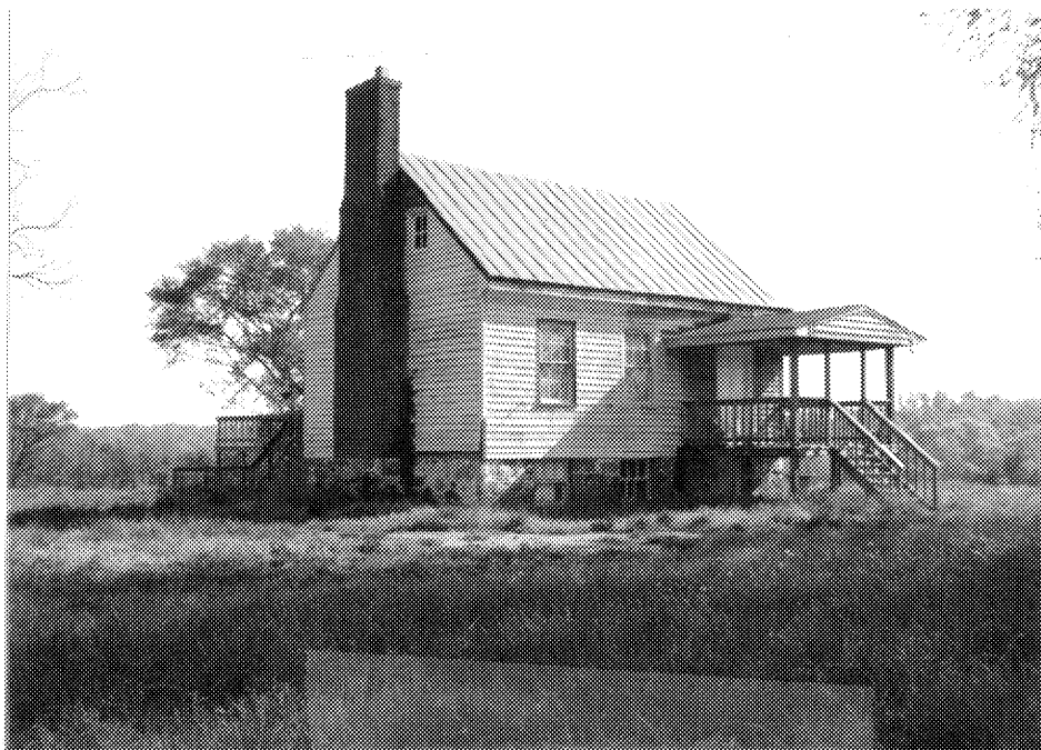
Figure 14: Center Hill (72-5), South and West Elevations Source: Tracerics, 1991
