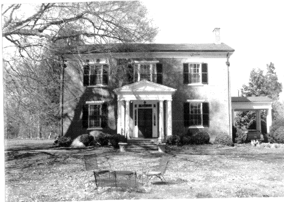
Figure 23: Mill Quarter Plantation (72-27), South Elevation Source: Traceries, 1991
