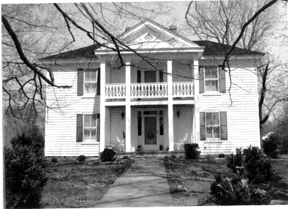
Figure 70: Birdland Farm (72-255), South Elevation Source: Tracerics, 1991
