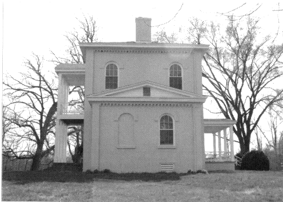
Figure 35: Fighting Creek (72-15), North Elevation Source: Tracerics, 1991
