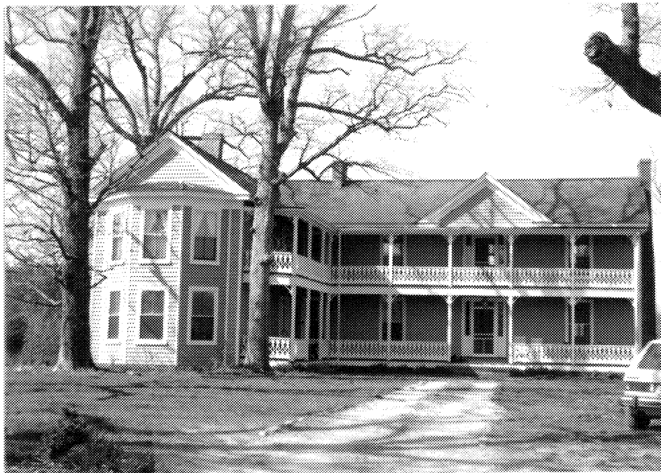
Figure 19: Rudd House (72-242), South Elevation Source: Tracerics, 1991
