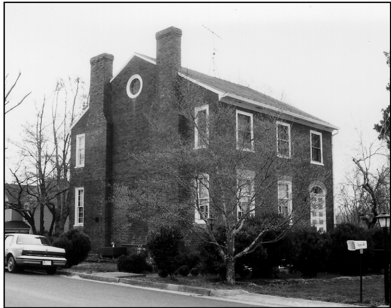
Figure 22: Hugh Weir House
