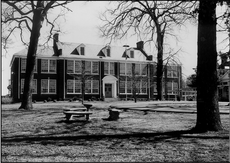
Figure 31: Chatham Elementary School
