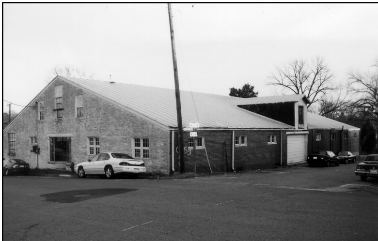
Figure 35: Building, 14 Pruden Street
