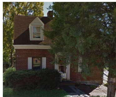
939 Paxton St. (108-5853) Colonial Revival Cape Cod, ca. 1941
