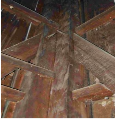
Timber framing inside Nuckols Barn 1
