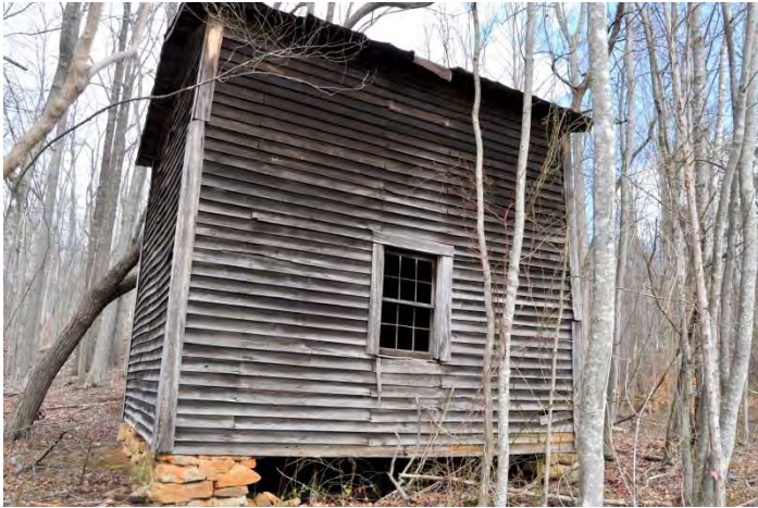
A one-room, wood-framed pack barn in Pittsylvania County.
