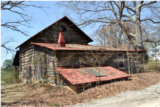
A log and frame pack barn in Pittsylvania County showing various rooms and roof configurations. The partially below-ground, shed-roofed section in the foreground is the stripping room and the ordering pit is under the center section.
