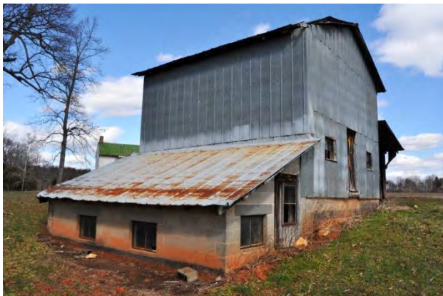
A mid- 20 th century wood-frame and concrete block pack barn in Pittsylvania County. The shed-roofed section is the stripping room.
