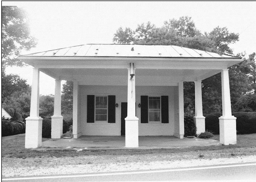
Figure 128. Jenkins Bus Station, Main Street (322-0011-0025)
