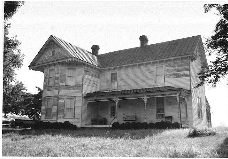
Figure 41. House, 1188 F.T. Valley Road (078-5065)
