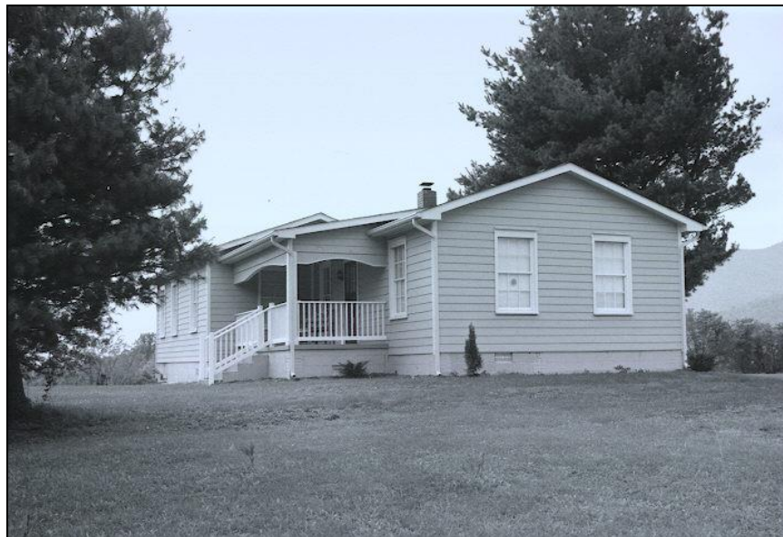
Figure 110. Rose Cottage, Dearing Road (078-5109)
