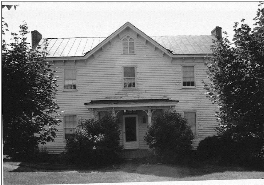
Figure 34. House, 3594 Slate Mills Road (078-5076)
