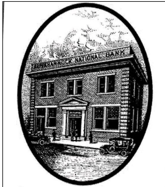
Figure 68. Rappahannock National Bank in Washington (322-0011-0051)
