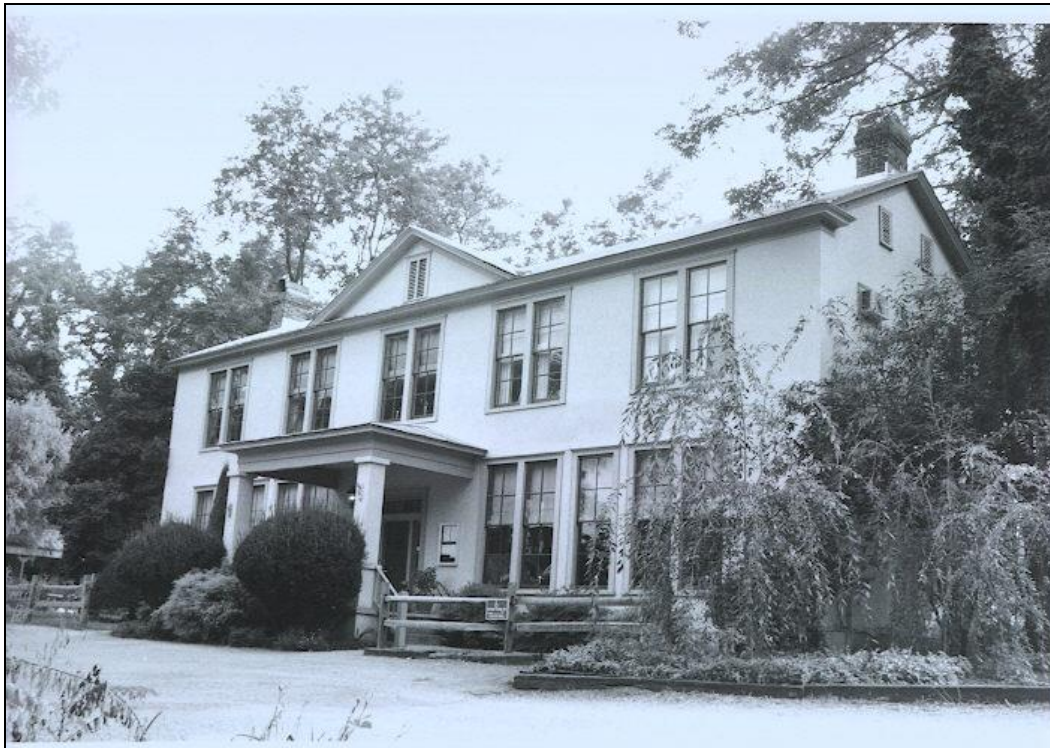
Figure 50. Flint Hill School (078-5018-0008), 2002 Survey Photograph
