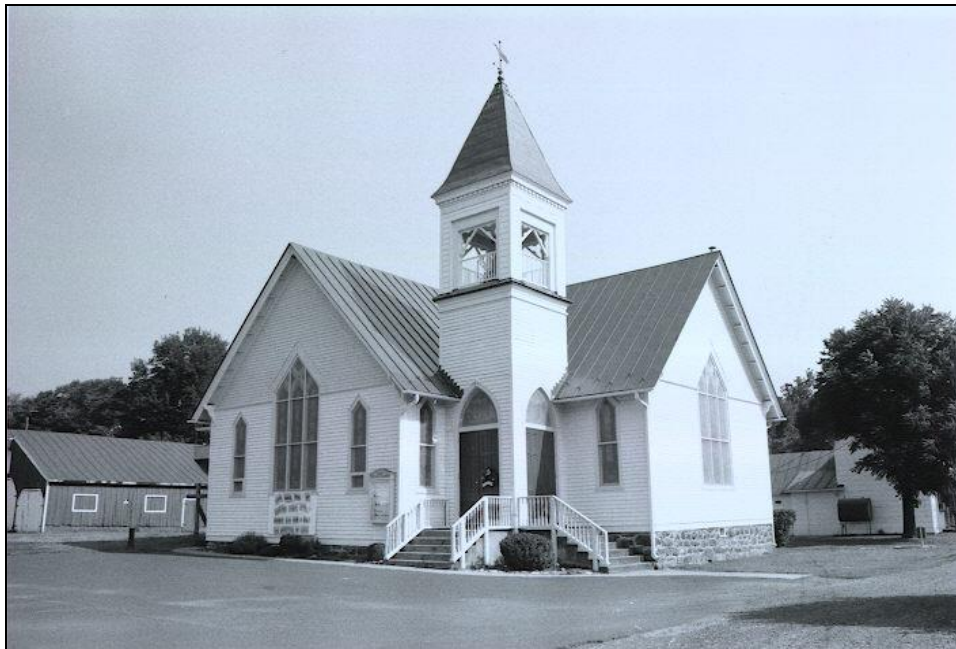
Figure 115. Sperryville United Methodist Church (078-0093-0034)
