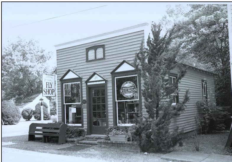
Figure 57. Commercial Building, Sperryville (078-0093-0047)
