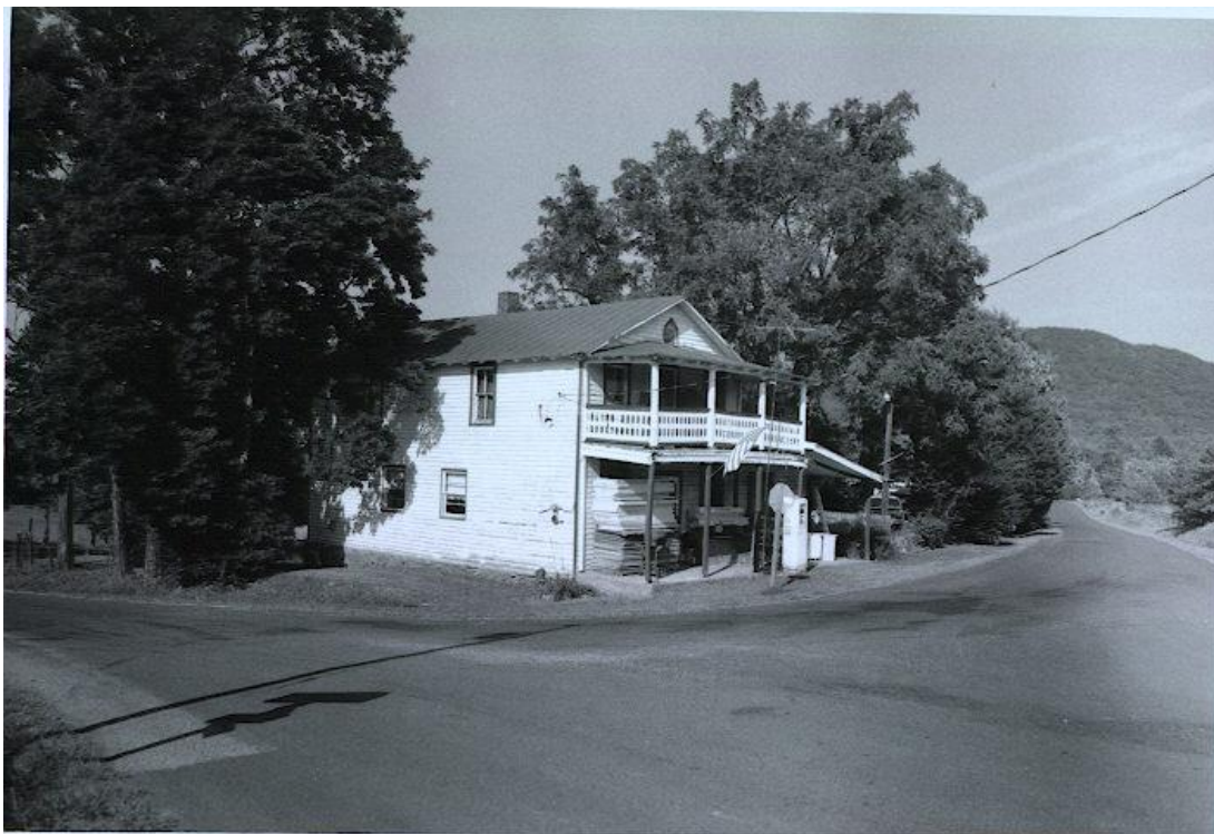
Figure 66. Store/Dwelling at 3 Castleton View Road (078-5101)
