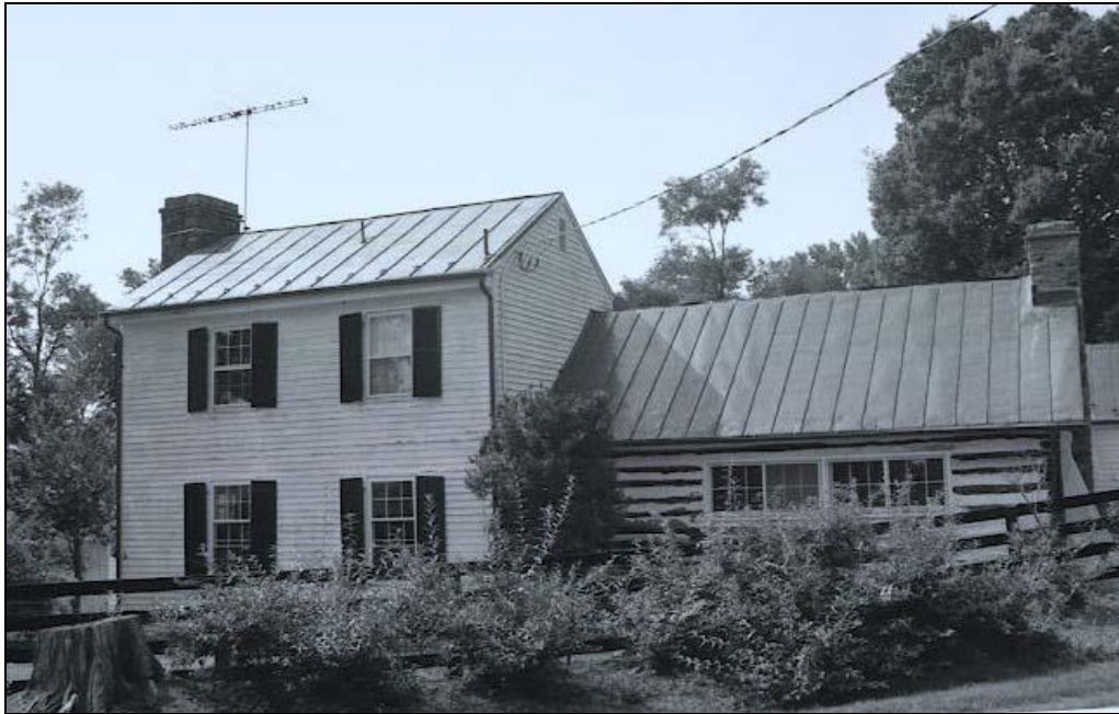
Figure 122. Keysville Post (078-5022) with Original Mule Barn Wing
