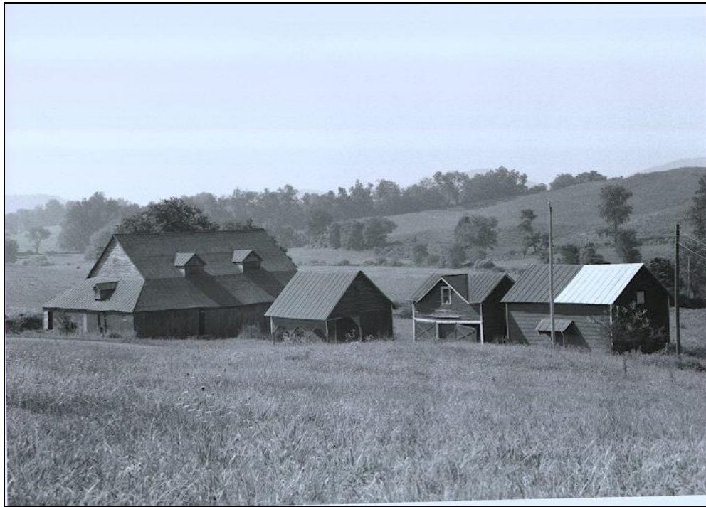
Figure 121. Miller House (078-5067), Tobacco Barn and other Farm Buildings
