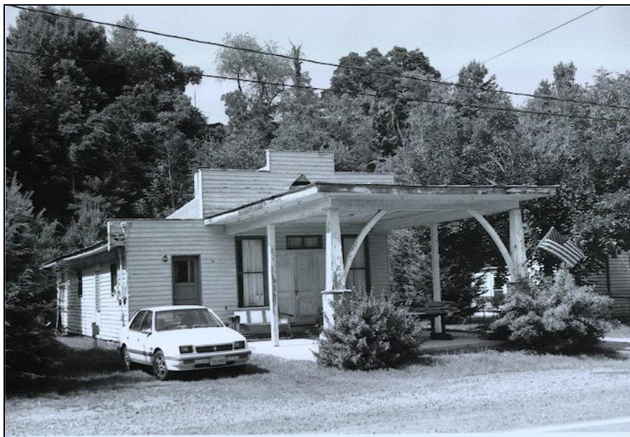
Figure 67. Service Station, 12004 Lee Highway (078-5042)
