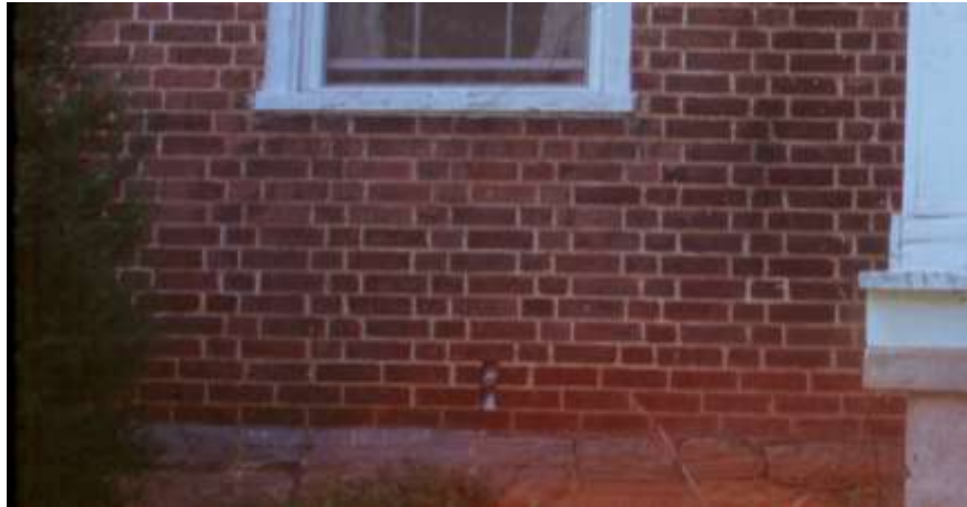
Figure 1: Staggered Flemish Bonding
