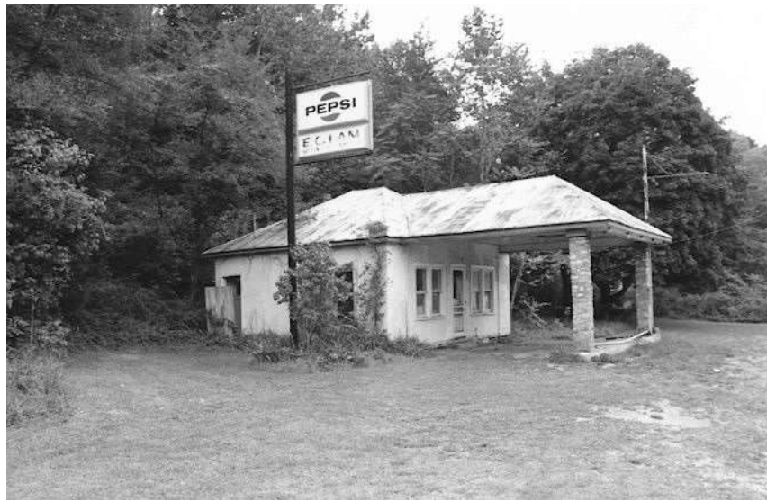
Figure 21: Service Station at 18700 Spotswood Trail (082-5180)
