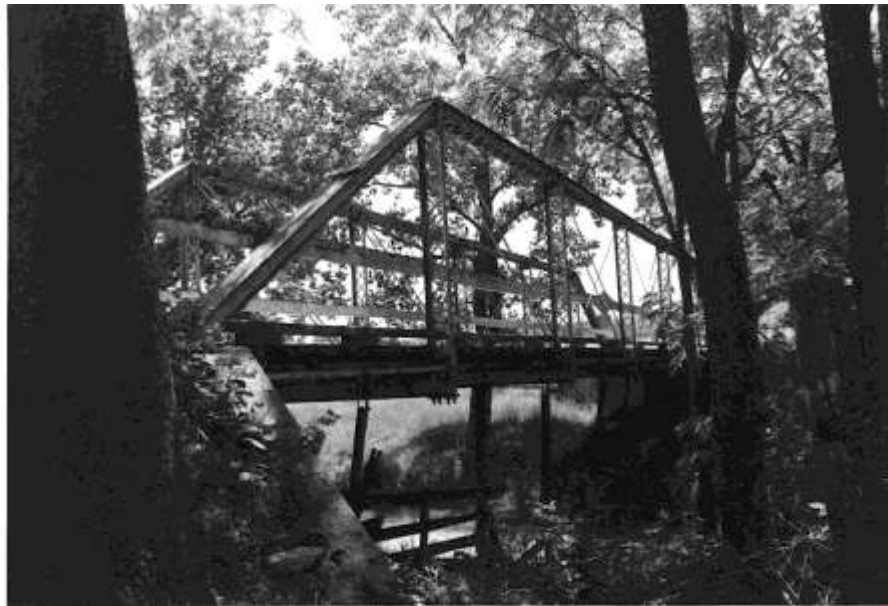
Figure 45: Bridge on Williamsburg Road (082-5020)
