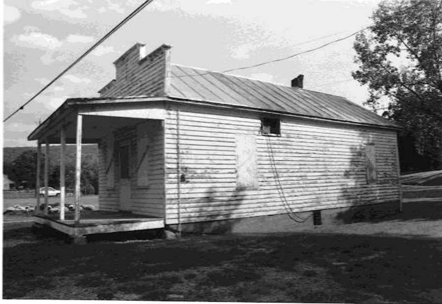
Figure 24: Store at 19968 Naked Creek Road (082-5167)
