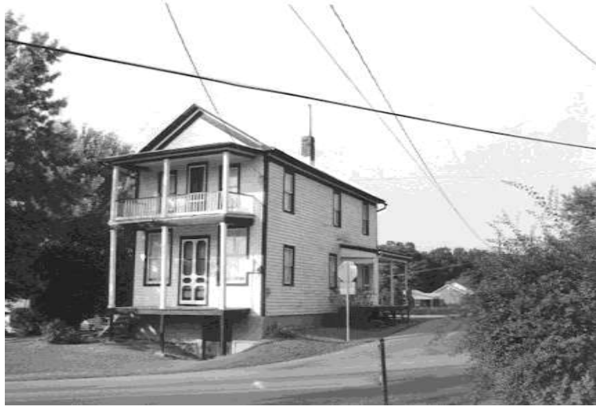
Figure 26: Store/Dwelling at 2619 Newtown Road (082-5169)
