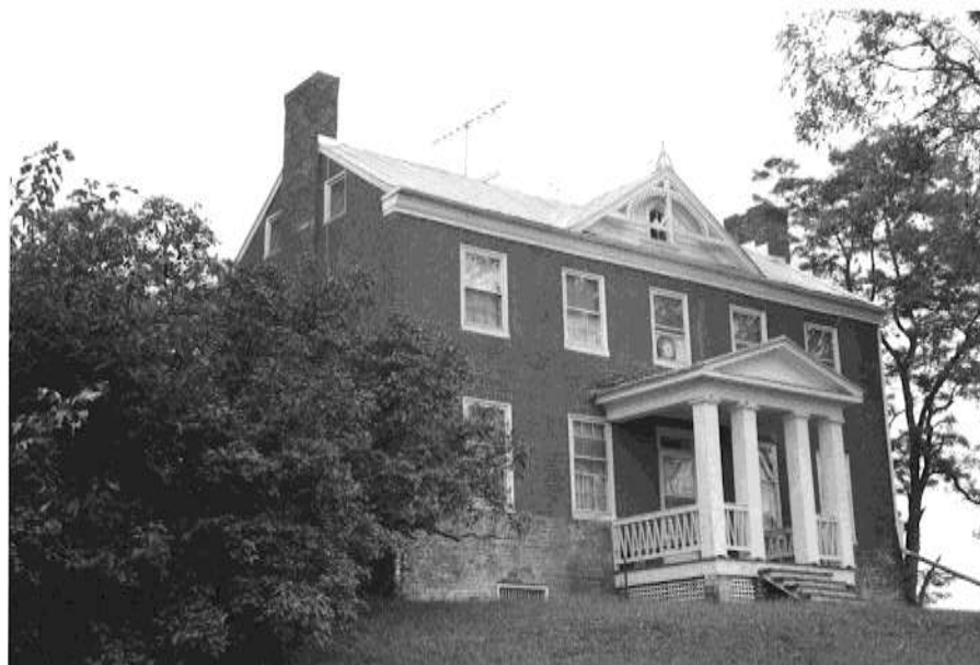
Figure 10: House at 8254 Ironhorse Road (082-5105)
