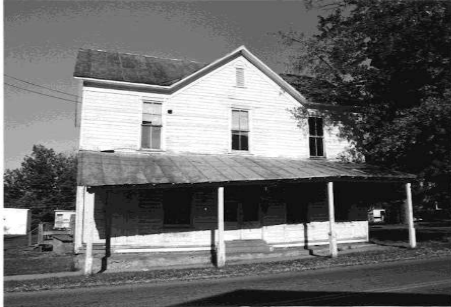
Figure 13: Store/Dwelling at 401 Aspen Avenue (228-5001-0010)
