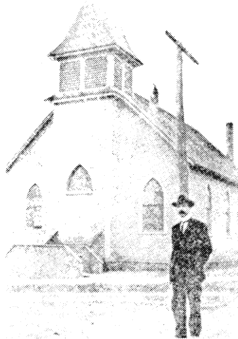
Figure 13: Belmont Methodist Church Building
