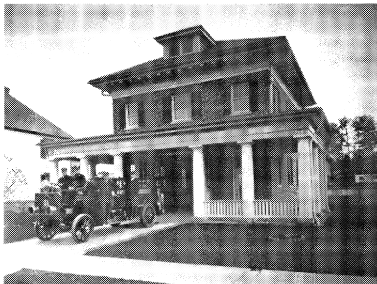
Figure 12: Belmont Fire Station Number 6 (Roanoke City Firehouse)
