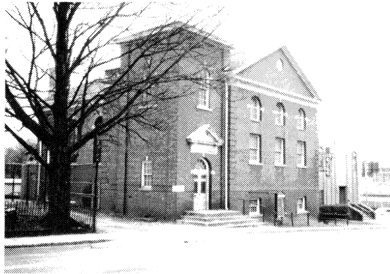
Figure 53: First Methodist Church, 407 Tazewell Avenue
