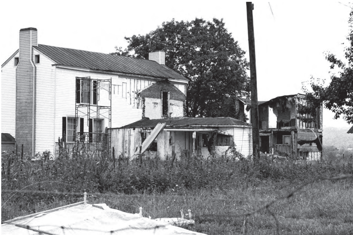
Figure 95. Slave quarters, Fields House (083-5094), Route 628, Old Castlewood (2008).
