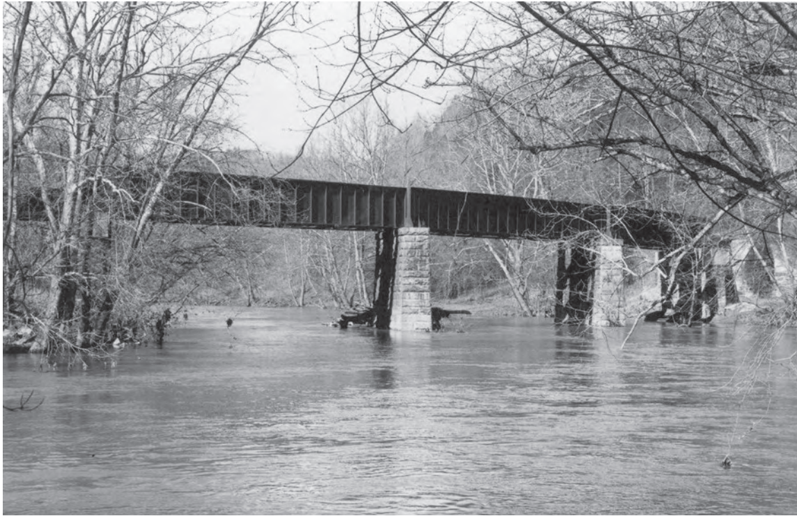
Figure 197. Railroad bridge (083-5207), Red Oak Ridge Road, Clinch River (2008).
