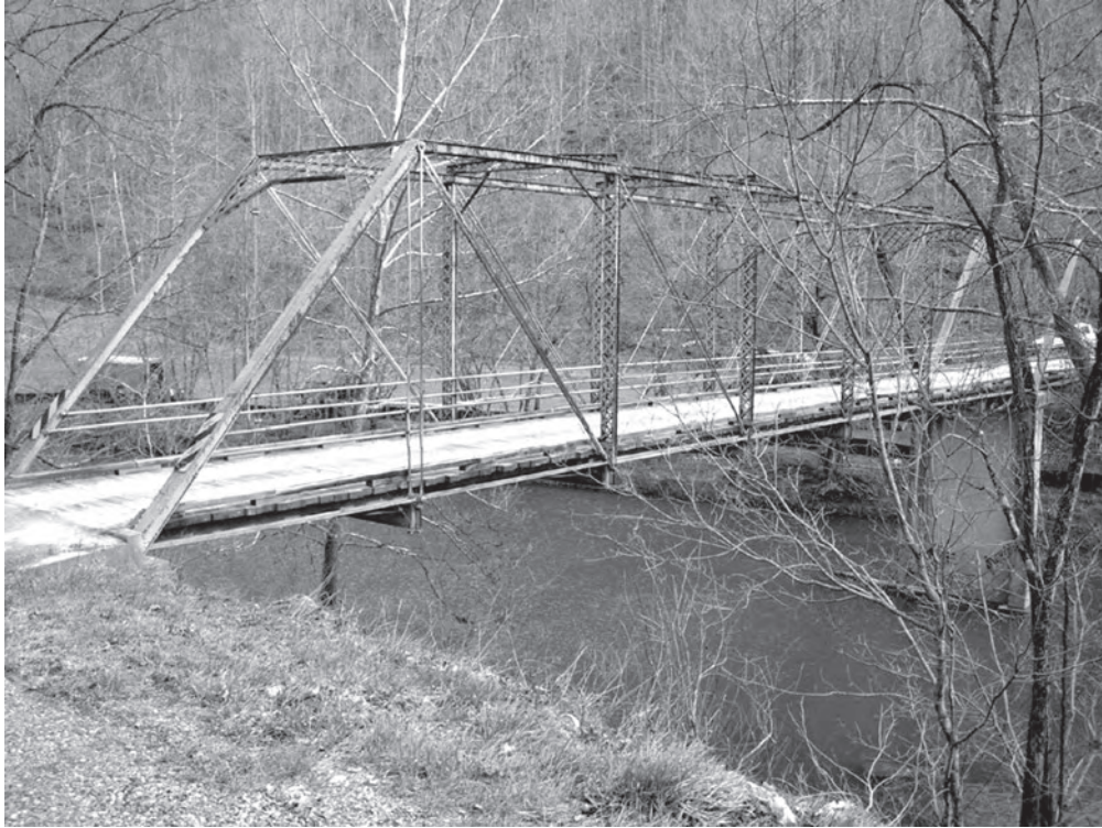
Figure 187. Iron truss bridge (083-0060), Route 652, Puckett's Hole (2008).
