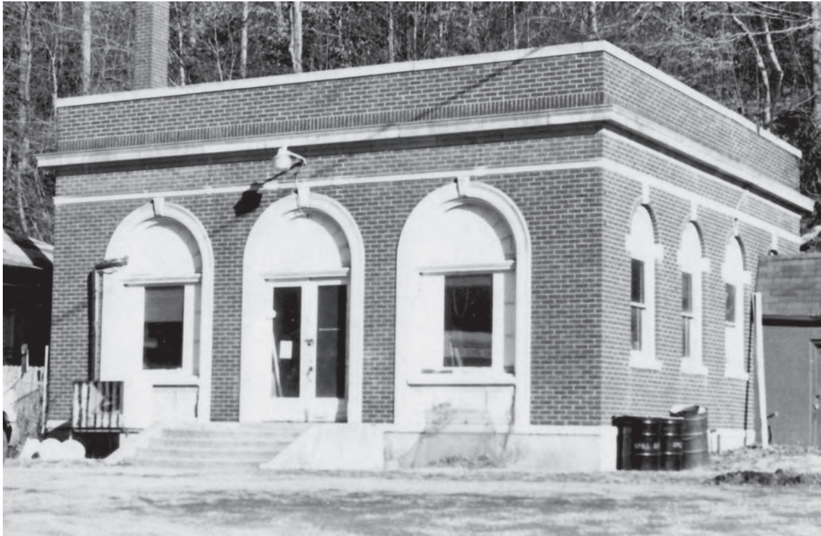
Figure 129. Dante Bank Building (083-5119), Dante (2001).
