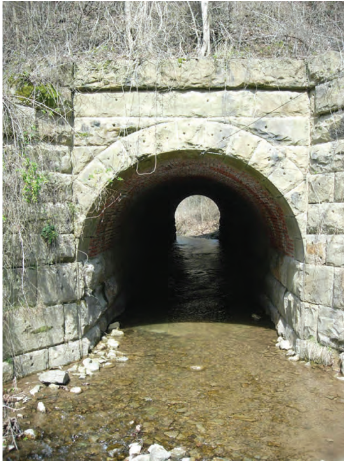
Figure 191. Thompson Creek Tunnel #5 (083-5061), Thompson Creek Road, near Honaker (2008).
