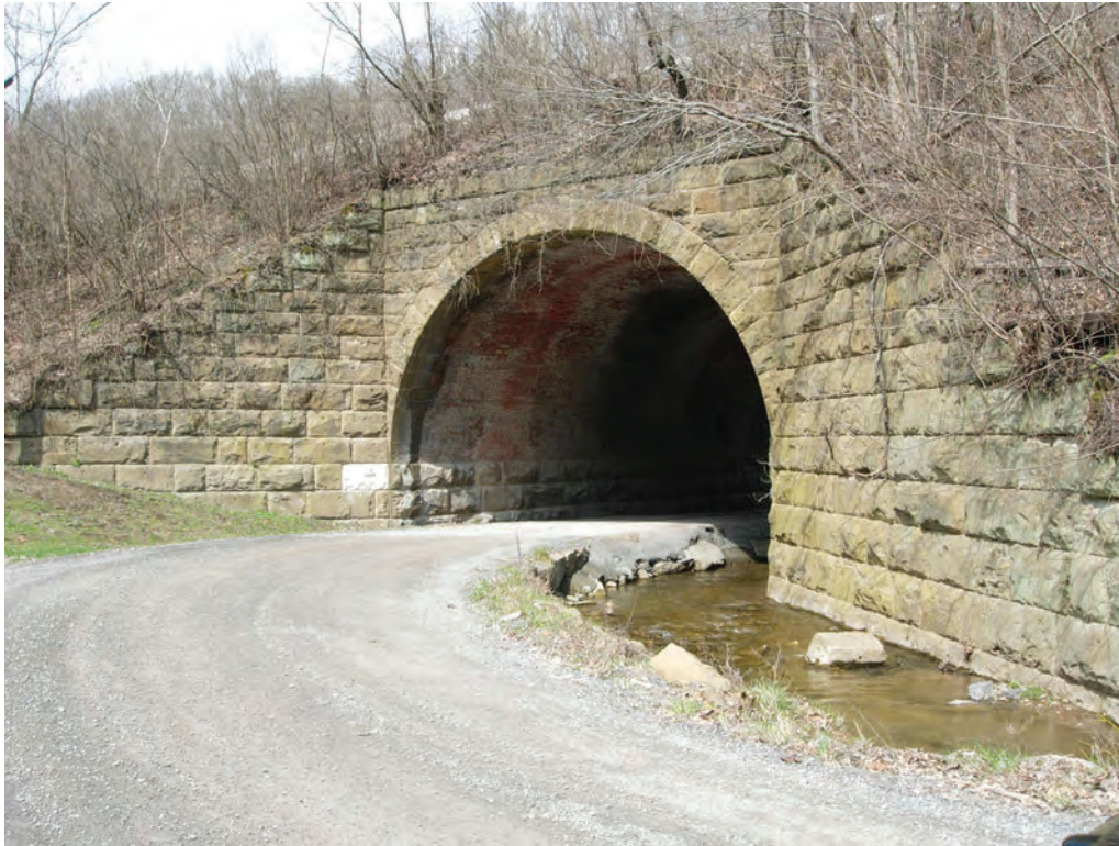
Figure 98. Thompson Creek Tunnel (083-5014), Thompson Creek Road (2008).
