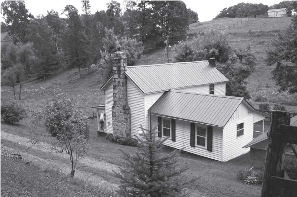
Figure 54. I-house (083-5282), Route 606, Moccasin Valley (2008).
