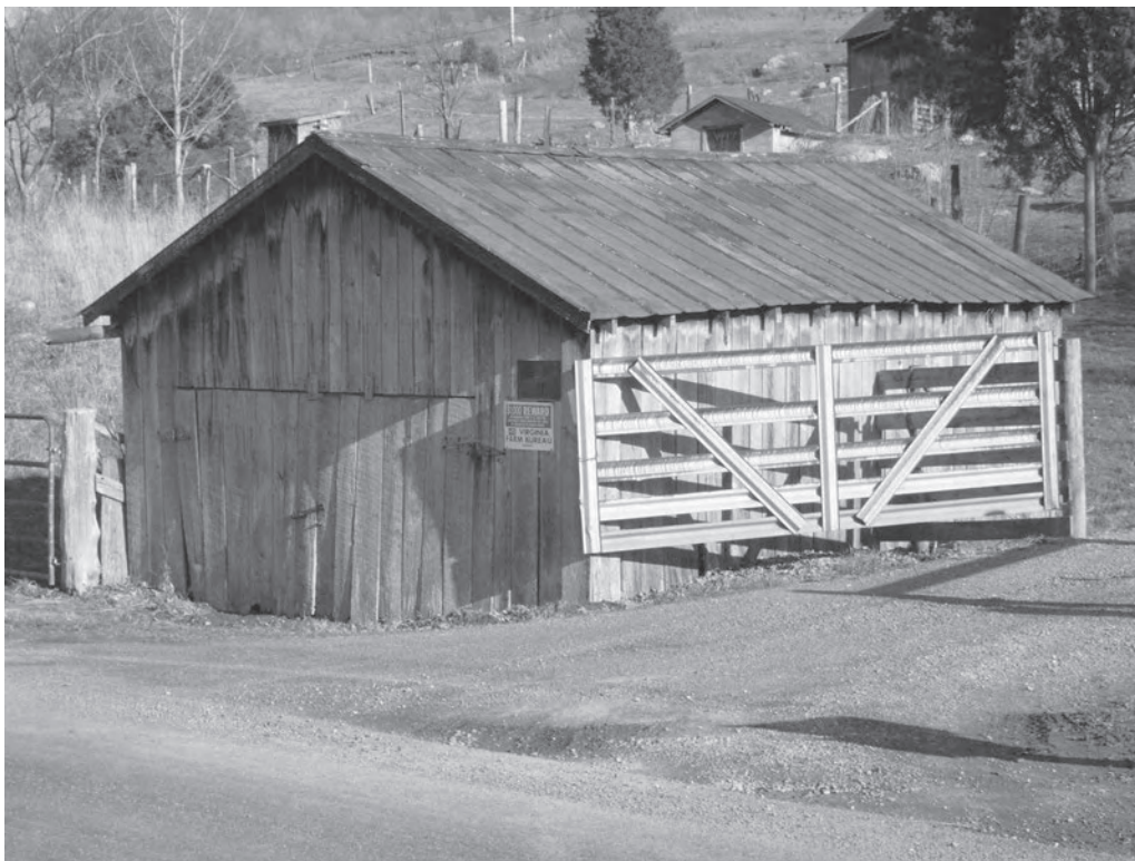
Figure 178. Barn (083-5222), Green Valley Road, Elk Garden (2008).
