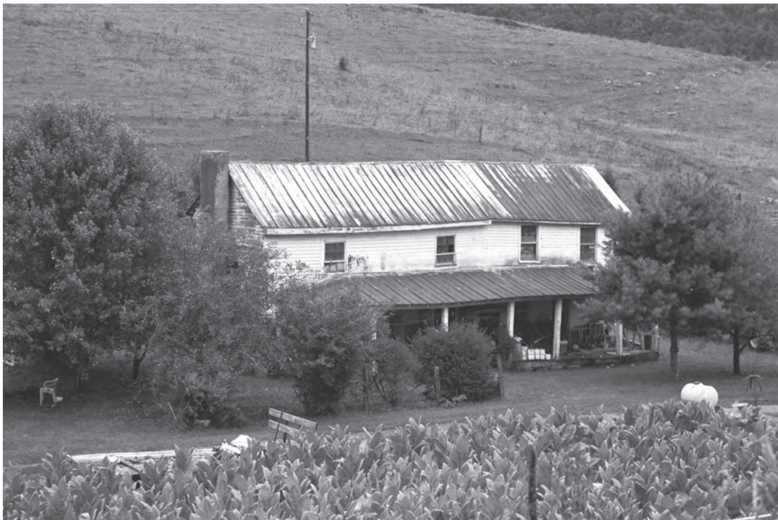
Figure 59. I-house (083-5289), Route 613, Moccasin Valley (2008).
