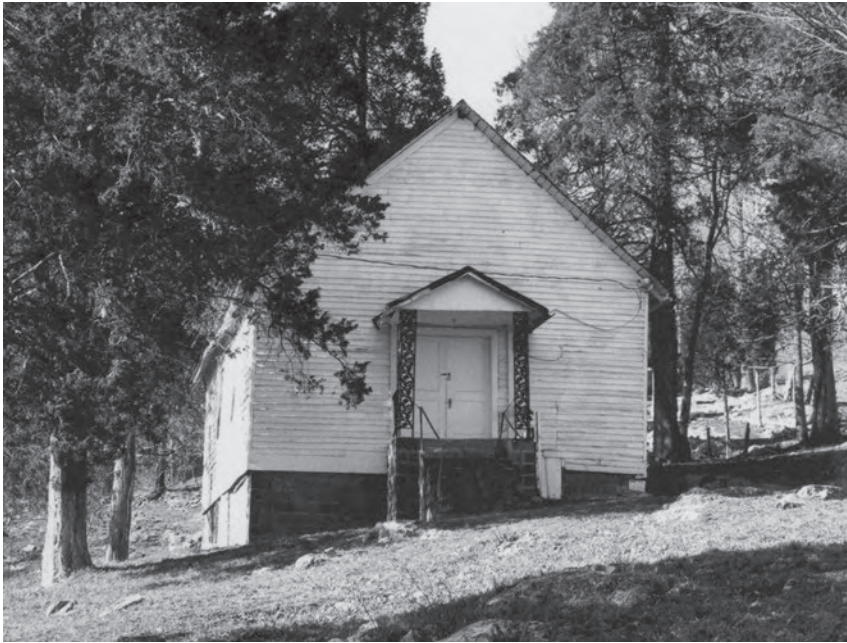
Figure 96. Bundy's Chapel A.M.E. Zion Church (083-5204), Route 628, New Castlewood (2008).
