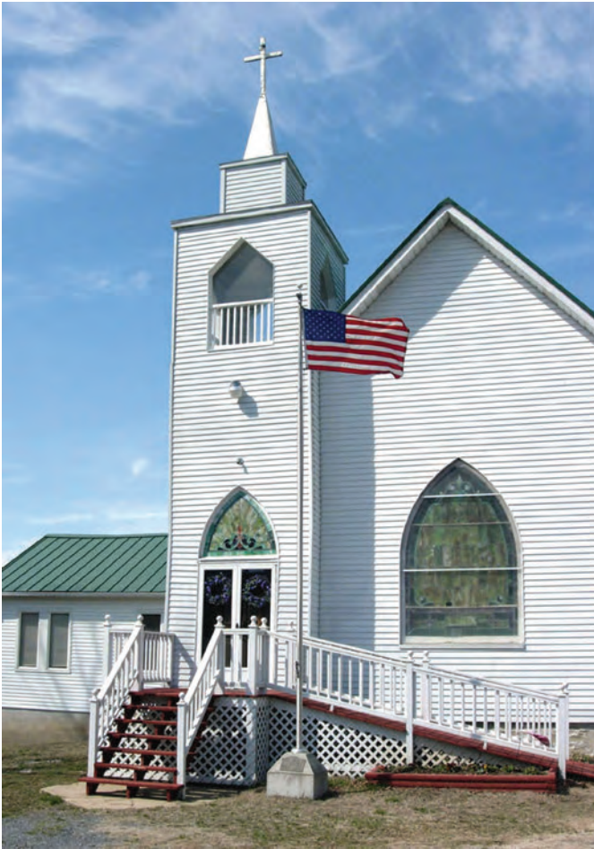
Figure 157. Sulphur Springs United Methodist Church (083-5213), Route 58, Hansonville (2008).
