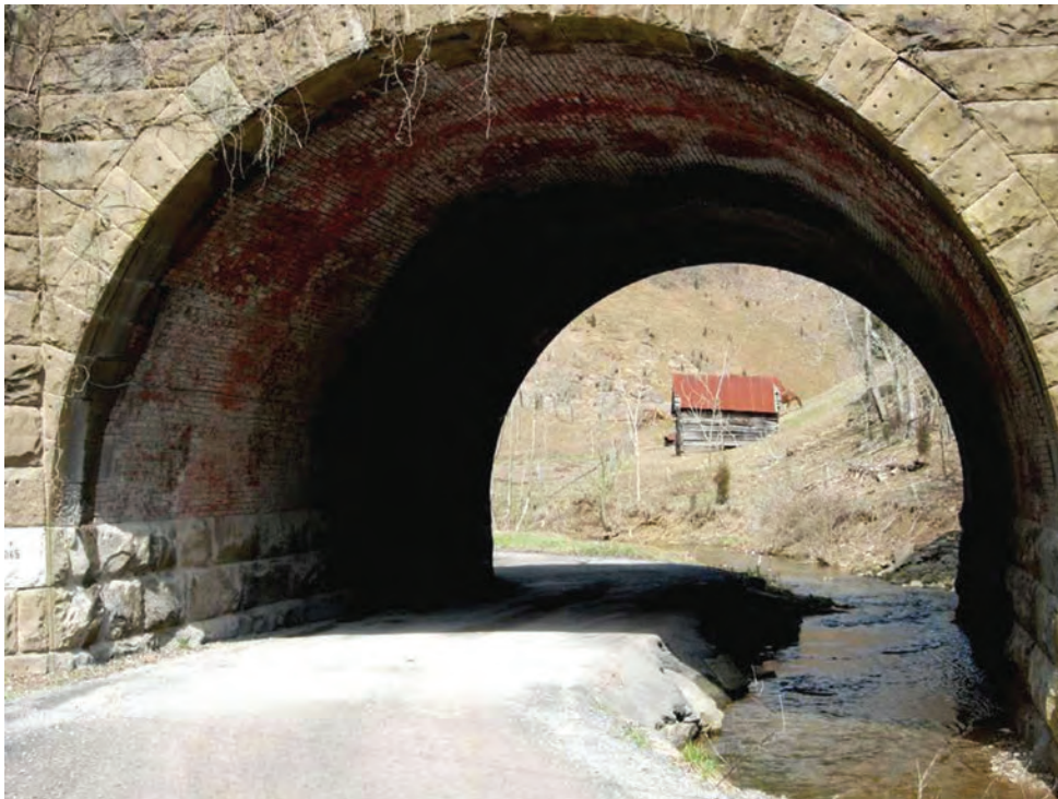
Figure 196. Brick vault, Thompson Creek Tunnel #6 (083-5014), Thompson Creek Road, near Honaker (2008).
