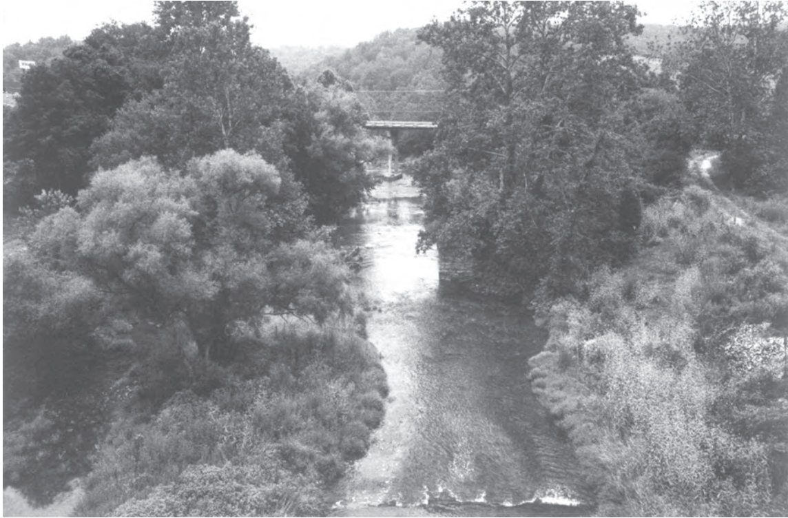
Figure 189. Bridge piers (083-5260), Route 658, Lebanon (2008).
