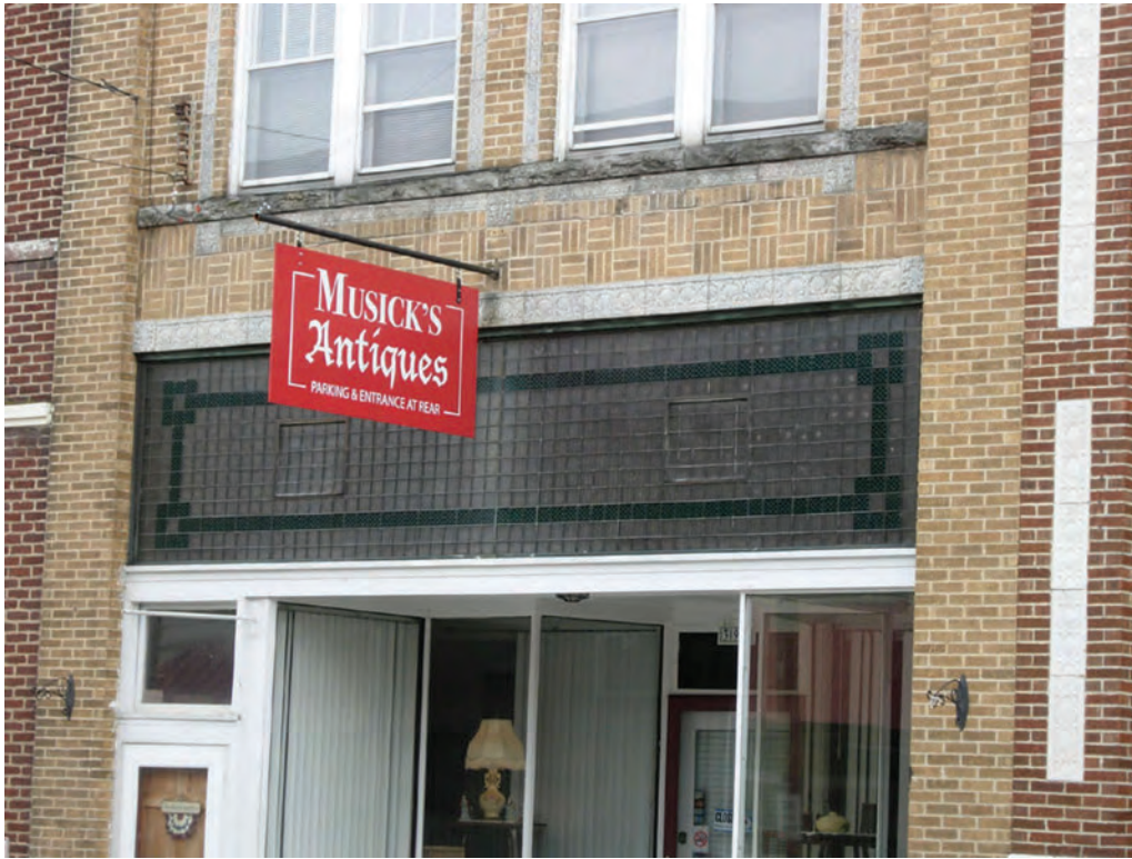
Figure 39. Display windows and prism lights, Musicks's Antiques (239-5012), Main Street/Railroad Avenue, Honaker (2008).
