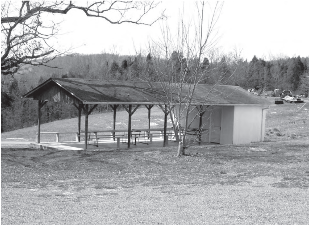
Figure 161. Picnic Shelter, Sulphur Springs United Methodist Church (083-5213), Route 58, Hansonville (2008).
