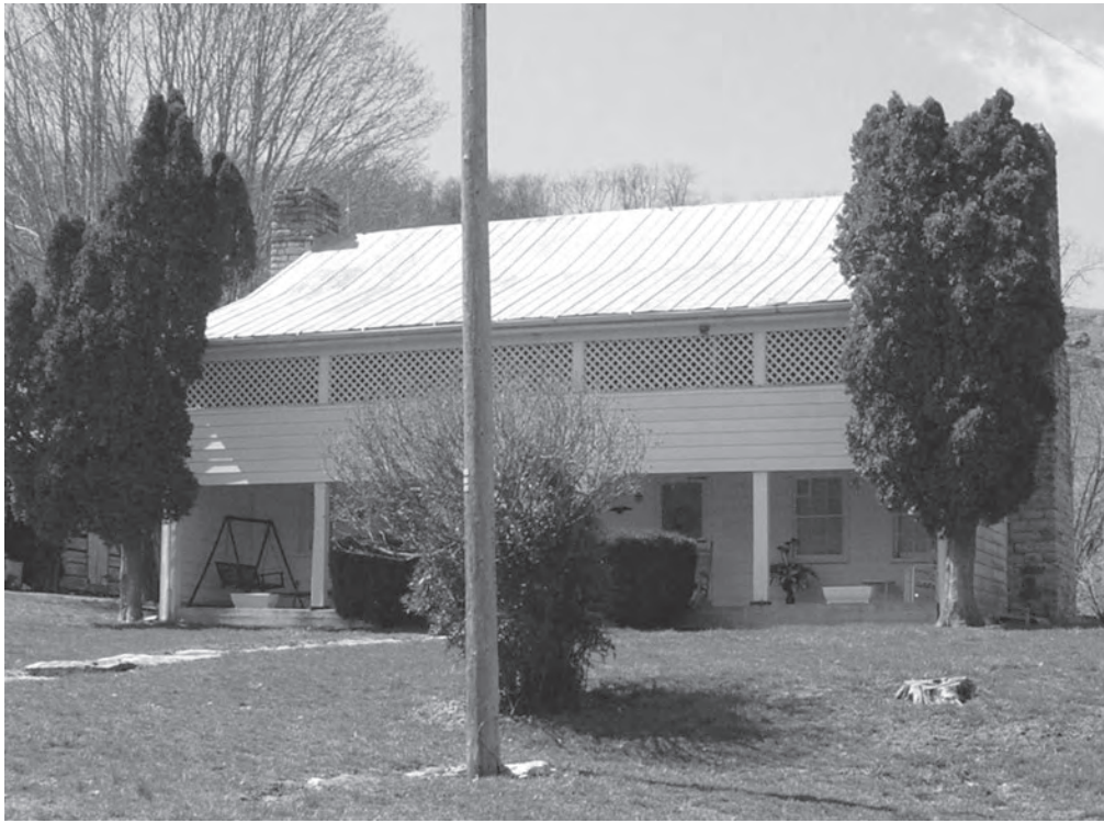
Figure 200. Will Browning House, former overnight tavern (083-5214), Route 80 (2008).
