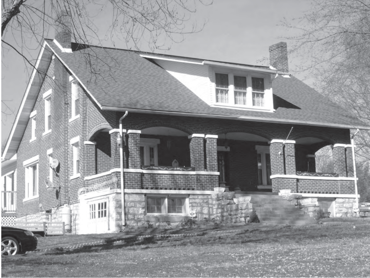
Figure 83. Easterly-Owens House (252-5018), Old Fincastle Road, Lebanon (2008).
