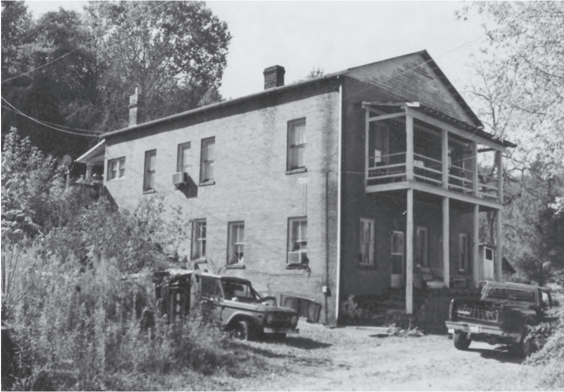
Figure 109. Post office (083-5106, Old Castlewood (2008).
