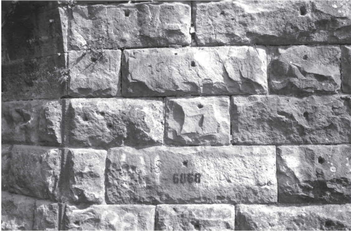
Figure 193. Tool marks, Thompson Creek Tunnel #3 (083-5015), Thompson Creek Road, near Honaker (2008).
