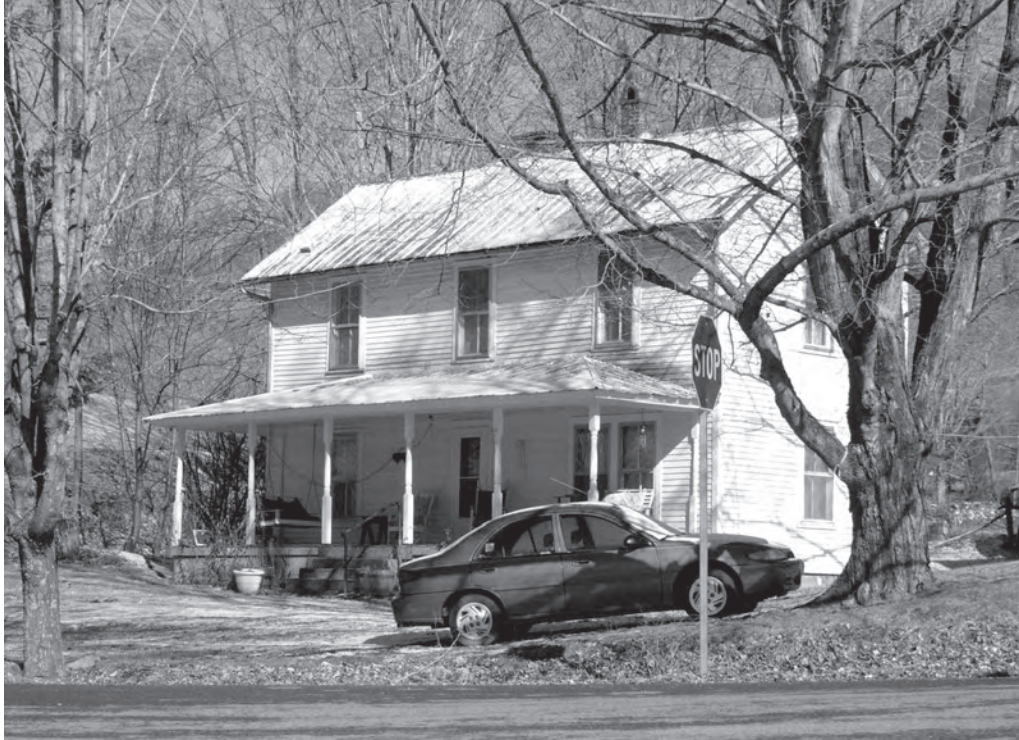
Figure 58. I-house (083-5177), Spring City Road, Lebanon (2008).
