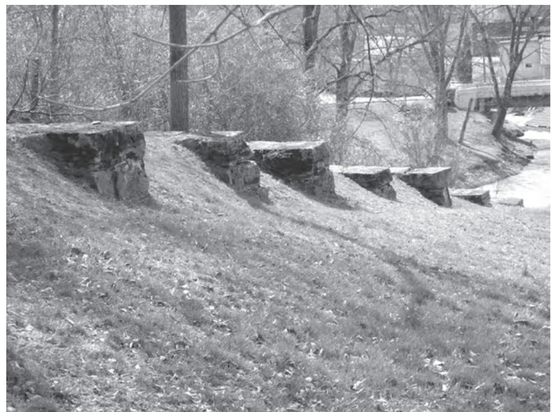
Figure 201. Railroad piers (239-5022), Fairmont Street, Honaker (2008).
