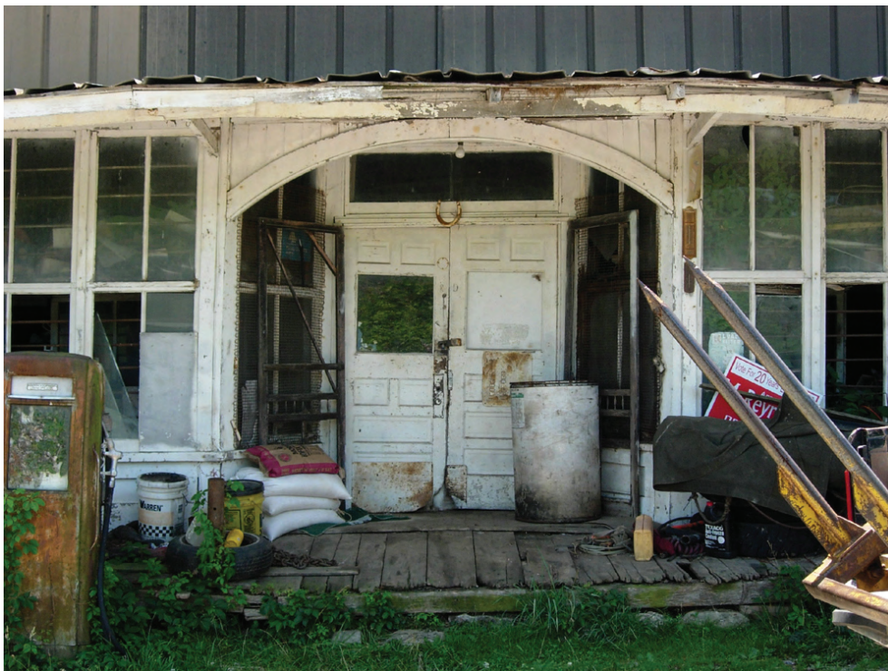
Figure 34. Country Store (083-5261), Route 71, Grassy Creek (2008).
