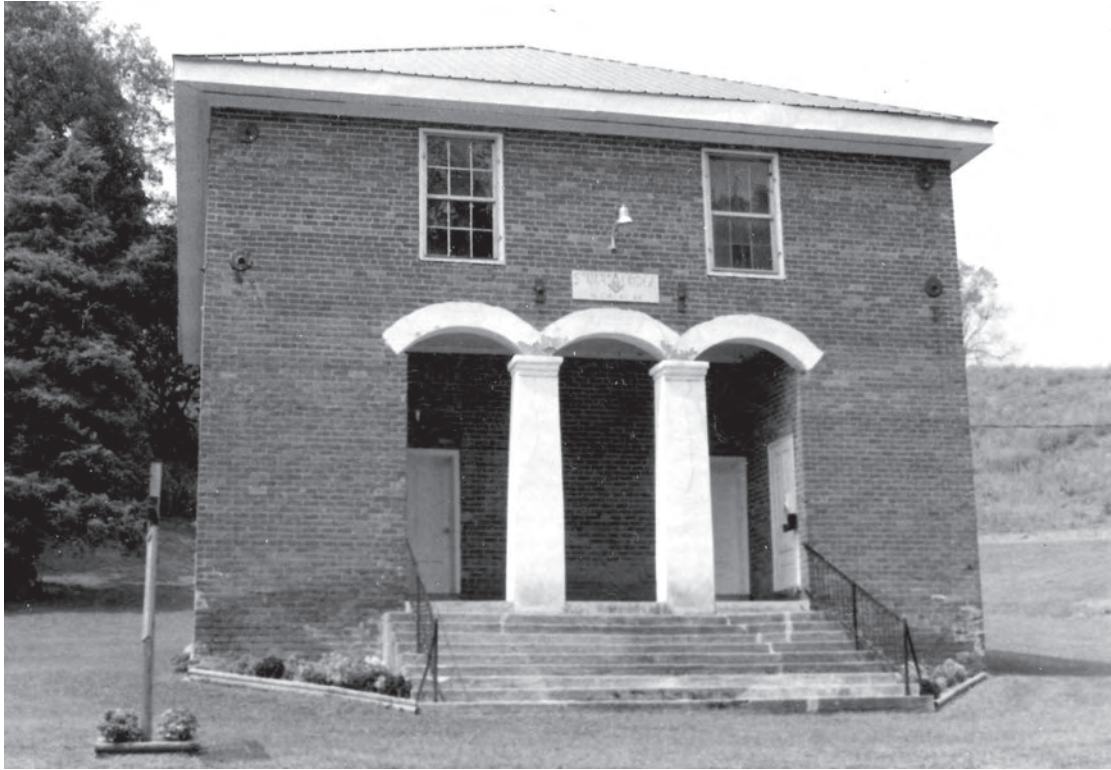
Figure 153. Stuart Chapel (083-5021), Route 613, Collingwood (2001).
