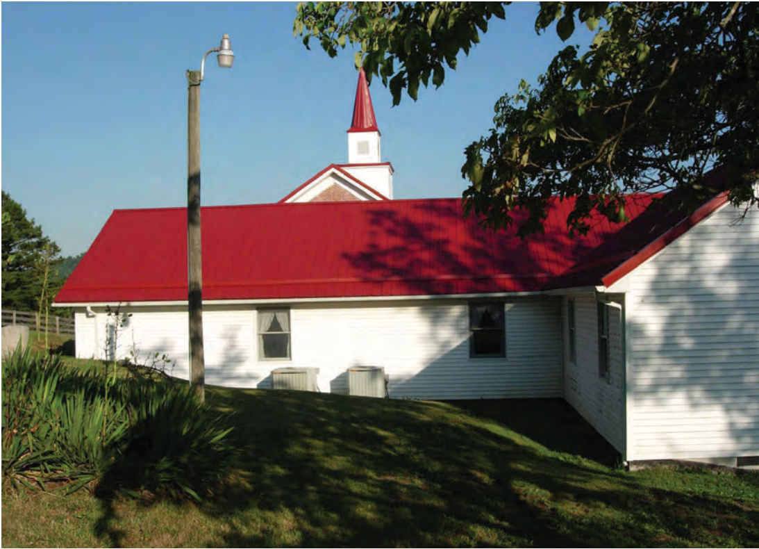
Figure 160. Fellowship hall, Old Brick Baptist Church, Old Brick Baptist Church (083-5100), Route 682, Banners Corners (2008).
