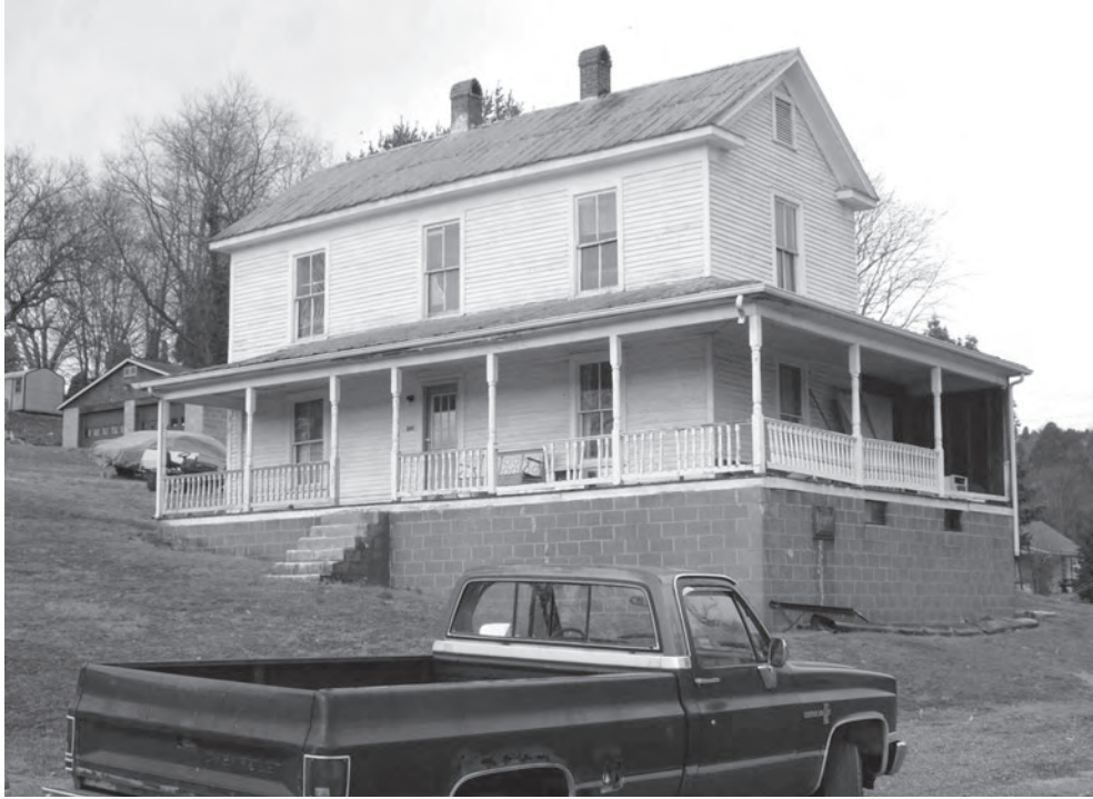
Figure 50. Waggoner House (252-0004), Old Fincastle Road, Lebanon (2008).
