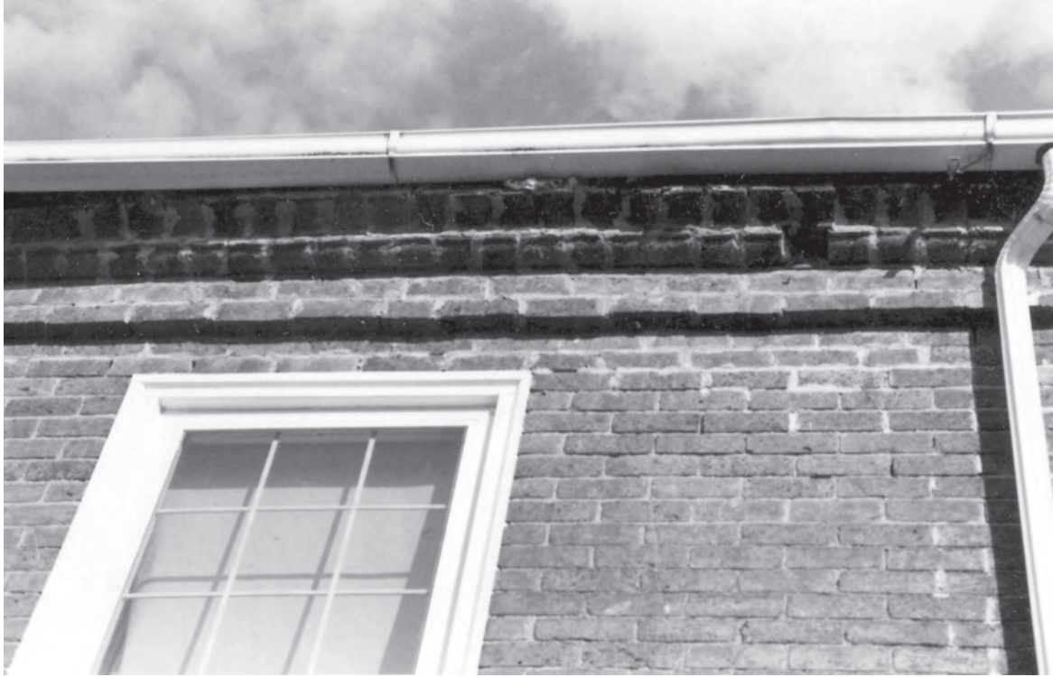
Figure 62. Molded, corbelled cornice, Shomaker Farm (083-5024), Route 676, Hansonville (2001).
