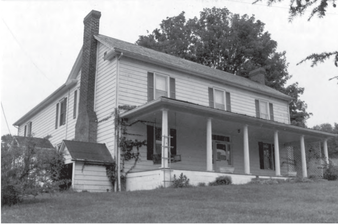
Figure 52. Aston-Fletcher House (083-5046), Route 71, Dickensonville (2001).
