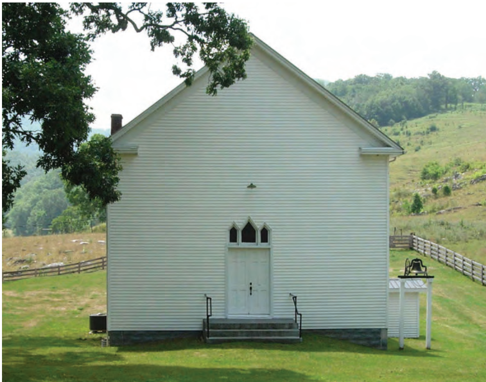
Figure 149. Cedar Grove Baptist Church (083-5242), Clinch Mountain Road, Bolton (2008).
