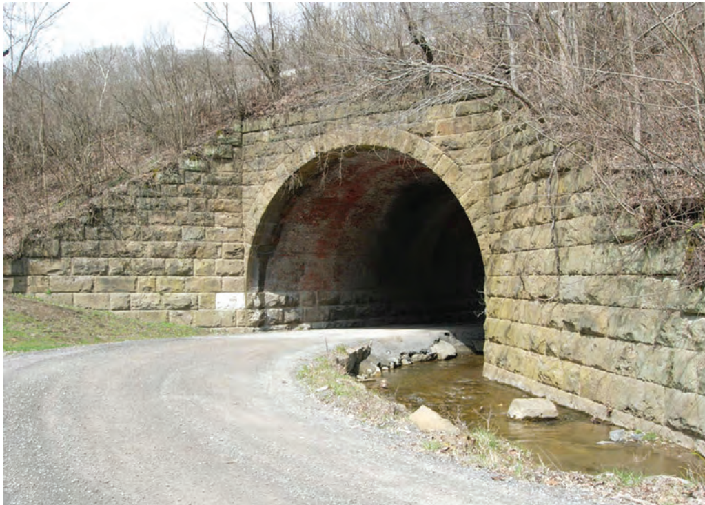
Figure 192. Thompson Creek Tunnel #6 (083-5014), Thompson Creek Road, near Honaker (2008).
