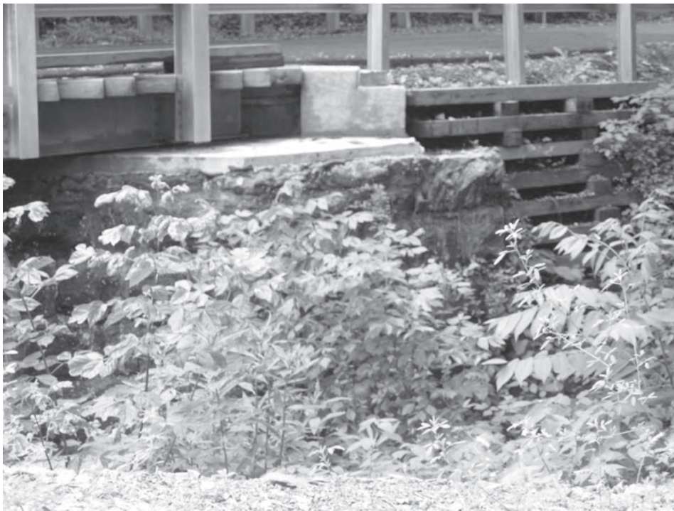
Figure 190. Bridge piers (083-5232), Route 614, Carterton (2008).
