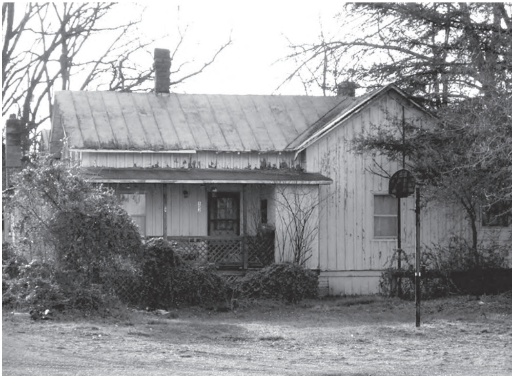
Figure 204. Station agent house (239-5018), Honaker (2008).
