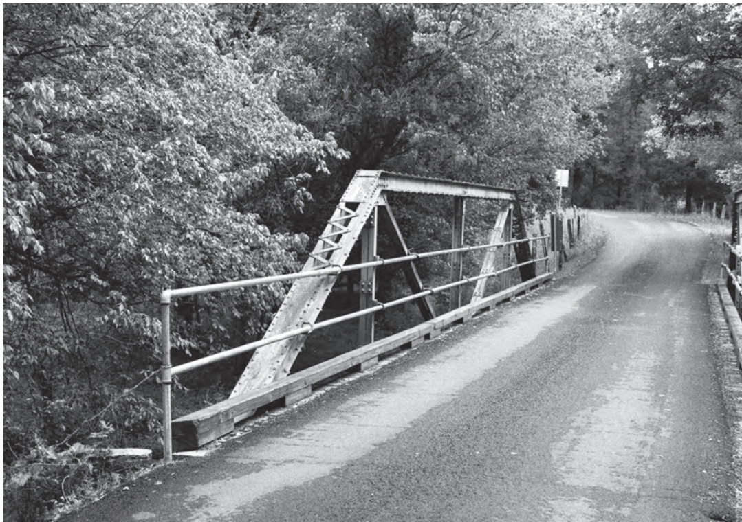
Figure 188. Iron truss bridge (083-5285), Route 606, Moll Creek (2008).
