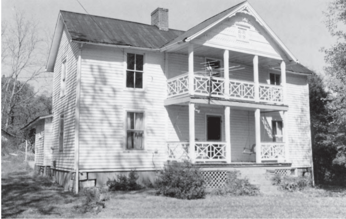
Figure 73. Dorton House (083-5041), Route 71, Dickensonville (2001).
