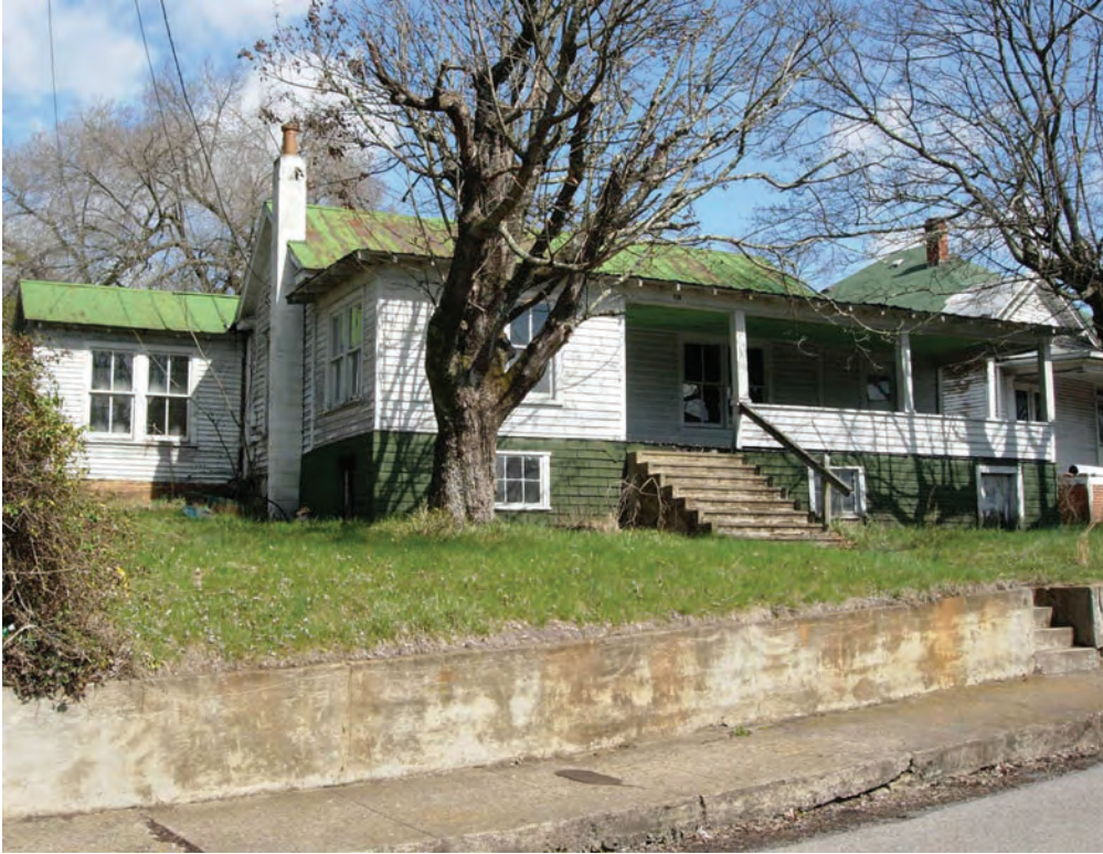
Figure 20. Modest dwelling (239-5027), Tunnel Hill Road, Honaker (2008).
