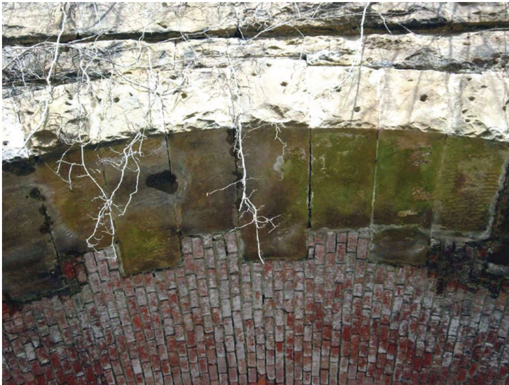
Figure 194. Keystone and voussoirs, Thompson Creek Tunnel #6 (083-5014), Thompson Creek Road, near Honaker (2008).
