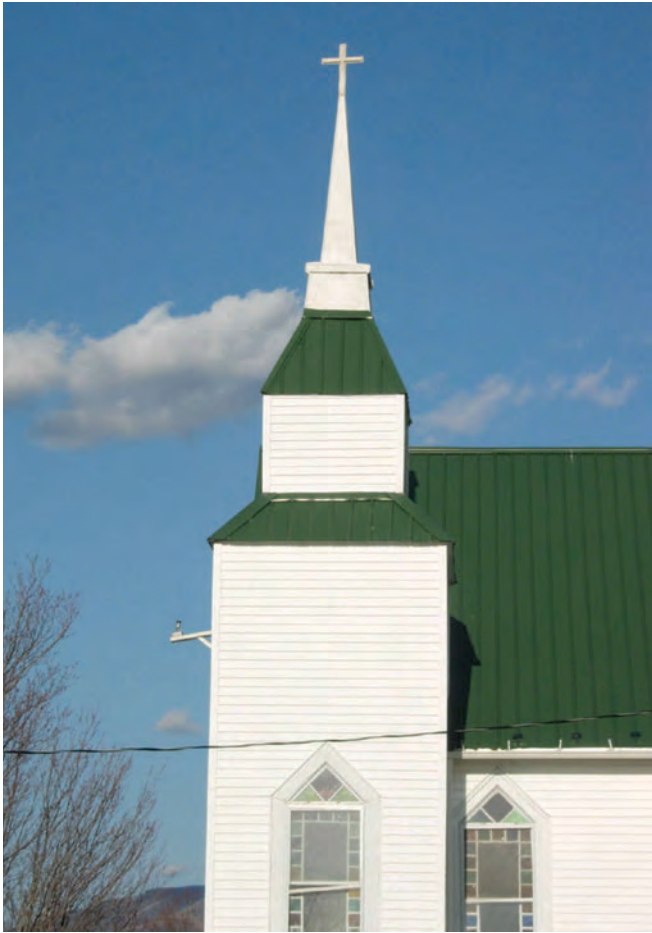
Figure 144. Tower, Bascom Church (083-5209), Green Valley Road (2008).
