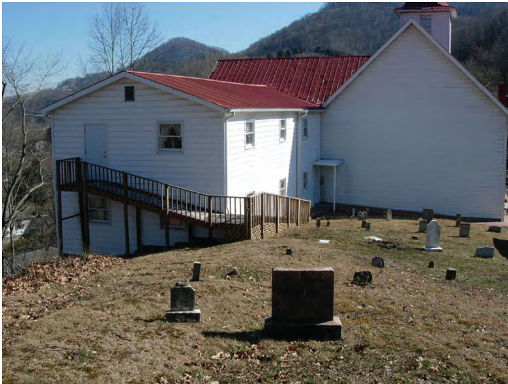
Figure 103. Churchyard, Cleveland Baptist Church (193-5006), Hall Street and Tank Hollow Road, Cleveland (2008).
