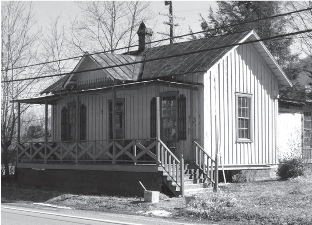
Figure 203. Station agent house (193-5008), Cleveland (2008).
