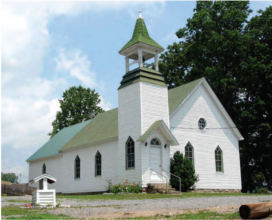
Figure 151. Church Hill United Methodist Church (083-5251), Route 657 (2008).
