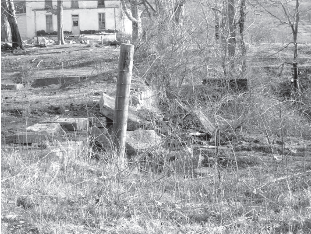
Figure 116. Foundation remains, Elk Garden Mill (083-0002), Elk Garden (2008).
