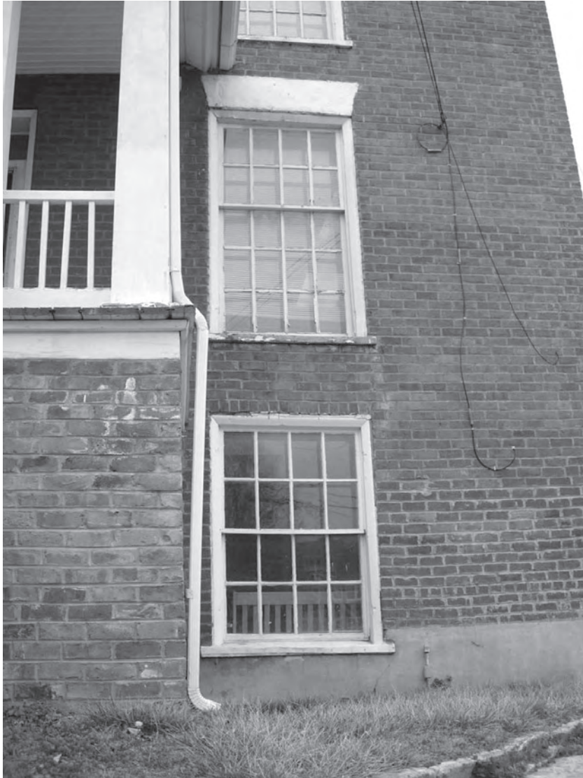
Figure 64. Windows, G. Garrett/ David B. Hanson House (252-0002), Main Street, Lebanon (2008).
