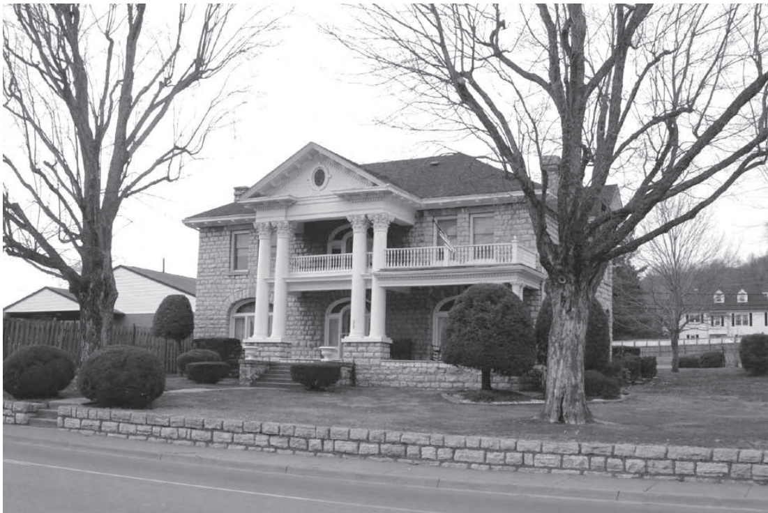
Figure 16. Prominent Main Street dwelling (252-5025), Lebanon (2008).
