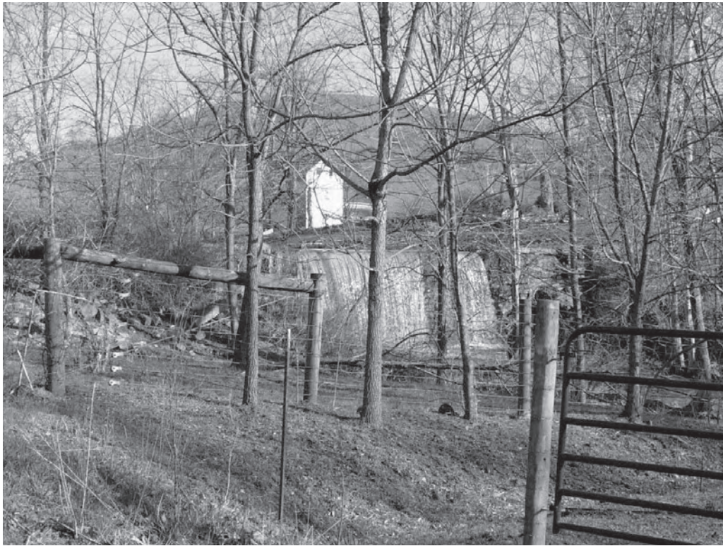
Figure 117. Dam, Elk Garden Mill (083-0002), Elk Garden (2008).
