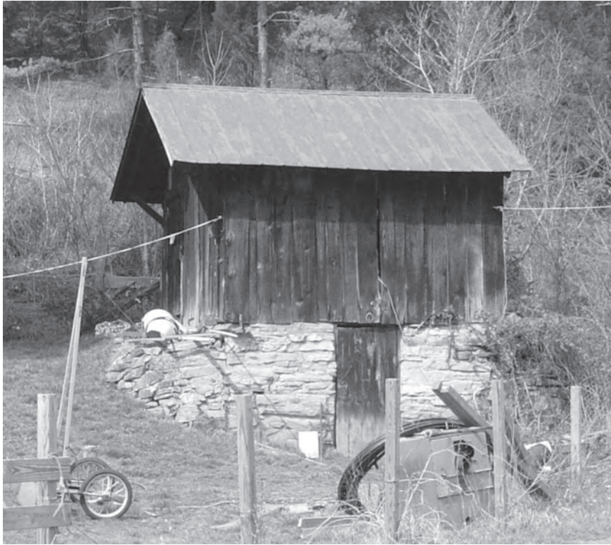
Figure 175. Stone outbuilding (083-5187), Haunt's Crossing, Finney/Coulwood (2008).
