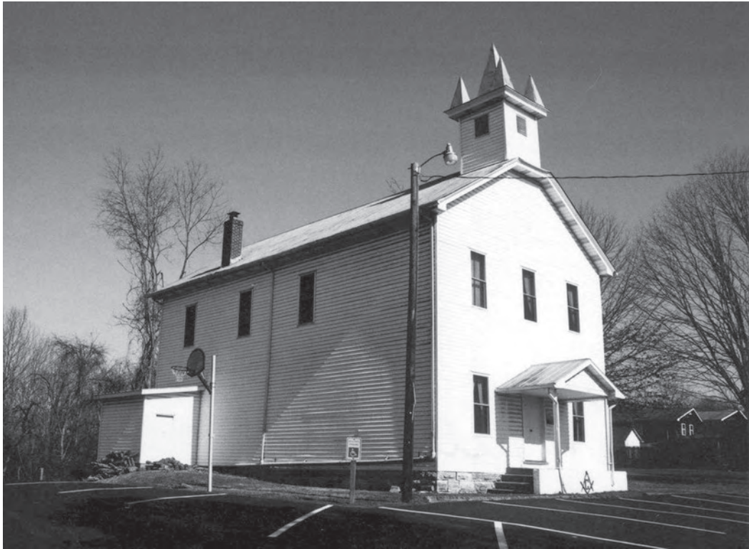
Figure 162. Castlewood Masonic Lodge (083-5111), Church Street and Route 615, New Castlewood (2008).
