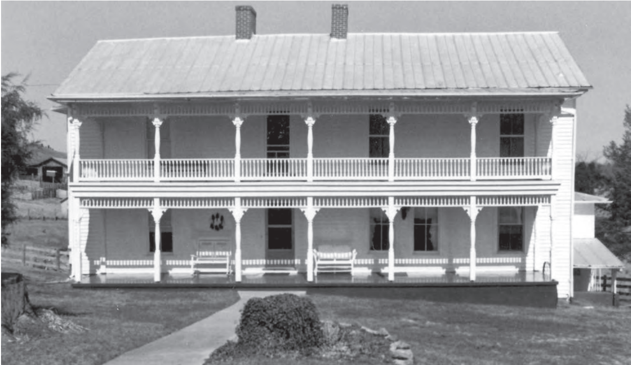
Figure 70. Gose-Dickenson Farm (083-5088), Route 640, Old Castlewood (2001).
