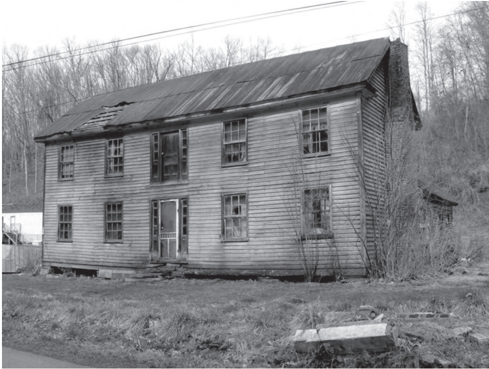
Figure 94. I-house (083-5182), Hubbard Town Road, near Honaker (2008).
