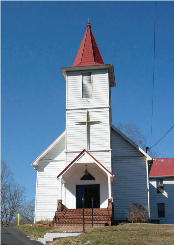
Figure 150. Cleveland Baptist Church (193-5006), Hall Street and Tank Hollow Road, Cleveland (2008).
