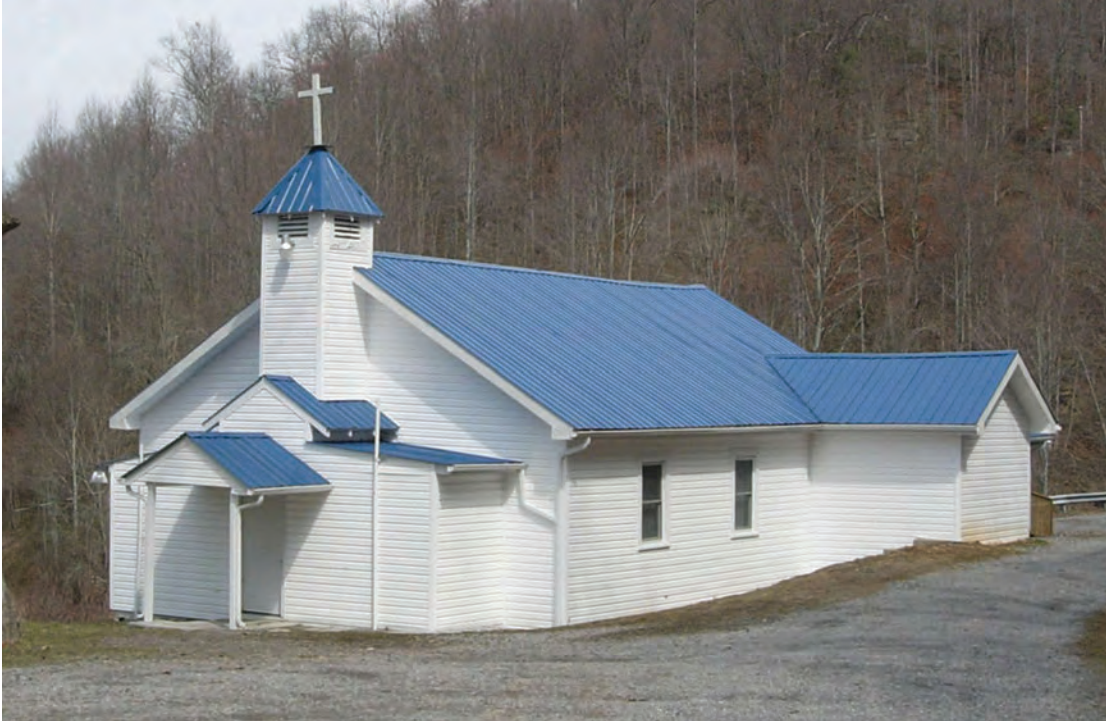
Figure 159. Drill Chapel Freewill Baptist Church (083-5166), Route 24, Drill (2008).
