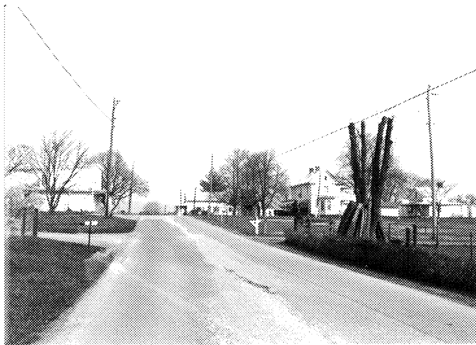
Fig. 34. Oranda (85-505). View looking northwestward along Rt. 629. (Photo: Maral S. Kalbian, 1993)
