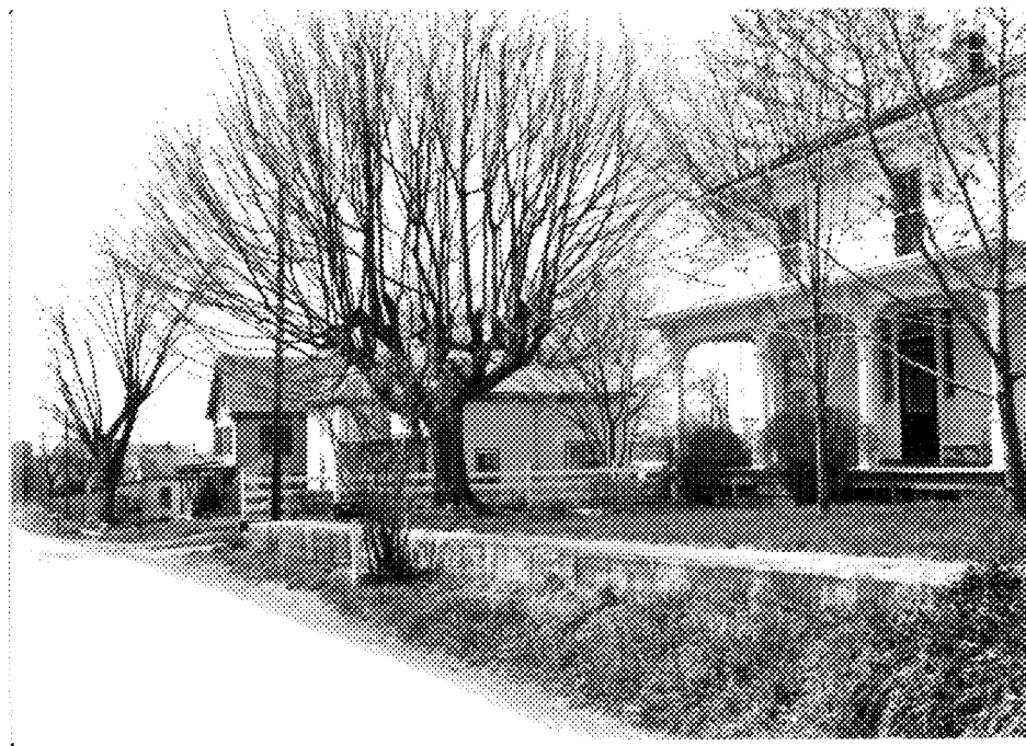
Fig. 36. Saumsville (85-503). View of houses and outbuildings on north side of Rt. 652. (Photo: Maral S. Kalbian, 1993)
