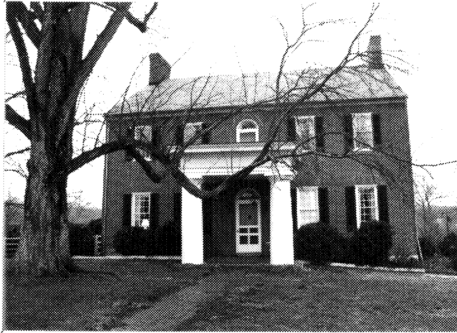
Fig. 13. Spengler Hall (85-9). House, south (front) elevation. (Photo: Maral S. Kalbian, 1993)
