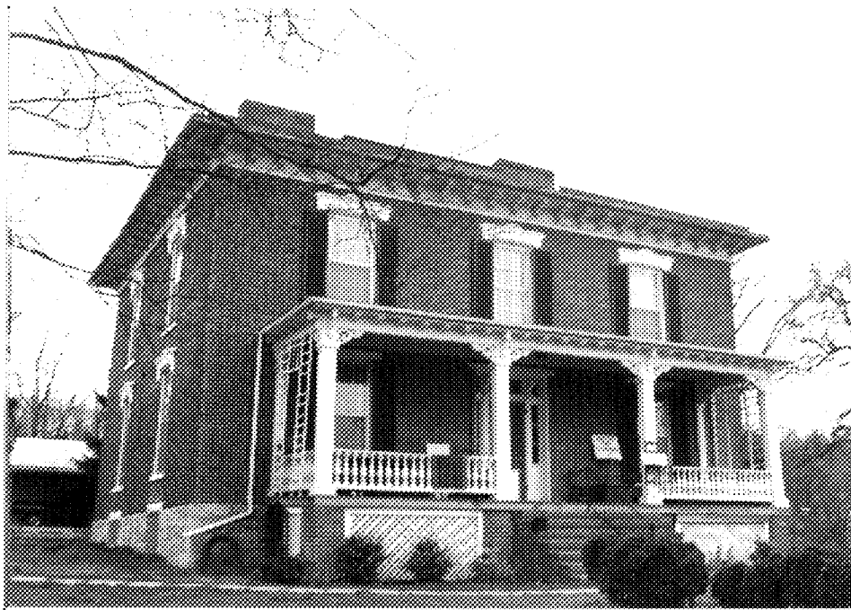
Fig. 21. Vesper Hall (85-73). House, front (east) elevation. (Photo: Maral S. Kalbian, 1993)
