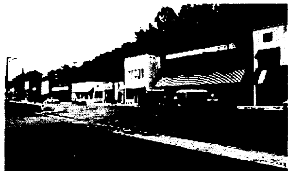
Potential Saltville Historic District
