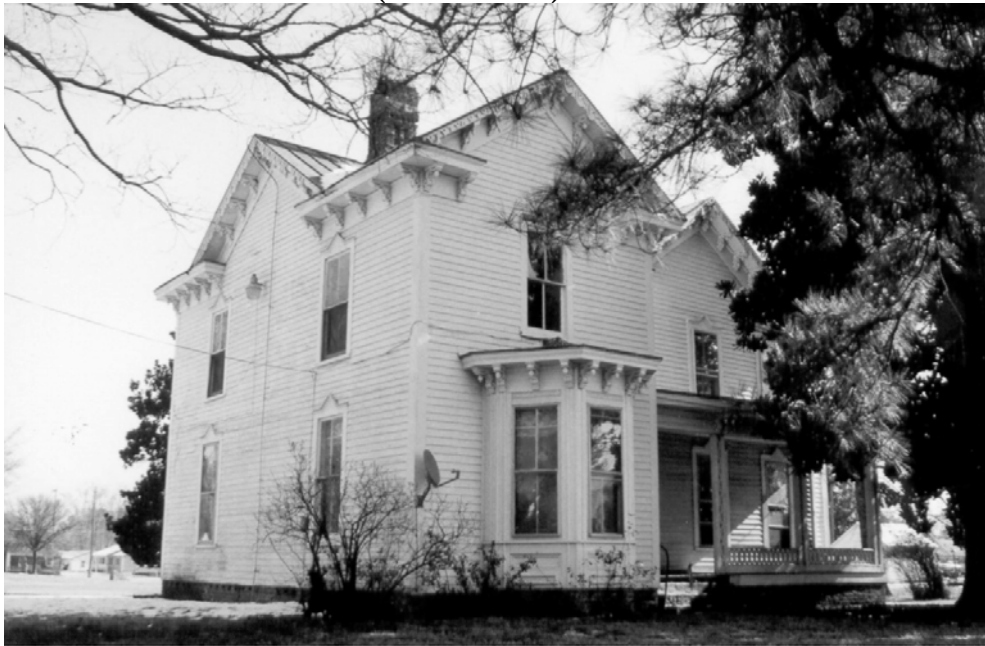
Figure 3.12: 22125 Main St in Courtland (201-5001-0008)
