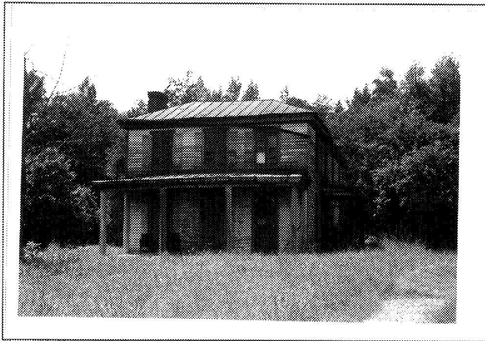
Figure 84: House on Jefferson Davis Highway (88-10)
