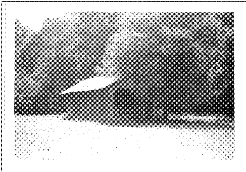
Figure 47: Shed at 6113 Hickory Ridge Road (88-295)
