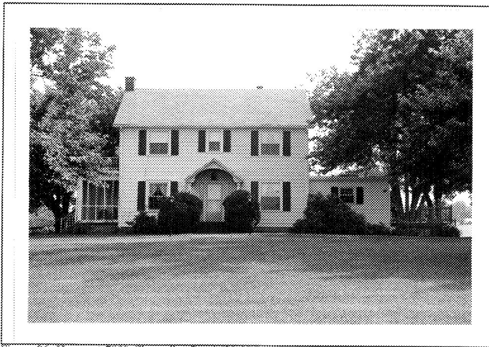
Figure 86: House at 7800 Chancellor Road (88-276)
