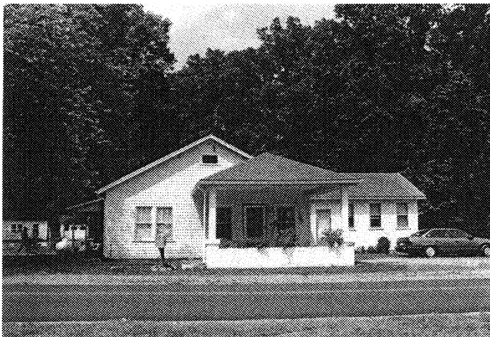
Figure 17: Service Station and House at 8701 Brock Road (088-0028)
