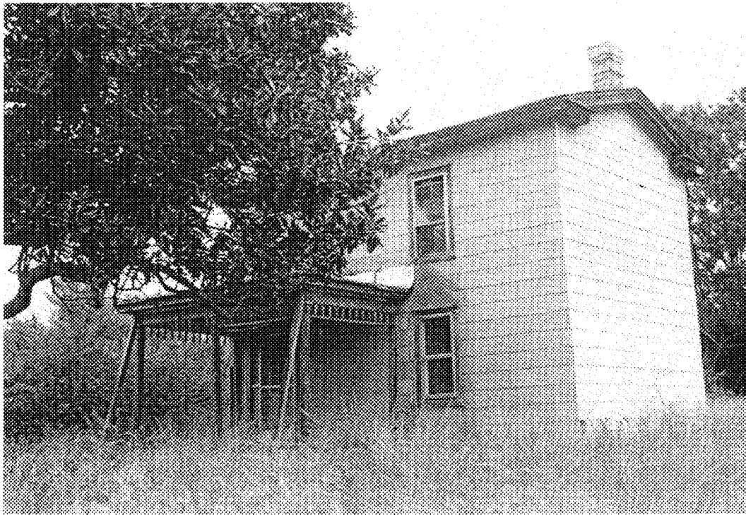
Figure 39: House at 7117 Grand Brooks Road (088-5051)
