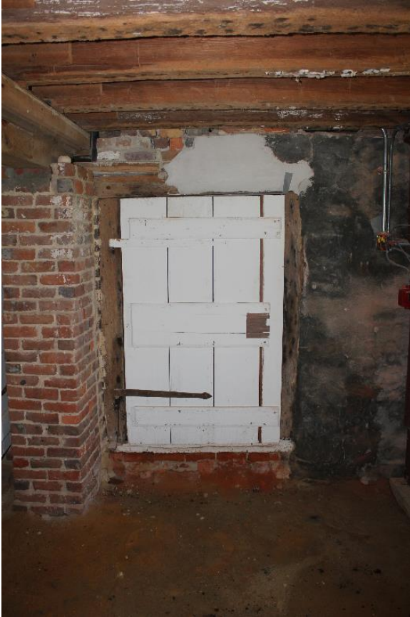
Figure 5.92, Bacon's Castle, ca. 1665 dwelling, Basement, West room, Room 005, door detail.
