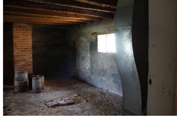
Figure 5.88, Bacon's Castle, ca. 1665 dwelling, Basement, West room, Room 005, general view northwest.
