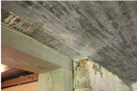
Figure 5.121, Bacon's Castle, Basement, Room 011, cased opening detail.
