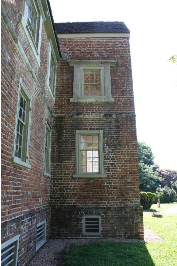
Figure 5.50, Bacon's Castle, West elevation, south tower.
