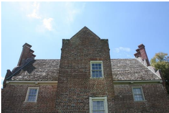
Figure 5.20, Bacon's Castle, North elevation, detail of parapets.
