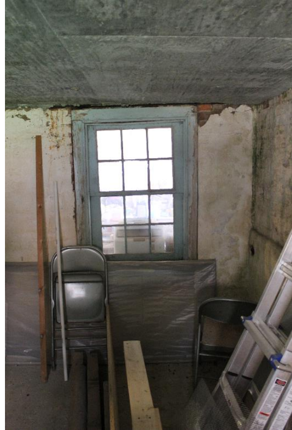
Figure 5.119, Bacon's Castle, Basement, Room 011, window on east wall.
