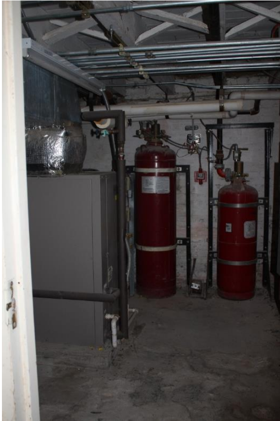
Figure 5.122, Bacon's Castle, Hyphen, Room 012, general view north.
