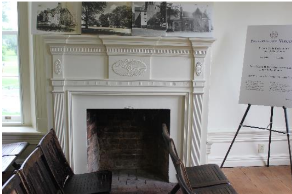
Figure 5.171, Bacon's Castle, ca. 1854 addition, First Floor, Room 108, detail of fireplace.
