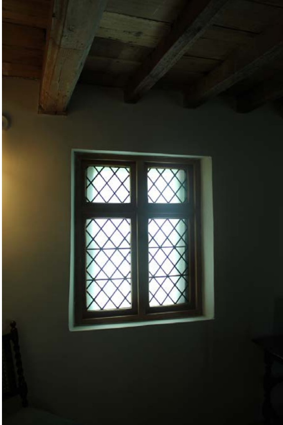
Figure 5.197, Bacon's Castle, ca. 1665 building, Second Floor, West Chamber, Room 203, window detail.
