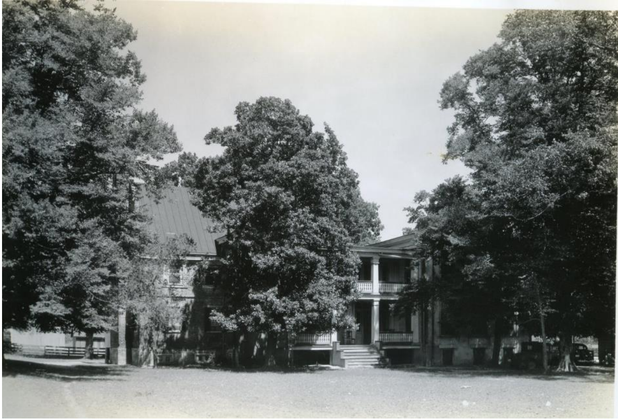
Figure 50: Bacon's Castle, photograph of south (front) elevation, National Park Service, 1937.
