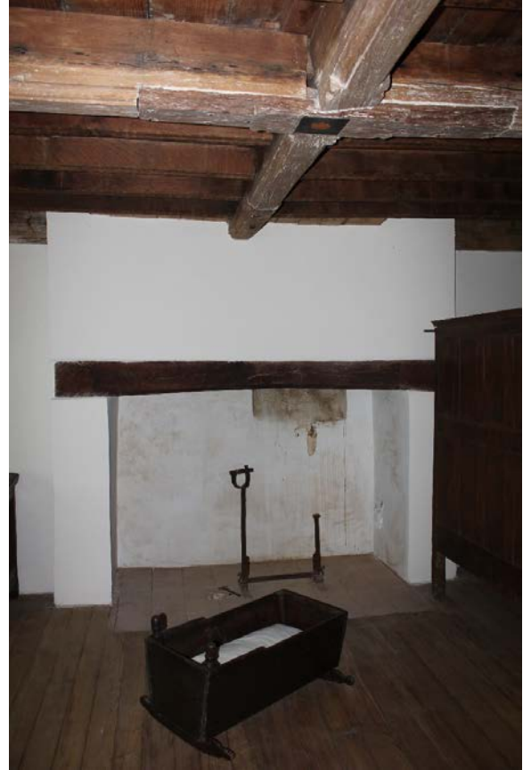
Figure 5.198, Bacon's Castle, ca. 1665 building, Second Floor, West Chamber, Room 203, mantel detail.
