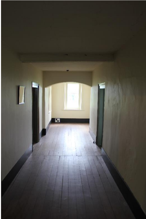
Figure 5.132, Bacon's Castle, ca. 1665 building, Corridor, Room 102, general view south.
