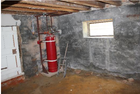
Figure 5.86, Bacon's Castle, ca. 1665 dwelling, Basement, West room, Room 005, general view southeast.
