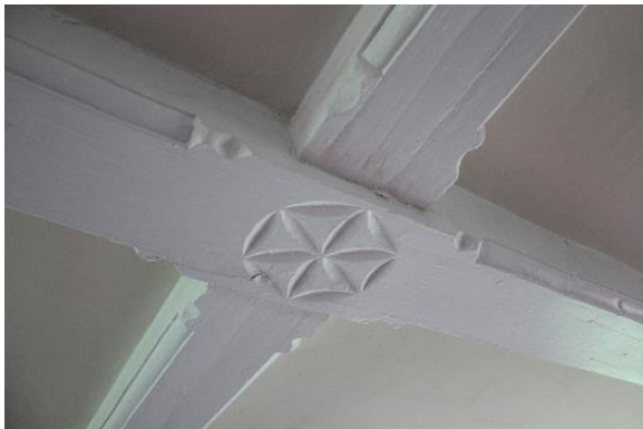
Figure 5.140, Bacon's Castle, ca. 1665 building, West Room, Room 103, detail of beam intersection.
