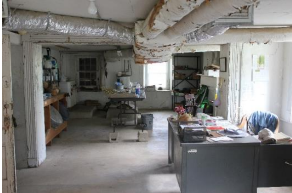
Figure 5.106, Bacon's Castle, ca. 1854 addition, Basement, Room 008,009, general view north.
