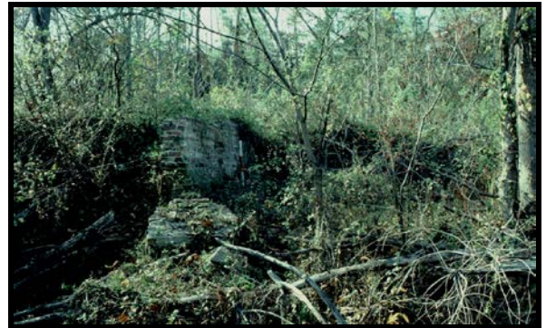
Figure 3.25: Brick foundations along Castle Mill Run.
