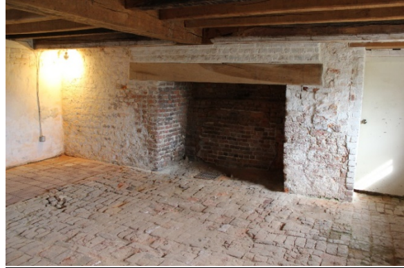
Figure 2.91: Bacon's Castle, Cellar, East Room, view to east. Photograph Commonwealth Architects, 2015.
