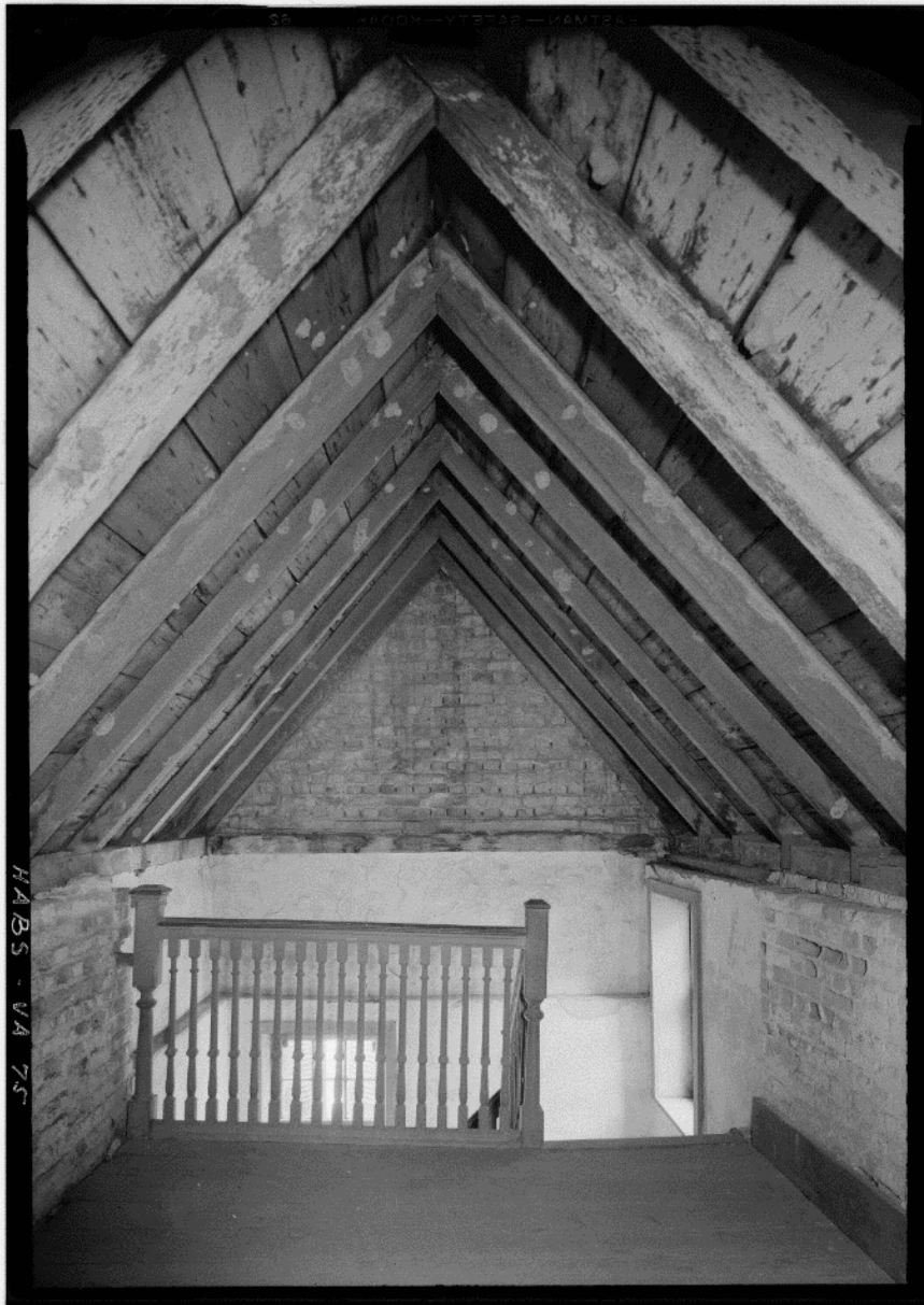
Figure 41: Bacon's Castle, photograph of garret floor, Room 301, ca. 1665 section, view north, Historic American Buildings Survey, ca. 1937.
