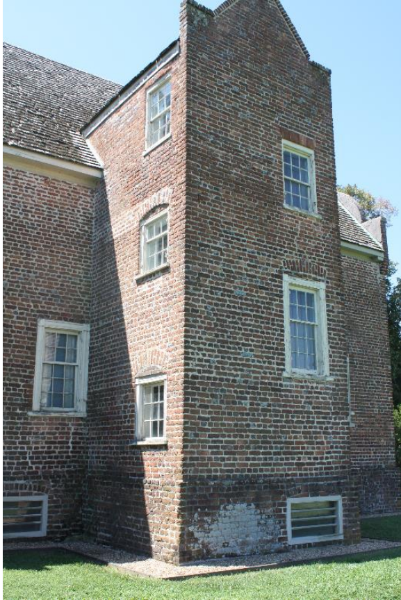
Figure 5.35, Bacon's Castle, East elevation, ca. 1665 north tower.
