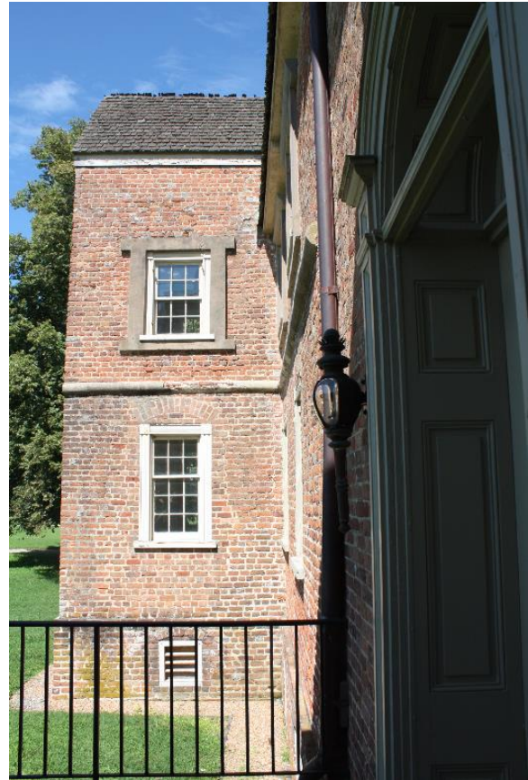
Figure 5.34, Bacon's Castle, East elevation, ca. 1665 south tower.
