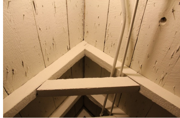
Figure 5.242, Bacon's Castle, ca. 1665 portion, Garret Floor, Room 303, detail of ceiling.
