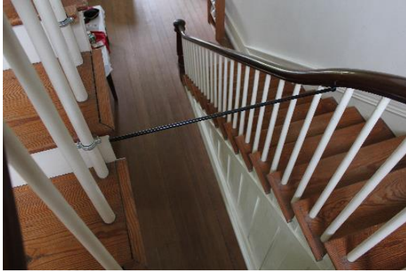
Figure 5.166, Bacon's Castle, ca. 1854 addition, First Floor, Room 107, detail of bracing.
