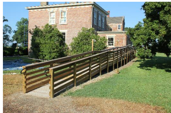
Figure 5.43, Bacon's Castle, East elevation, modern handicapped ramp.
