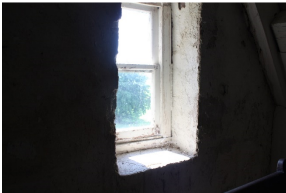
Figure 5.240, Bacon's Castle, ca. 1665 portion, Garret Floor, Room 302, detail of window.
