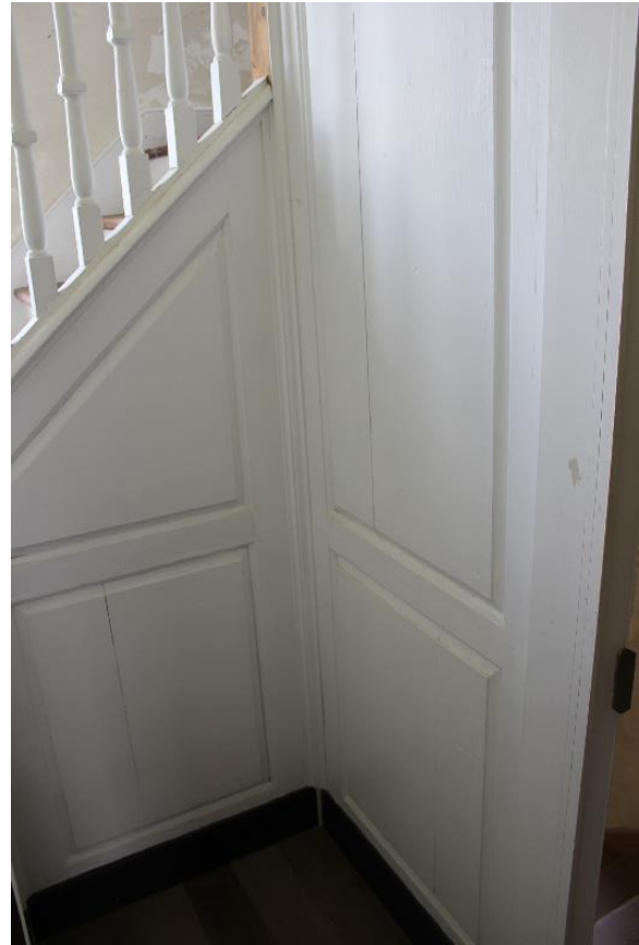
Figure 5.131, Bacon's Castle, ca. 1665 building, North Tower, Room 101, detail of stair paneling.
