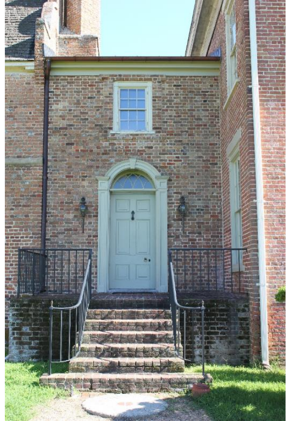
Figure 5.14, Bacon's Castle, South elevation, present porch.
