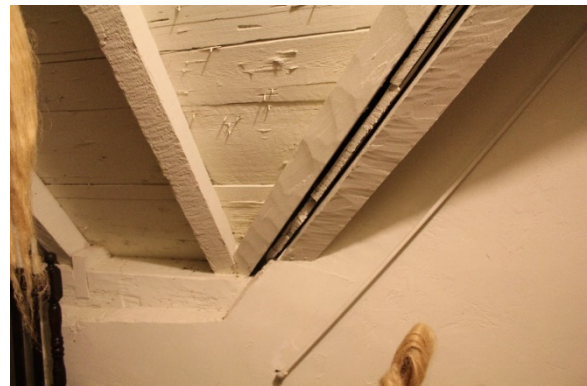
Figure 5.243, Bacon's Castle, ca. 1665 portion, Garret Floor, Room 303, detail structural joint.
