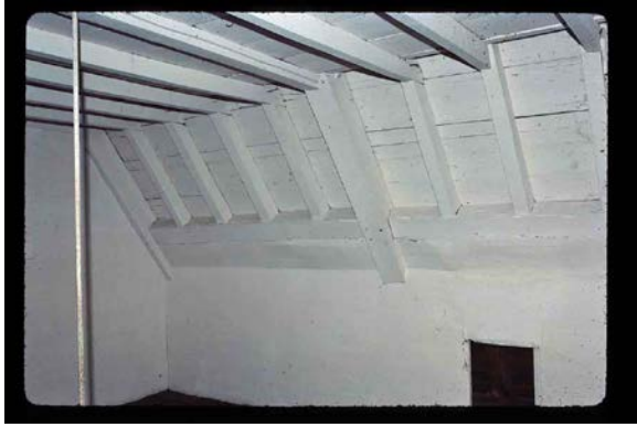
Figure 2.134: Bacon's Castle, garret, 1976. Virginia Department of Historic Resources.
