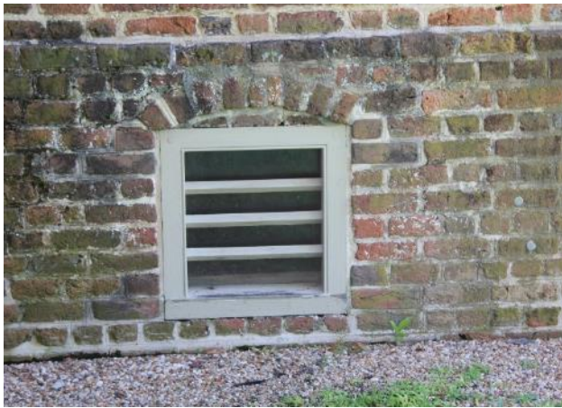
Figure 5.58, Bacon's Castle, West elevation, south tower, basement window.
