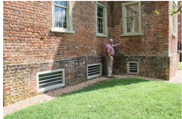
Figure 5.15, Bacon's Castle, South elevation, detail of foundation.
