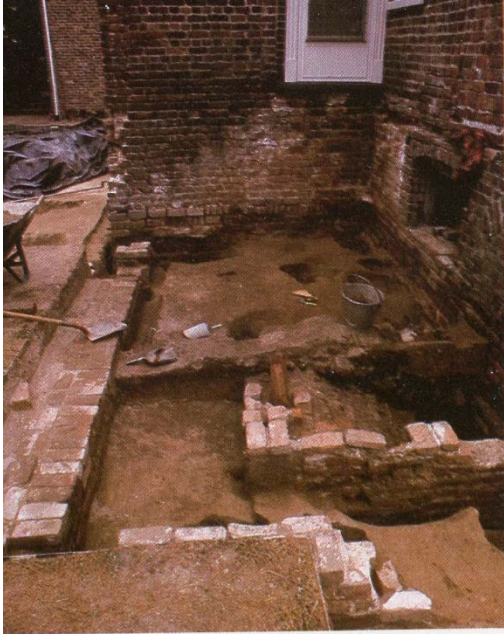
Figure 2.120: Bacon's Castle, archaeological excavations along north elevation, 1982. Preservation Virginia.
