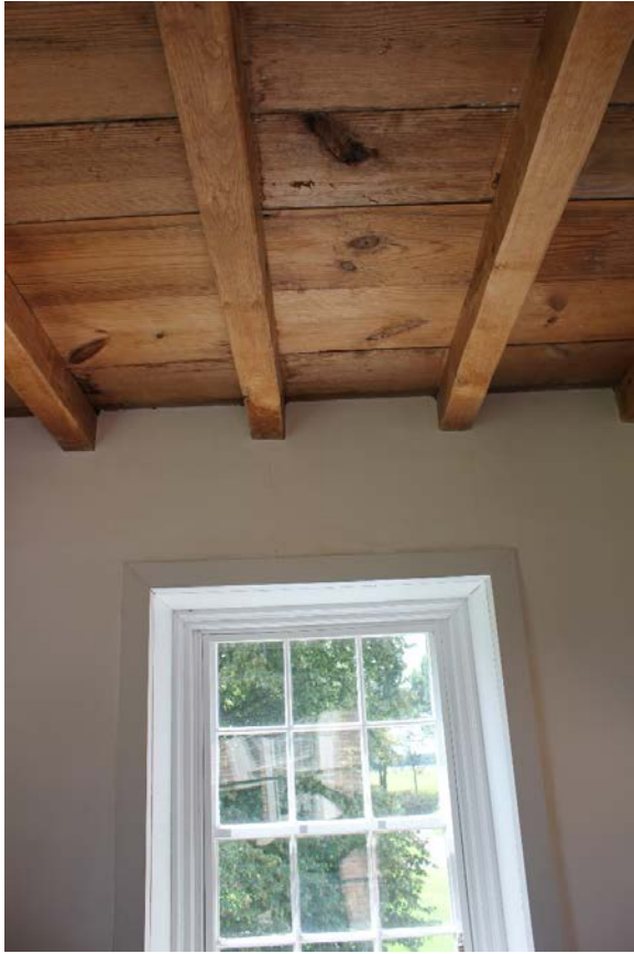
Figure 5.200, Bacon's Castle, ca. 1665 building, Second Floor, South Tower, Room 204, view west.
