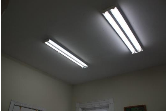
Figure 5.185, Bacon's Castle, ca. 1950s addition, First Floor, Room 113, ceiling detail.
