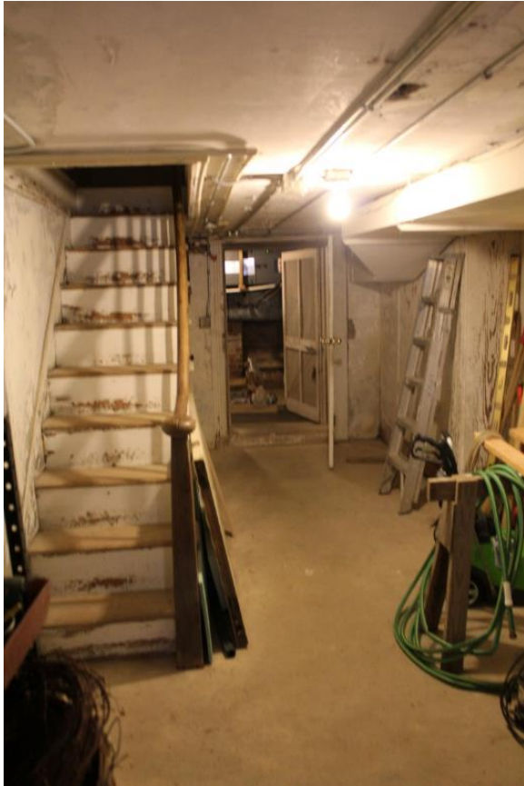
Figure 5.100, Bacon's Castle, ca. 1854 addition, Basement, Room 007, View north.
