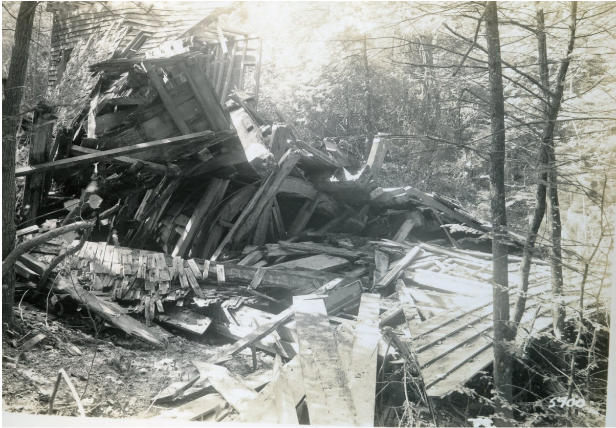
Figure 4: Photograph of Castle Mill Run ruins, National Park Service, 1937.
