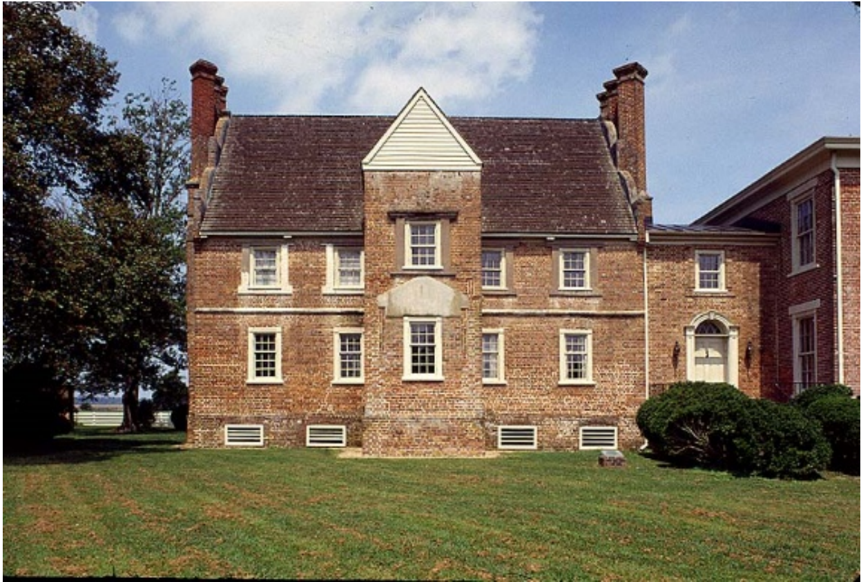
Figure 125: Bacon's Castle, photograph of front (south) elevation looking north, 2004. Courtesy Virginia Department of Historic Resources.
