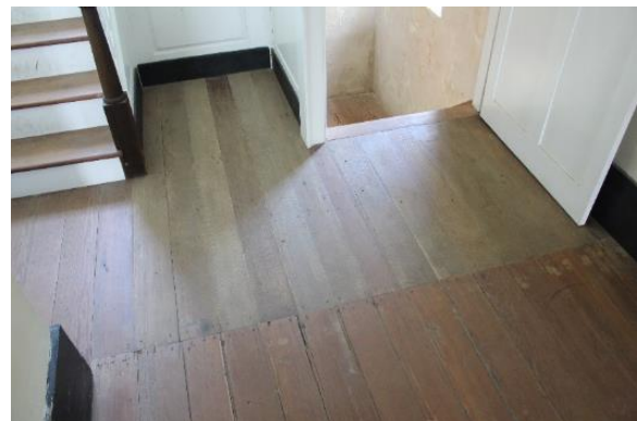
Figure 5.130, Bacon's Castle, ca. 1665 building, North Tower, Room 101, floor transition.
