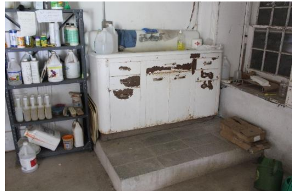
Figure 5.113, Bacon's Castle, ca. 1854 addition, Basement, Room 008,009, view northwest. Elevated platform, cabinet and sink detail. Note the rust on the sink.
