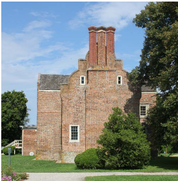
Figure 2.16: Bacon's Castle, West elevation. Photograph 26 July 2015.
