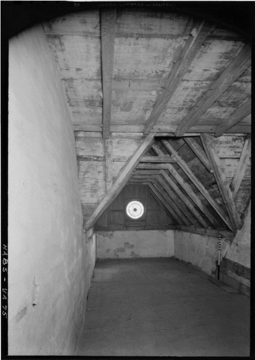
Figure 42: Historic American Buildings Survey, photograph of south garret, Historic American Buildings Survey, ca. 1937.
