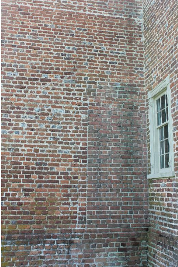
Figure 5.59, Bacon's Castle, West elevation, north tower, in-filled door opening and porch ghosting.
