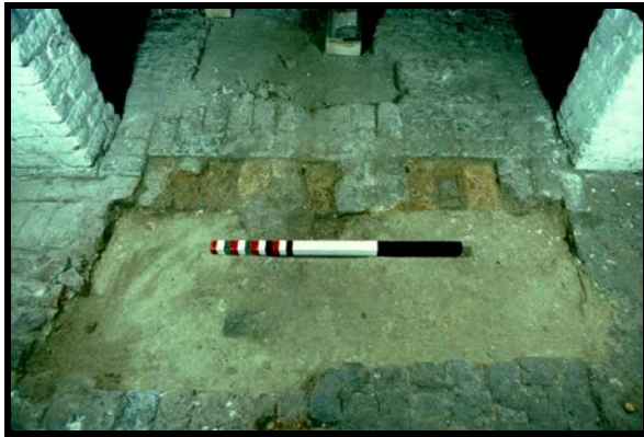
Figure 3.18: Footing of oversized brick at the south end of the west side of the cellar kitchen.
