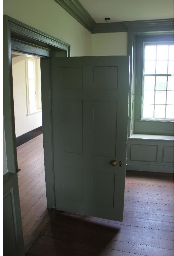
Figure 5.143, Bacon's Castle, ca. 1665 building, West Room, Room 103, door detail
