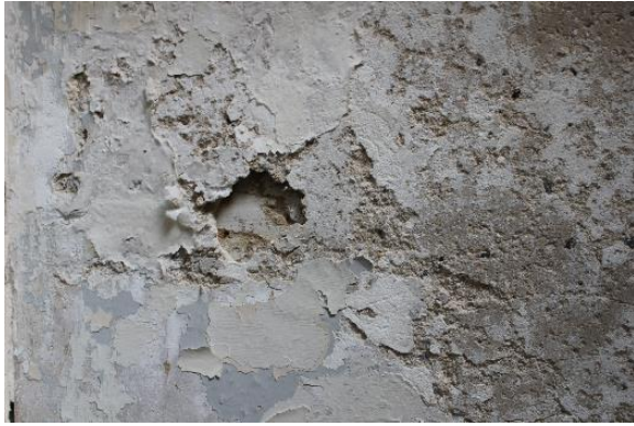
Figure 5.142, Bacon's Castle, ca. 1665 building, West Room, Room 103, detail of efflorescence.
