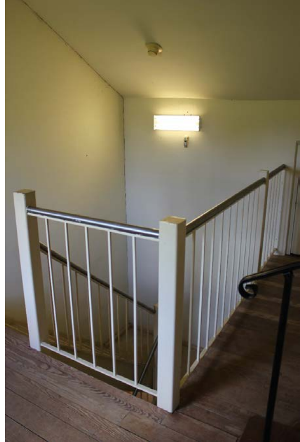
Figure 5.213, Bacon's Castle Hyphen, Second Floor, Room 206, detail of stair railings.
