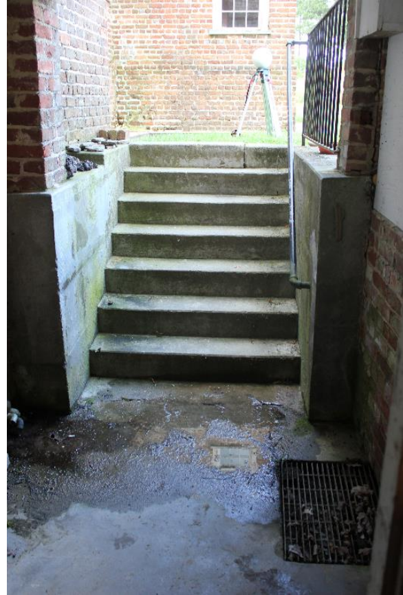
Figure 5.115, Bacon's Castle, ca. 1950s addition, Basement, Room 010, view west.
