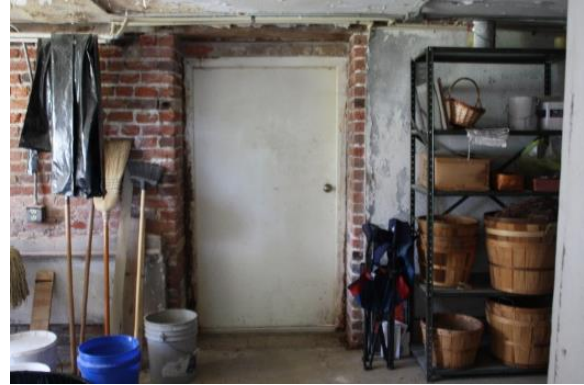
Figure 5.103, Bacon's Castle, ca. 1854 addition, Basement, Room 007, modern metal door.
