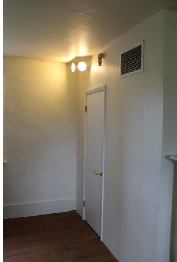
Figure 5.207, Bacon's Castle, ca. 1665 building, Second Floor, East Room, Room 205, view northeast. Note the modern closet, door, light, halon suppression system, and vent.
