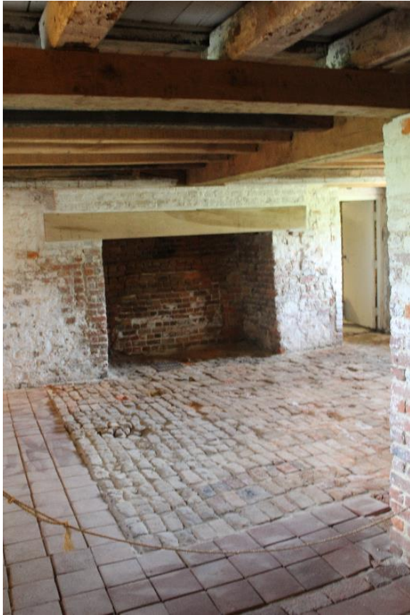
Figure 5.74, Bacon's Castle, ca. 1665 dwelling, Basement, Kitchen, Room 003, general view.
