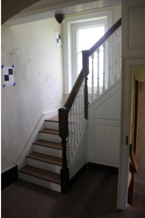
Figure 5.126, Bacon's Castle, ca. 1665 building, North Tower, Room 101, view northwest.
