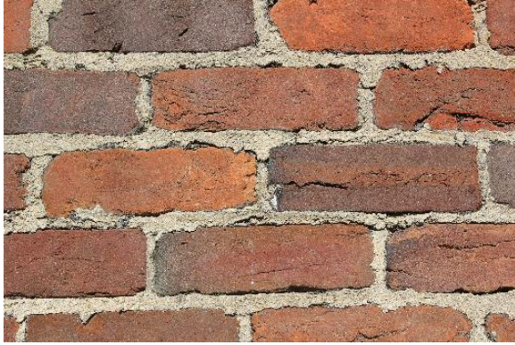
Figure 5.37, Bacon's Castle, East elevation, detail of masonry wall.
