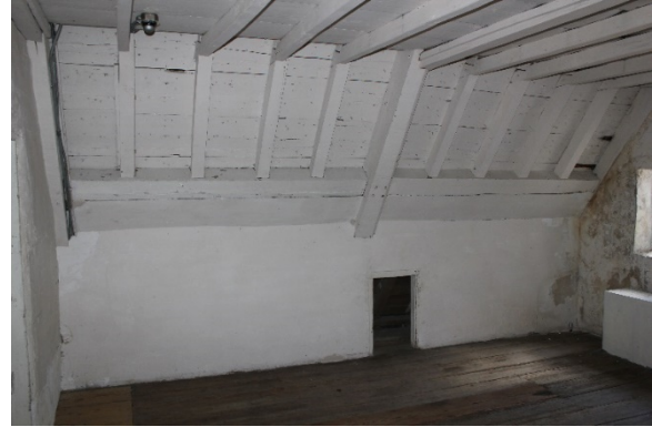
Figure 5.247, Bacon's Castle, ca. 1665 portion, Garret Floor, Room 304, view northeast.
