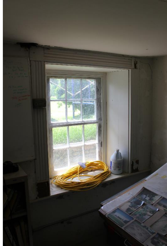
Figure 5.108, Bacon's Castle, ca. 1854 addition, Basement, Room 008,009, western window, south wall.
