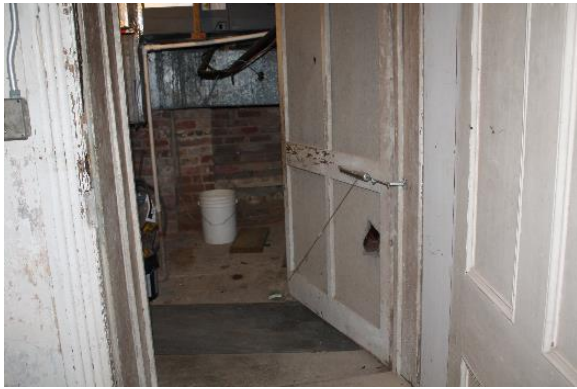
Figure 5.114, Bacon's Castle, ca. 1950s addition, Basement, Room 010, view northwest. Door Detail.
