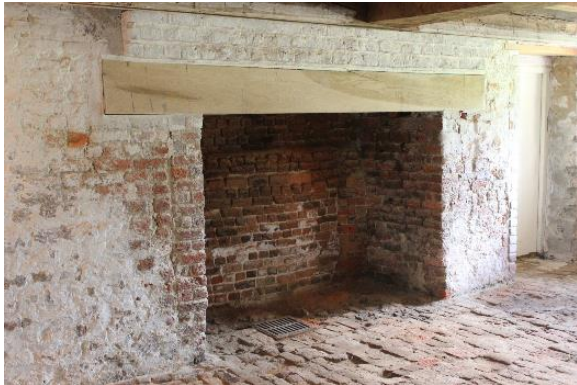
Figure 5.82, Bacon's Castle, ca. 1665 dwelling, Basement, Kitchen, Room 003, view of fireplace. Note the air grille.
