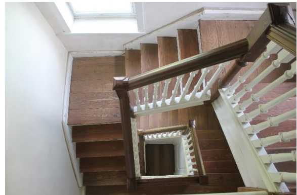
Figure 5.235, Bacon's Castle, ca. 1665 portion, Garret Floor, Room 301, stair.
