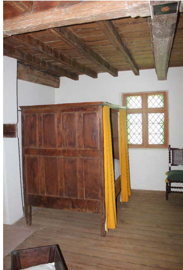
Figure 5.196, Bacon's Castle, ca. 1665 building, Second Floor, West Chamber, Room 203, view northwest.
