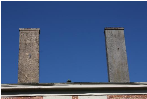
Figure 5.36, Bacon's Castle, East elevation, ca. 1854 addition chimney detail.
