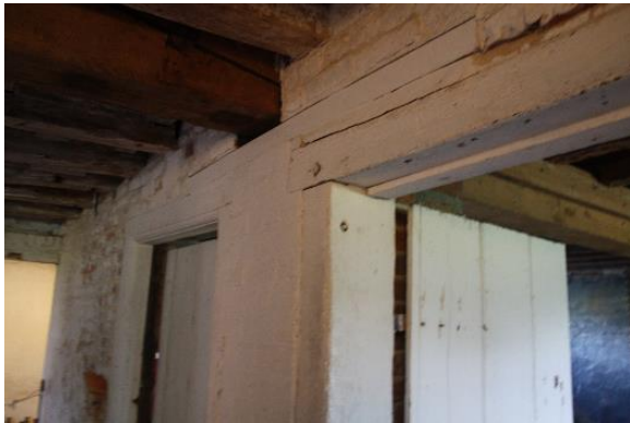
Figure 5.73, Bacon's Castle, ca. 1665 dwelling, Basement, Room 002, detail of door frame.
