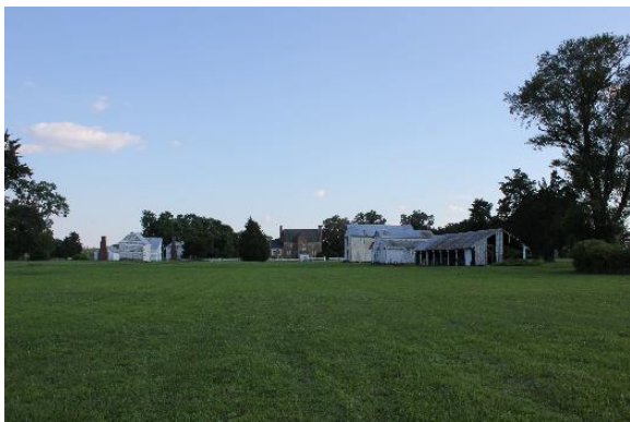
Figure 5.31, Bacon's Castle, North elevation, site, view north.
