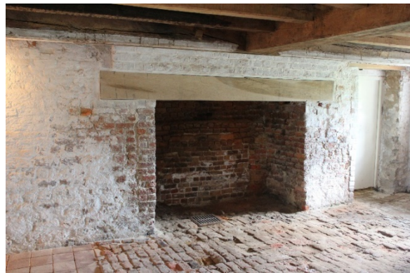
Figure 2.93: Bacon's Castle, Cellar, East Room, view to east. Photograph Commonwealth Architects, 2015.
