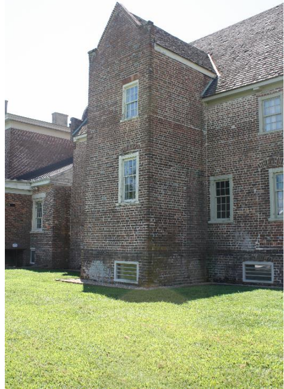
Figure 5.49, Bacon's Castle, West elevation, north tower elevation.
