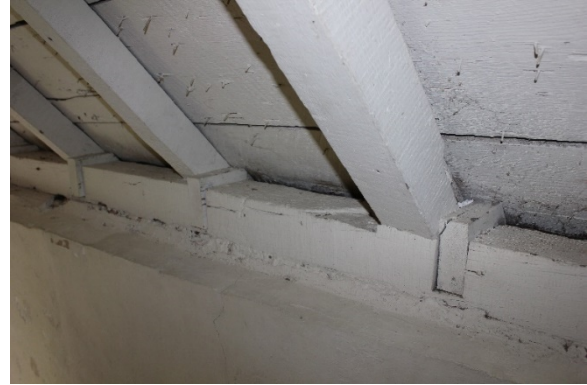
Figure 5.231, Bacon's Castle, ca. 1665 portion, Garret Floor, Room 301, framing detail.
