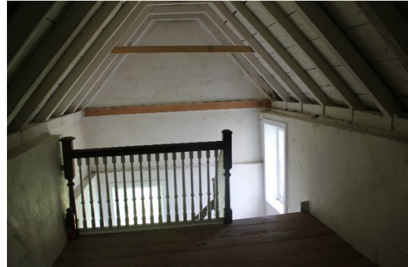
Figure 5.234, Bacon's Castle, ca. 1665 portion, Garret Floor, Room 301, view north.
