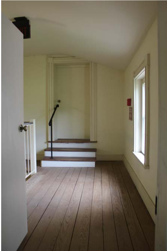
Figure 5.210, Bacon's Castle Hyphen, Second Floor, Room 206, view east.
