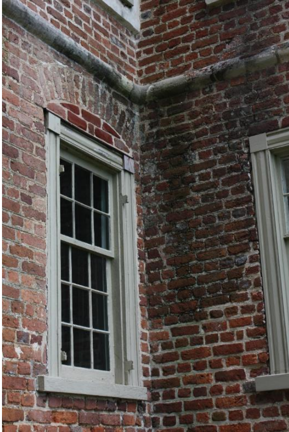
Figure 5.8, Bacon's Castle, South elevation, ca. 1665 building, first floor window.
