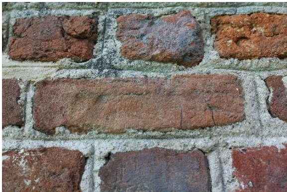
Figure 5.22, Bacon's Castle, South Elevation, restoration mortar.
