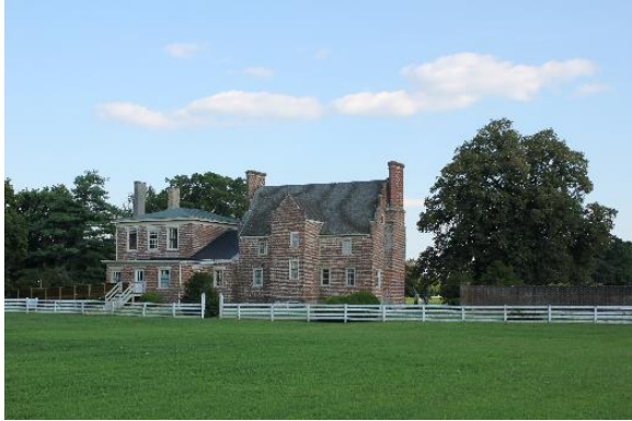
Figure 5.30, Bacon's Castle, North elevation, site, view southeast.
