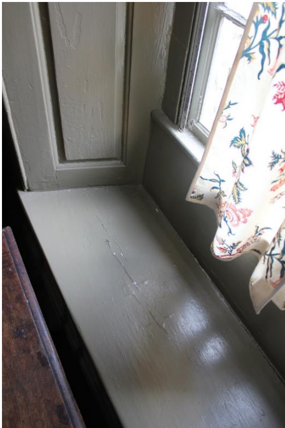
Figure 5.153, Bacon's Castle, ca. 1665 building, East Room, Room 105, detail of paneling and window trim.
