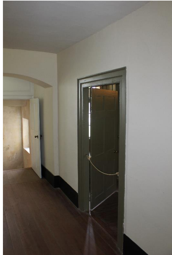
Figure 5.136, Bacon's Castle, ca. 1665 building, Corridor, Room 102, door detail.
