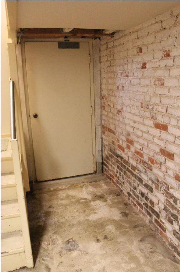
Figure 5.95, Bacon's Castle, Hyphen, Basement, Room 006, general view.
