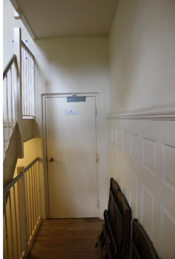
Figure 5.160, Bacon's Castle Hyphen, First Floor, Room 106, view north.
