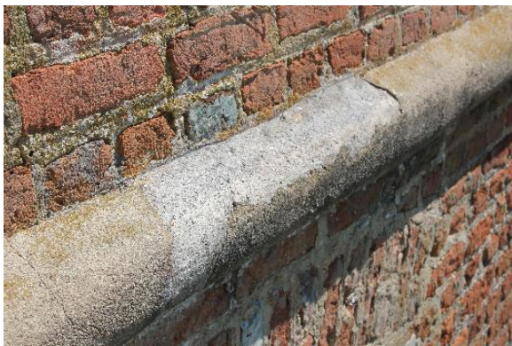
Figure 5.5, Bacon's Castle, South elevation ca. 1665 building, detail of string course.
