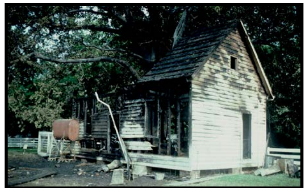
Figure 3.26: Burned 18 th /19 th frame building at Bacon's Castle, facing south.
