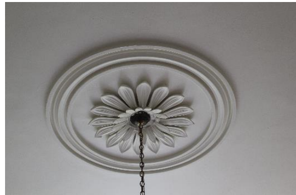
Figure 5.163, Bacon's Castle, ca. 1854 addition, First Floor, Room 107, detail of ceiling medallion.
