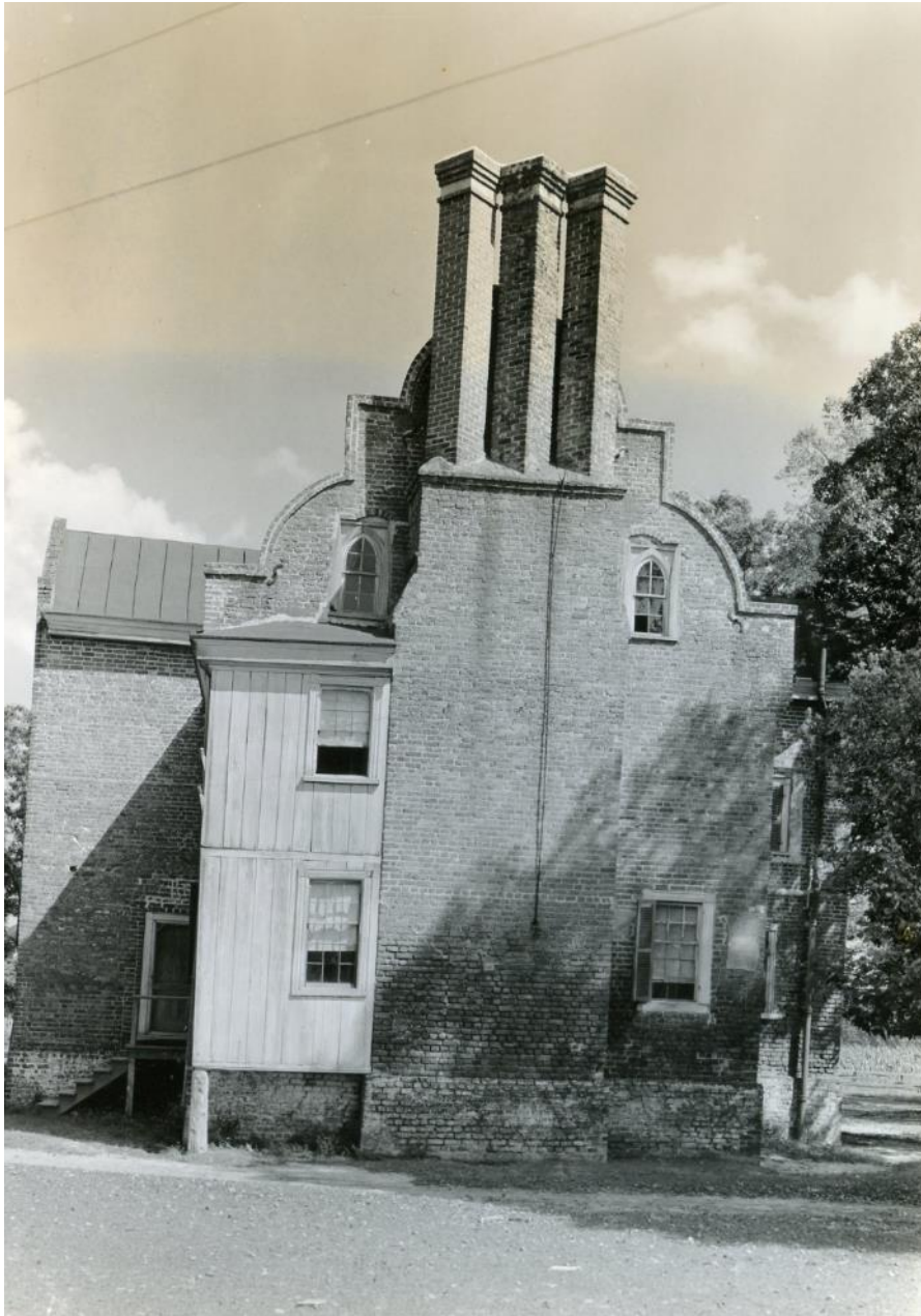
Figure 51: Bacon's Castle, photograph of west elevation, National Park Service, 1937.
