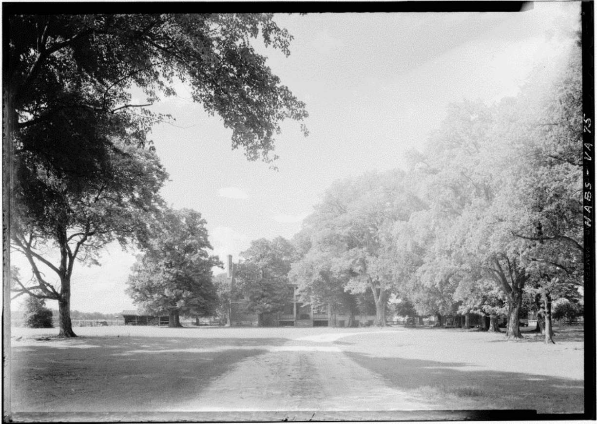
Figure 21: Bacon's Castle, photograph of approach to south (front) elevation, Historic American Buildings Survey, ca. 1937.
