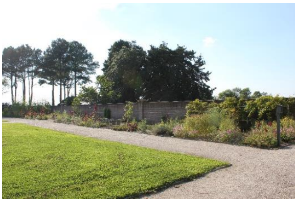
Figure 5.62, Bacon's Castle, West elevation, site, view northwest.
