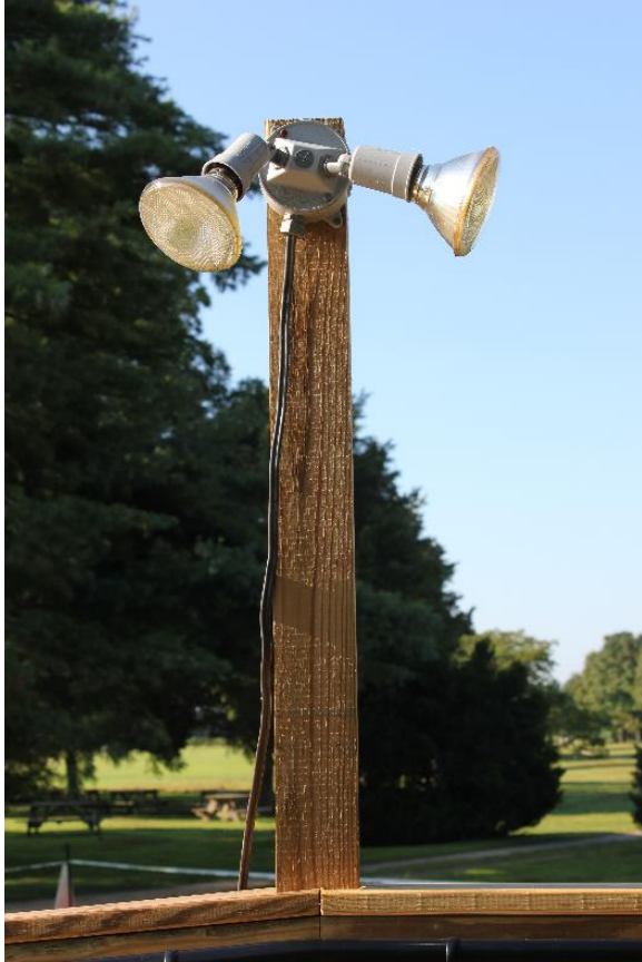
Figure 5.44, Bacon's Castle, East elevation, lighting located on the modern handicapped ramp.
