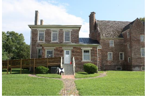
Figure 5.28, Bacon's Castle, North elevation, wooden porch and ADA-accessible ramp.
