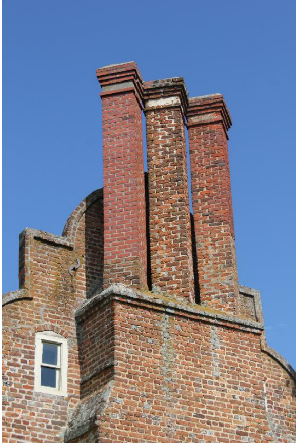
Figure 5.52, Bacon's Castle, West elevation, chimney detail.
