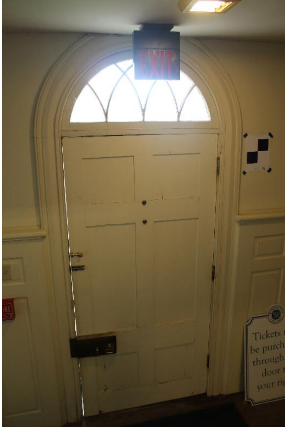
Figure 5.159, Bacon's Castle Hyphen, First Floor, Room 106, detail of museum's main entry. Note how the gypsum wall board intersects the upper trim of the door.
