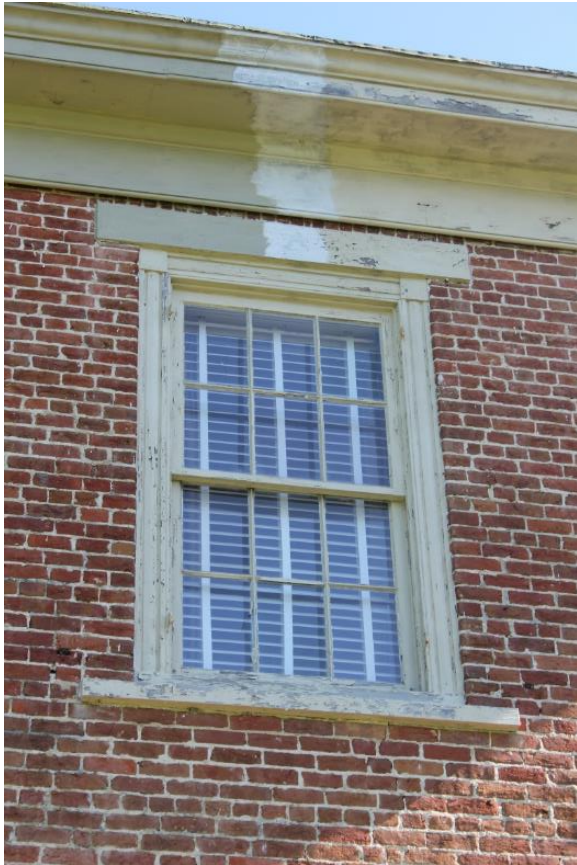
Figure 5.11, Bacon's Castle, South elevation, ca. 1854 addition, second floor window.
