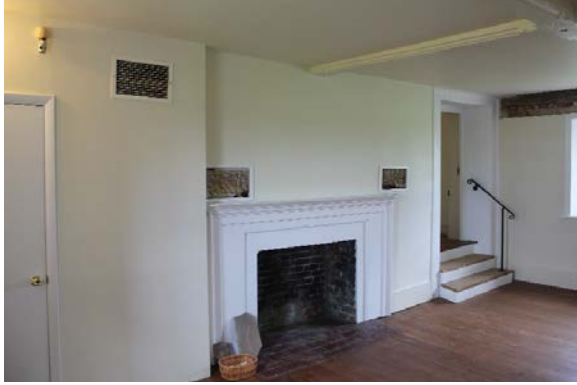
Figure 5.206, Bacon's Castle, ca. 1665 building, Second Floor, East Room, Room 205, view east.
