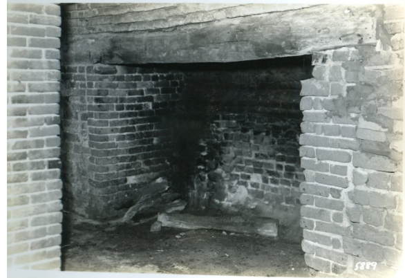
Figure 2.62: Bacon's Castle, Basement, fireplace in east wall. Victor C. Sloane, Architectural Report on Bacon's Castle, Surry County, Virginia. National Park Service, 20 September 1937.
