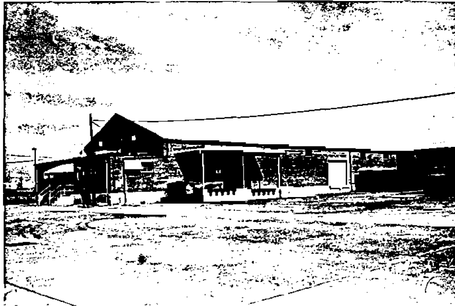
Fig. 14. Waller Depot, Henrico County, general view. (Land and Community Associates)
