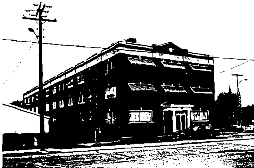
Fig. 27. Manufacturing Buildings, Virginia Industries for the Blind, Charlottesville. (Land and Community Associates)
