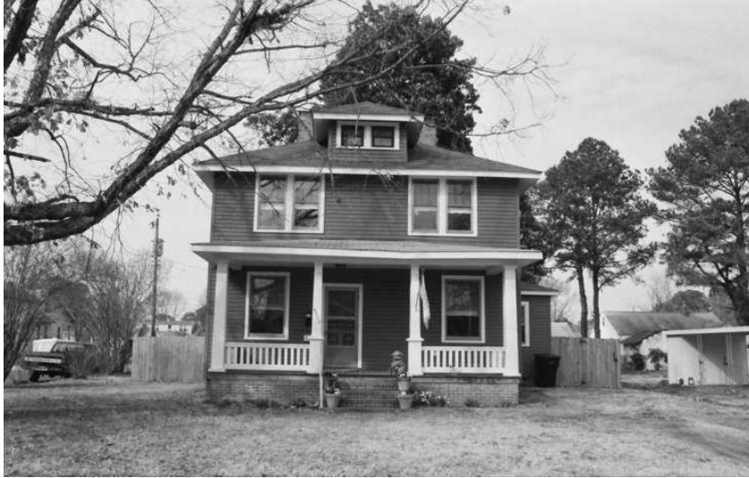
Figure 16. Example of American Foursquare style (124-5107) in the Waterview area of Portsmouth.
