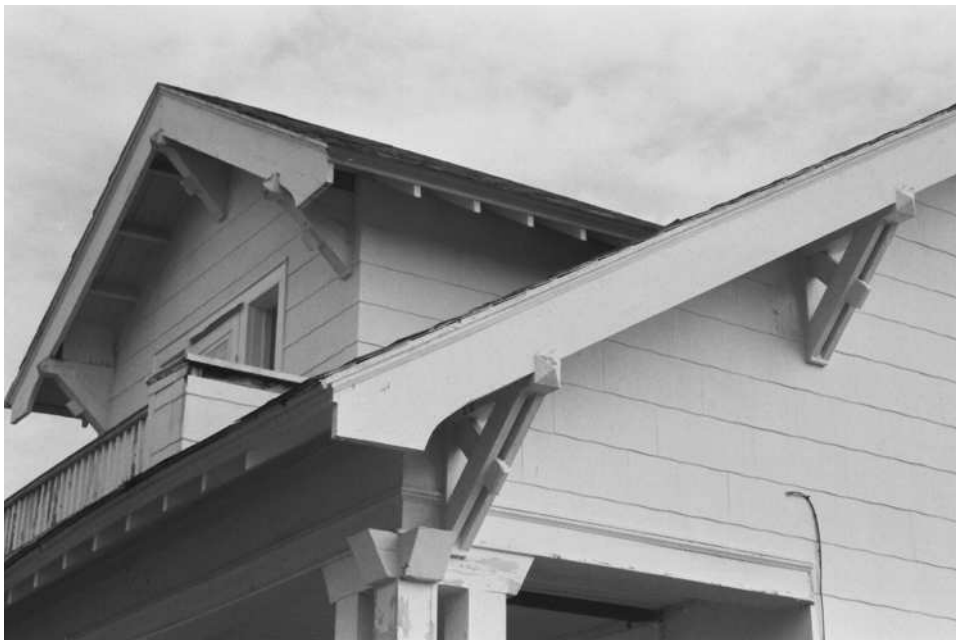
Figure 40. Detail of roof brackets on Sears Westly model (124-5106) in the Waterview area of Portsmouth.
