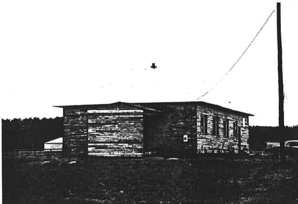
Figure 26: Photograph of Old Charity School Auditorium
