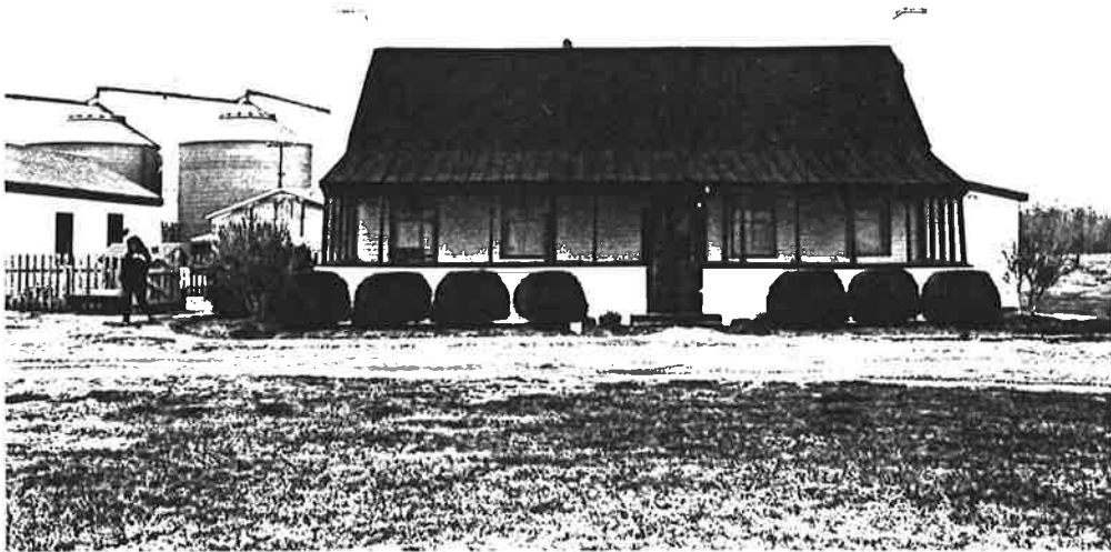
Figure 16: Photograph of the Farmhouse at 773 Princess Anne Road
