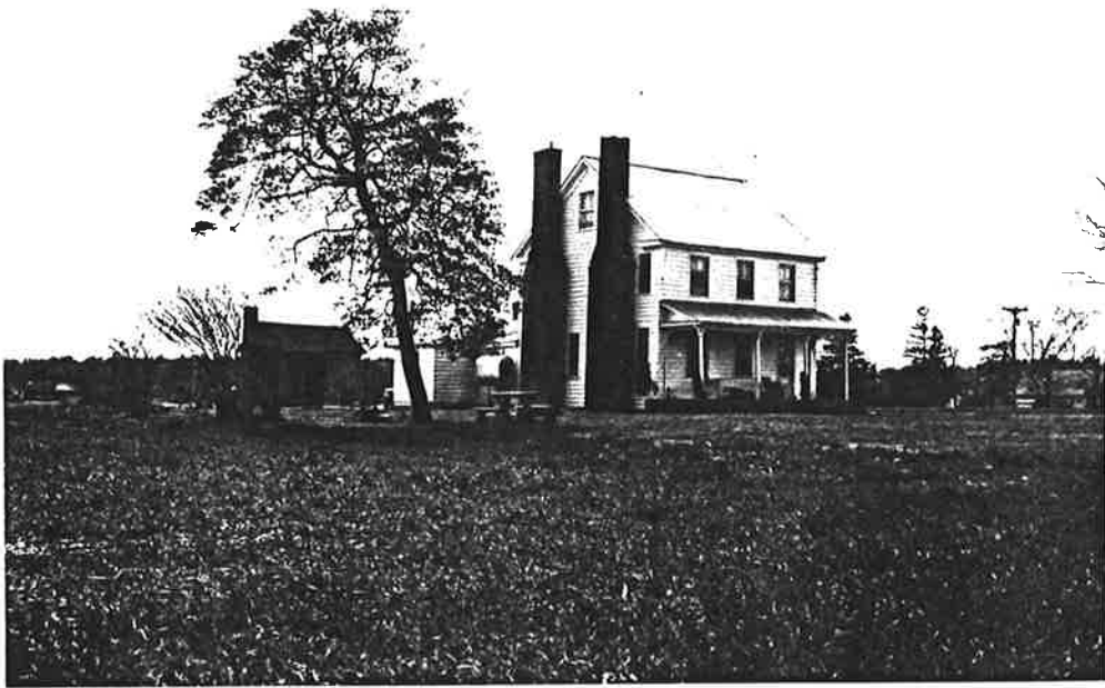
Figure 15: Photograph of James House
