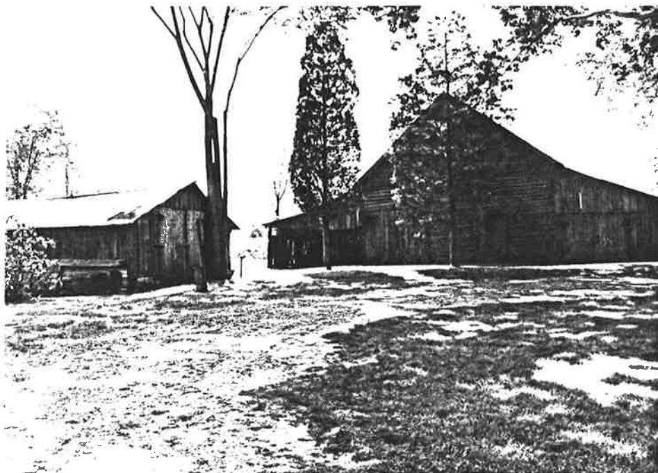
Figure 6: Photograph of Farm Buildings at Davis Farm
