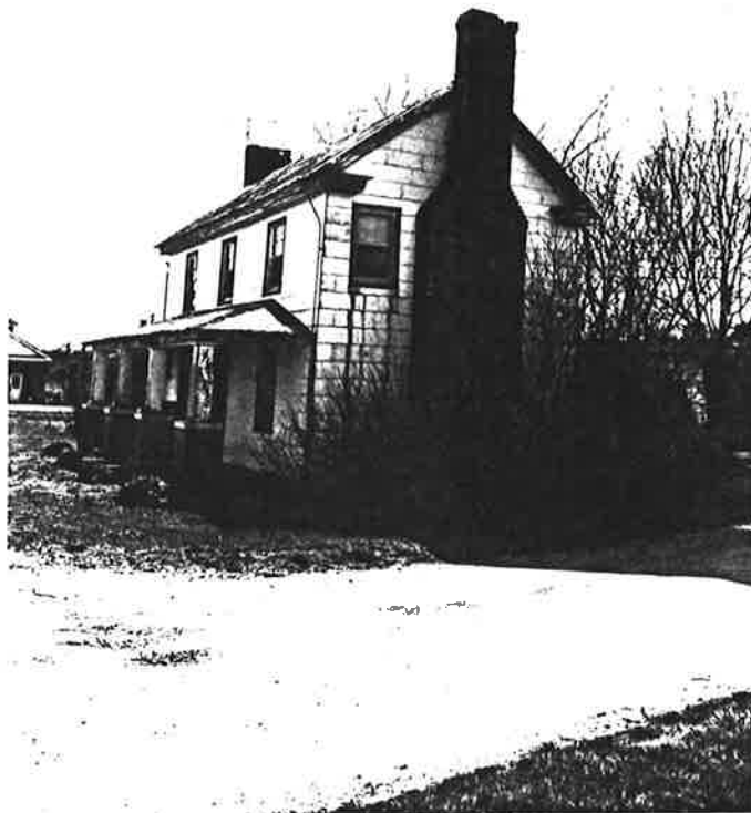
Figure 19: Photograph of Fisher House
