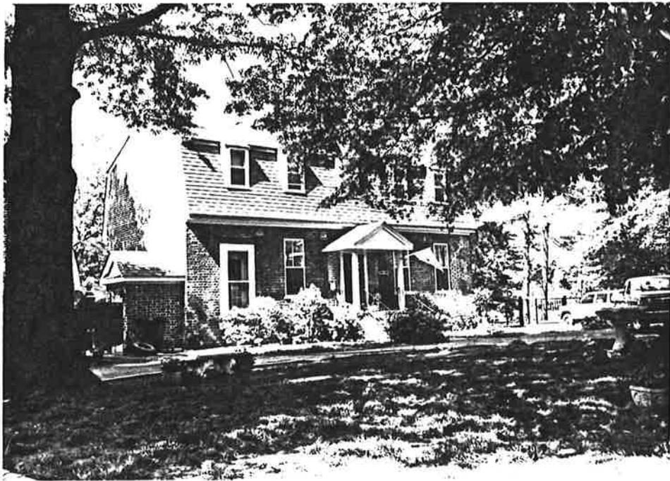
Figure 10: Photograph of the Isaac Murry House
