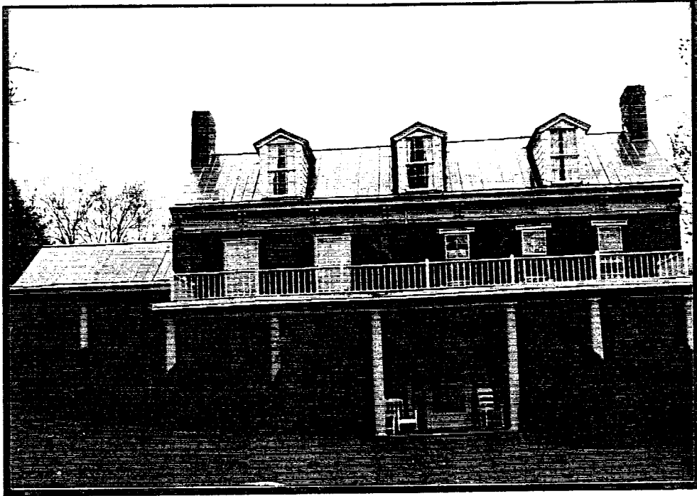
Figure 16: Retirement at 702 Colonial Road (140-6).
