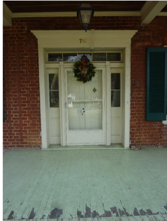
Figure A17: North Façade Entry Door.
