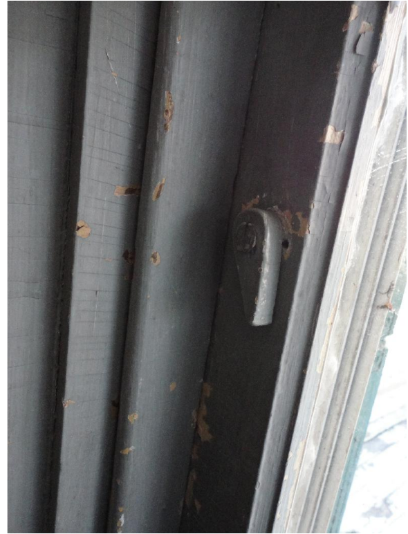
Figure A8: Pivot for propping windows open.
