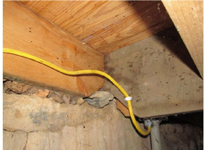
Figure S4: Porch framing
