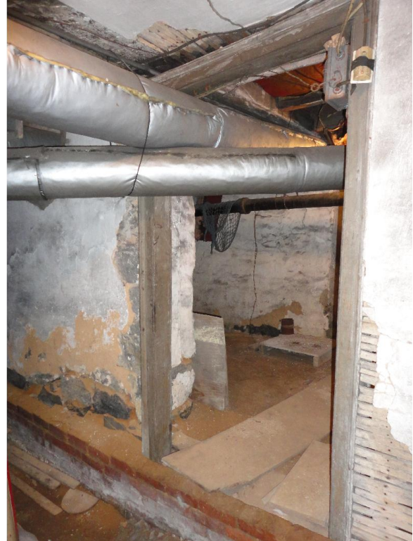
Figure A11: Western basement room, looking toward the eastern room.
