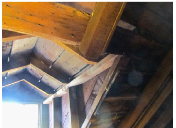
Figure S15: Dormer window framing
