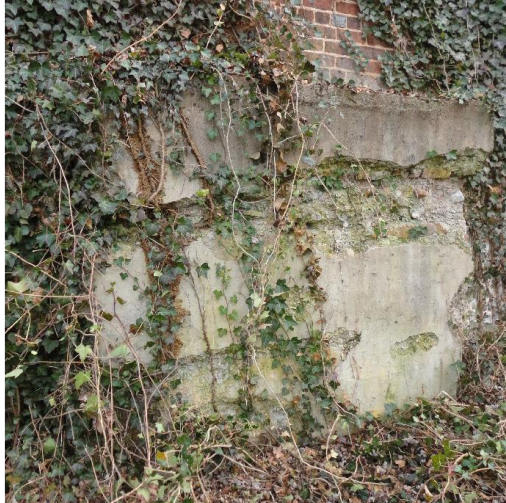
Figure A44: Concrete at west facade.
