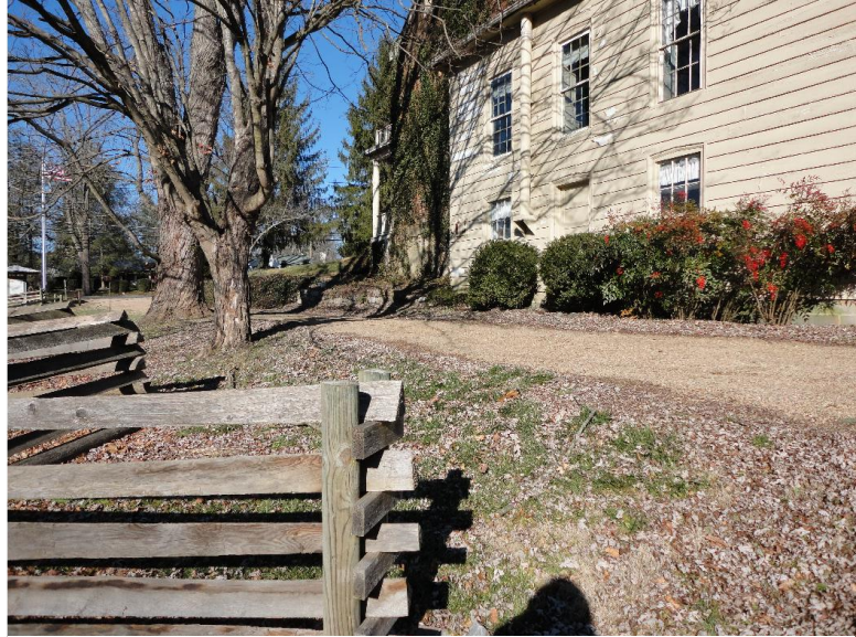
Figure A25: West Façade of Rear Addition. Source: DBA.
