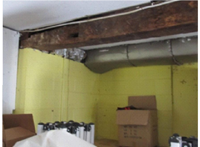
Figure S19: Rear wood-framed addition basement
