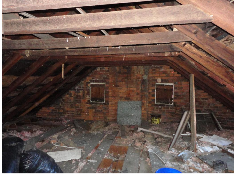
Figure A15: Attic view, looking west toward original gable end.
