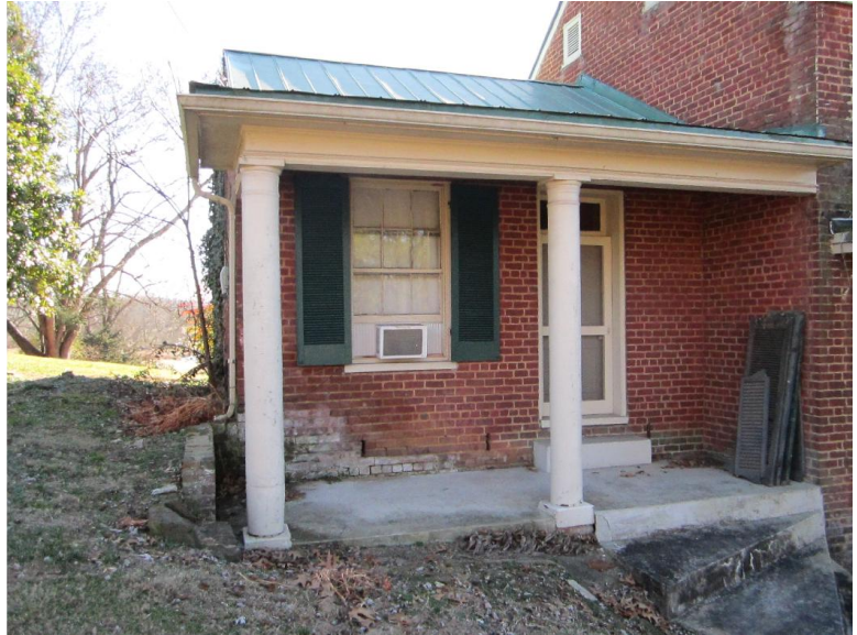
Figure A18: North façade of Office. Source: LPA.
