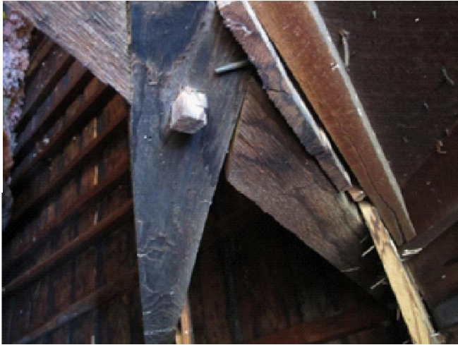
Figure S10: Attic framing at Retirement I
