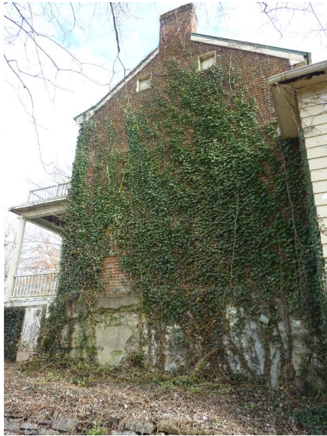
Figure A34: West facade.
