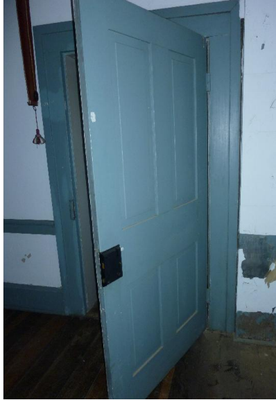
Figure A49: Door D10 showing raised panels.
