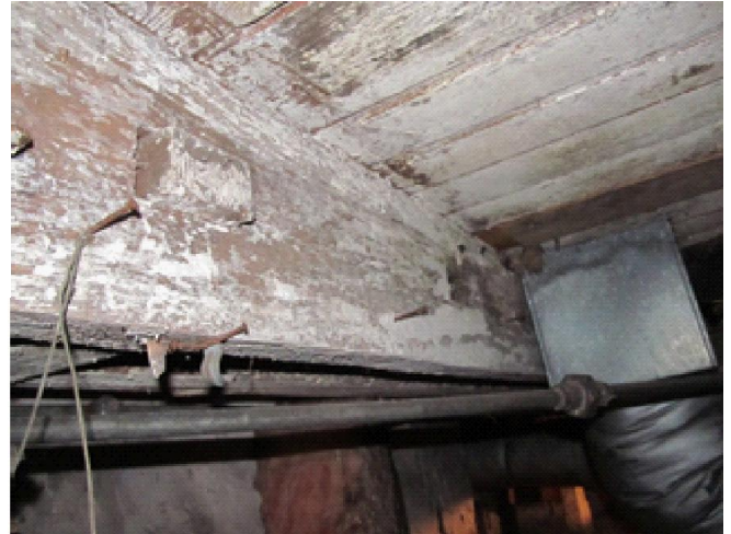
Figure S7: Mortise/tenon connection
