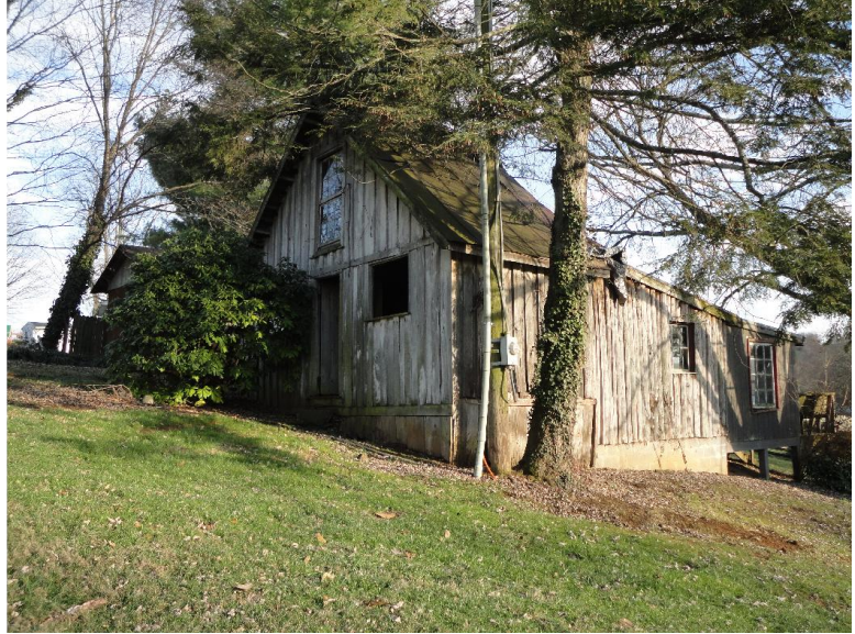
Figure A33: Outbuilding, showing two additions.
