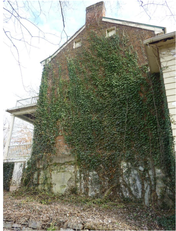
Figure A10: West Façade.
