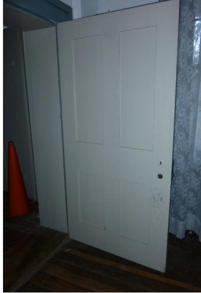
Figure A50: Door D10 showing flat panels.
