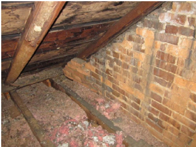
Figure S12: Gable end brick
