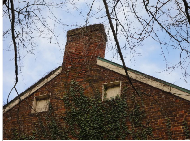
Figure A43: West chimney.
