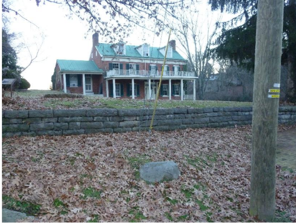
Figure A62: New metal roof.
