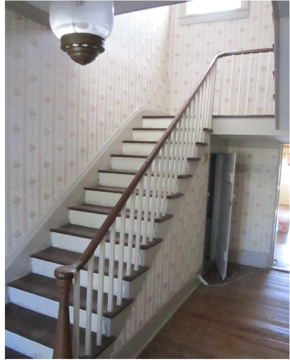
Figure A21: New main stair, Entry 100.
