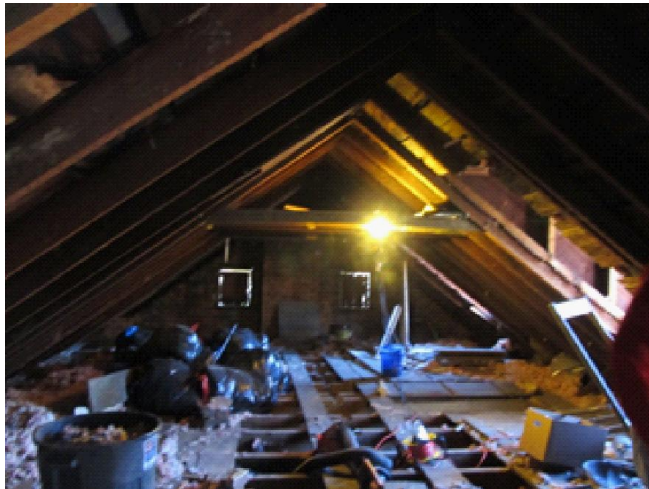
Figure S11: Attic framing
