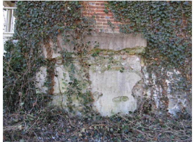
Figure S1: Concrete Cap at West Facade
