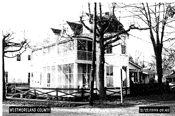
Figure 97 House Irving Avenue South (199-5018-0018), Digital Collection, HaAR
