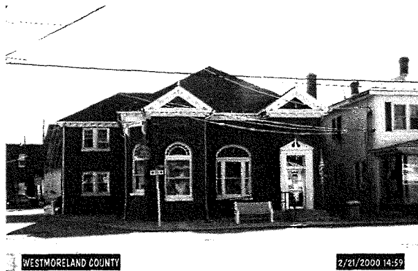
Figure 115 Former Bank of Westmoreland (199-5006-0006), Digital Collection, HaAR
