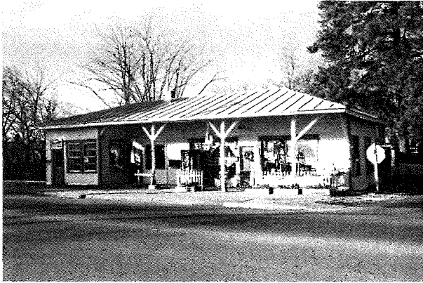
Figure 125 Former Auto Repair Garage (199-5012-0012), Digital Collection, HaAR
