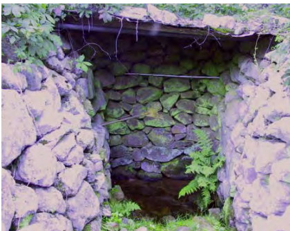
Figure 40. Detail of spring chamber.
