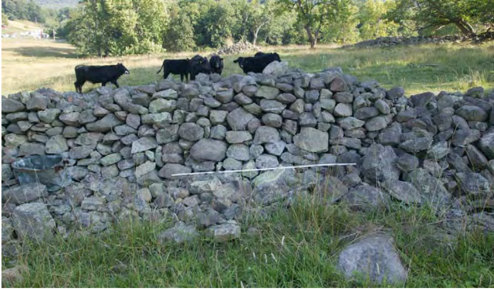
Figure 59. Elevation at Area 11, looking south.
