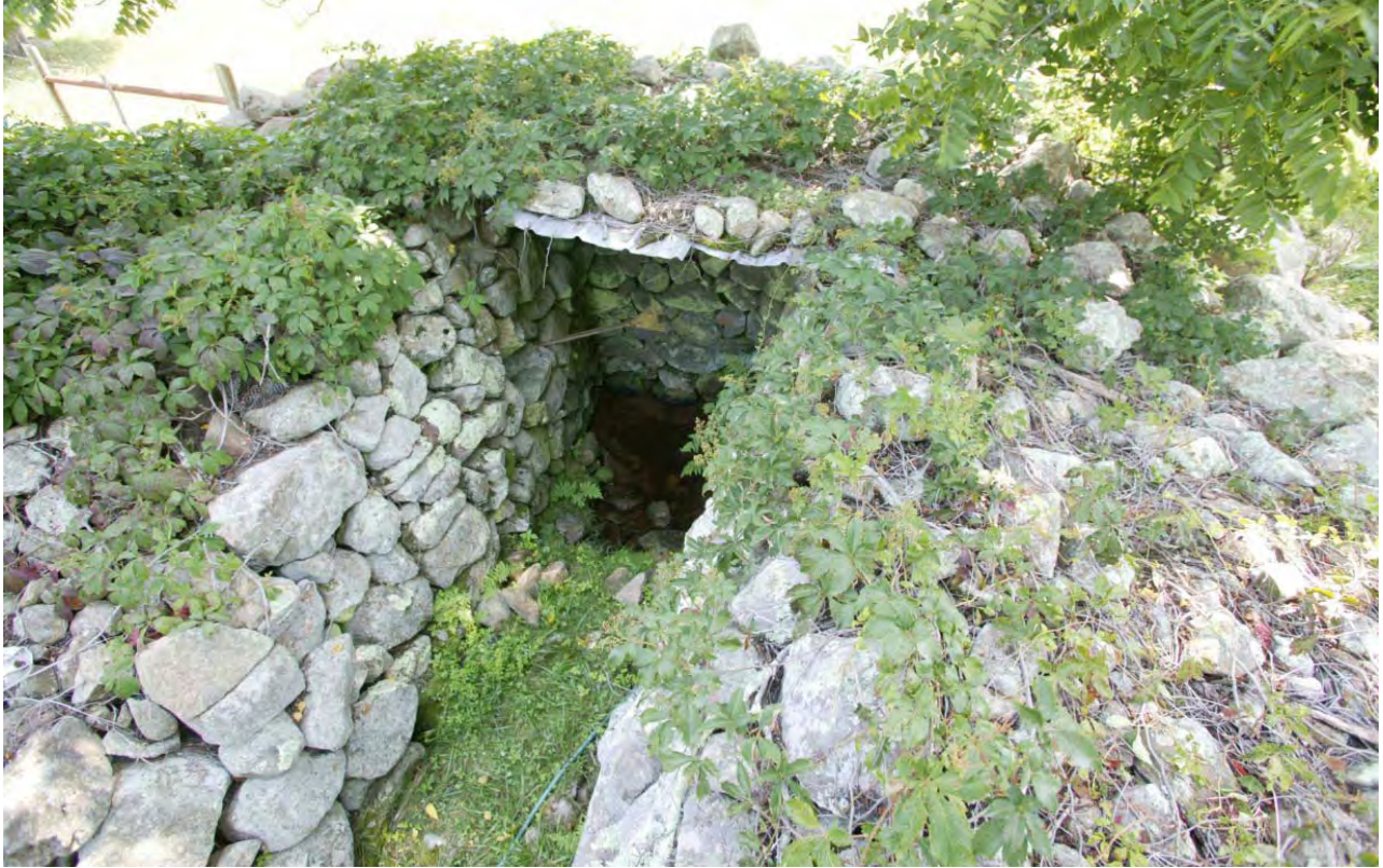
Figure 37. Overhead view of entranceway to spring enclosure.
