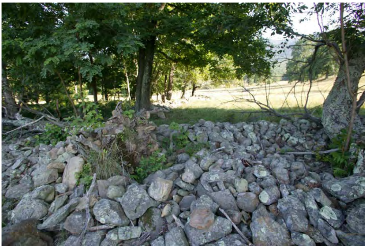
Figure 62. Area 13, collapsed spur of main wall, looking southeast.
