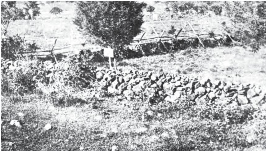
Figure 76. Stone walls in front of Giles Partlow farmhouse (above) and on the battlefield at Gettysburg, Pennsylvania (left, Horan 1955:Plate 138), both supplemented by wood fencing. With these adaptations, a low wall becomes an effective enclosure while considerably reducing expenditure on timber. Also, posts supported by cobbles (above) would resist rot much longer than when planted in the moist ground.
