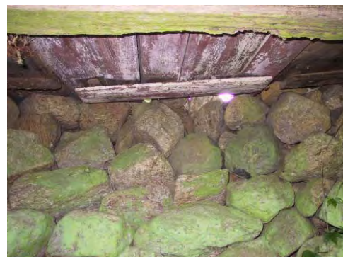
Figure 41. Roof of spring chamber.
