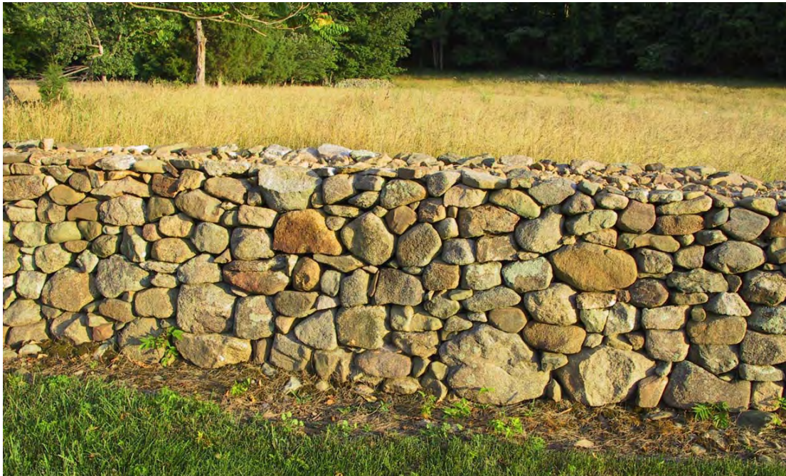
Figure 72. Face of wall rebuilt by Clem brothers showing tightly fitting face stones.
