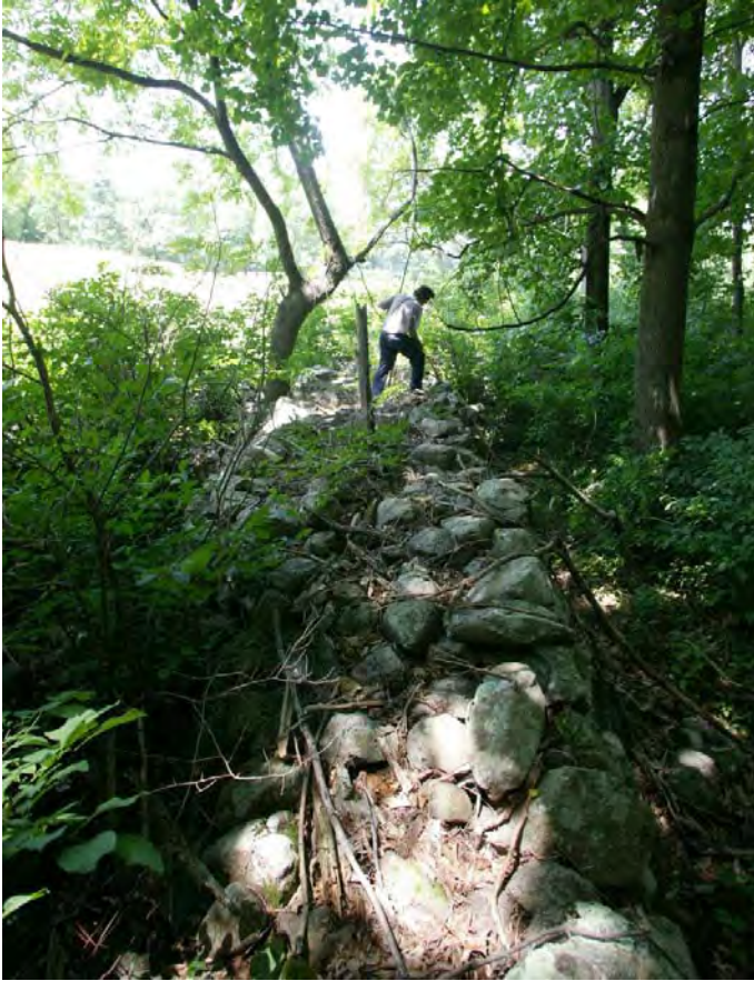
Figure 29. Top of massive wall that parallels upper portion of Gooney Run, looking north.
