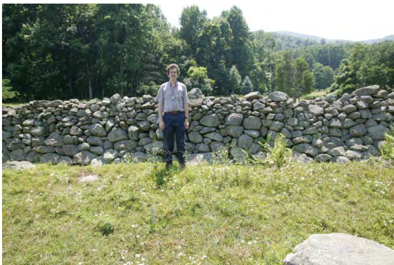
Figure 33. View of northern face of Area 6 wall.
