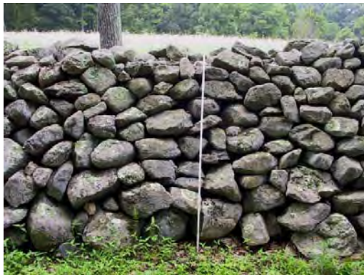
Figure 21. Elevation view of high west wall at the lower end of lane. (Measuring stick is 6.6 ft.)
