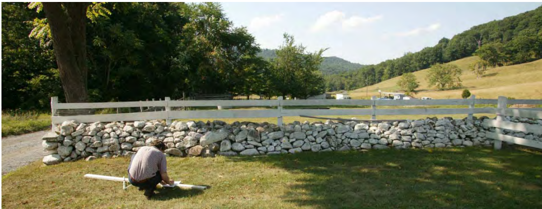
Figure 51. Elevation of wall on north side of driveway, looking north.
