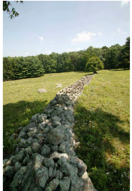
Figure 32. View to the east along top of wall at Area 6.
