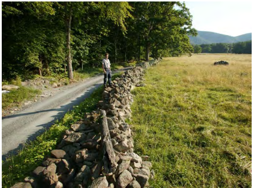
Figure 64. Roadside wall north-east of Perna property, looking southwest.
