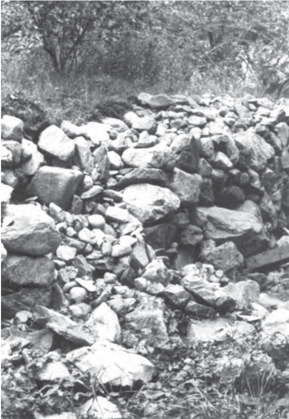
Figure 75. Partially collapsed New England walls made of smoothed glacial rock (Wooley and Raitz 1992:100).
