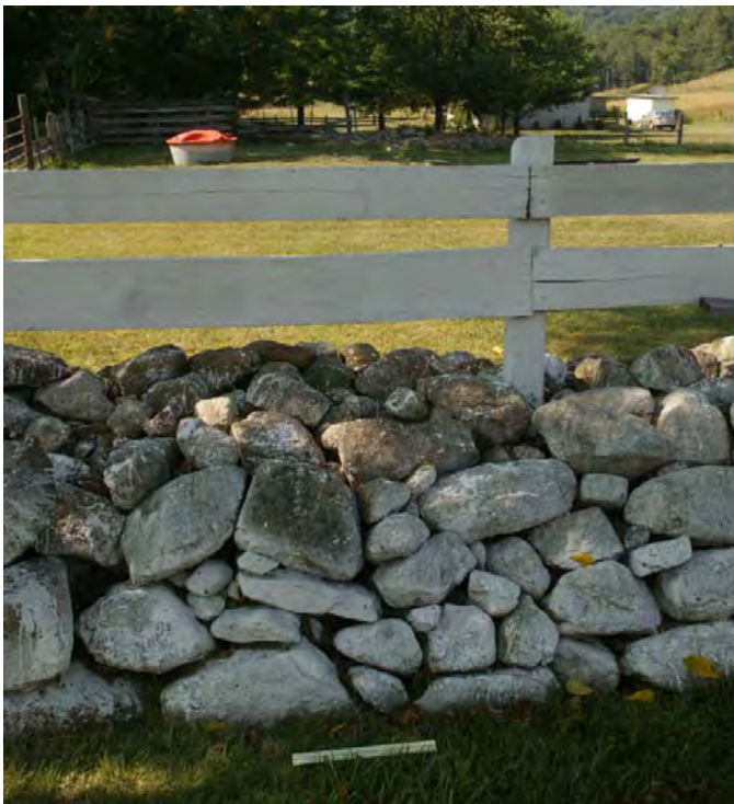
Figure 52. Detail of wall on north side of driveway topped with wooden fence.
