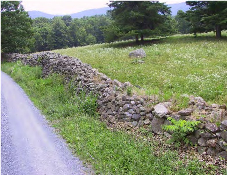
Figure 18. Road frontage walls at western edge of Perna property. Apart from the section in the foreground much of the wall is in good condition.
