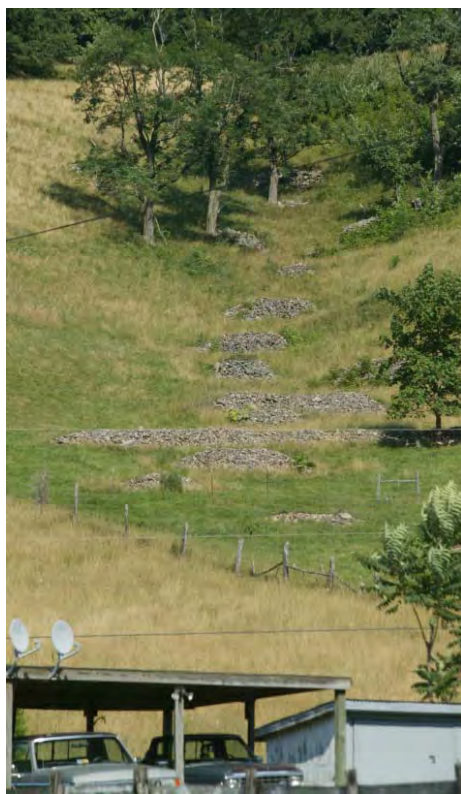
Figure 54. Check dams in gully, looking southeast.
