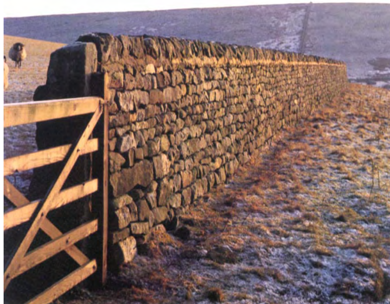
Figure 25. Typical steep-sided Yorkshire wall suitable for enclosing the sheep shown on the left side of the picture (Lund et al. 1992:17).
