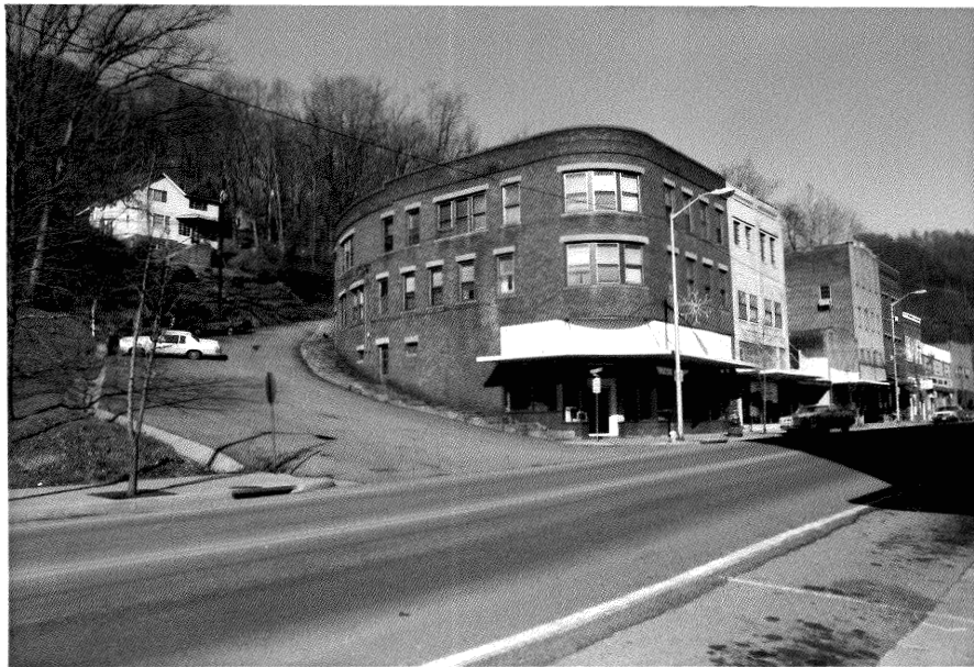
Figure 26: Commercial/Residential Building (97-28) Southwest & Southeast Elevations
