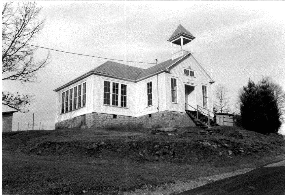
Figure 45: Dewey School (97-390) West & South Elevations
