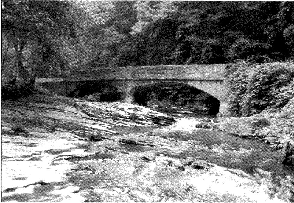
Figure 67: Bridge (97-197) West Elevation
