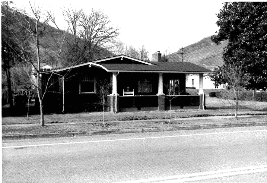
Figure 40: House (101-57-12), Big Stone Gap Southeast Elevation
