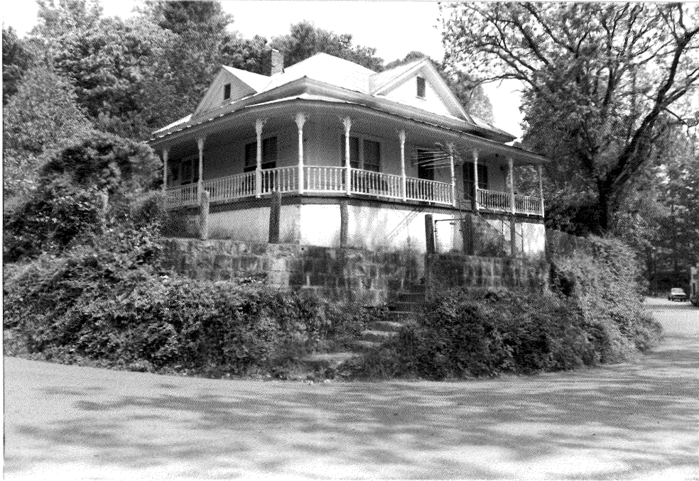
Figure 29: Hamm House (97-18) Southwest & Souteast Elevations
