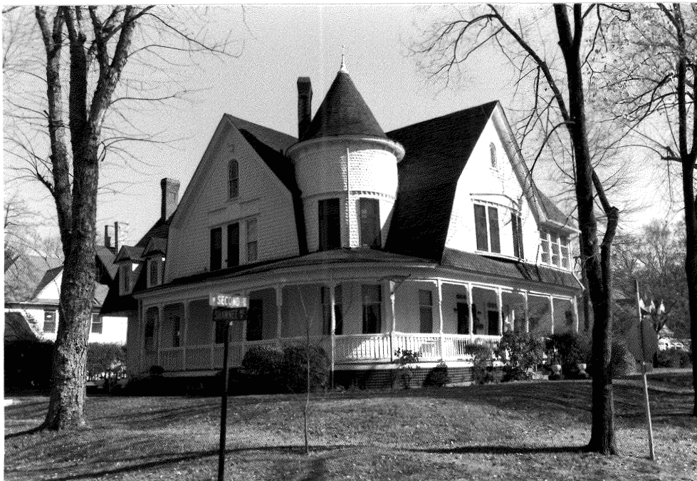
Figure 19: Ted Wentz House (101-13) West Corner
