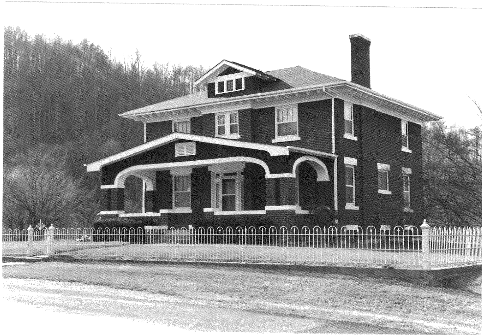
Figure 22: Taylor House (97-324) Southeast & Northeast Elevations
