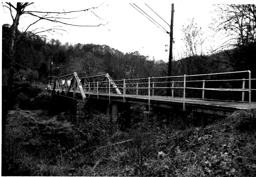
Figure 69: Bridge (101-40) Looking Southwest
