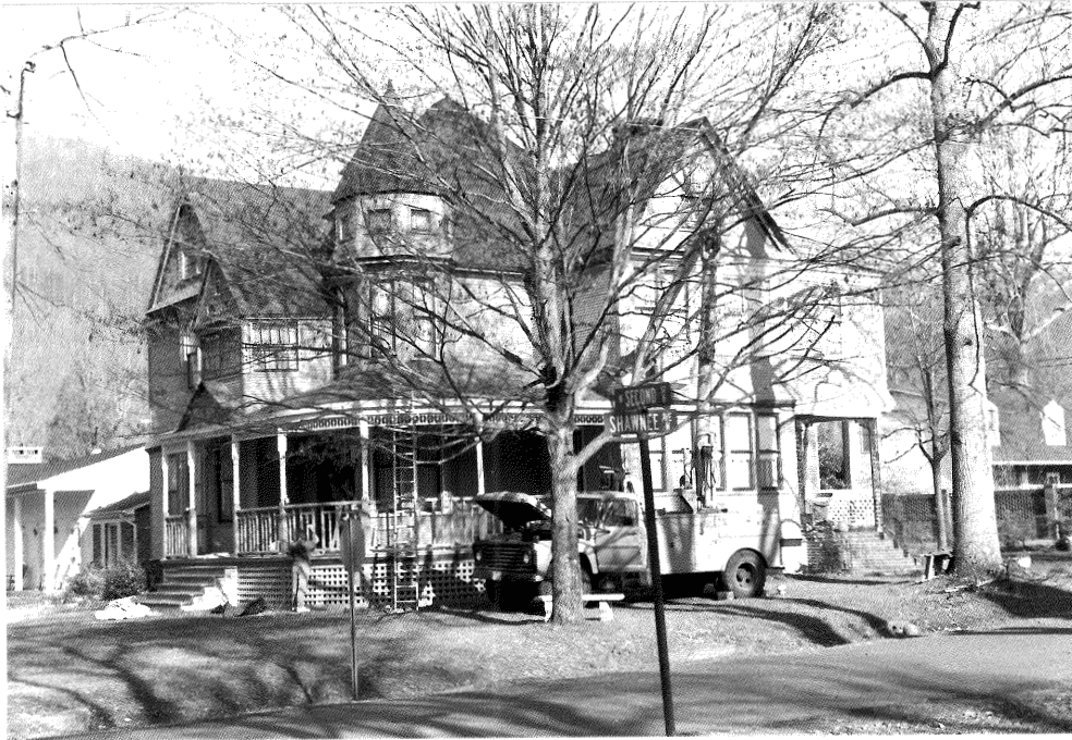
Figure 18: John K. Taggard House (101-15) South Corner
