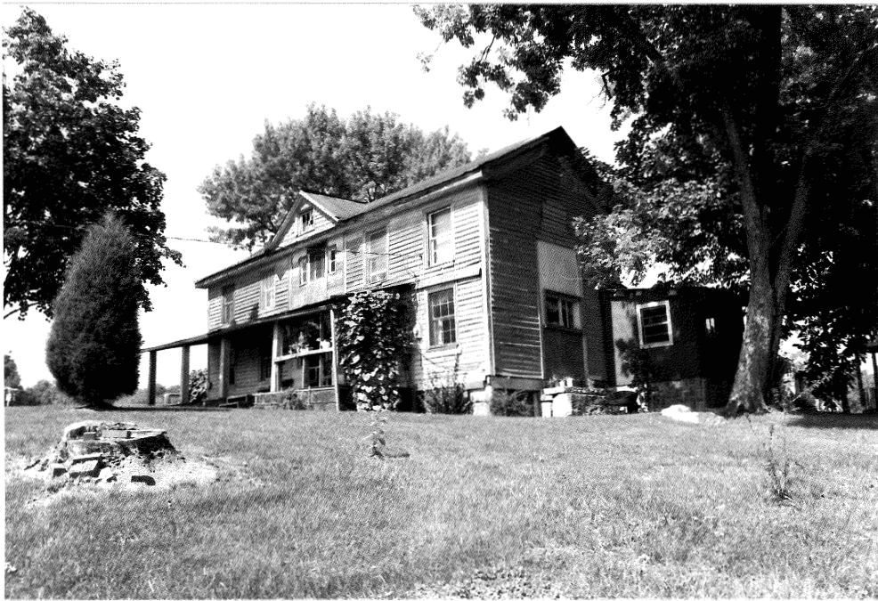
Figure 15: Wycliffe Nash House (97-258) West & South Elevations
