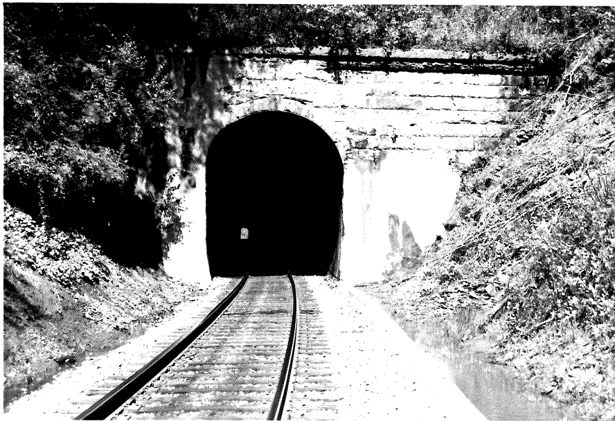
Figure 66: Holbrook Tunnel (97-227) East Entrance
