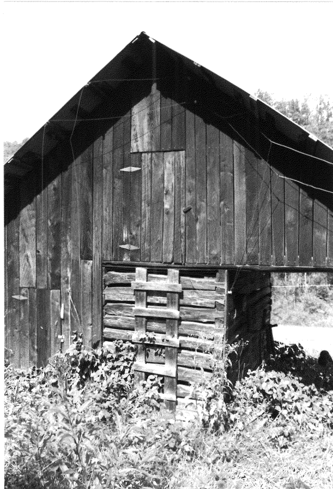
Figure 38: Log crib Travis Baker Farm (97-298) South Elevation
