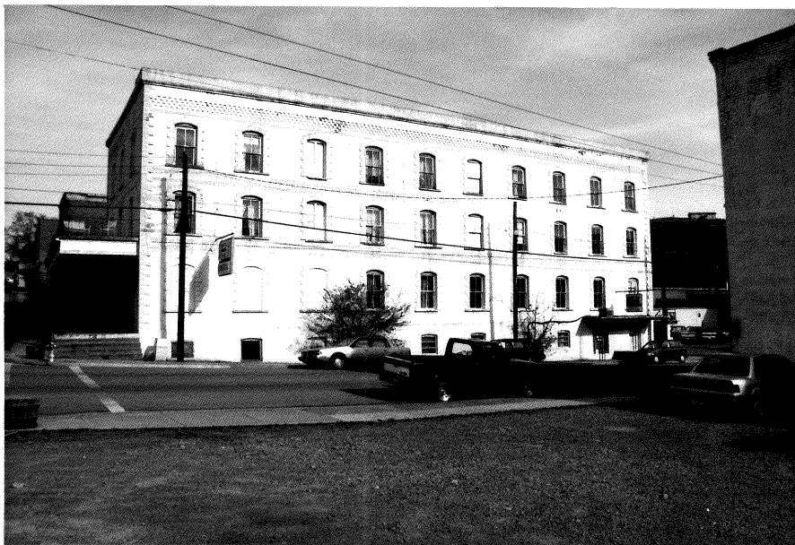
Figure 27: Blue Sulphur Hotel (97-178-1) West Elevation
