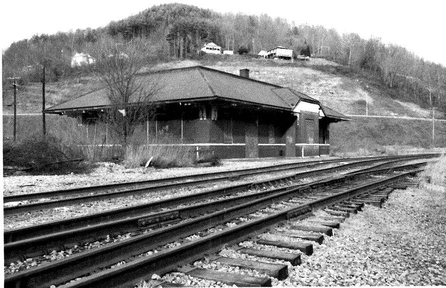
Figure 63: L & N Railroad Station (97-31) Southwest & Southeast Elevations
