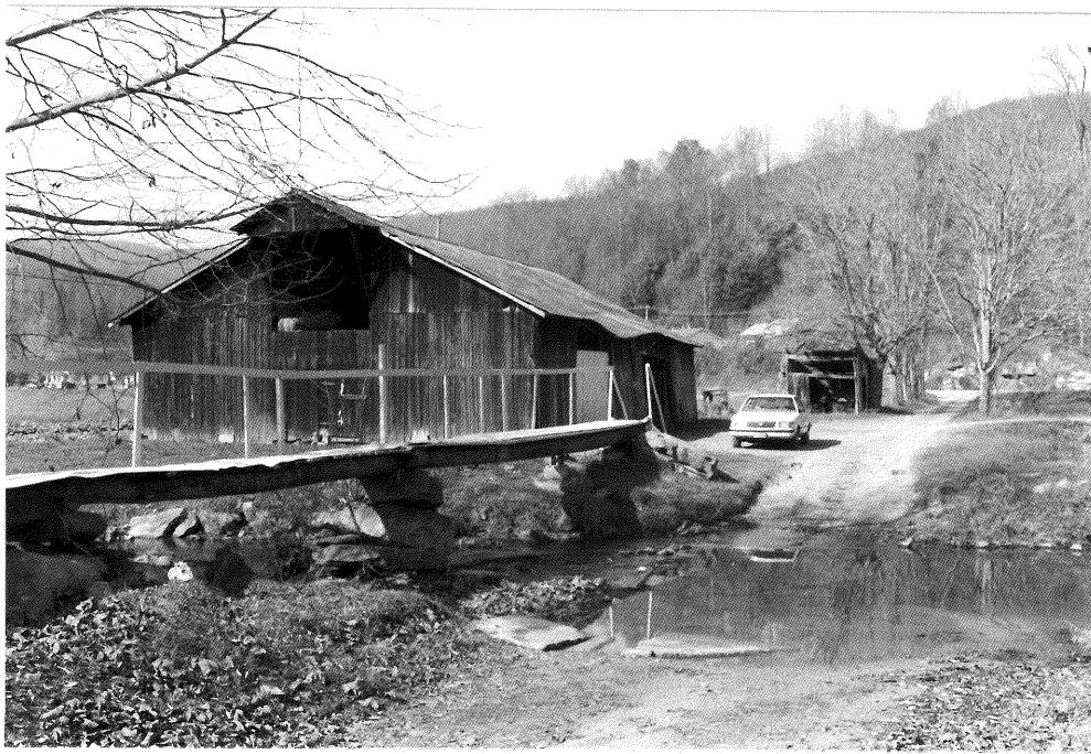
Figure 35: Slemp Farm (97-334) Looking North
