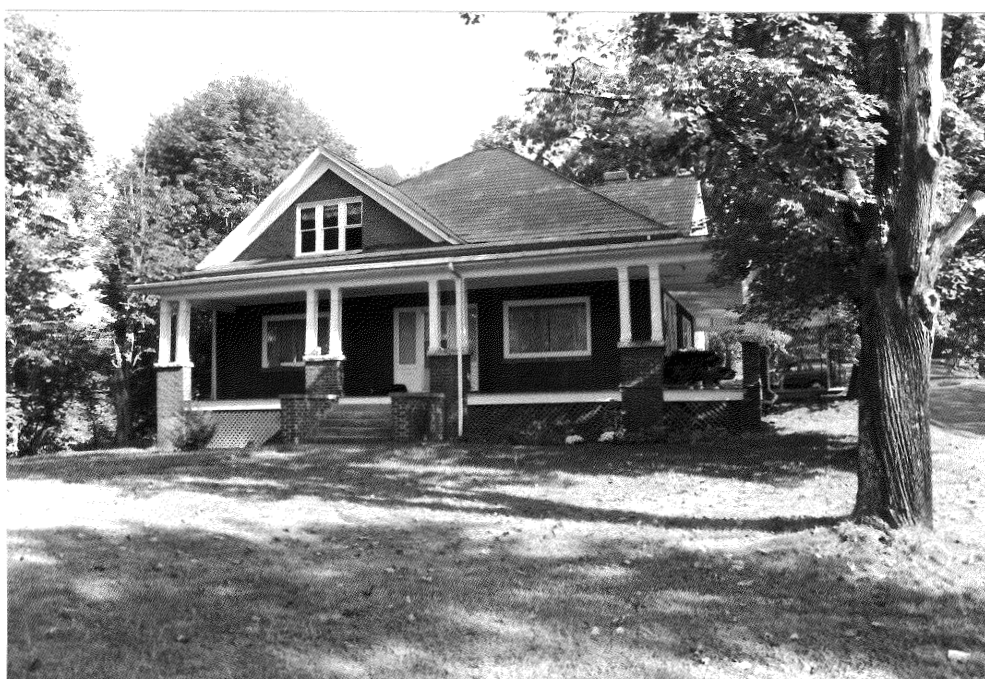
Figure 21: Hillman/Banner House (97-228-5) South Elevation
