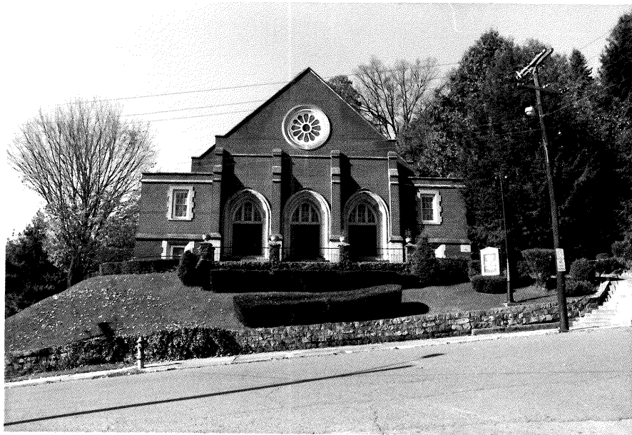
Figure 51: Norton United Methodist Church (146-11) East Elevation
