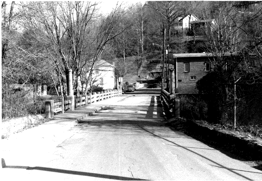
Figure 68: Inman Street Bridge (97-362-12) Looking East
