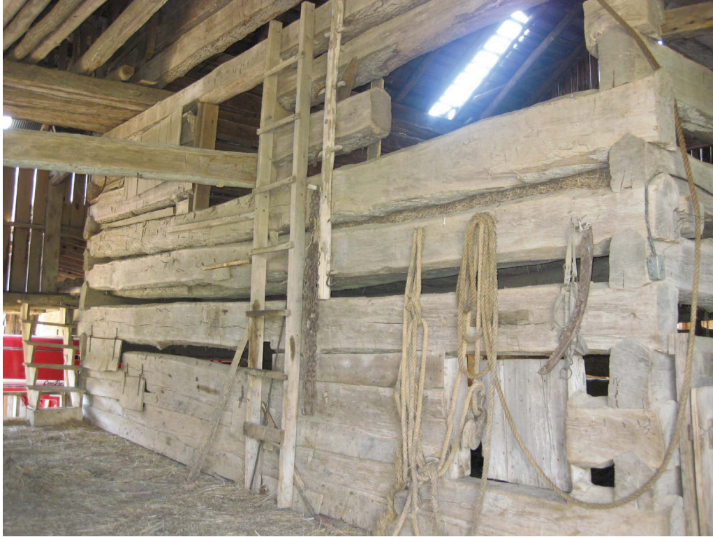
Figure 95. Fracture Creek Farm (098-5190), log barn interior.
