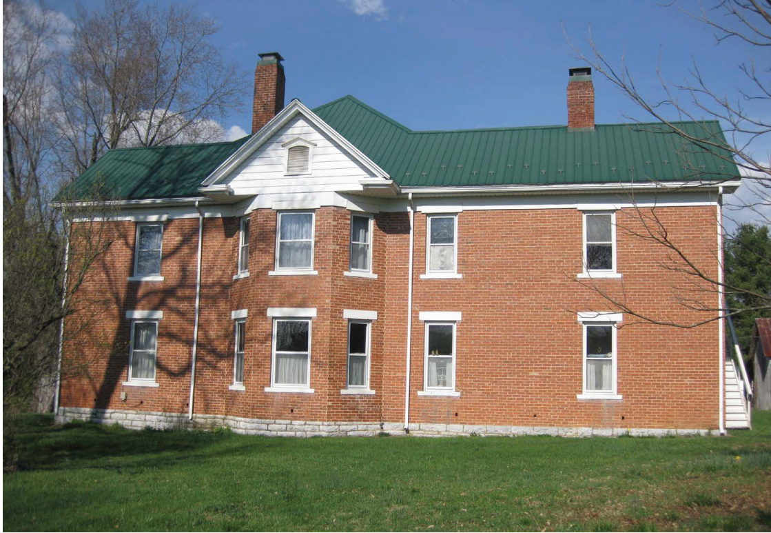
Figure 37. Mill Creek Studio (098-5191), southwest elevation.
