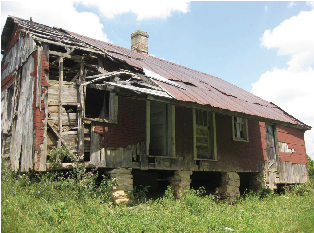
Figure 54. Tenant House, Peppers Ferry Road (098-5330), south elevation.
