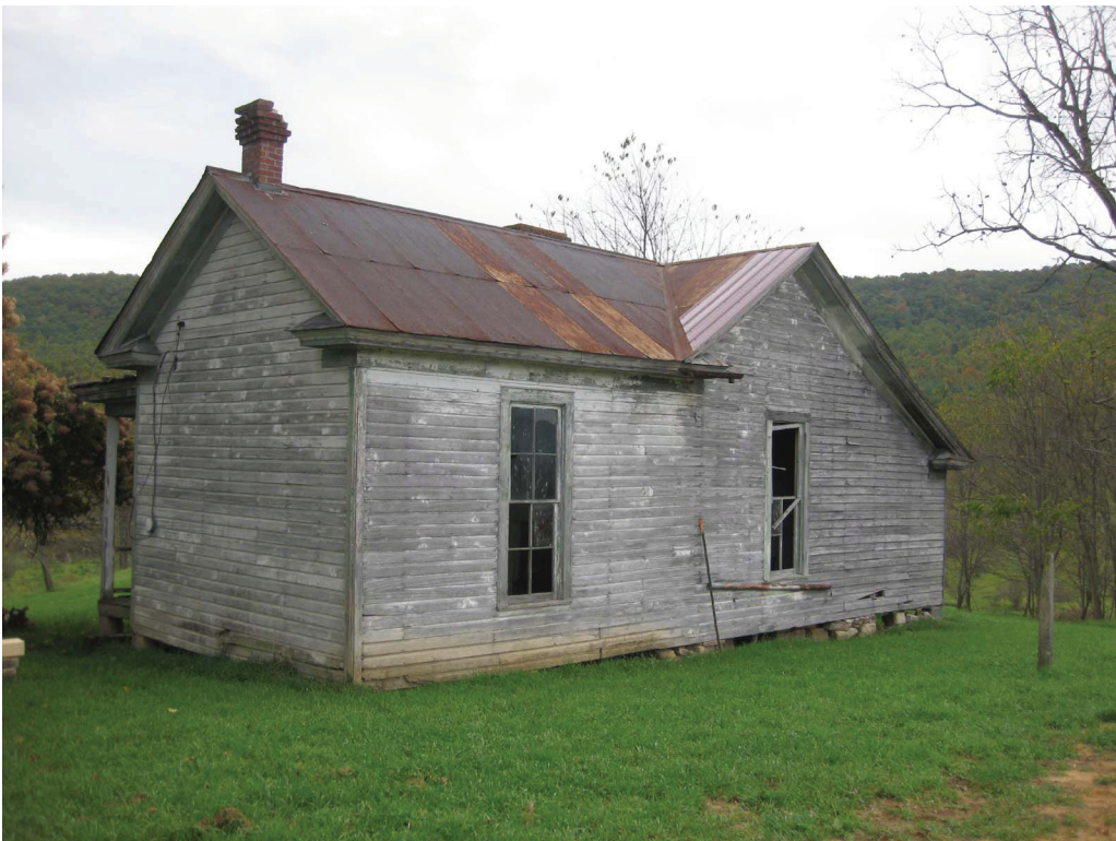
Figure 34. House, Crocketts Cove Road (098-5383), southwest elevation.
