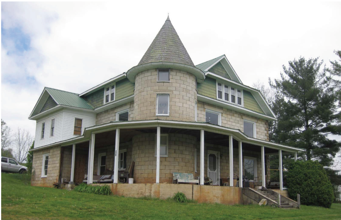
Figure 42. House, Austinville Road (098-5195), south corner.
