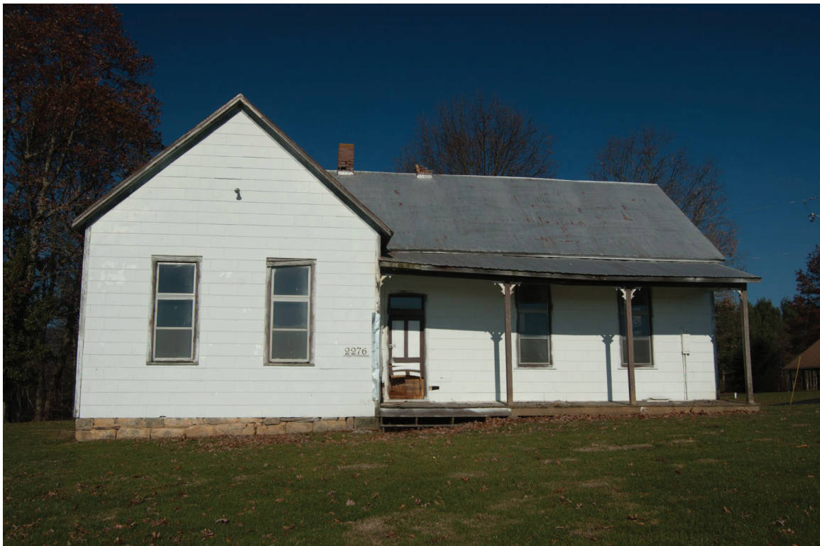
Figure 62. Fairview Elementary School (098-5503), south elevation.
