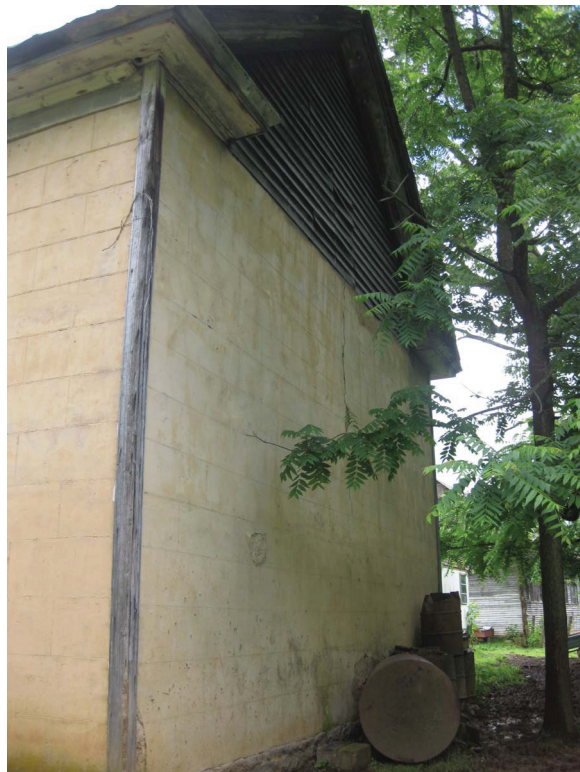
Figure 86. Quaker Meeting House (098-5266), west elevation showing scoring of stucco.
