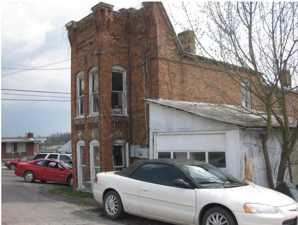
Figure 16. Commercial Building, 121 North Main Street (292-5013) in Rural Retreat, north elevation.
