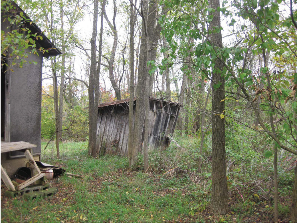
Figure 91. House, 528 Piney Mountain Road (098-5379), poultry house.
