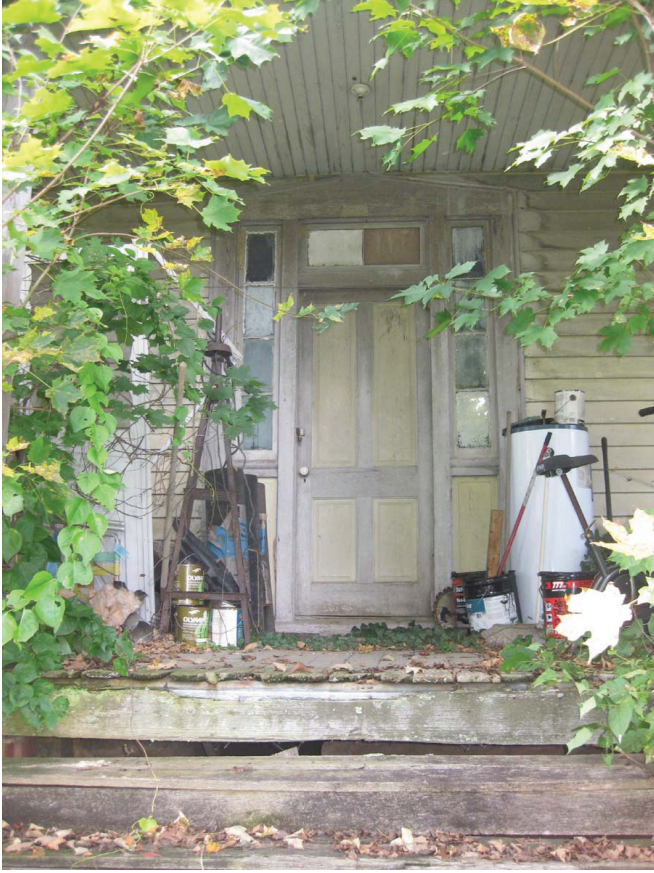
Figure 35. House, Peppers Ferry Road (098-5386), Greek Revival entrance surround.
