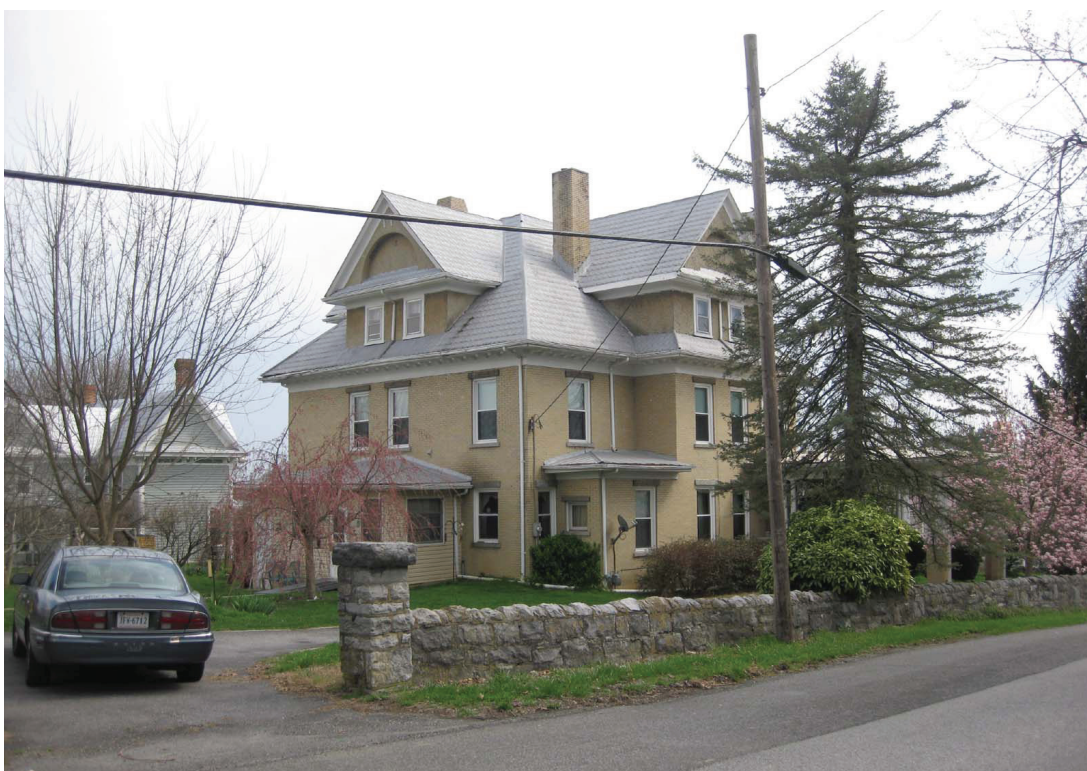
Figure 38 House, 106 Delp Avenue (292-5017), northwest corner.
