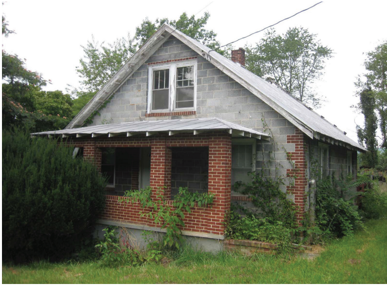
Figure 55. House, Castleton Road (098-5290), south and east elevations.
