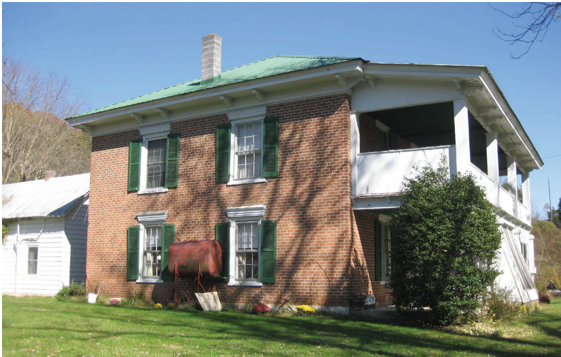
Figure 36. House, 408 Dunford Road (098-5404), southwest corner.
