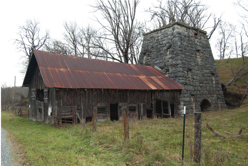
Figure 71. Noble Furnace (098-0040), south and east elevations.
