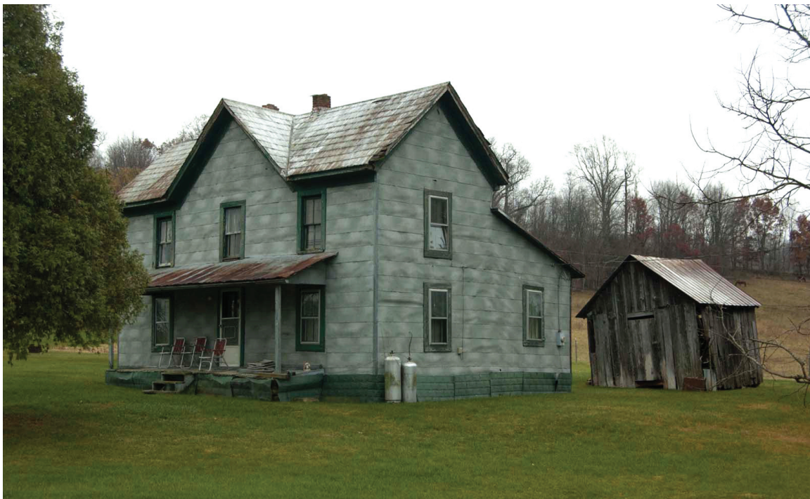
Figure 31. House, Cripple Creek Road (098-5434), south and west elevations.
