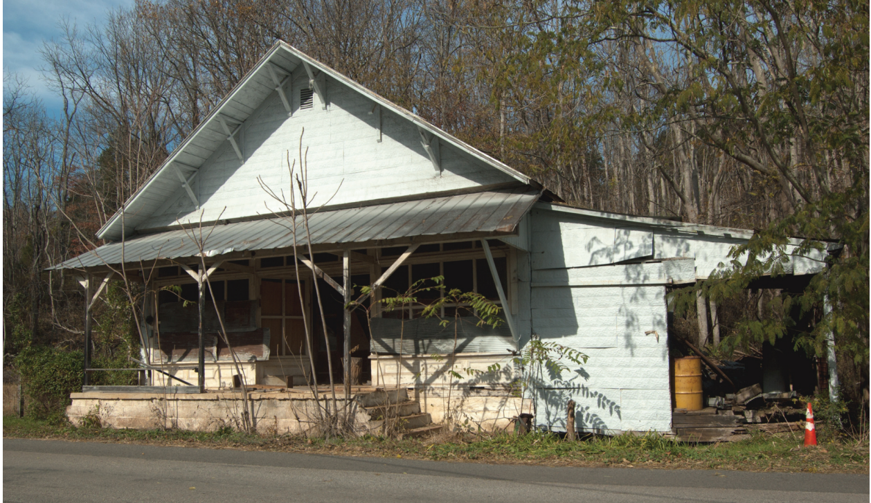
Figure 21. Commercial Building, Pope Road (098-5471), south elevation.
