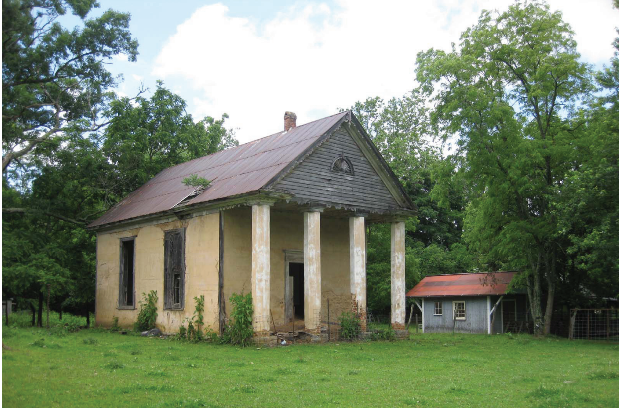
Figure 85. Quaker Meeting House (098-5266), south and east elevations.
