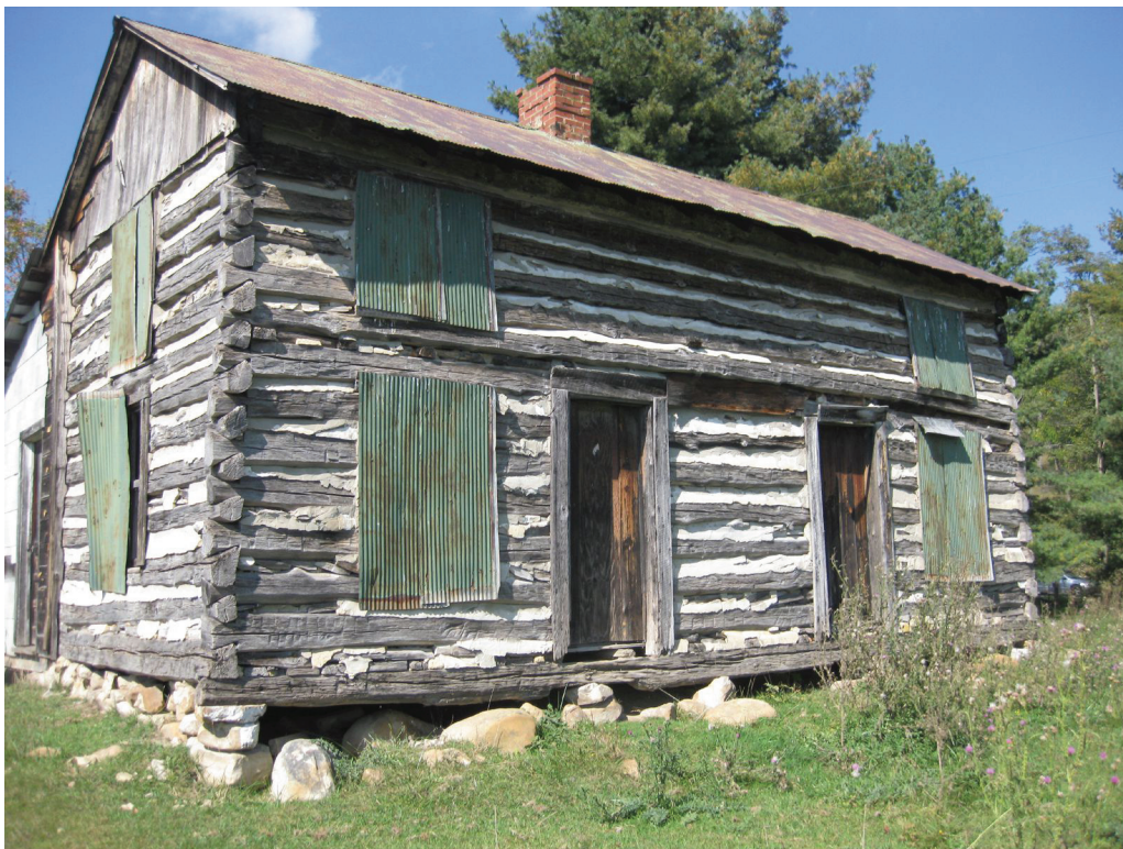
Figure 25. House, Felts Lane (098-5401), east elevation; a rare surviving example of a Wythe County log dwelling with dovetail corner joints.
