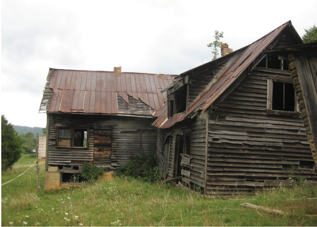
Figure 73. Store/House, Castleton Road (098-5289), west and south elevations.
