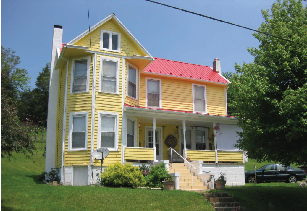
Figure 39. House, 544 Painters Hill Road (098-5244), south elevation.
