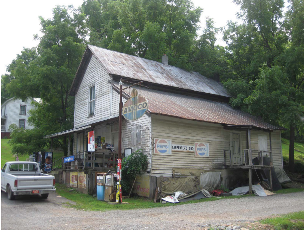
Figure 13. Carpenter's Grocery (098-5302), north and west elevations.
