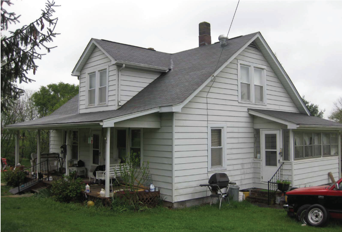
Figure 51. House, 1219 Lead Mine Road (098-5202), southeast corner.
