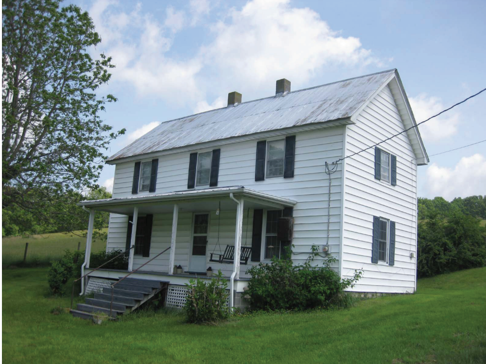
Figure 30. House, 3563 Fairview Parkway (098-5224), southeast corner.
