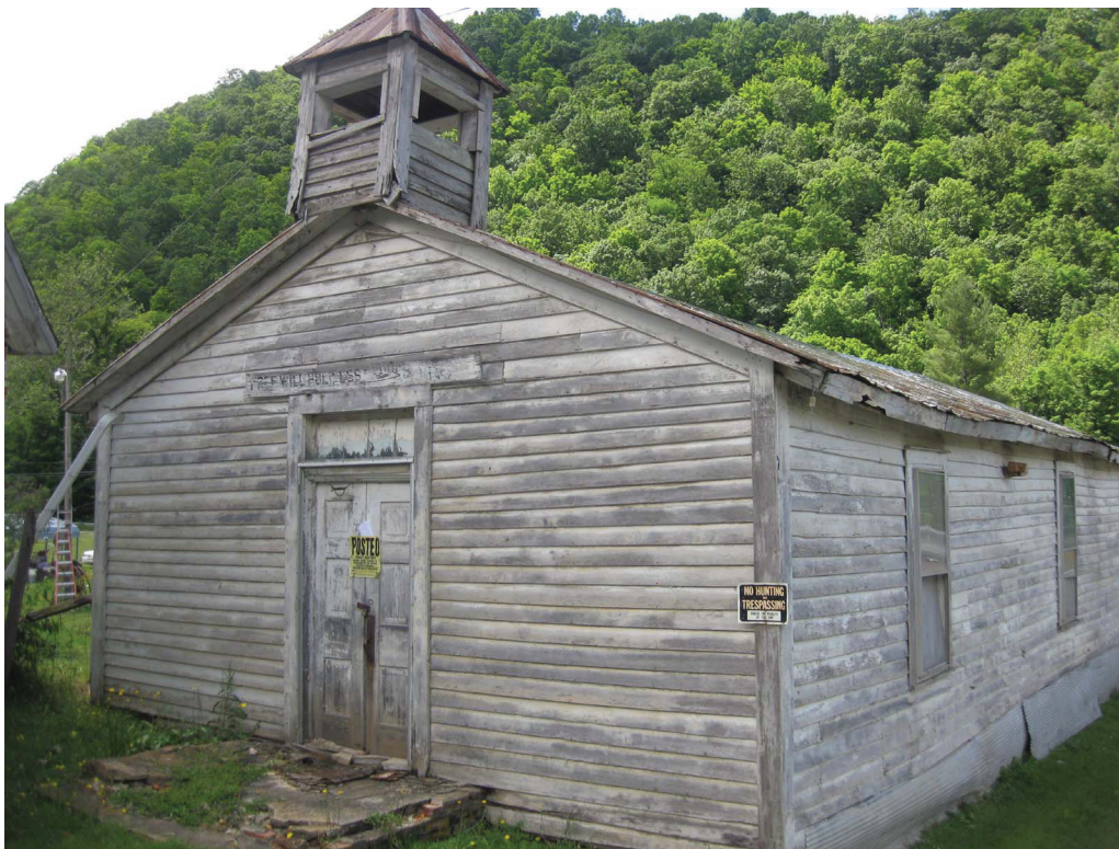
Figure 82. Free Will Holiness Church (098-5269), south and east elevations.
