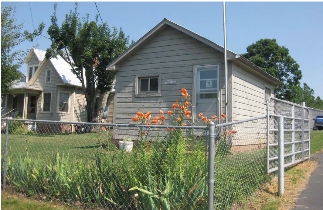
Figure 67. Foster Falls Post Office (098-5300), south and east elevations.
