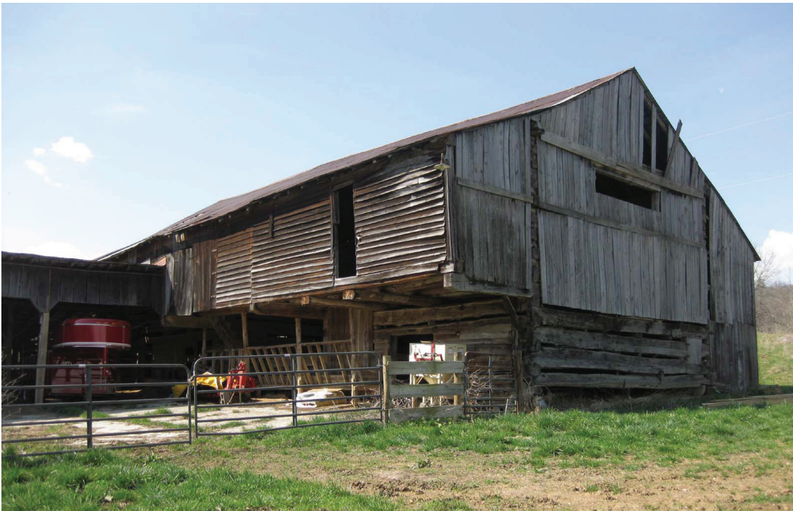
Figure 94. Fracture Creek Farm (098-5190), log barn.
