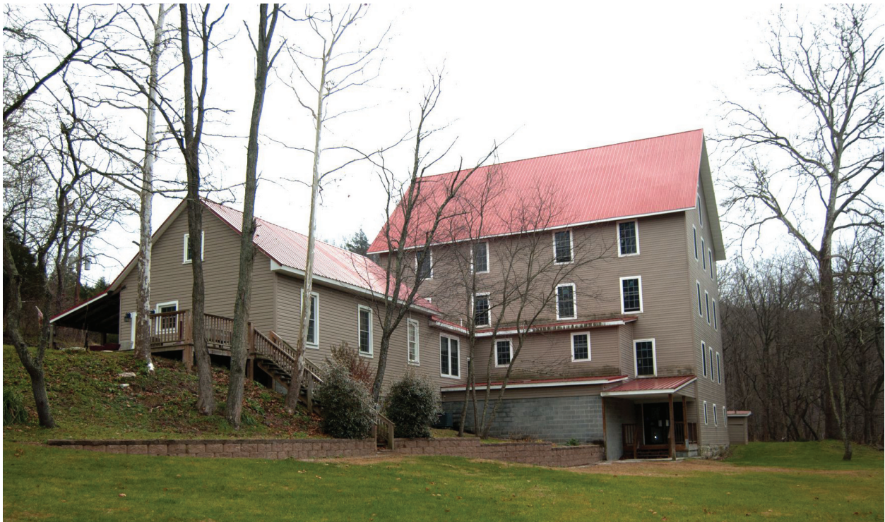
Figure 76. Beverly Mill (098-0050), north and west elevations.
