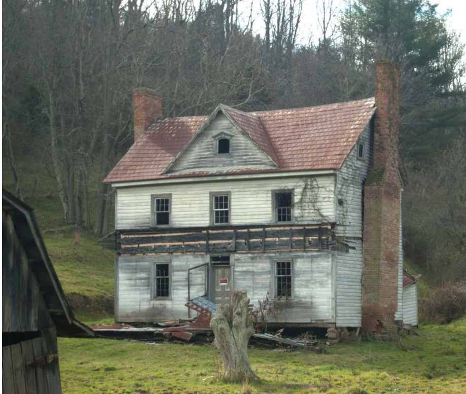
Figure 26. House, Huckleberry Road (098-5496), east and north elevations.
