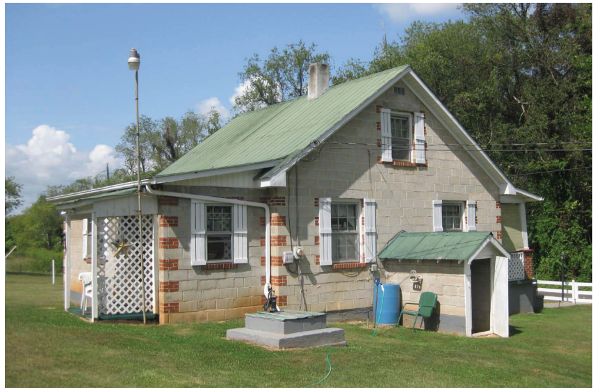
Figure 56. House, 1287 Sanders Mines Road (098-5373), east elevation.
