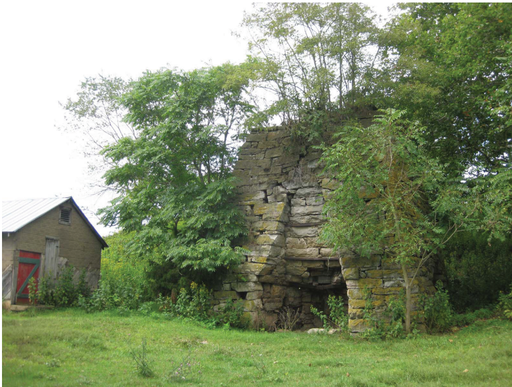
Figure 72. Walton Furnace (098-0044), east elevation.
