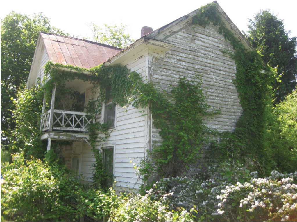
Figure 33. House, 669 Painters Hill Road (098-5240), northwest corner.
