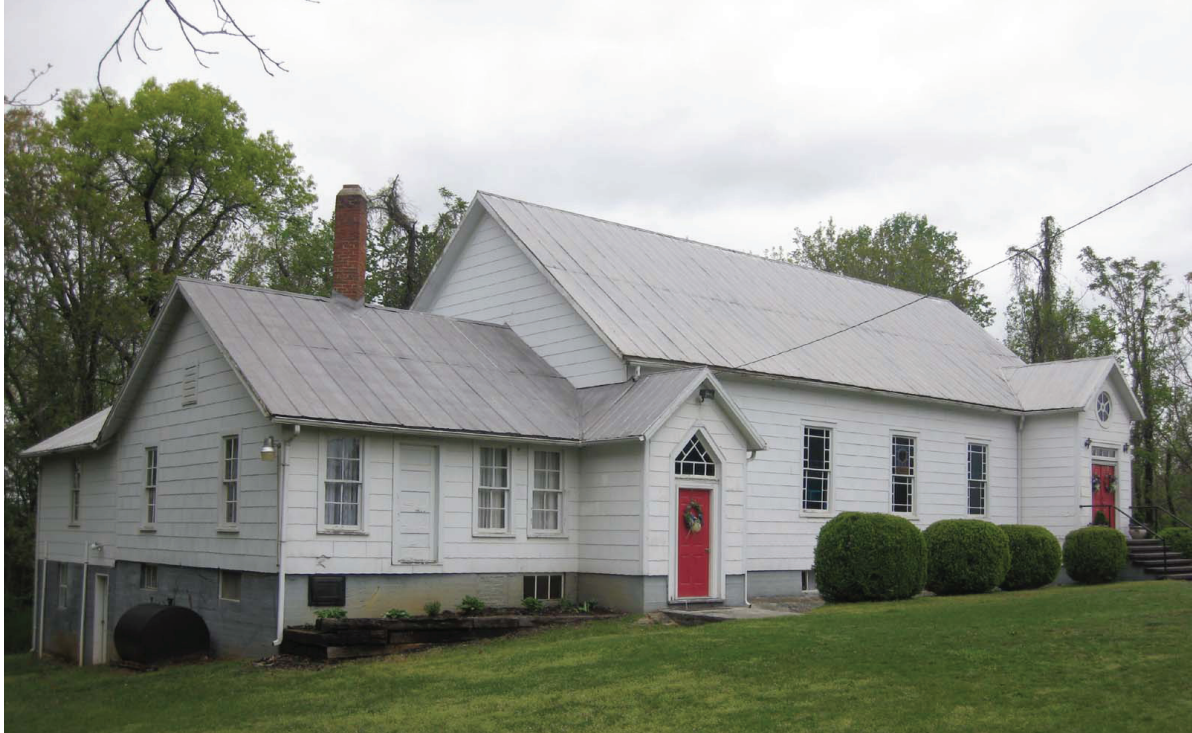
Figure 81. Trinity Church (098-5042-0012), southwest corner.
