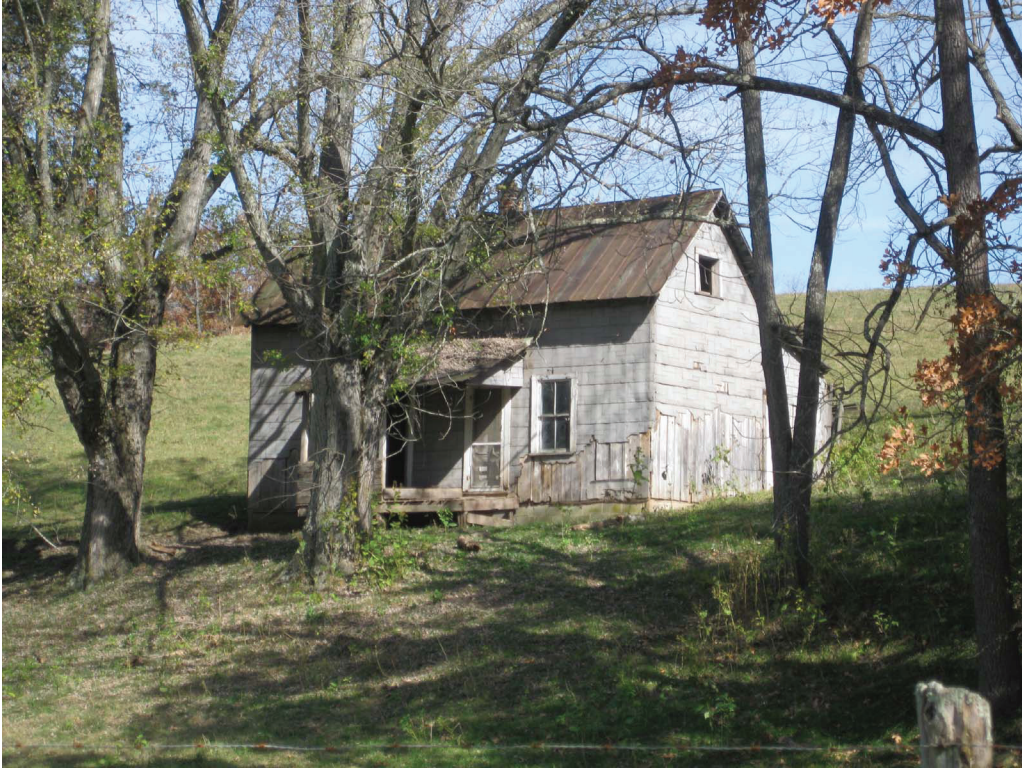
Figure 53. Tenant House, Walton Furnace Road (098-5423), southwest corner.
