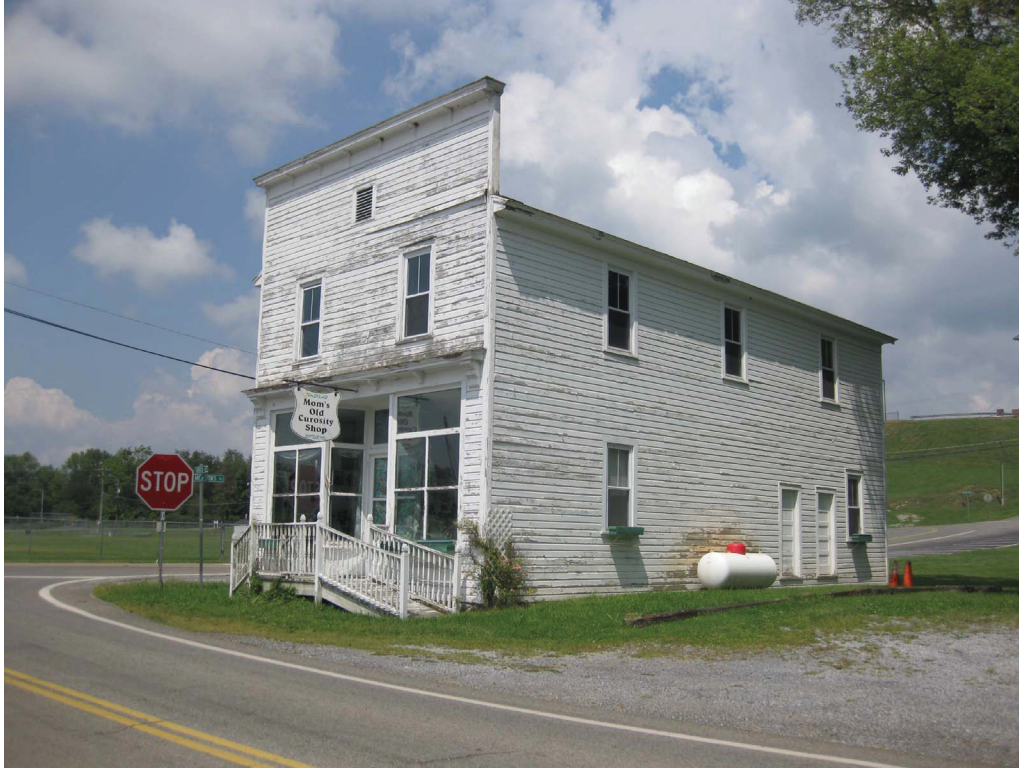
Figure 15. Mom's Old Curiosity Shop (098-5361) in Max Meadows, south and east elevations.
