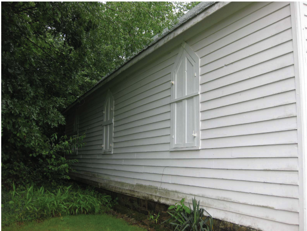
Figure 84. Saint Patrick Catholic Church (098-5257), north elevation.
