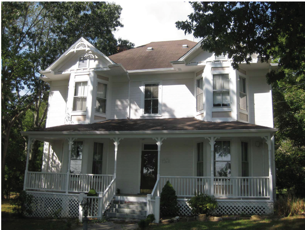
Figure 48. House, 3286 Austinville Road (098-5366), east elevation.
