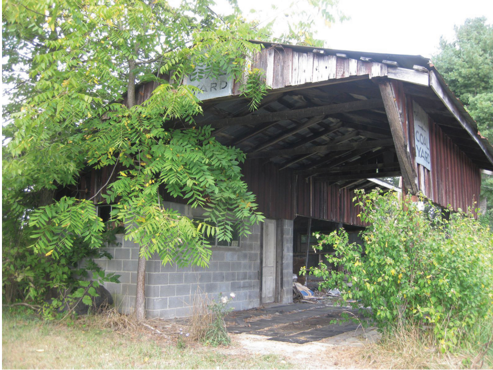
Figure 74. Thompson Coal Yard (098-5370), southeast corner.
