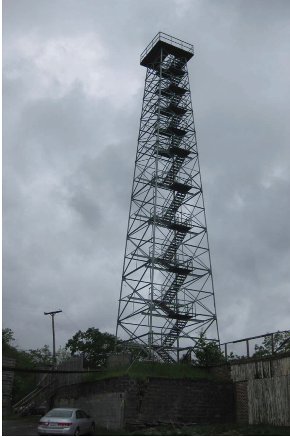
Figure 77. Big Walker Lookout Tower (098-5209), northeast corner.
