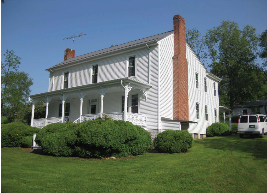
Figure 28. House, 1702 Crocketts Cove Road (098-5217), southeast corner.
