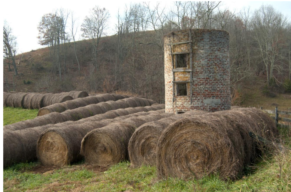
Silo Kiser Road
