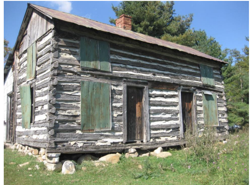
Log House Felts Lane
