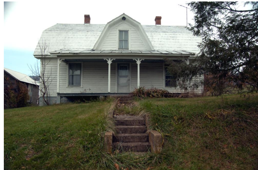
Colonial Revival Farm, Cripple Creek Road
