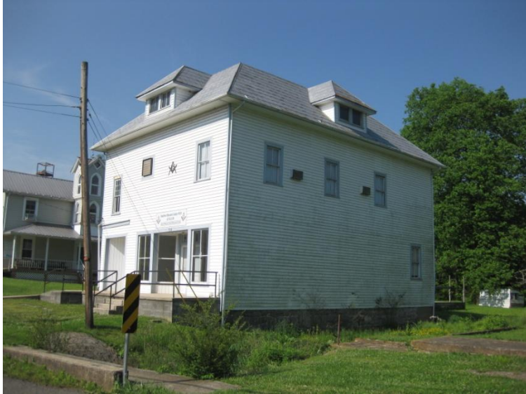
Lodge, Painters Hill Rd
