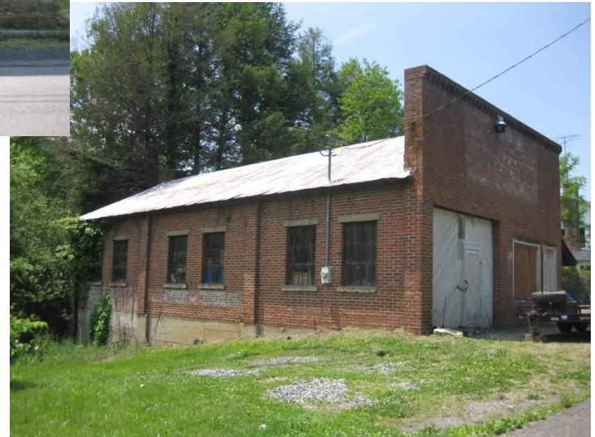
Commercial Building, Painters Hill Rd
