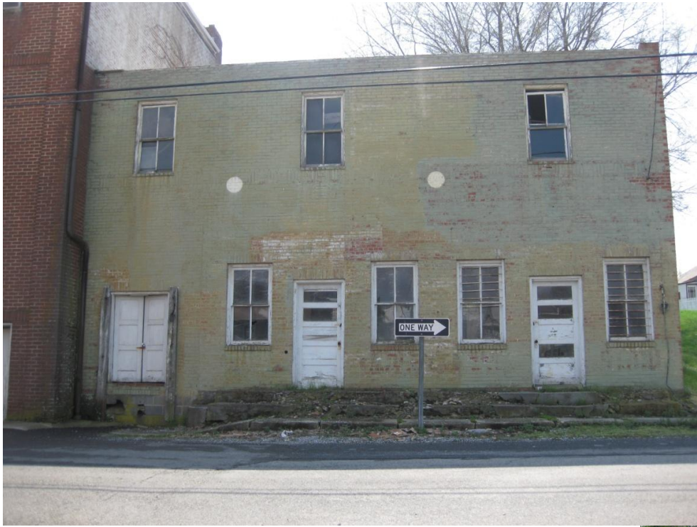
Commercial Building Baumgardner Ave
