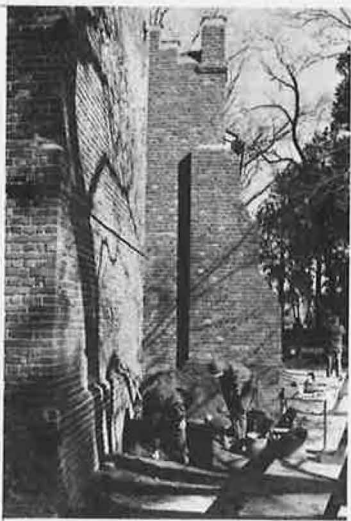
Test Trench at Jamestown Church Tower
