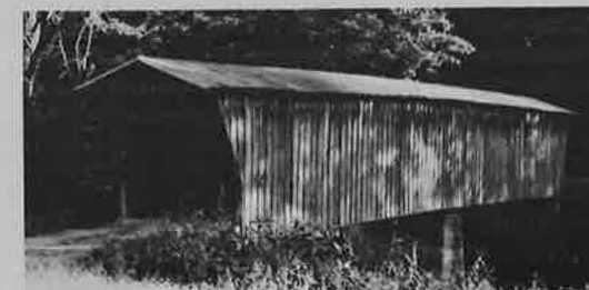
Bob White Covered Bridge, Patrick County
