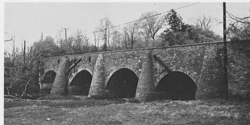
"Goose Creek Stone Bridge, Loudoun County"
