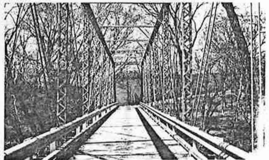
"Catoctin Creek Bridge"
