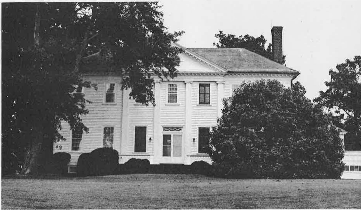
Rappahannock River facade of NANZATICO, King George County. Easement recorded 1972
