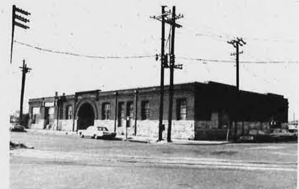
Byrd Street as a Freight Station, Richmond
