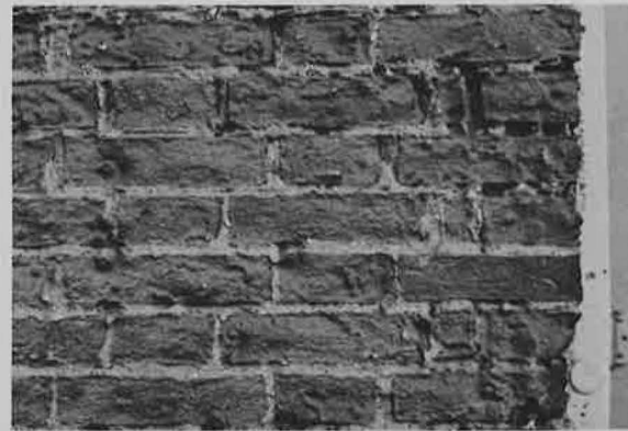
Early-nineteenth-century brickwork that has been sandblasted, after approximately ten years of weathering.
