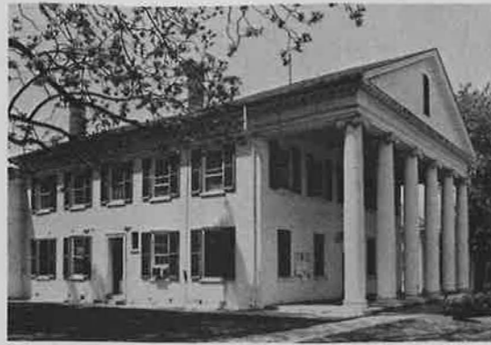
MECKLENBURG COUNTY COURTHOUSE: The temple-form brick court building follows a pattern set for the antebellum Piedmont by Thomas Jefferson. It was built in 1838-1842 by William A. Howard and enjoys the standard complementary structures, set in a shaded square.
