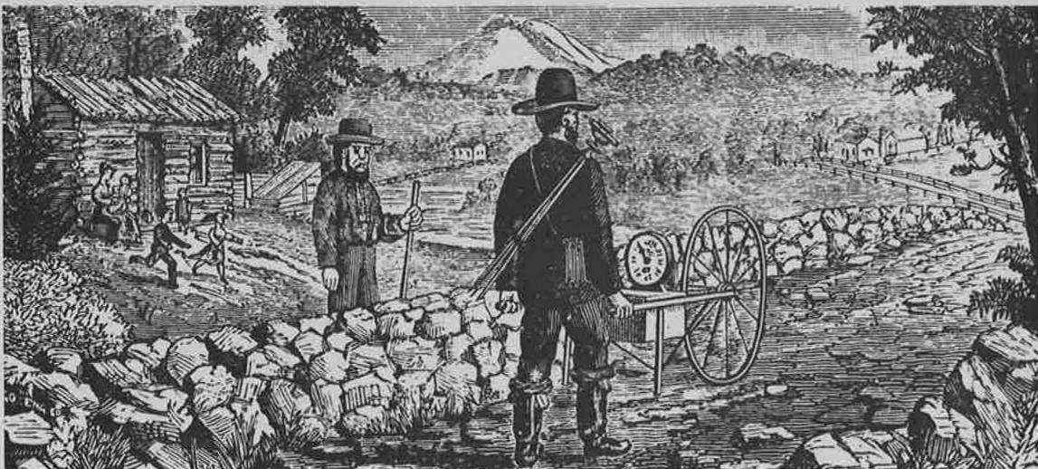
This illustration from Bates Harrington's How Tis Done (1879) shows a county map-maker of the period, with the essential tools of his trade, odometer, compass, and surveyor's transit.
